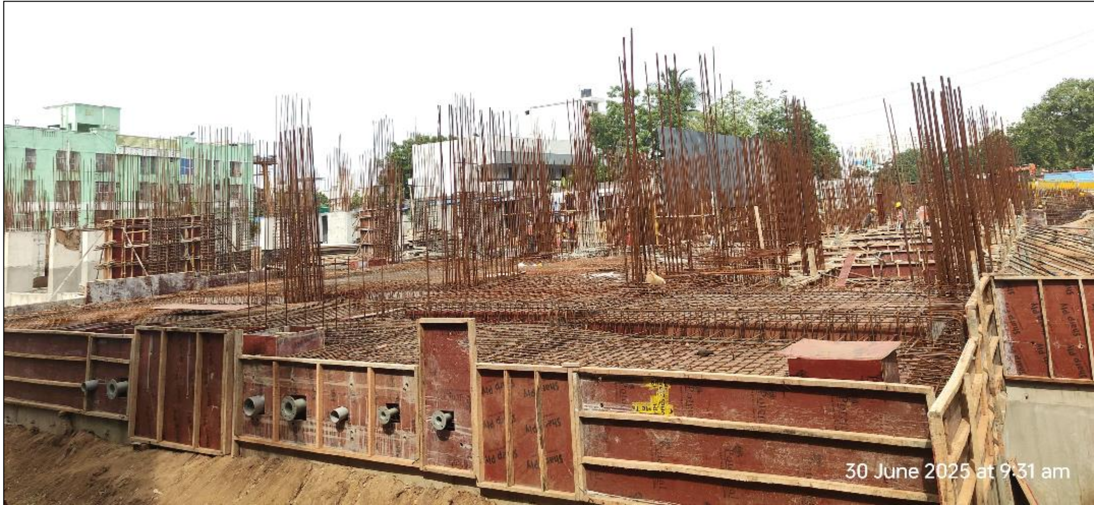
UG sump top slab reinforcement & shuttering work in progress
