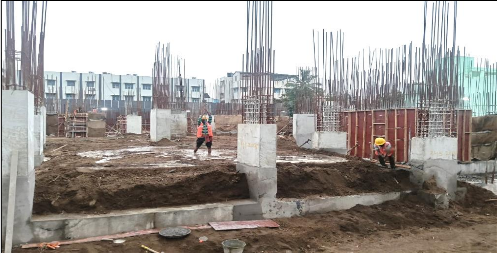
Main building – Pour 01 soil consolidation work in progress
