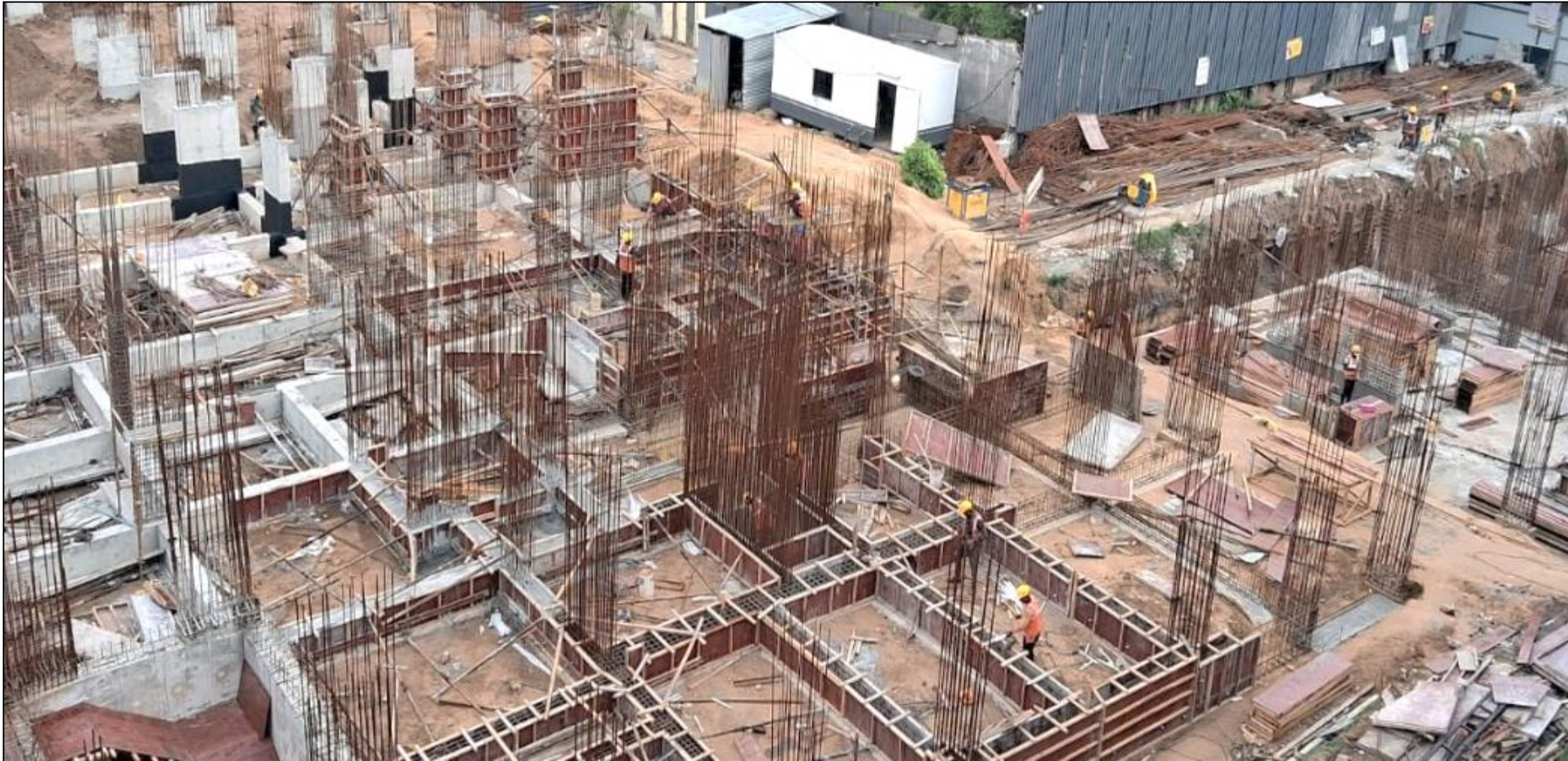
Main building – Pour 04 plinth beam shuttering work in progress
