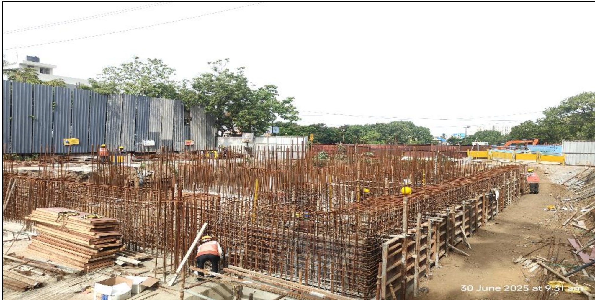
STP – 2 nd lift wall shuttering work completed
