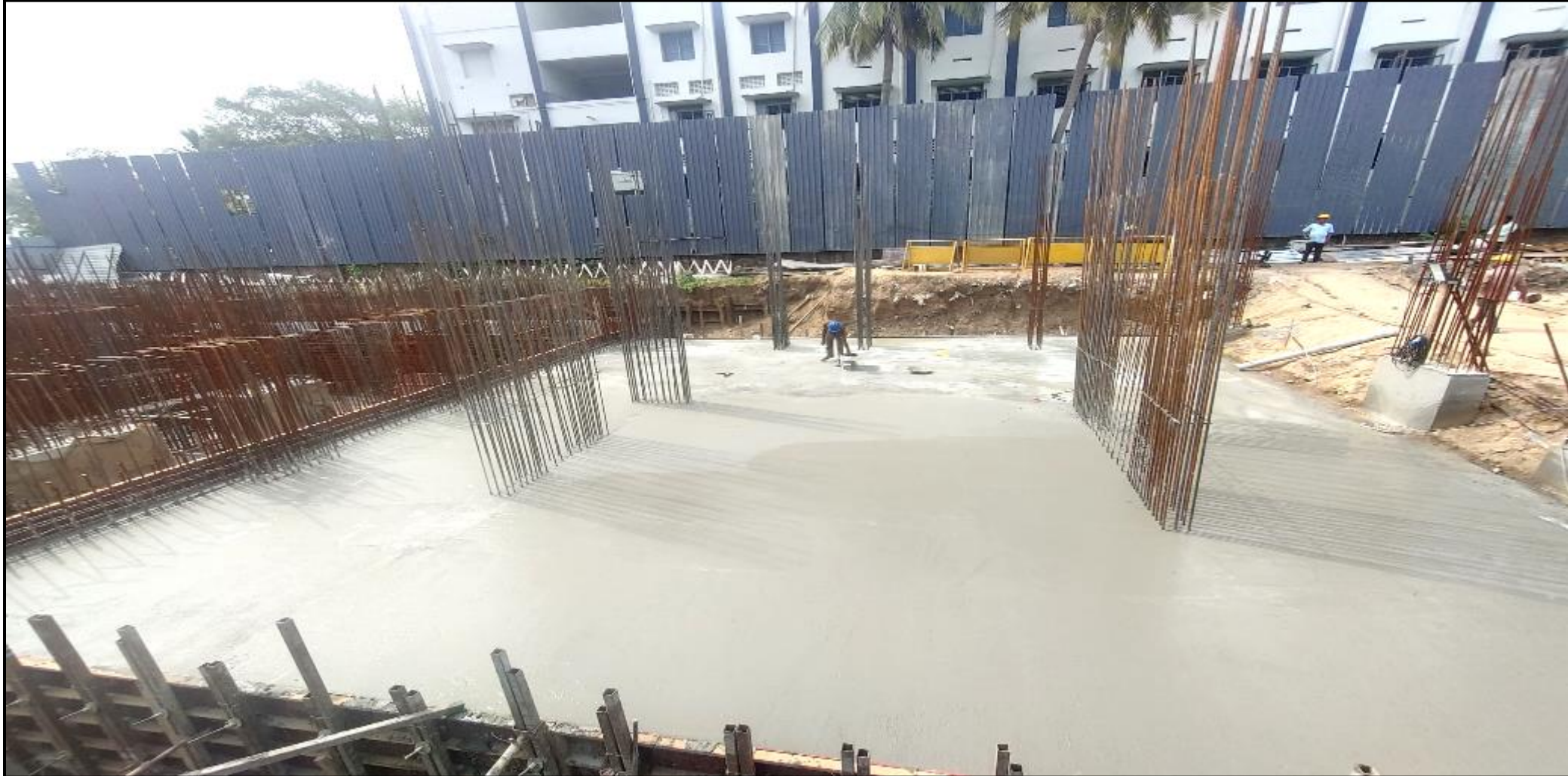
Main building – Pour 04 & Pour 5 joining area raft shuttering & concrete work completed.
