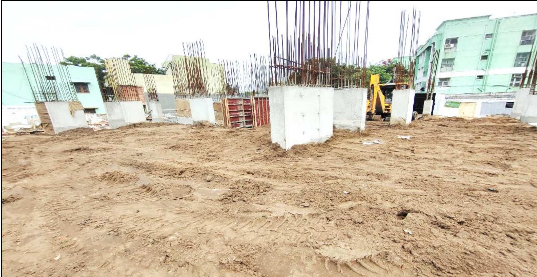
Main building – Pour 01 back filling work in progress
