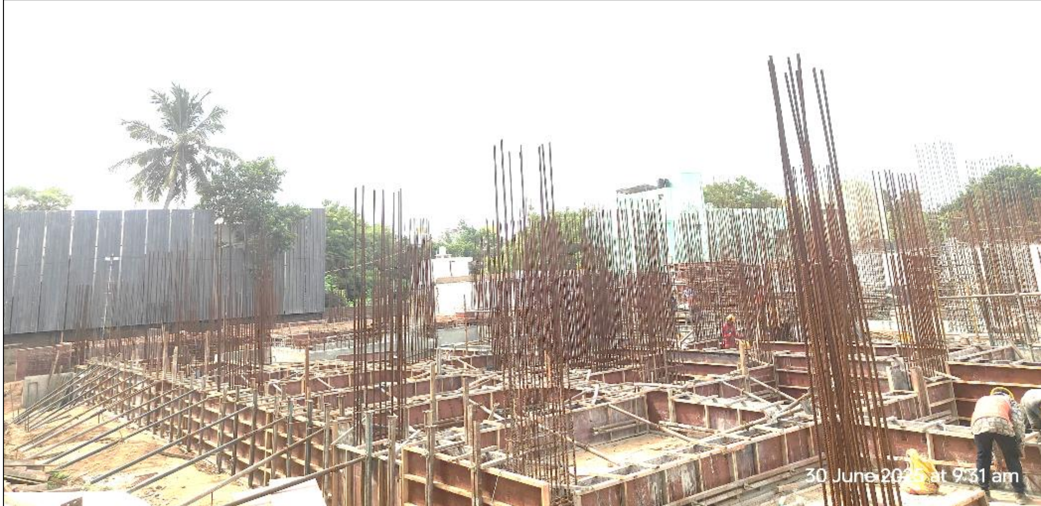
Main building – Pour 04 plinth beam concrete work in progress.
