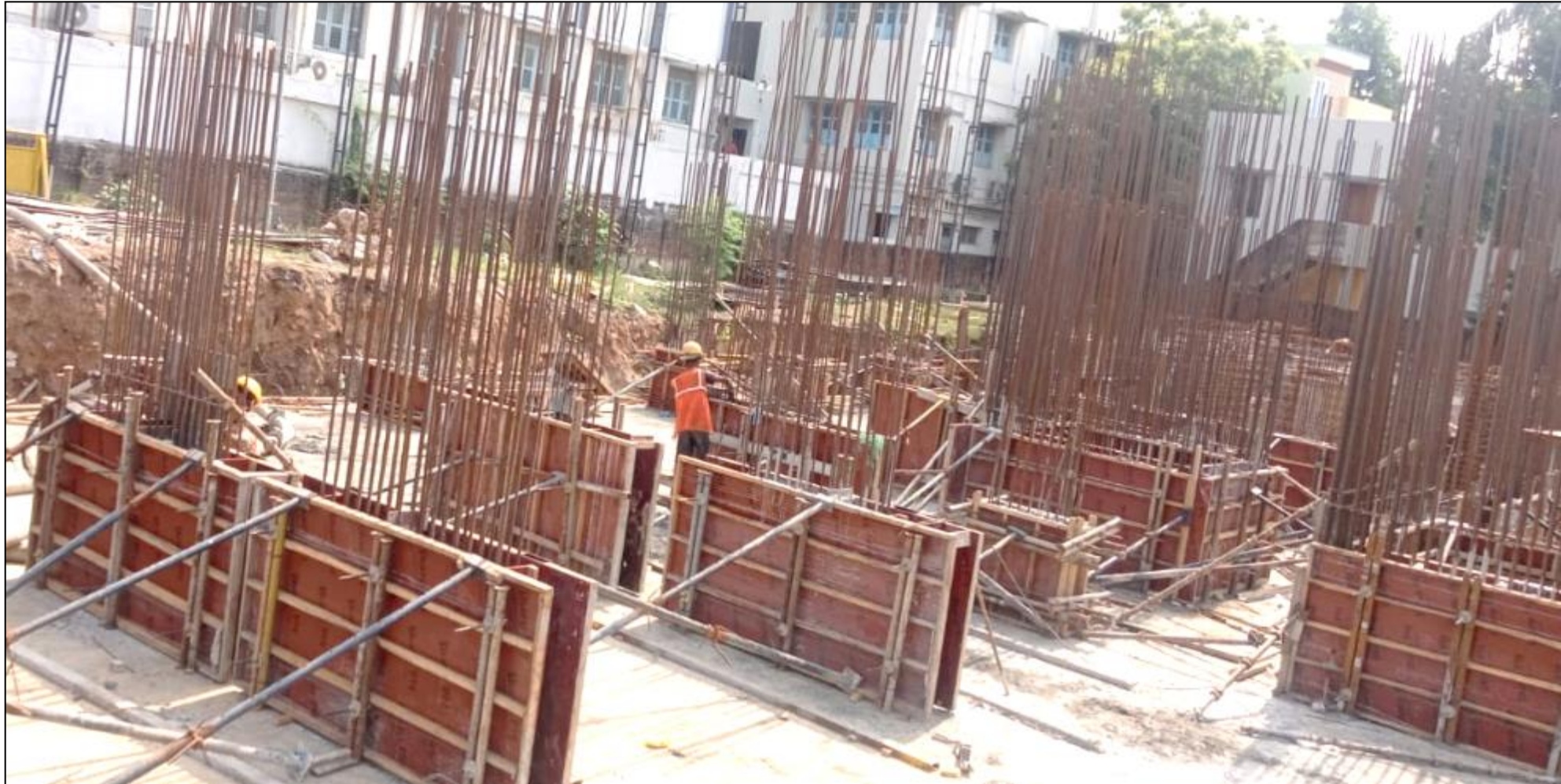
Main building – Pour 04 pedestal column concrete work completed.
