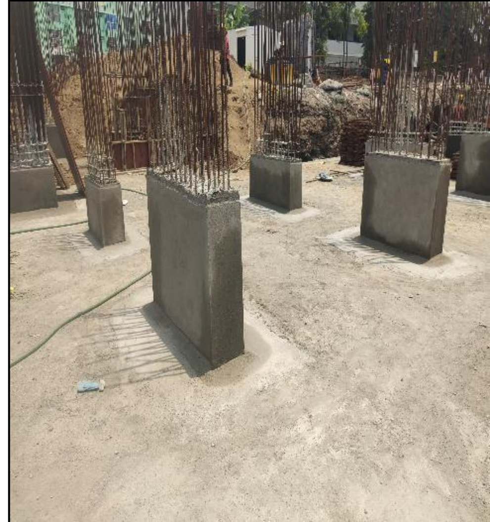
Main building – Pour 03 & 04 pedestal column DPC work completed
