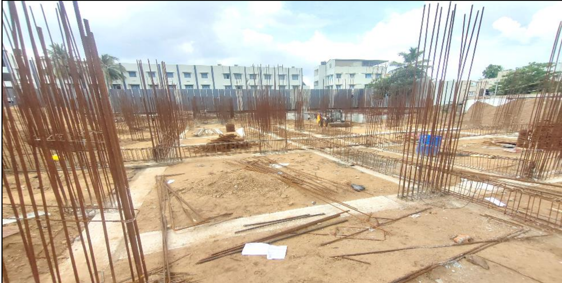
Main building – Pour 02 plinth beam reinforcement work in progress
