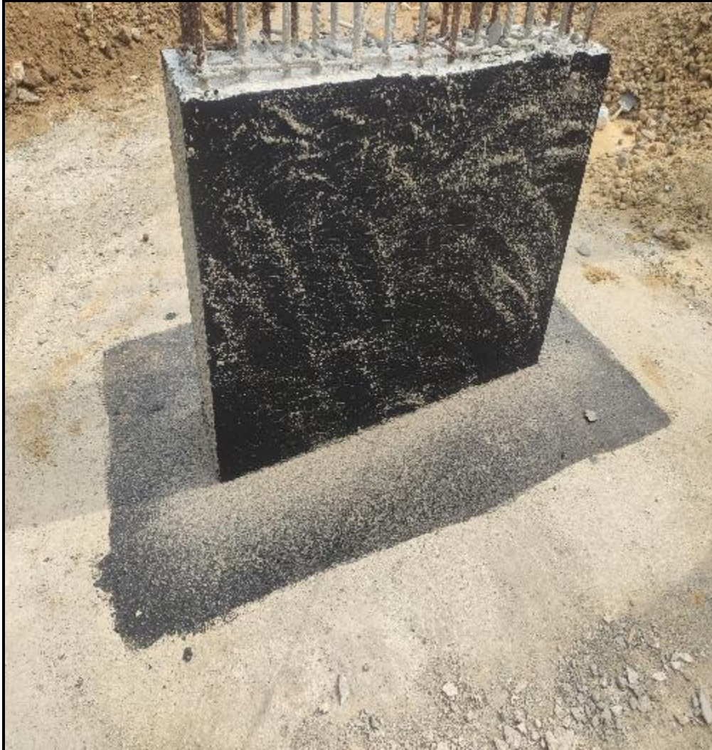
Main building – Pour 03 & 04 pedestal column DPC work completed
