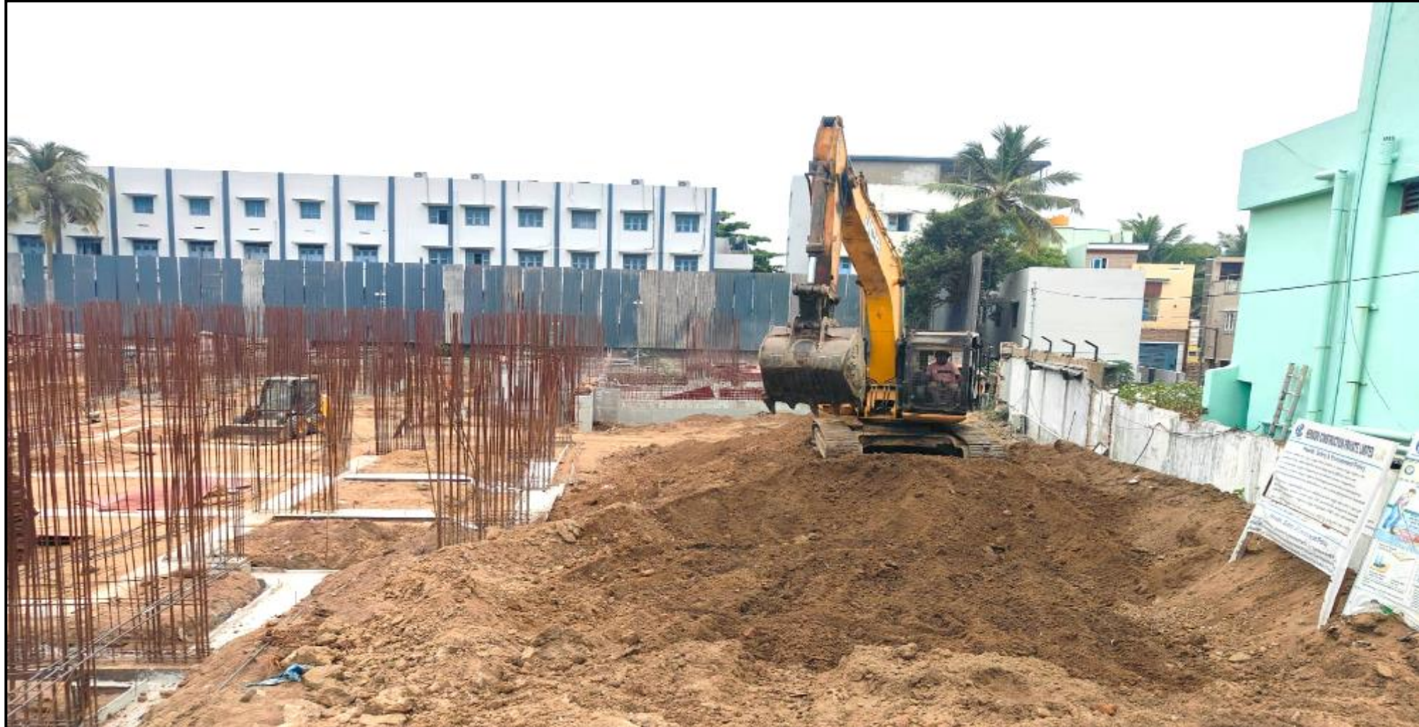
Setback area soil levelling work in progress
