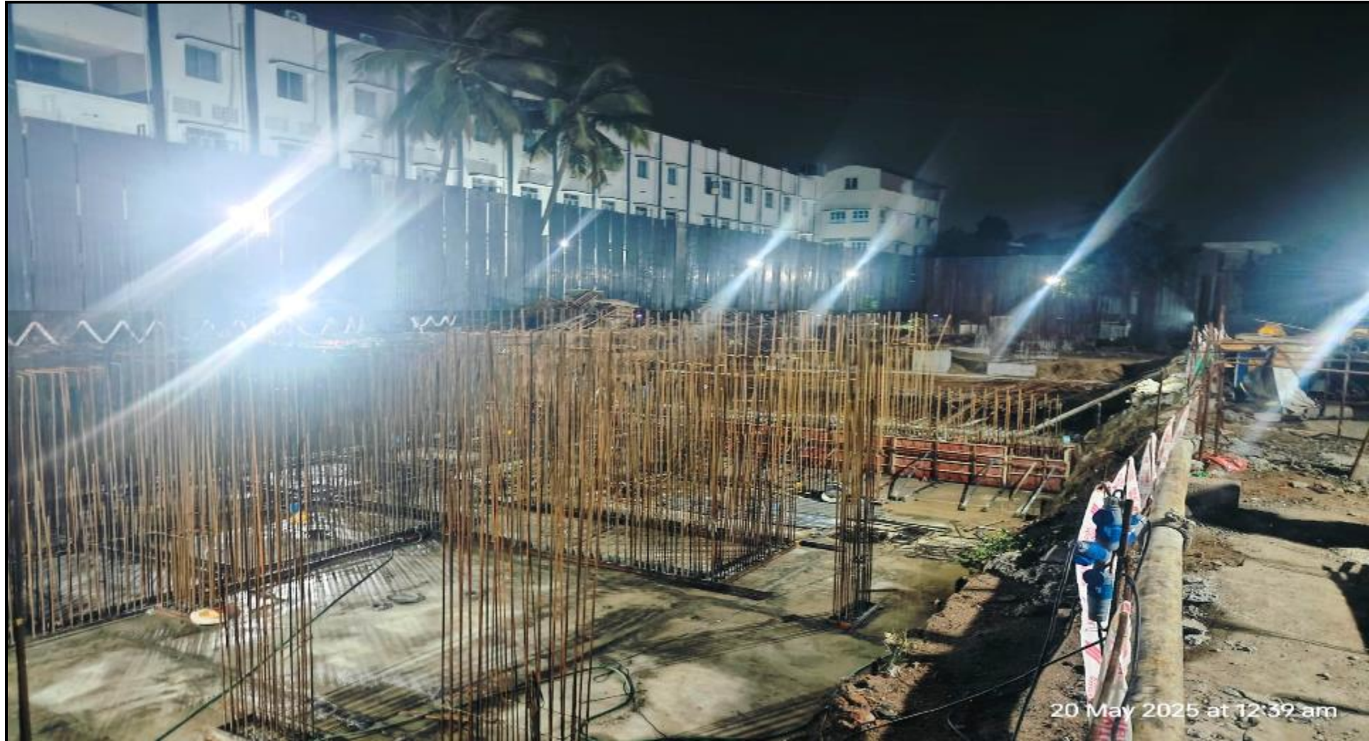
STP – Column & wall reinforcement work in progress
