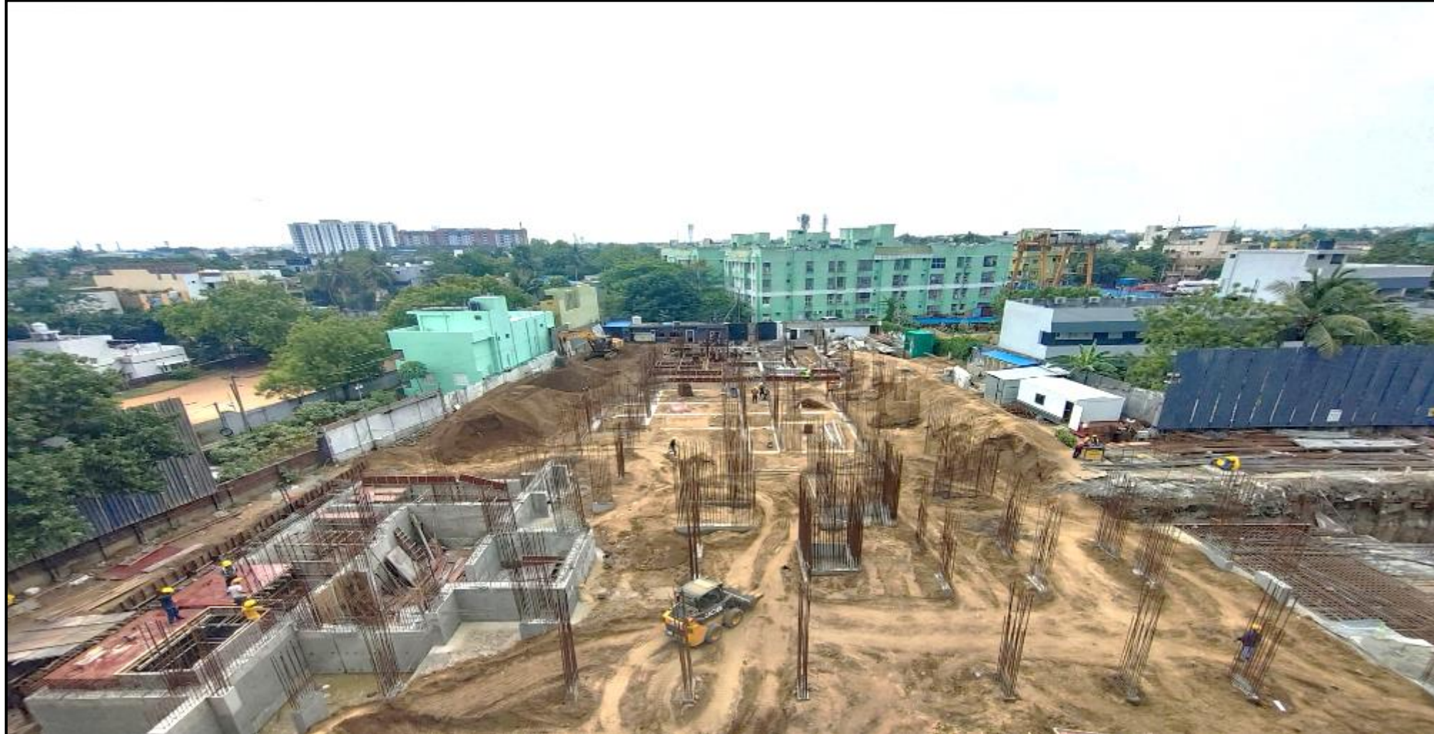
Main building – Pour 04 soil back filling work completed
