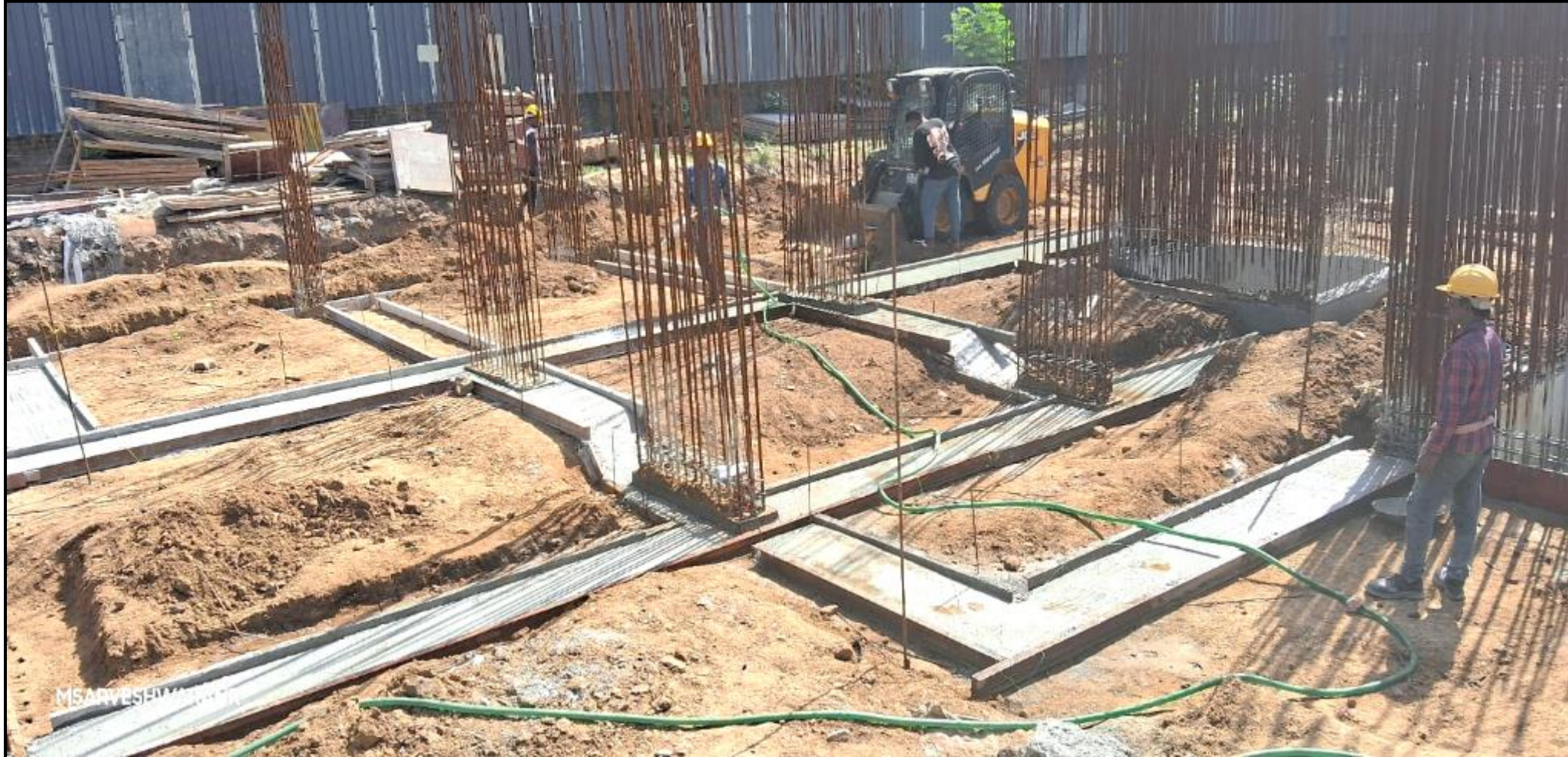
Main building – Pour 04 plinth beam pcc work in progress
