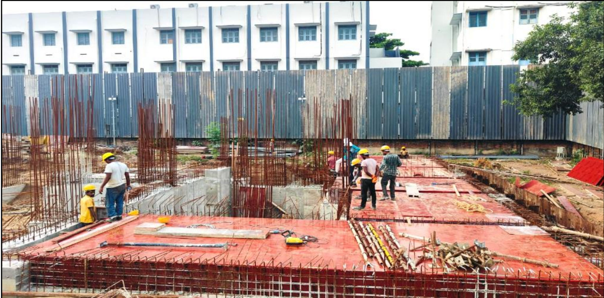
UG Sump – Cover slab shuttering work in progress
