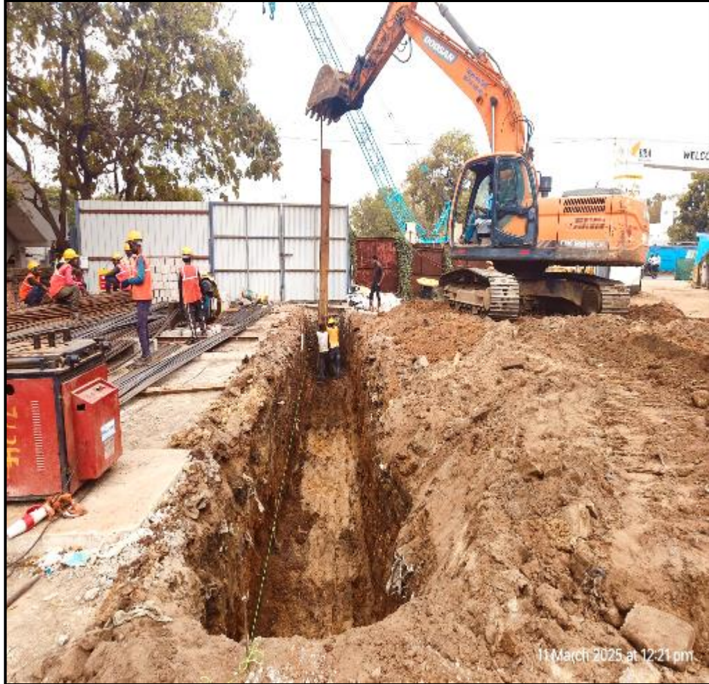
STP Shoring work in progress
