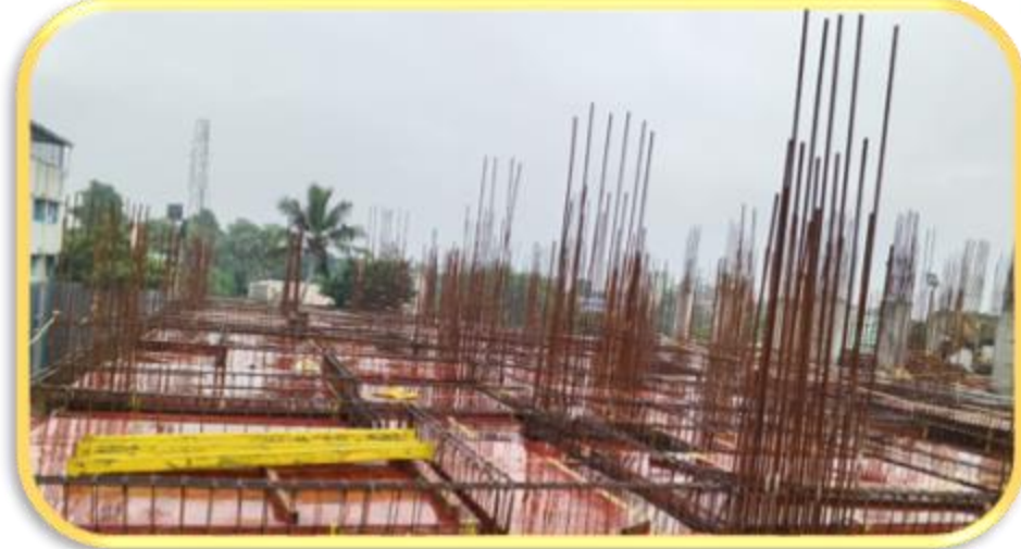
Main building – Pour 2 – 1 st floor roof slab beam reinforcement work
