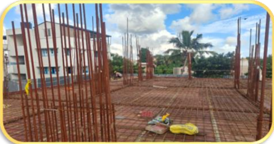
Main building – Pour 2 – 1 st floor roof slab reinforcement work
