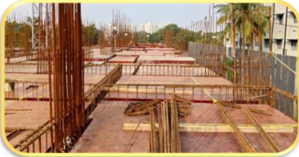
Main building – Pour 2 – 1 st floor roof slab shuttering work
