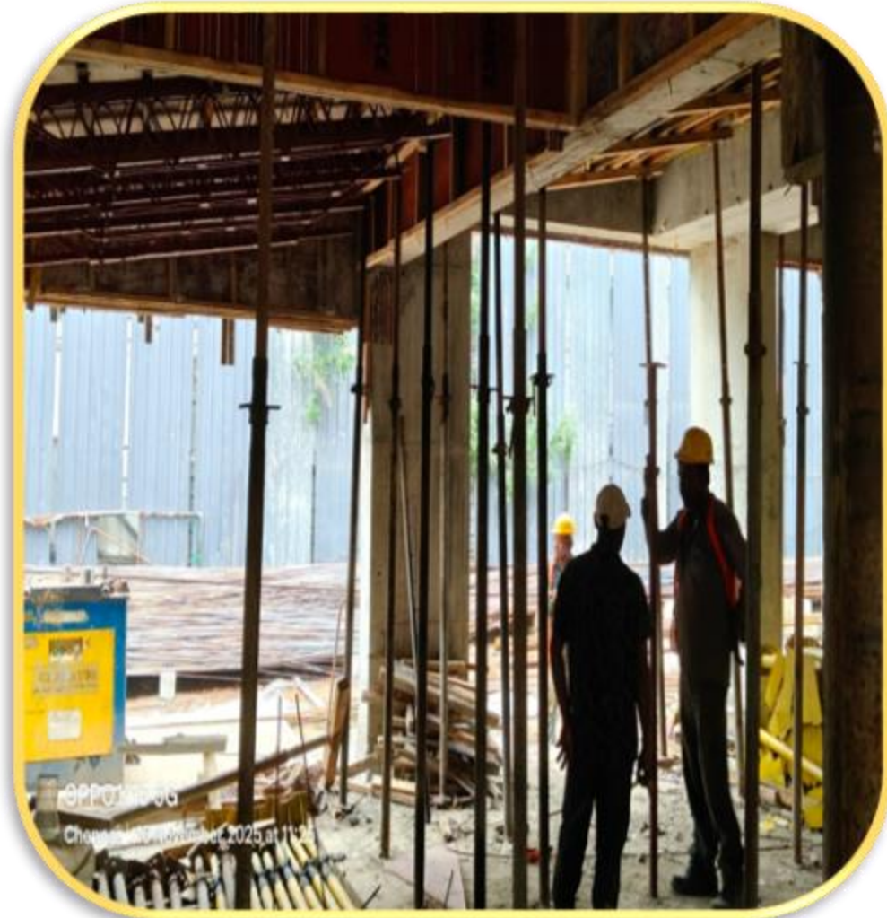
Main building – Pour 2 – Stilt floor roof slab de-shuttering work
