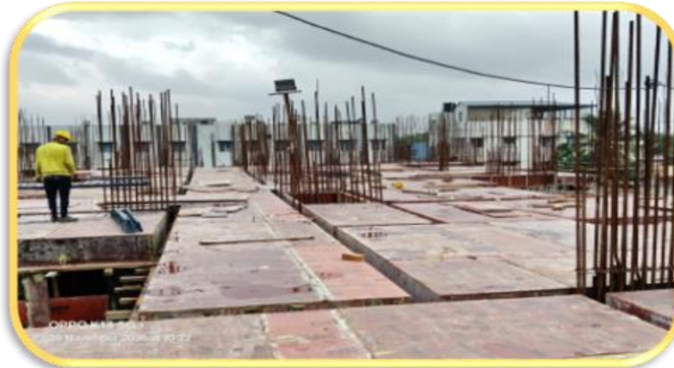
Main building – Pour 1 – 2 nd floor roof slab shuttering work in progress.
