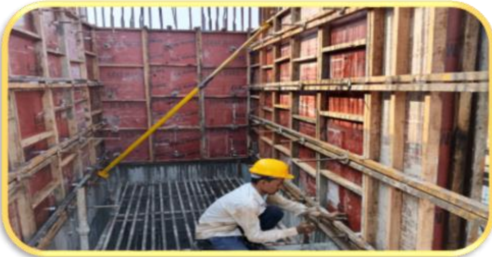
Main building – Pour 1 – 2 nd floor column & lift shuttering completed (57 Nos / 57 Nos) .
