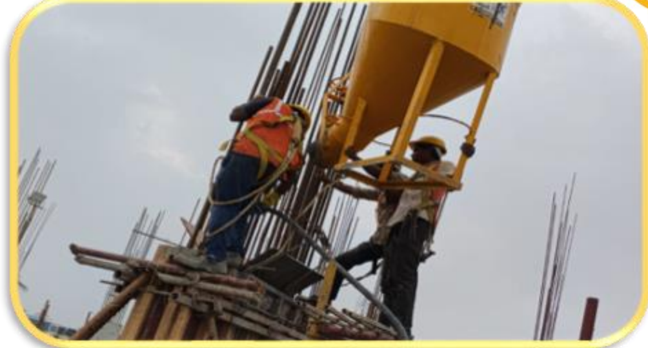
Main building – Pour 1 – 2 nd floor slab column concrete completed (57 Nos / 57 Nos)
