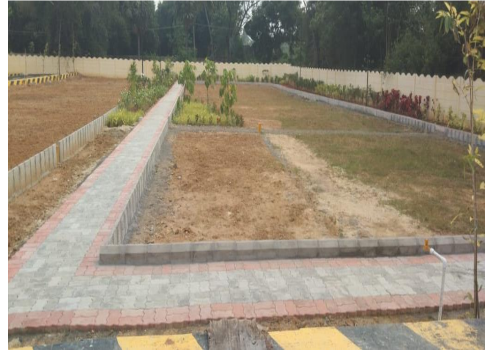
PARK PATHWAY PAVER BLOCK & KERB STONE LAYING WORK
