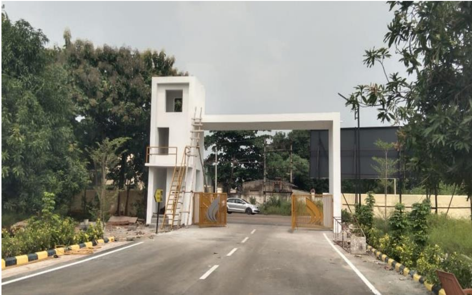
ENTRANCE ARCH GATE & STAIRCASE PRIMER WORK COMPLETED
