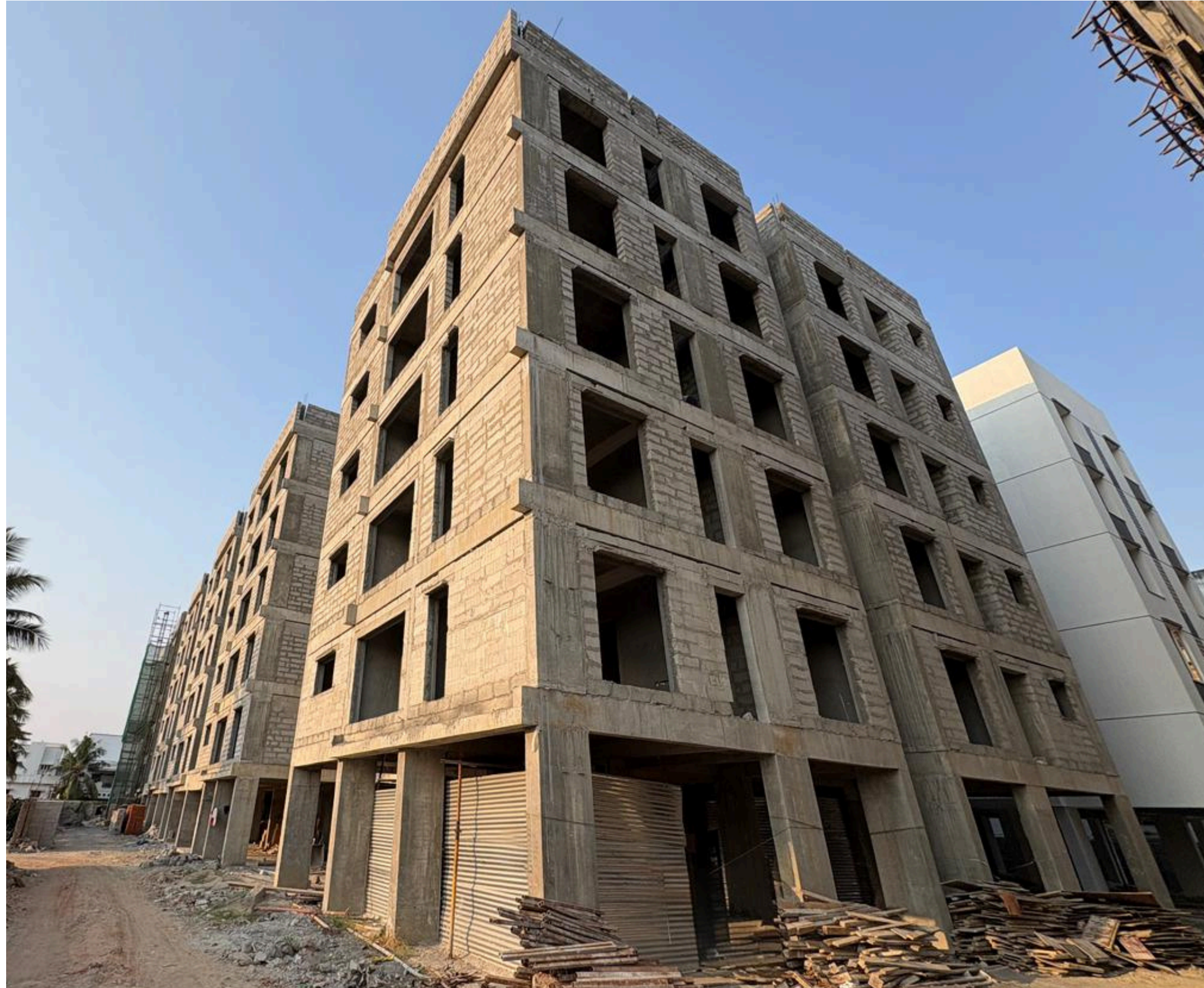
Block-02 – Elevation View
