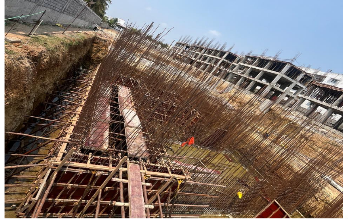
Block-1-STP Wall Shuttering Work in Progress
