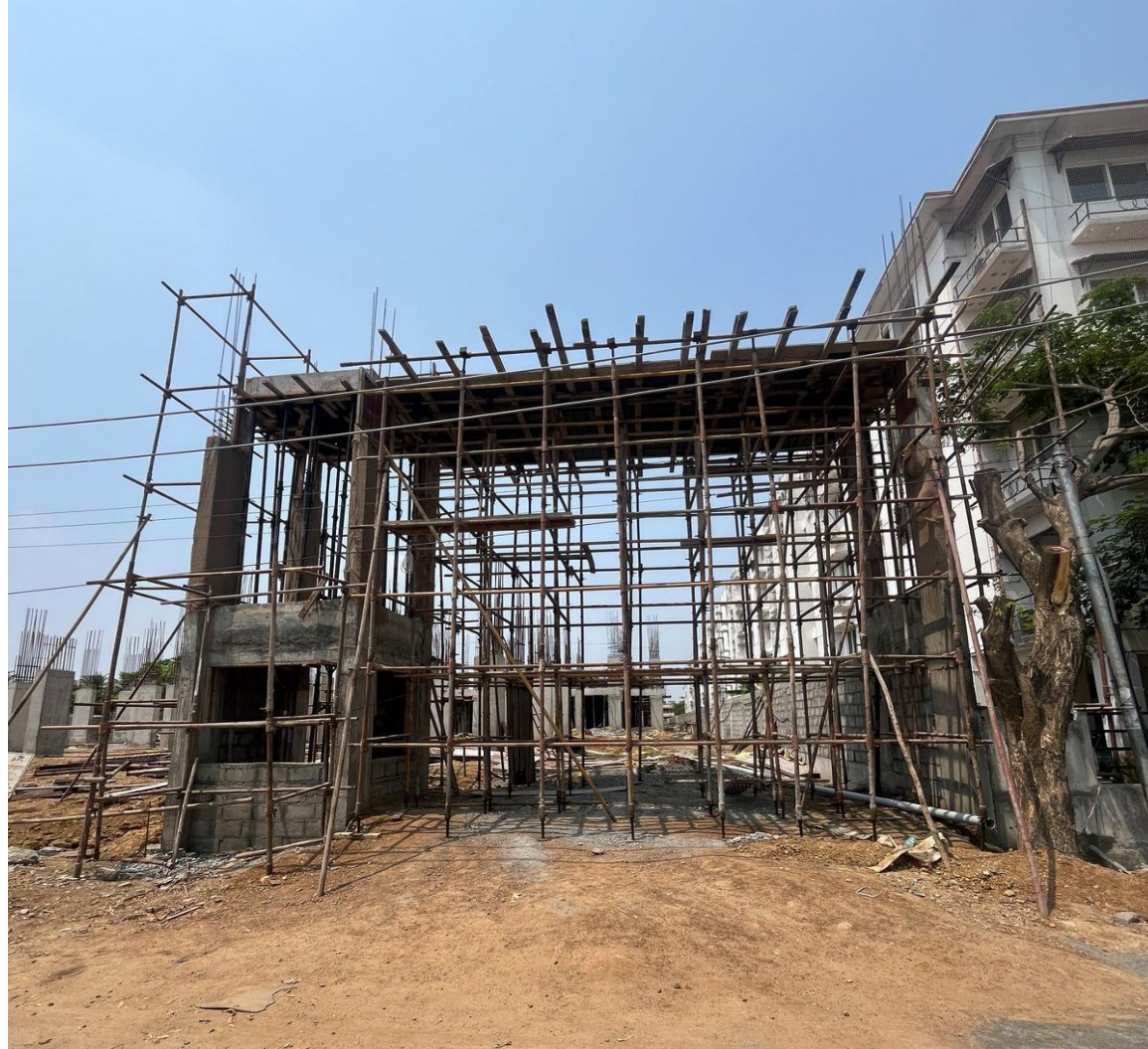
Exit Arch Slab Shuttering Work in Progress
