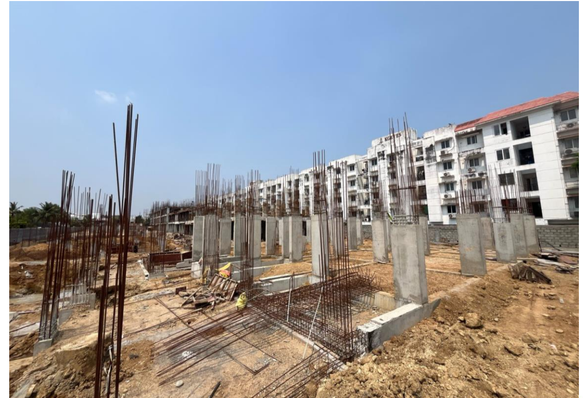
Block-1-Pour 1 – Footing PCC & Plinth Beam Concrete Work in Progress
