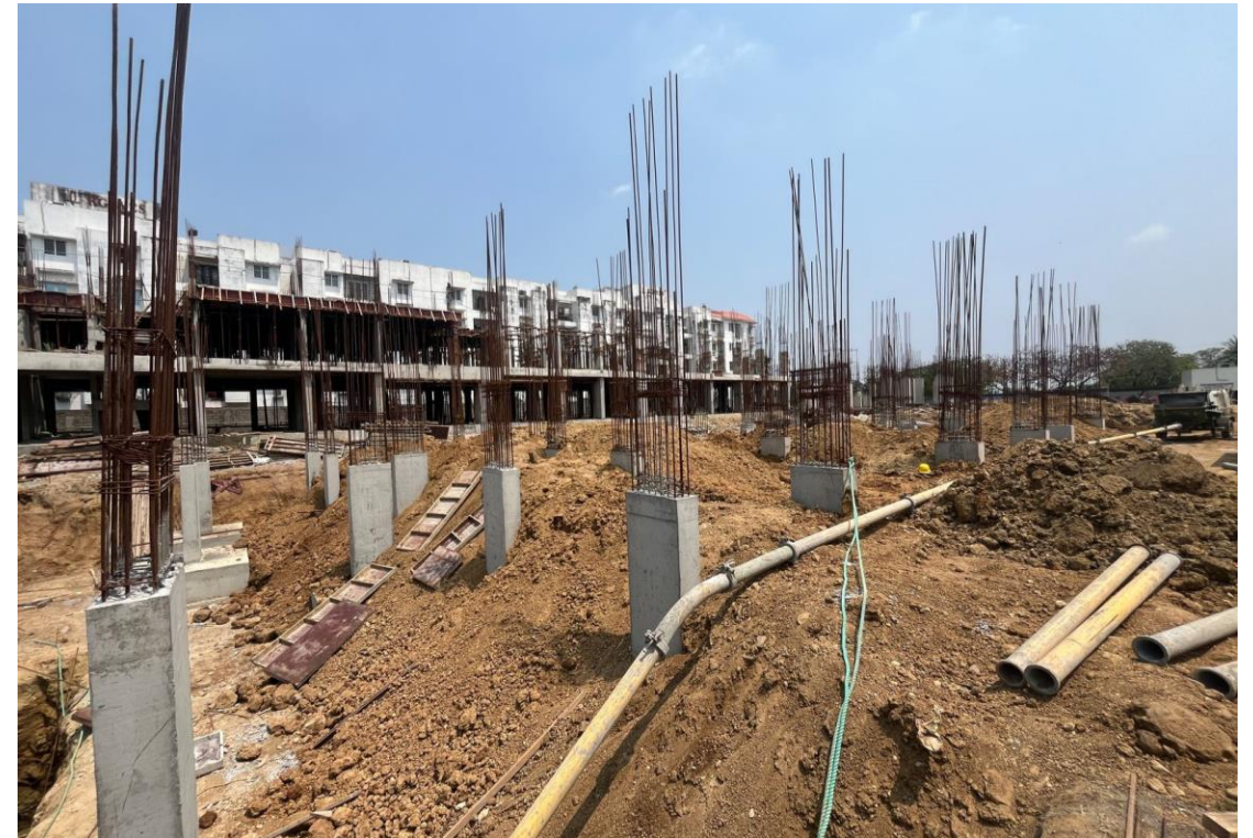
Block-1-Pour 2 Back Filling Work in Progress
