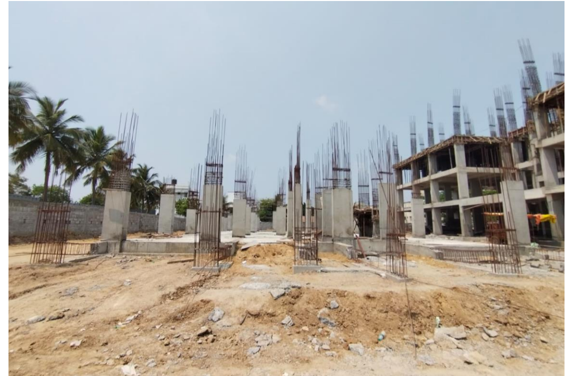
Block-2-Pour 2-Stilt PCC Work in Progress
