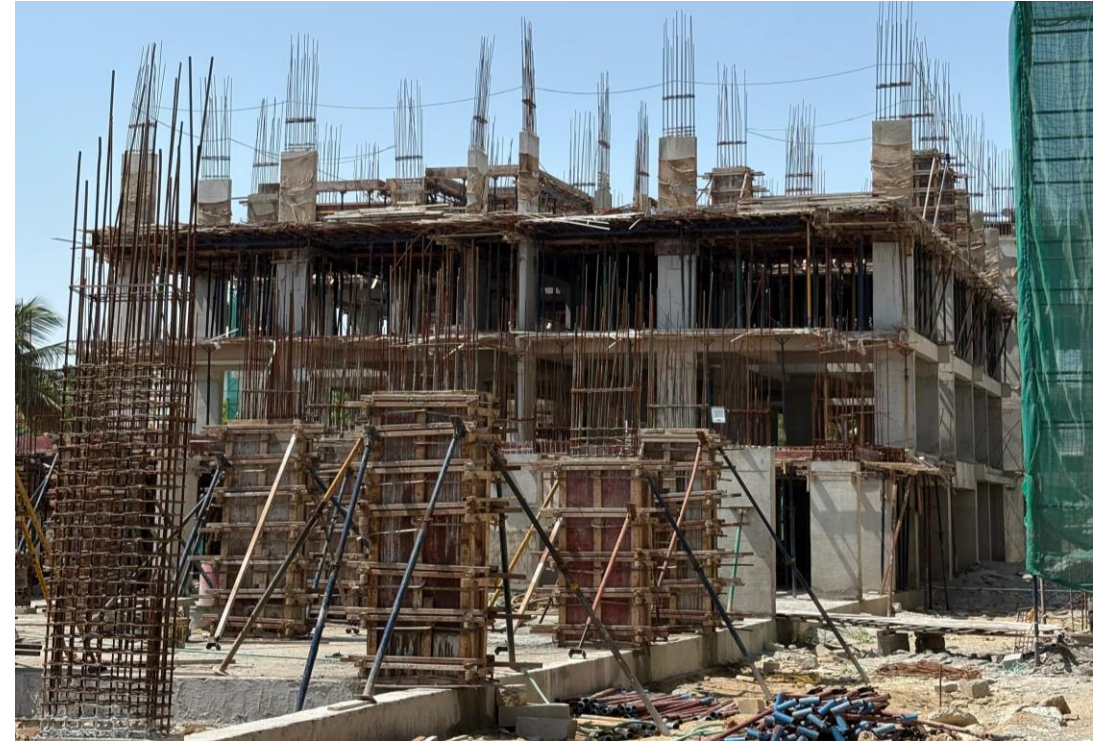
Block-2-Pour 2- Stilt Floor Column Concrete Work in progress
