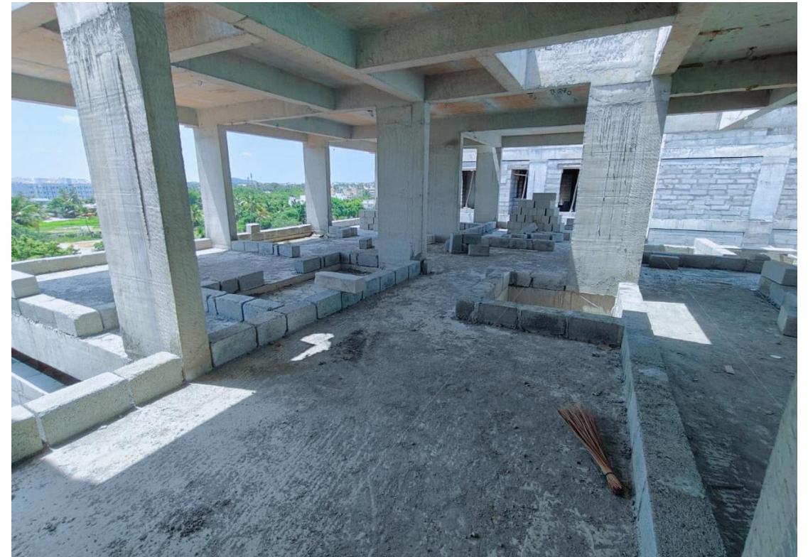
Block-4- Fifth Floor Layout Block Work in progress
