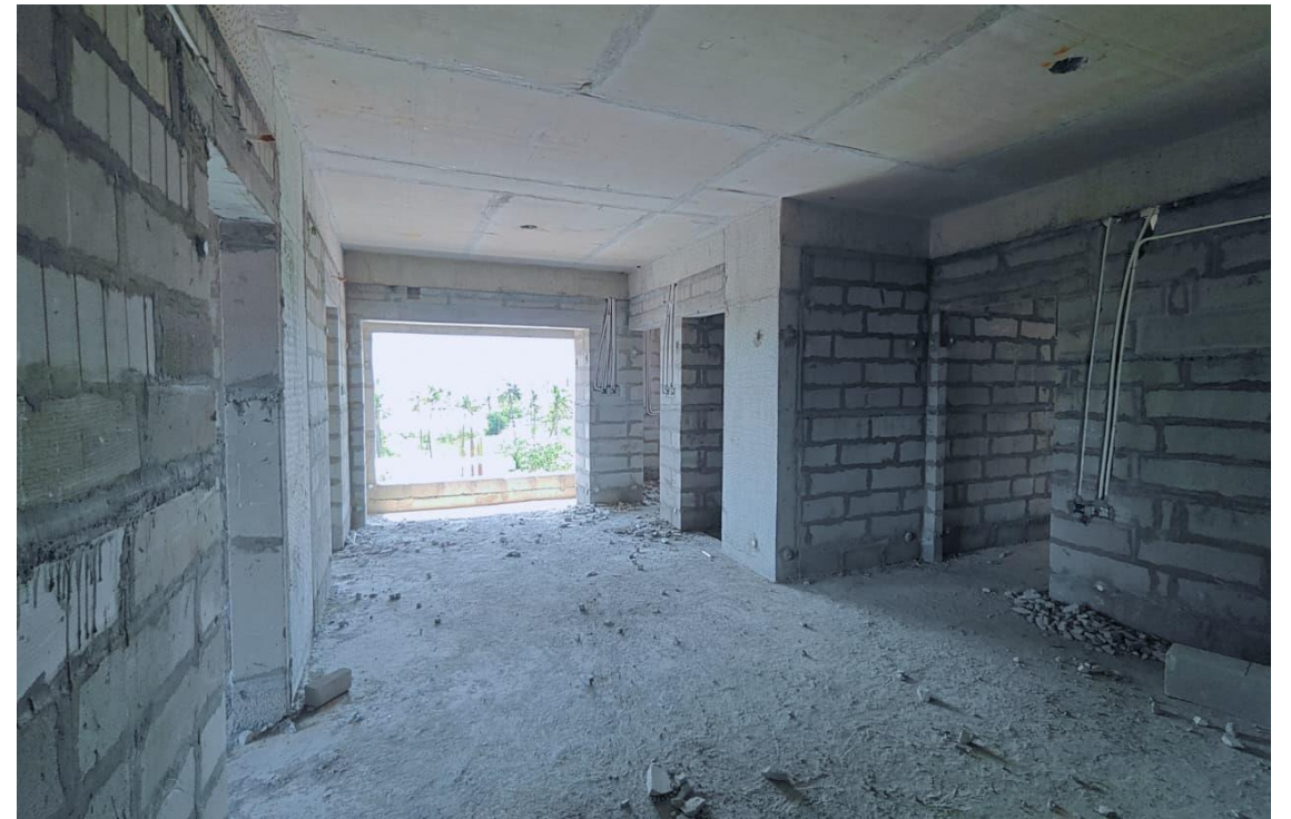
Block-4- Third Floor Electrical Wall Chasing & Conduit laying work in Progress
