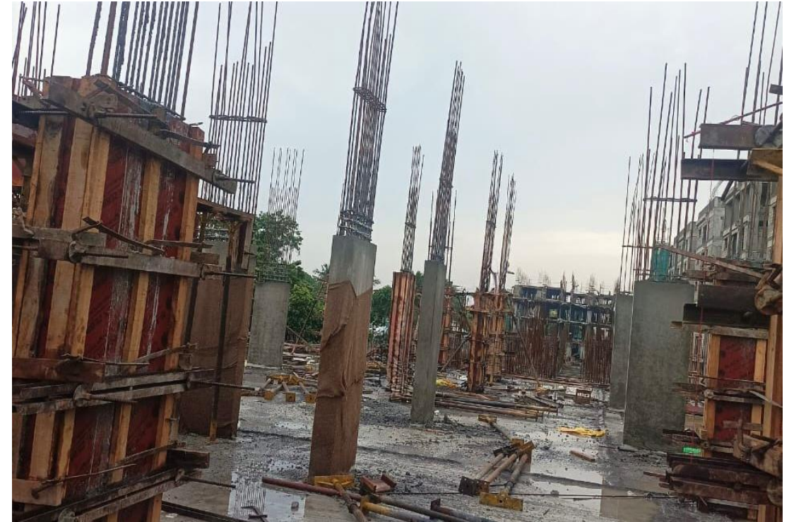
Block-1- Pour-1- First Floor Slab Column concrete work & Roof slab shuttering work in progress
