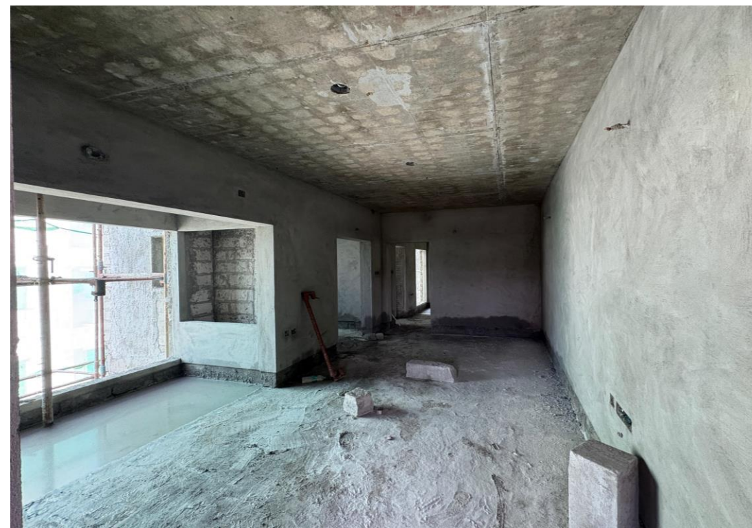
Block-3- Fourth Floor Wall Plastering work in Progress
