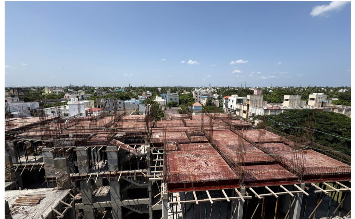
Block-2- Pour 1 – Fourth Floor Slab Reinforcement Work in Progress
