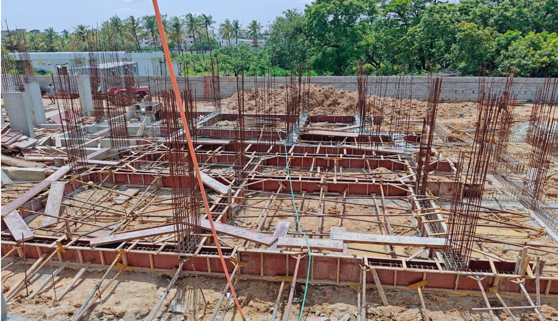
Block-1- Pour 3-Plinth Beam Concrete work in progress
