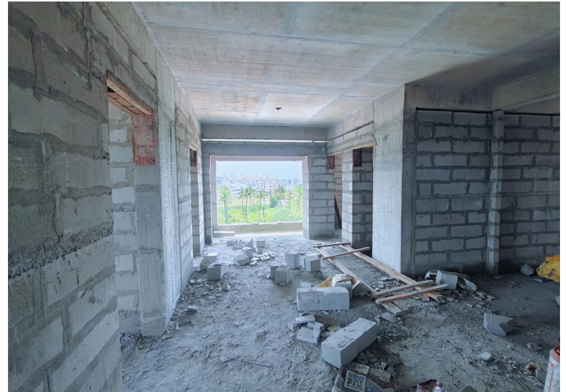
Block-4 Fourth Floor Above lintel Block work in progress
