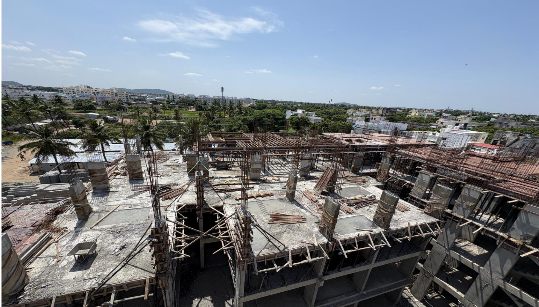
Block-2- Pour 1 – Fourth Floor Slab Shuttering Work in Progress
