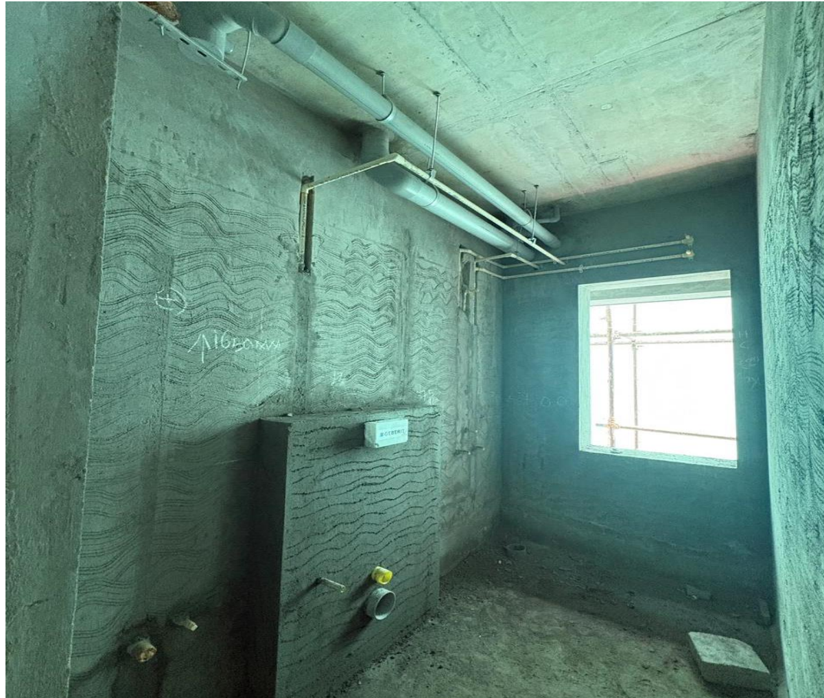
Block-3 First Floor Toilet Suspended Pipeline & Concealed Tank Brick Work in Progress
