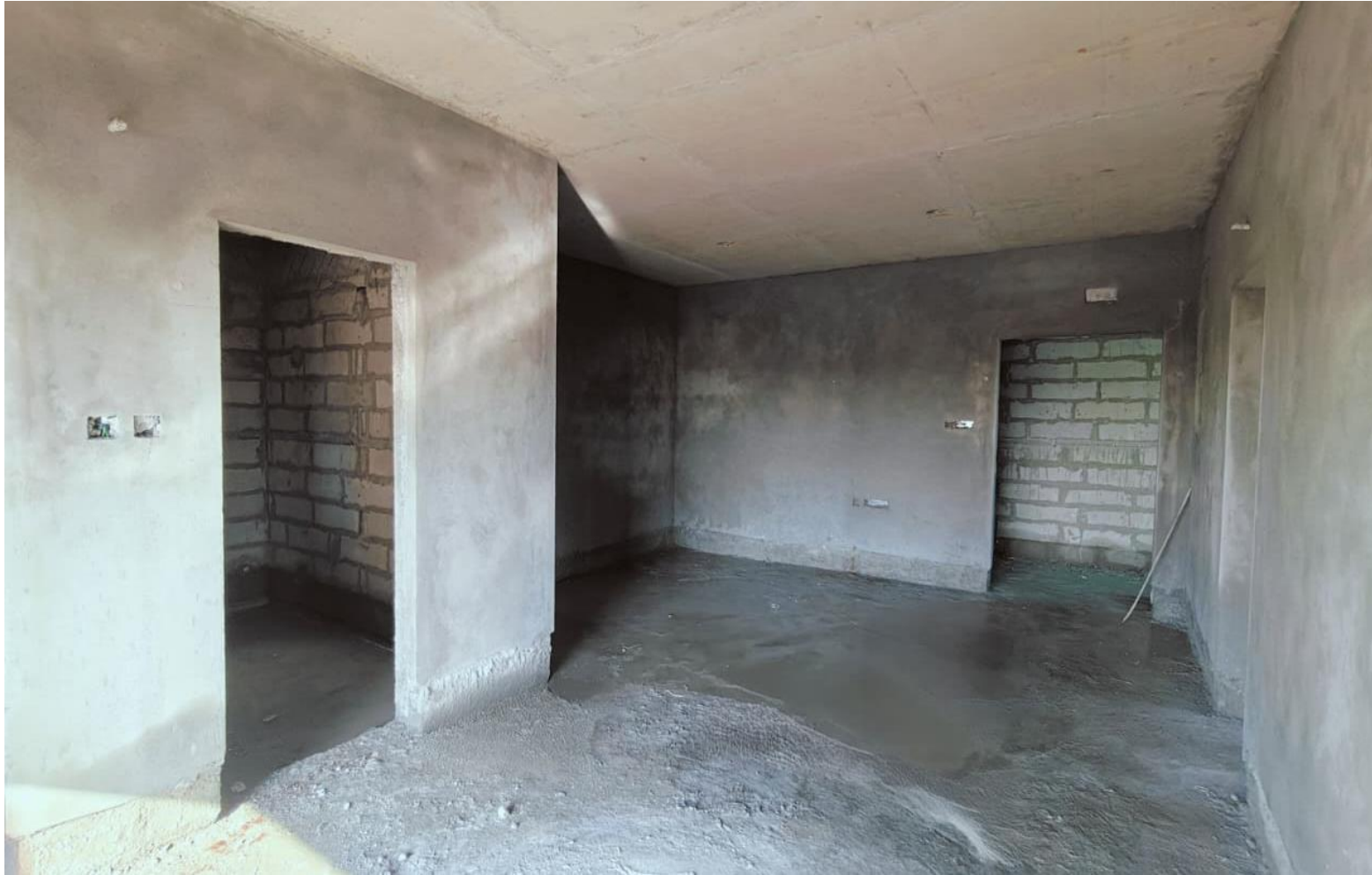
Block-4 Third Floor Plastering Work in Progress
