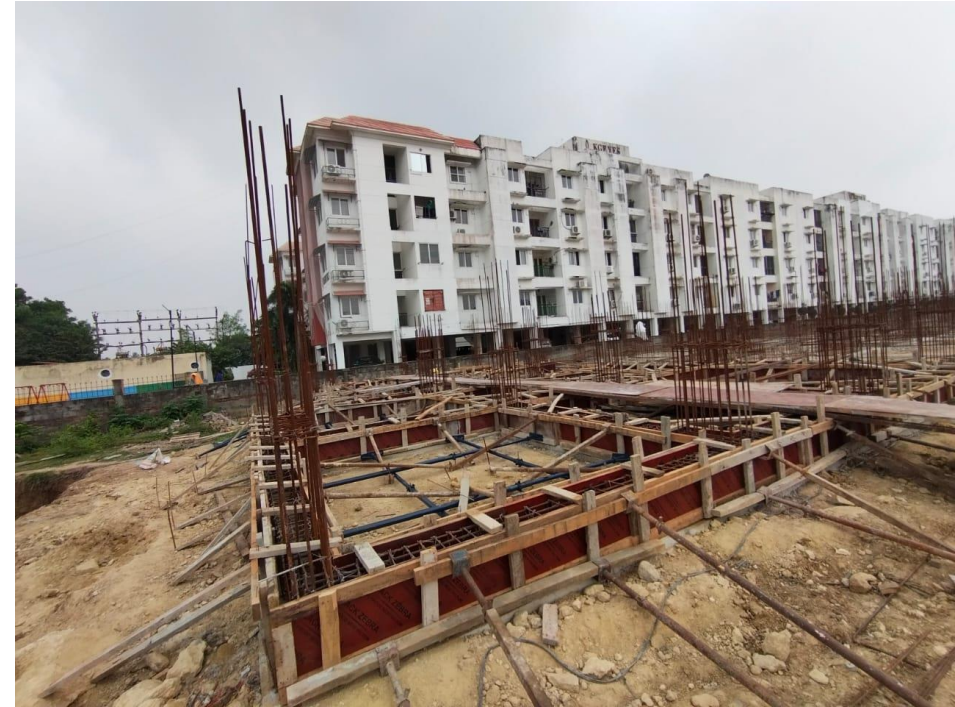
BLOCK-3 PLINTH BEAM REINFORCEMENT & CONCRETE WORK IN PROGRESS
