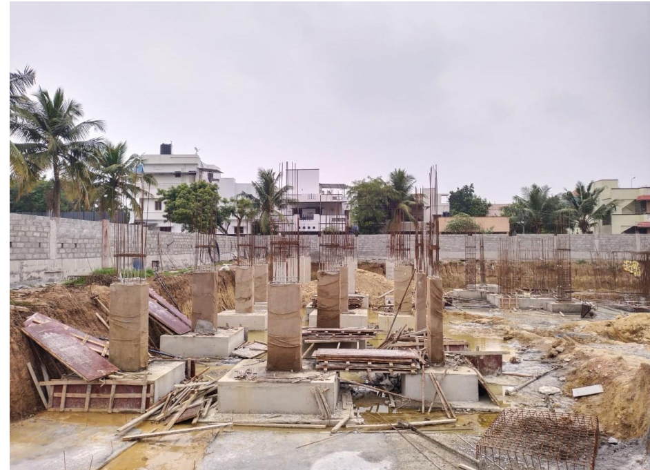
BLOCK-2-FOOTING & COLUMN CONCRETE WORK IN PROGRESS
