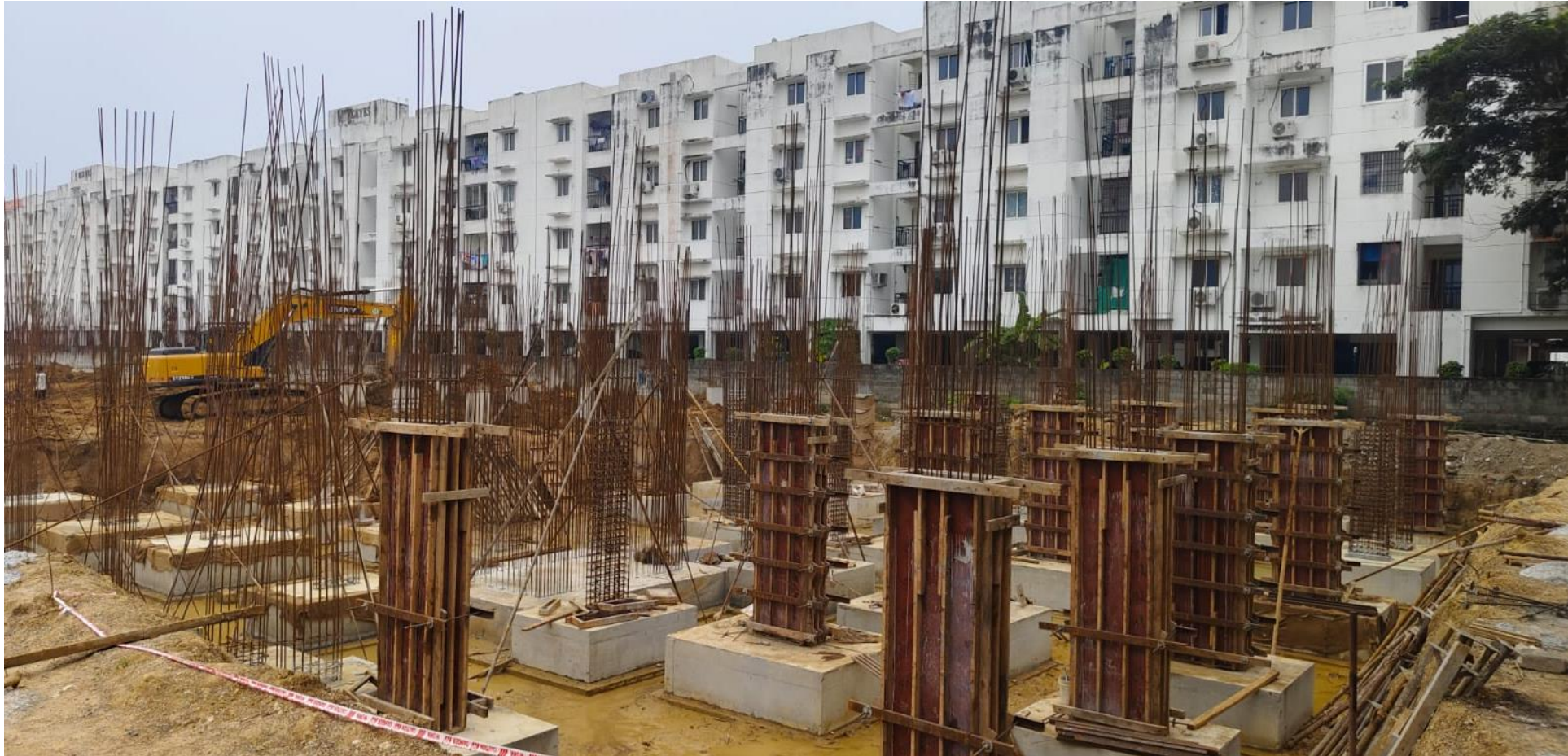
BLOCK -1- FOOTING & COLUMN CONCRETE WORK IN PROGRESS
