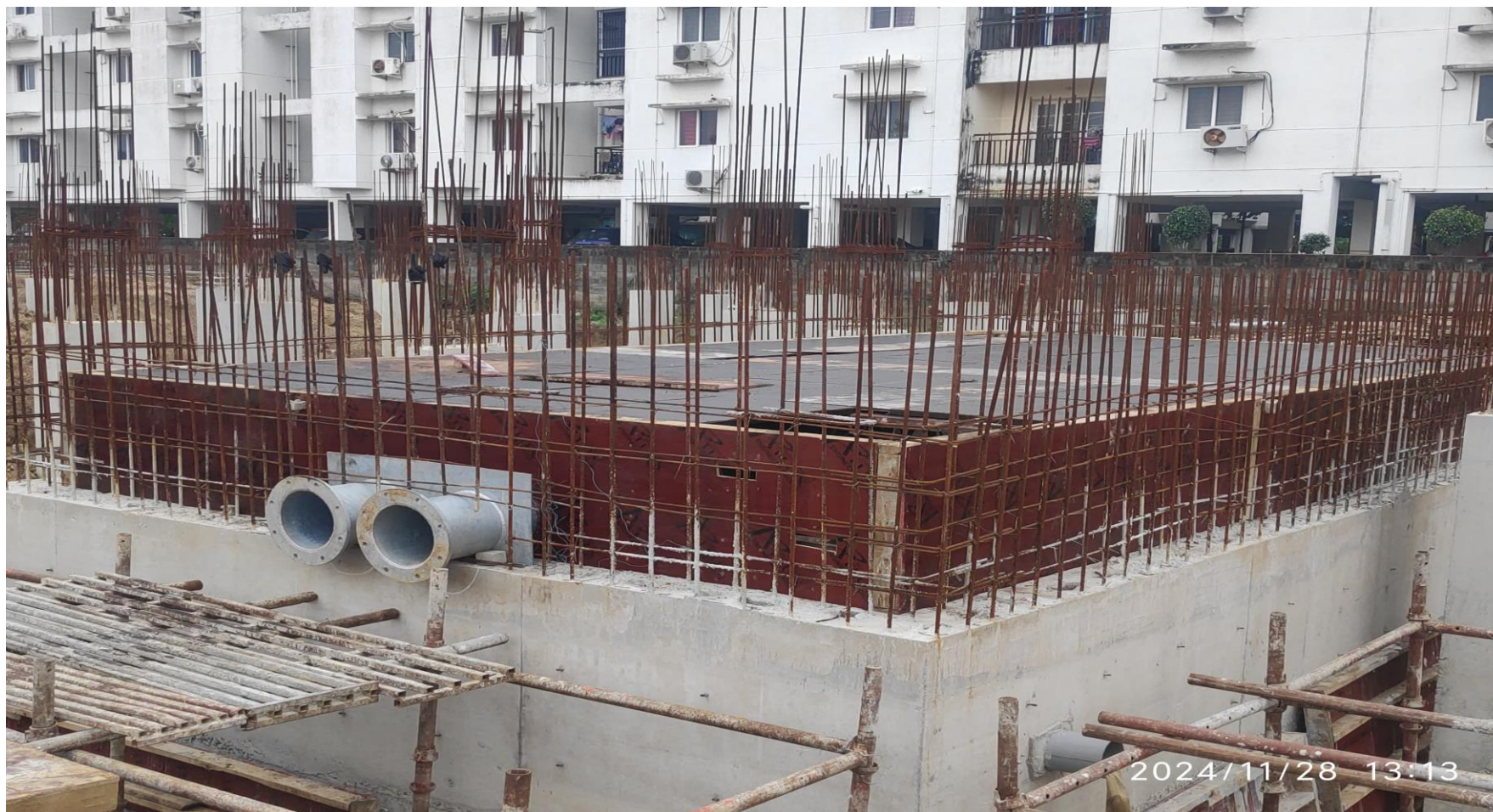
RAIN WATER AND SULLAGE TANK COVER SLAB SHUTTERING WORK IN PROGRESS
