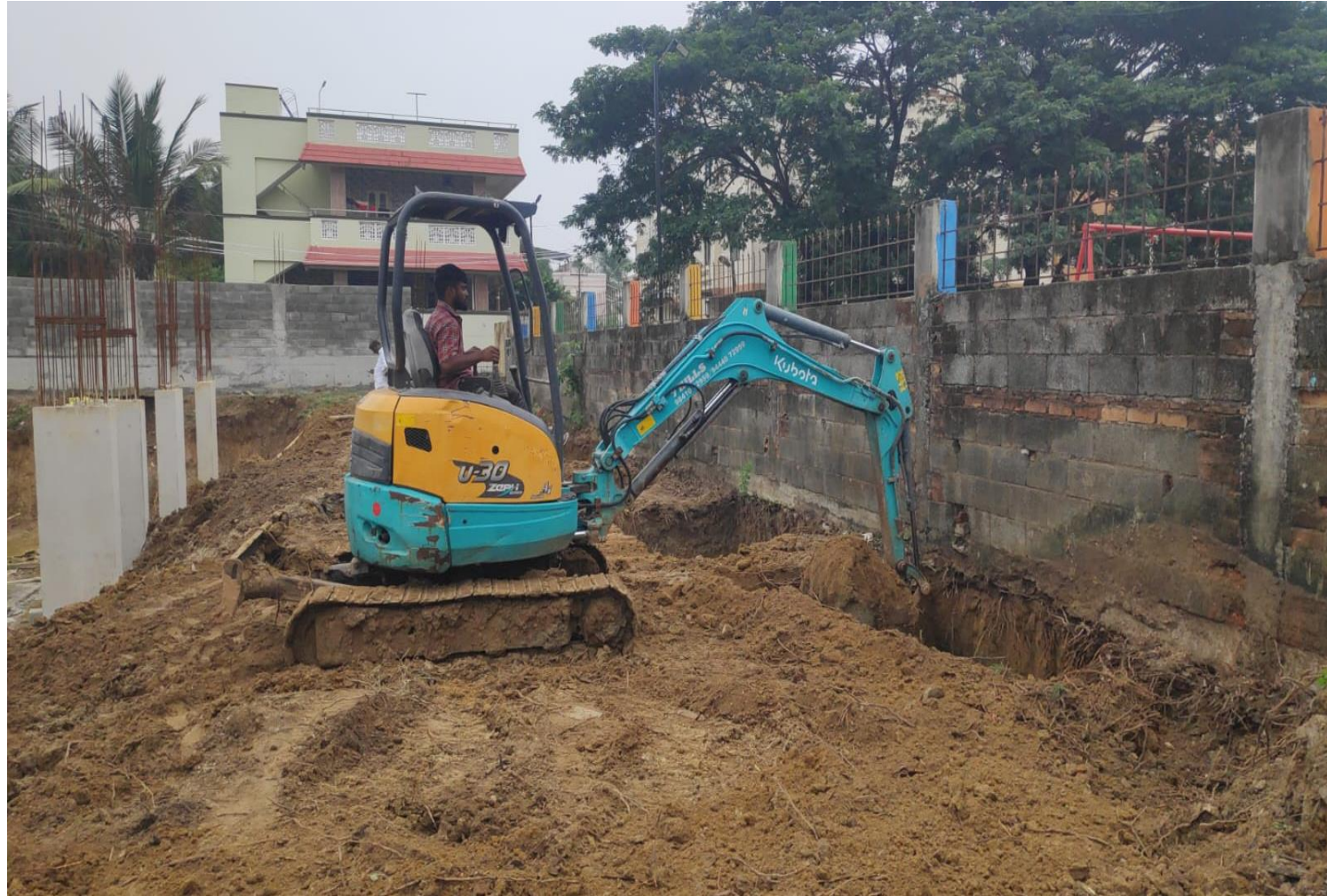
EXTERNAL-EAST SIDE COMPOUND WALL EXCAVATION COMMENCED
