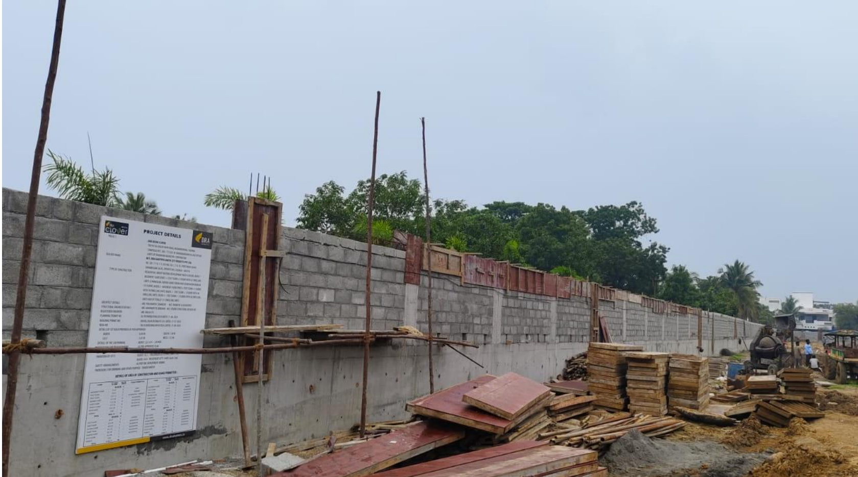
EXTERNAL-WEST & NORTH SIDE COMPOUND WALL COLUMN & COPING BEAM CONCRETE WORK IN PROGRESS
