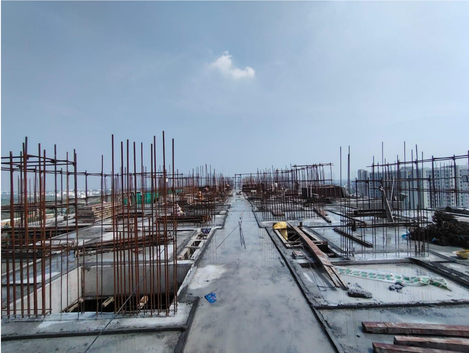
Eleventh Floor Roof Slab Concrete Completed
