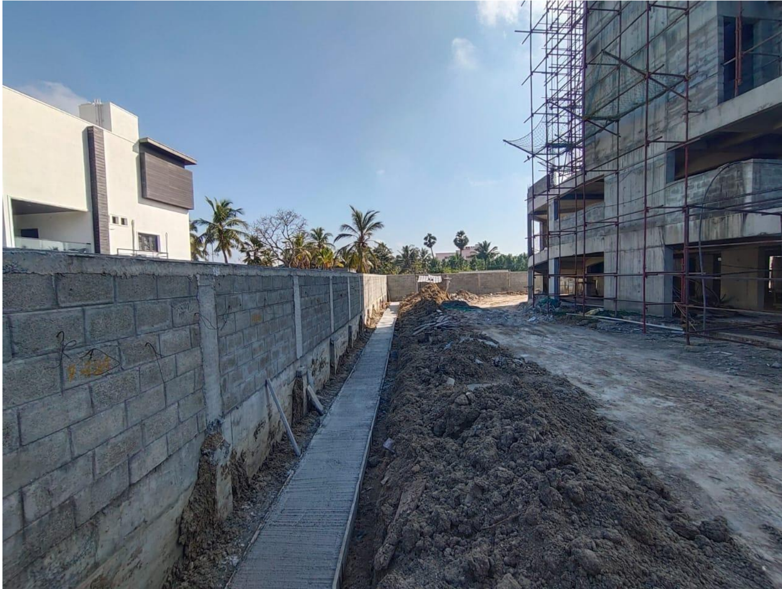
External – East Side Trench PCC Work on Progress
