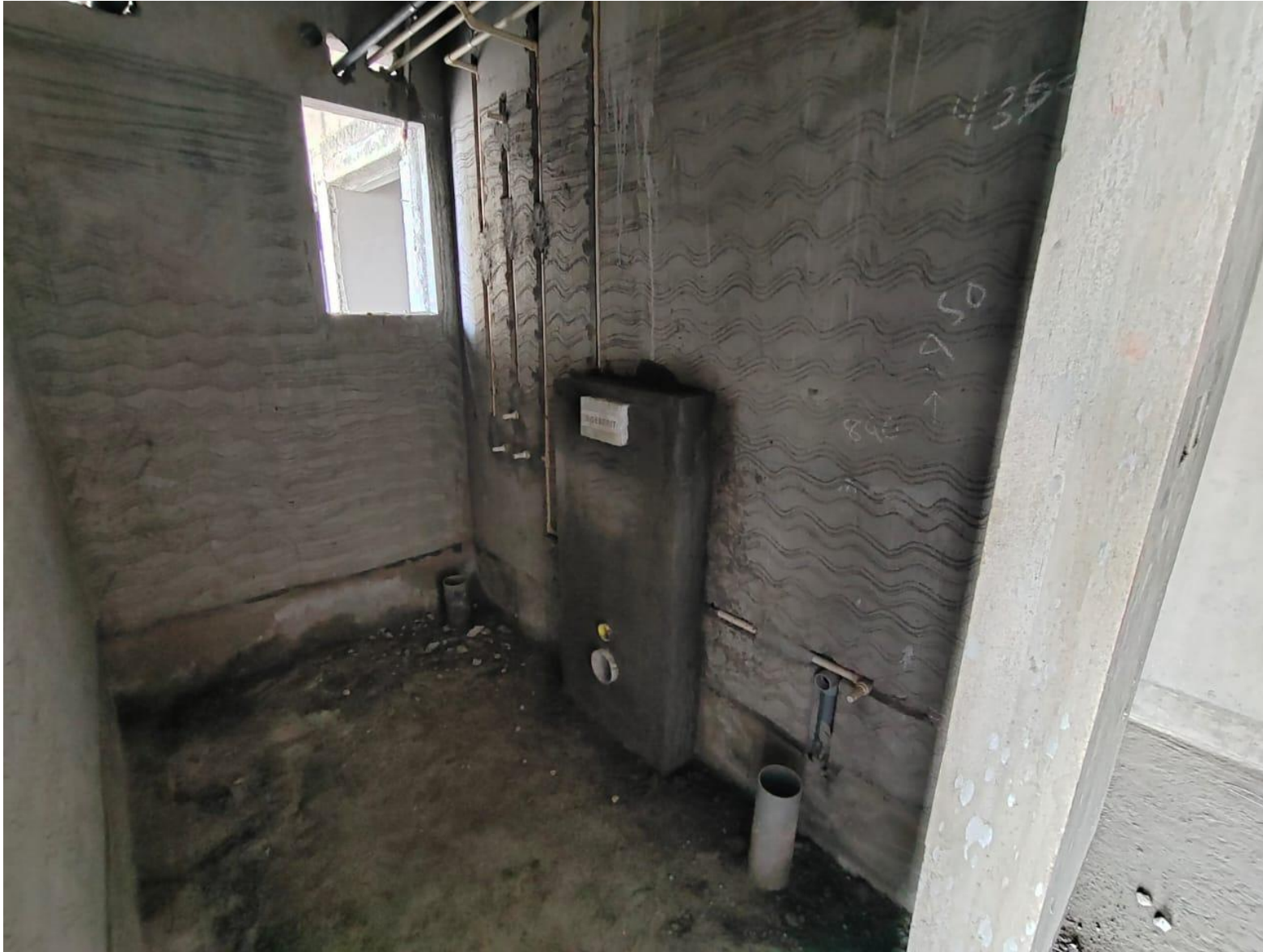
Plumbing – Second Floor Ledge Wall Work on Progress
