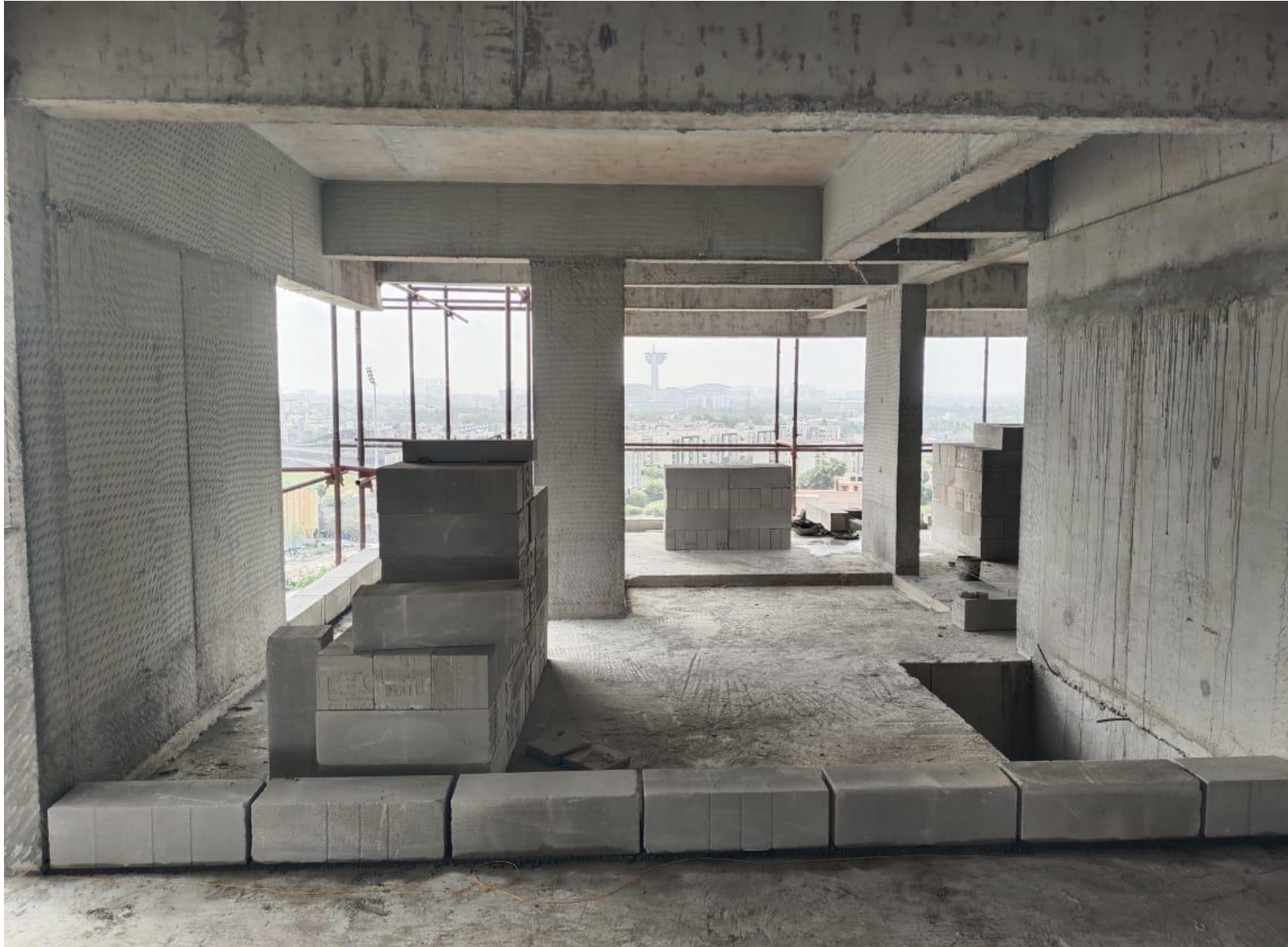
Eleventh Floor Block Work on Progress
