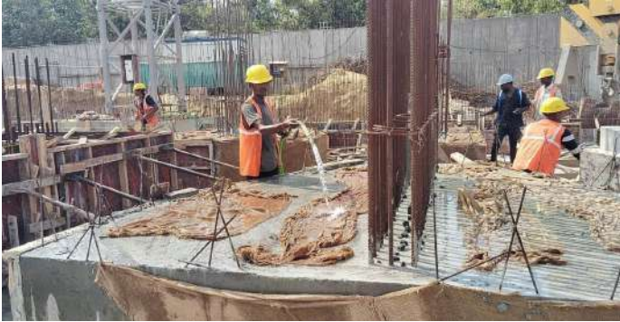
Raft & Pilecap Concrete
