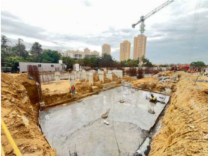
Antitermite Treatment / PCC
