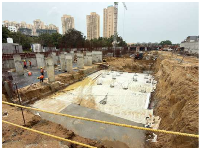
Grade Slab PCC
