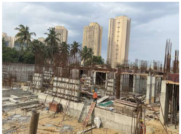
Retaining Wall & Column Reinforcement
