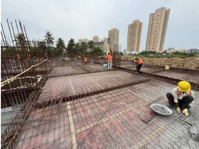
Stilt Floor Slab Shuttering
