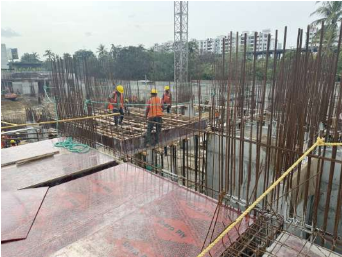
Stilt Floor Slab Shuttering
