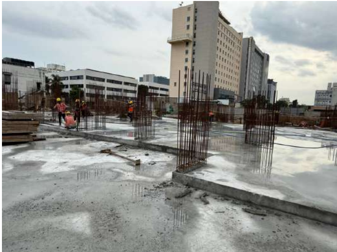
Stilt Floor Slab Shuttering
