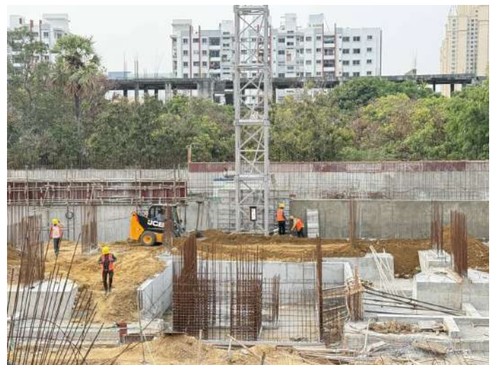
Backfilling & Compaction
