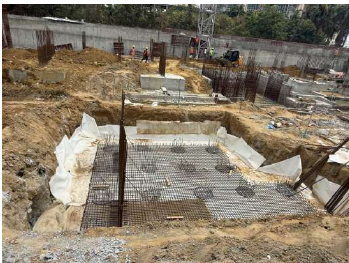
Raft & Pilecap Steel Reinforcement
