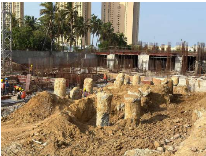
Pile Demolishing Works
