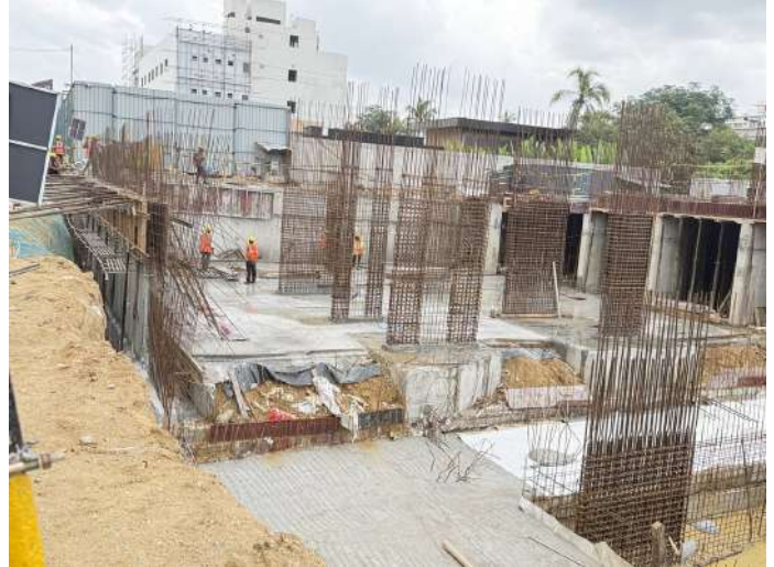
Antitermite Treatment / PCC
