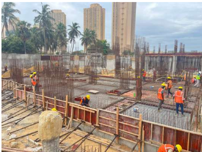
Steel Reinforcement for Cover Slab
