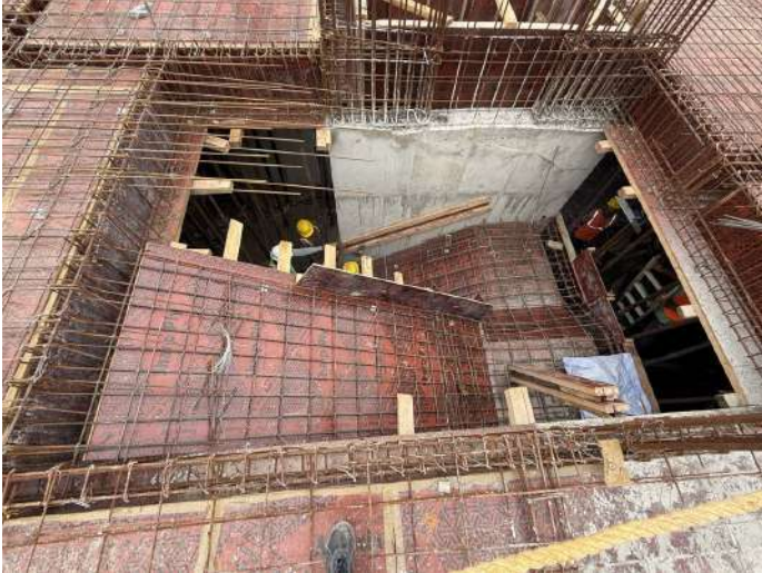
Staircase Reinforcement
