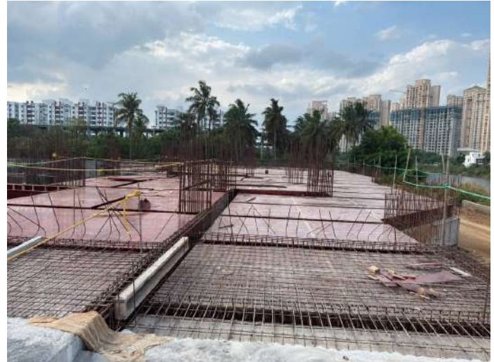
Stilt Floor Slab Shuttering
