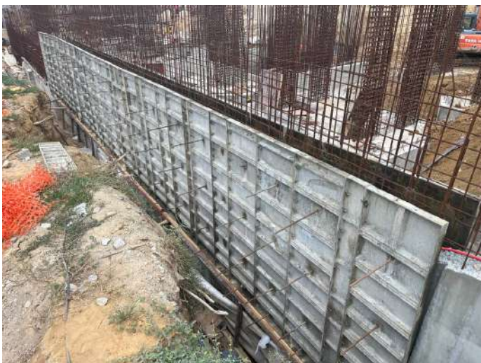
Retaining Wall & Column Shuttering
