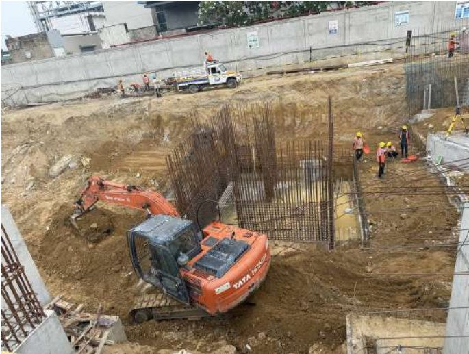
Backfilling & Compaction
