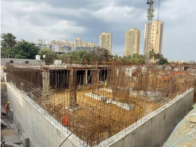
Retaining Wall & Column Reinforcement
