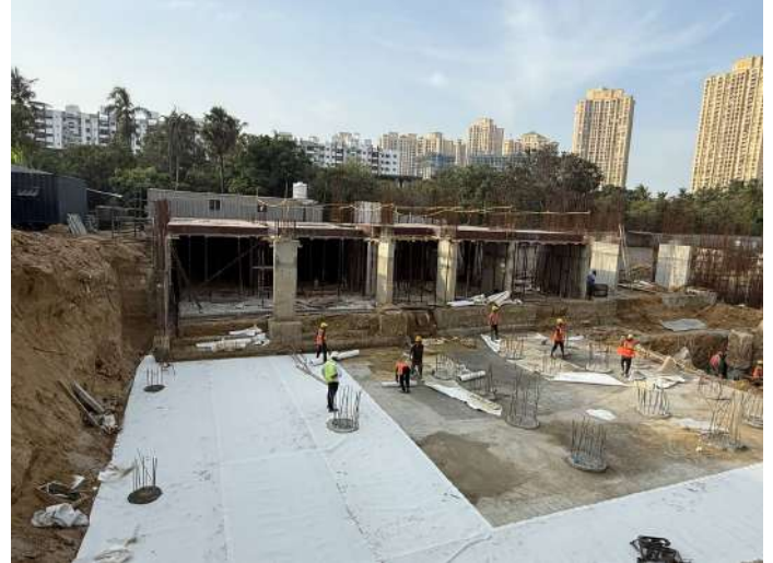
Waterproofing Works
