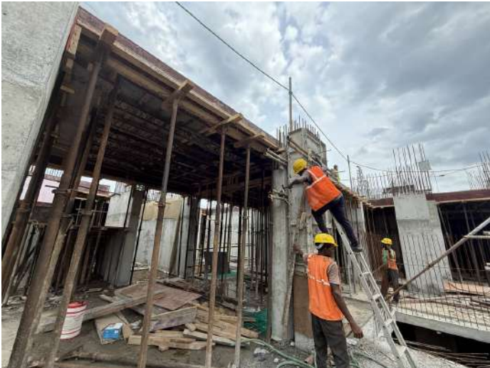
Retaining Wall & Column Shuttering
