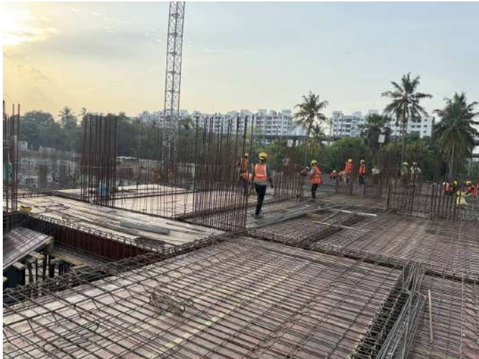
Stilt Floor Slab Shuttering
