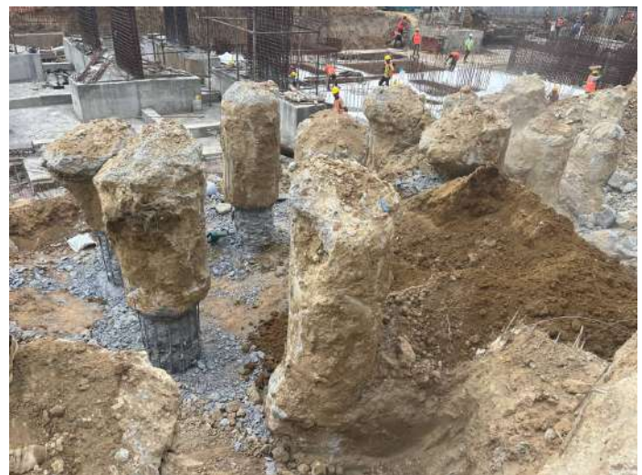
Pile Demolishing Works
