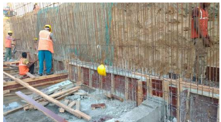
Retaining Wall & Column Reinforcement
