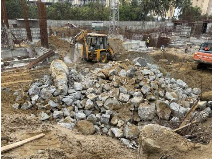
Pile Demolishing Works
