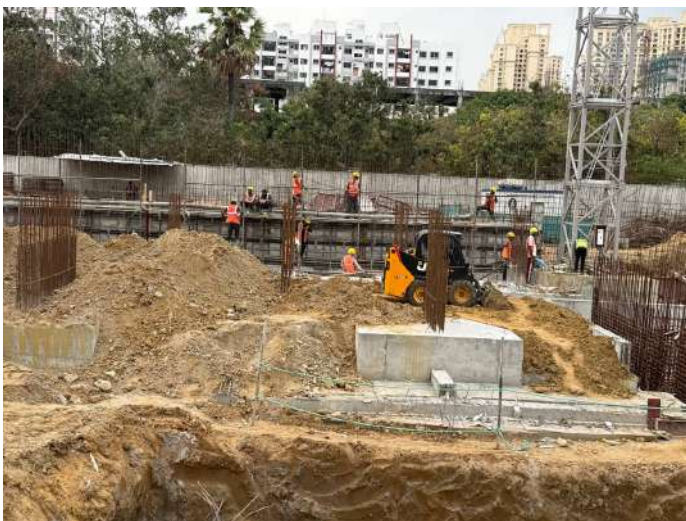
Retaining Wall & Column Starter Fixing
