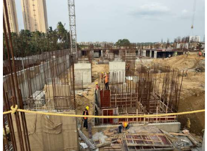
Raft & Pilecap Shuttering
