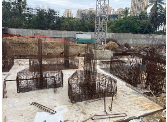
Raft & Pilecap Steel Reinforcement
