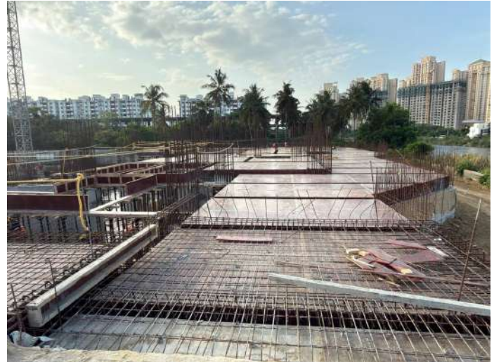
Stilt Floor Slab Shuttering
