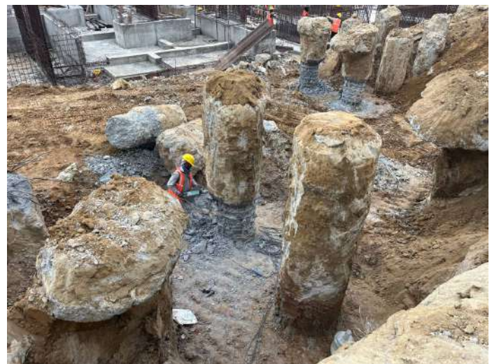
Pile Demolishing Works
