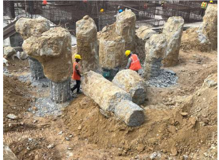
Pile Demolishing Works
