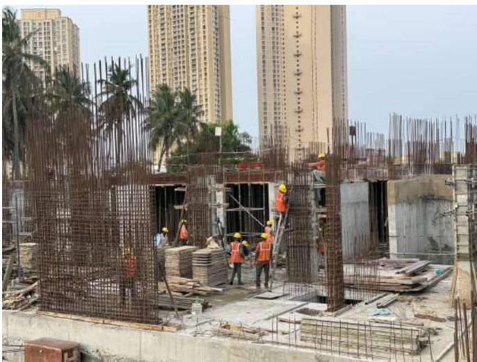
Retaining Wall & Column Shuttering
