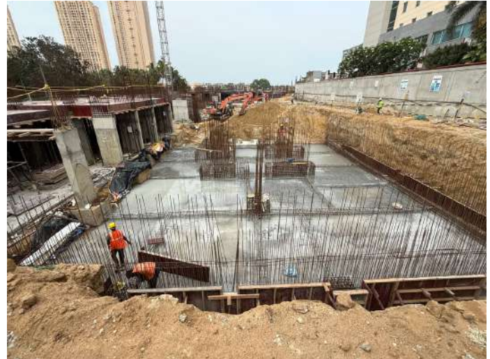
Raft & Pilecap Steel Reinforcement
