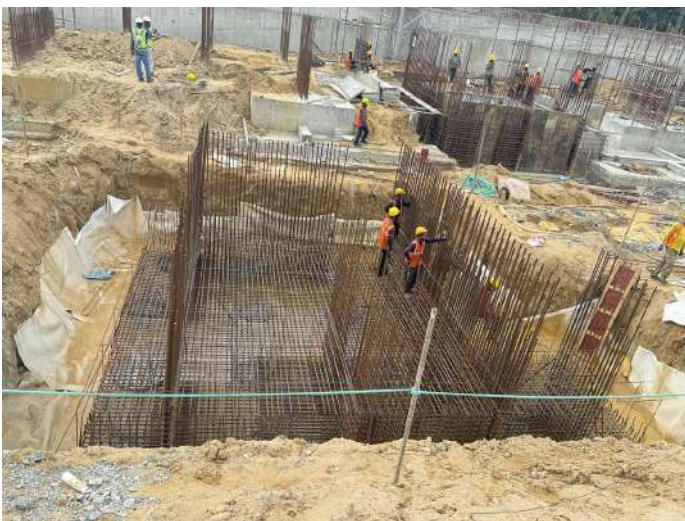
Raft & Pilecap Steel Reinforcement
