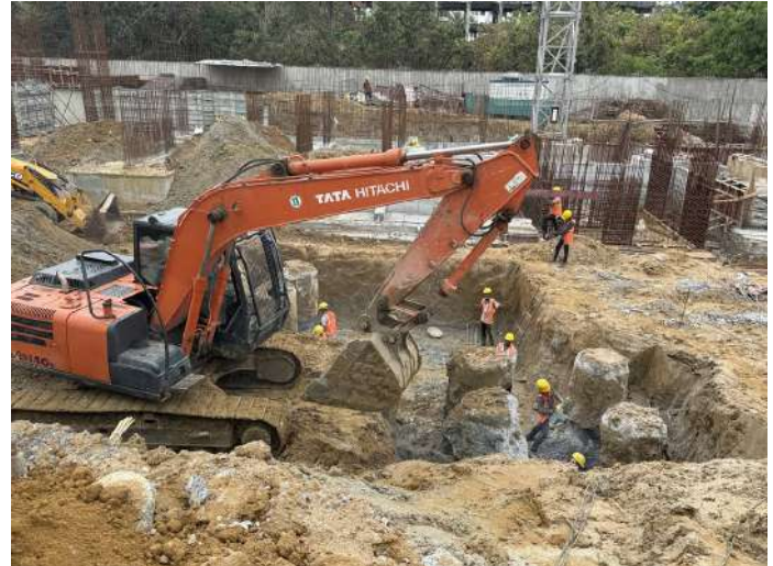
Pile Demolishing Works
