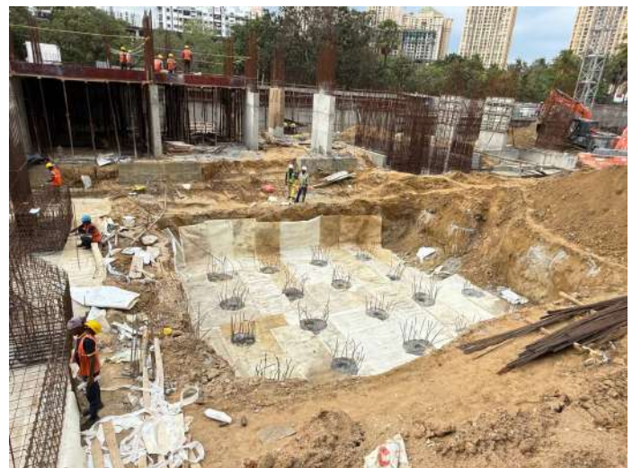
Waterproofing Works
