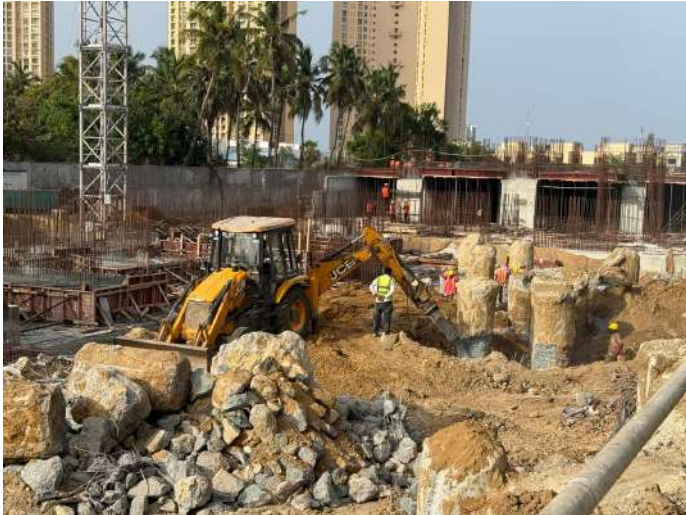
Pile Demolishing Works
