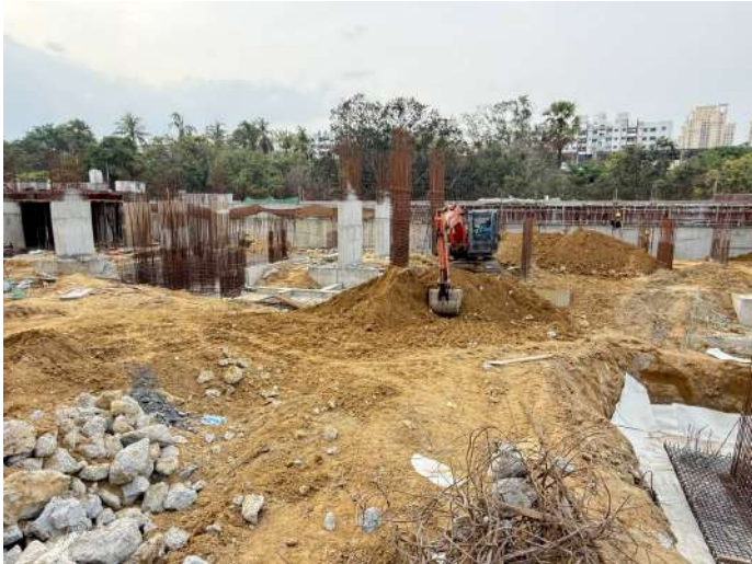
Backfilling & Compaction
