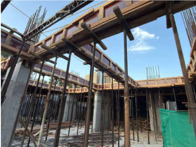
Stilt Floor Slab Shuttering
