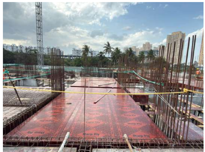
Stilt Floor Slab Shuttering
