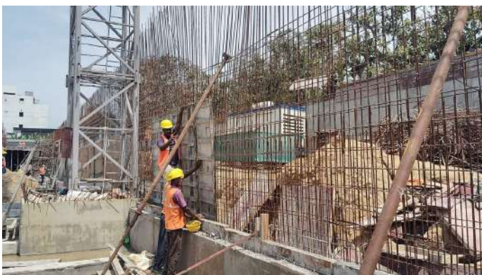
Retaining Wall & Column Shuttering
