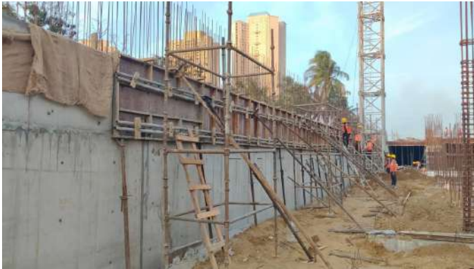
Retaining Wall & Column Reinforcement
