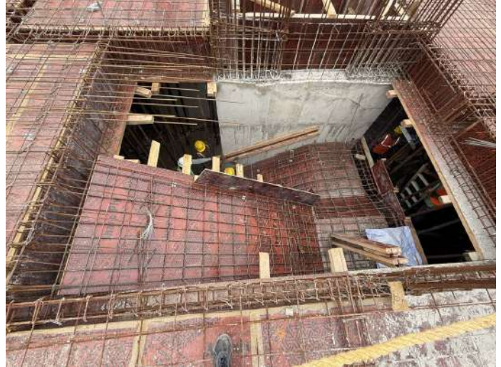
Staircase Shuttering
