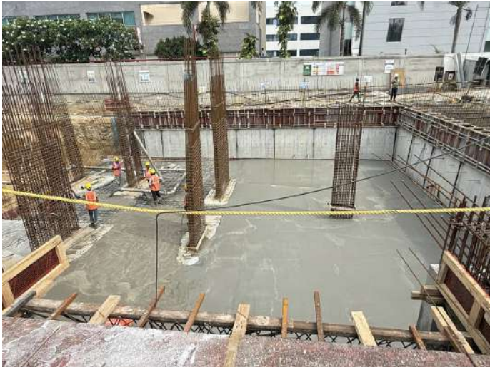
Grade Slab RCC
