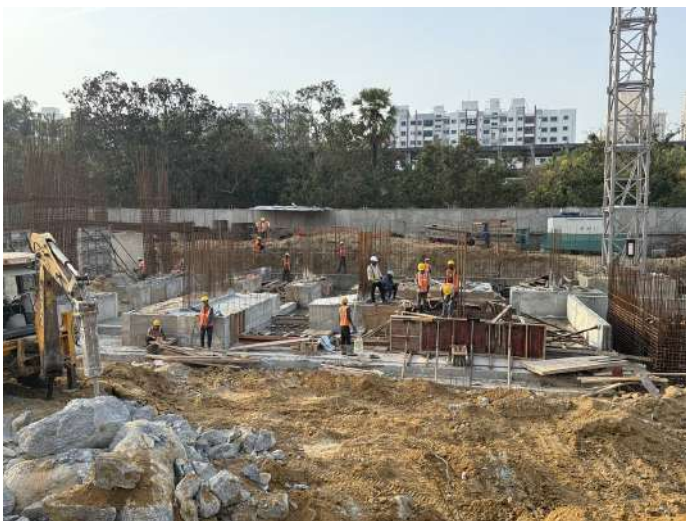
Raft & Pilecap Steel Reinforcement
