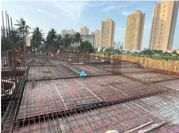
Stilt Floor Slab Reinforcement
