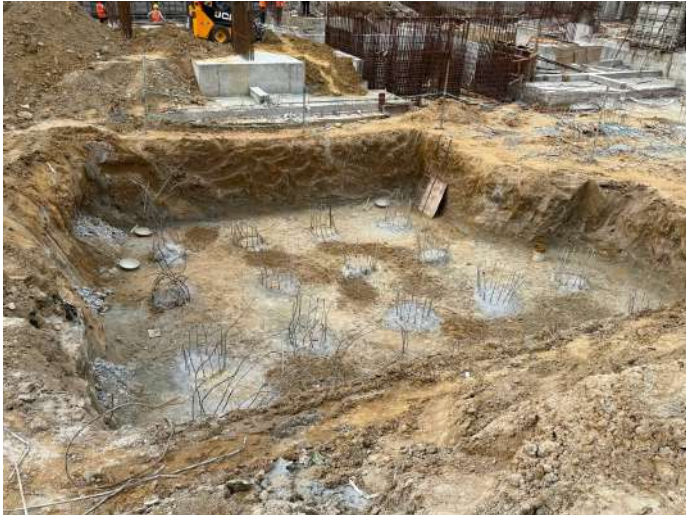
Pile Demolishing Works
