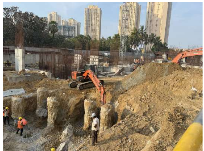
Pile Demolishing Works
