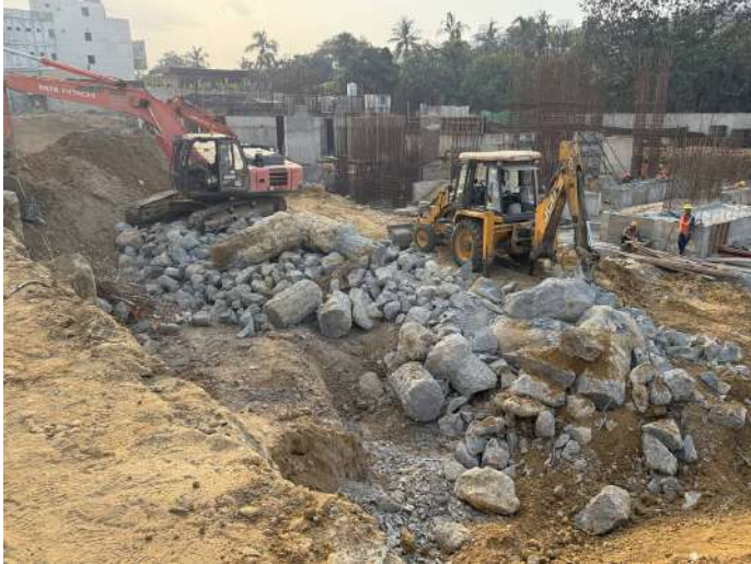
Pile Demolishing Works
