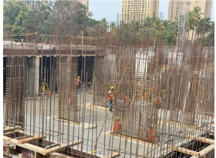
Retaining Wall & Column Starter Fixing
