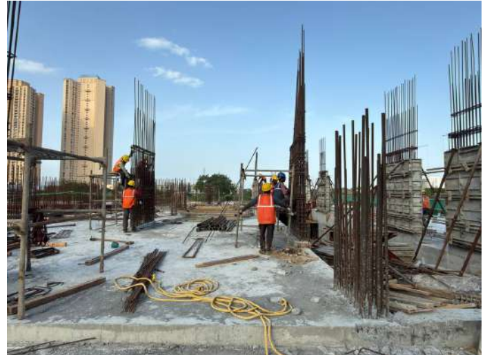
Column Reinforcement
