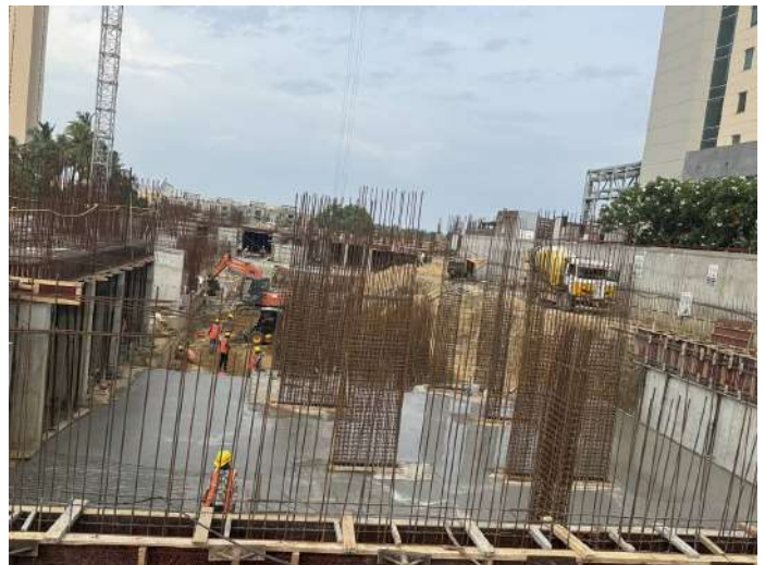
Grade Slab RCC
