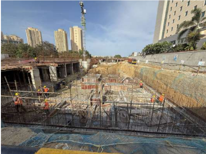
Raft & Pilecap Steel Reinforcement
