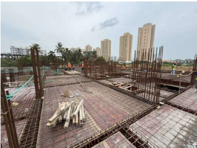
Stilt Floor Slab Reinforcement
