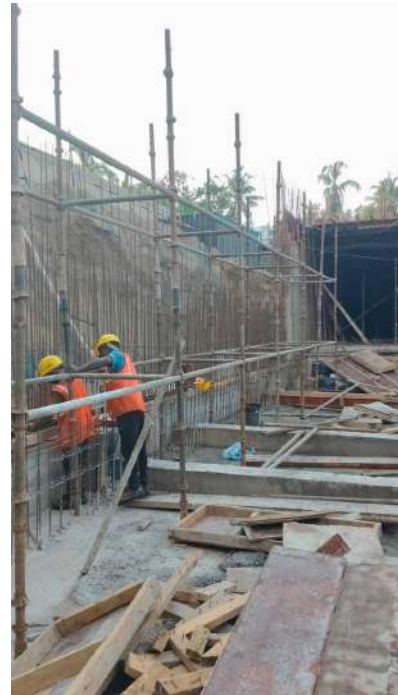
Retaining Wall & Column Reinforcement
