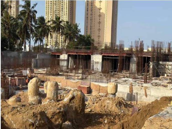
Stilt Floor Slab Shuttering
