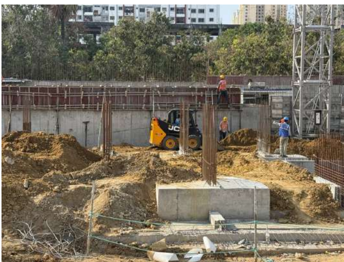
Backfilling & Compaction
