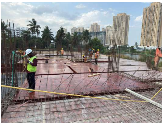
Stilt Floor Slab Shuttering
