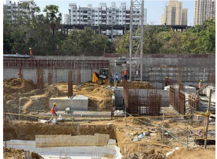
Backfilling & Compaction
