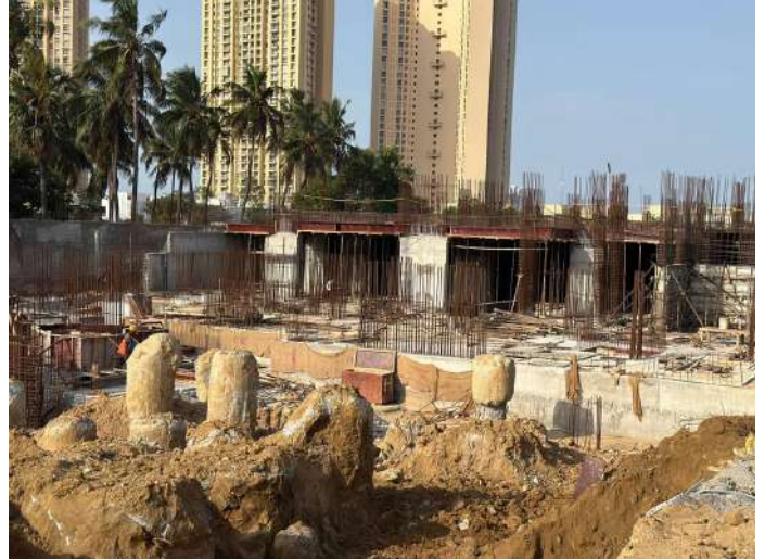
Stilt Floor Slab Shuttering
