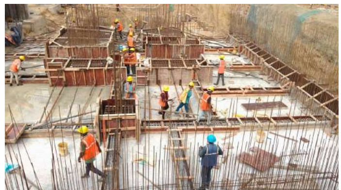
Raft & Pilecap Shuttering
