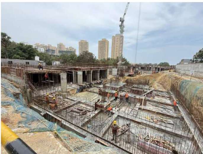
Raft & Pilecap Concrete
