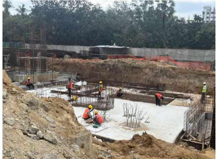
Raft & Pilecap Steel Reinforcement
