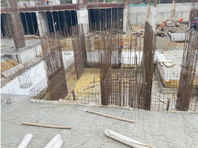
Antitermite Treatment / PCC
