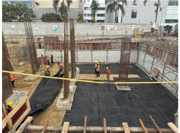
Antitermite Treatment / PCC
