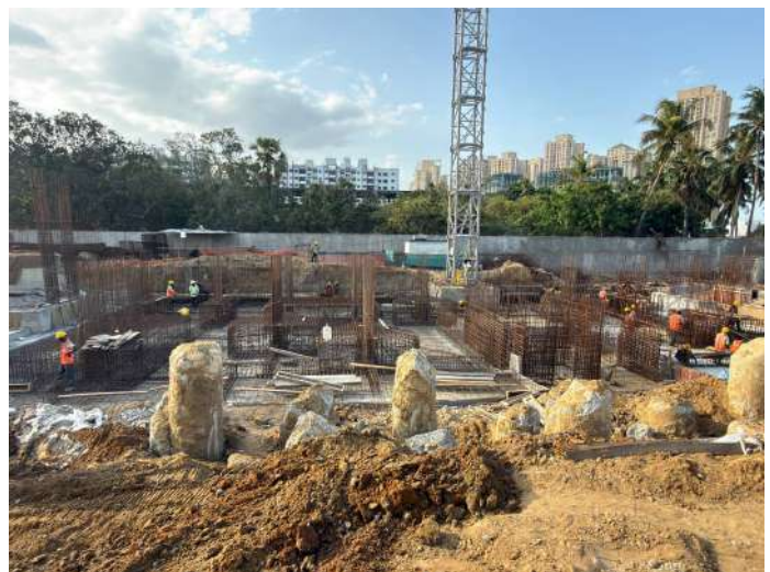
Pile Demolishing Works
