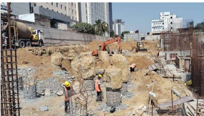
Pile Demolishing Works
