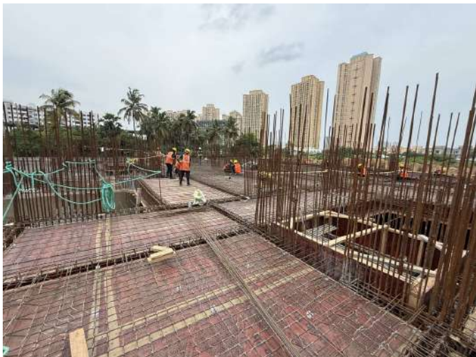
Stilt Floor Slab Reinforcement
