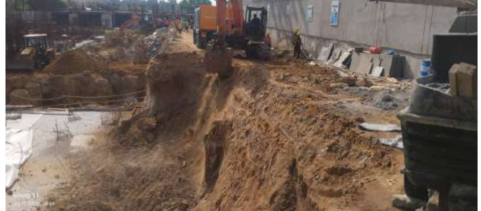
Pile Demolishing Works
