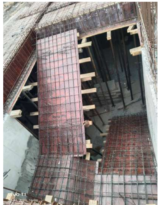
Staircase Shuttering
