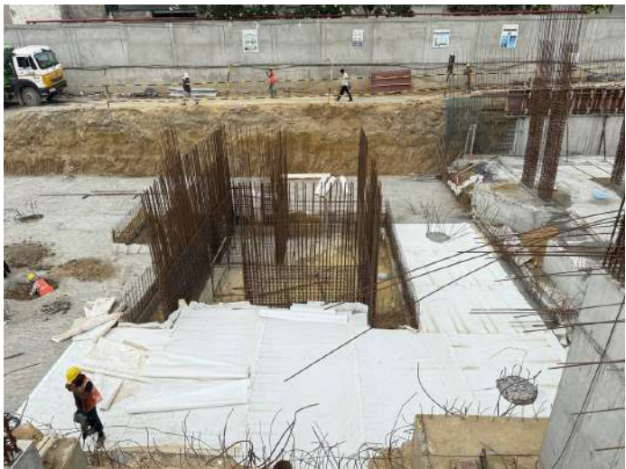
Waterproofing Works
