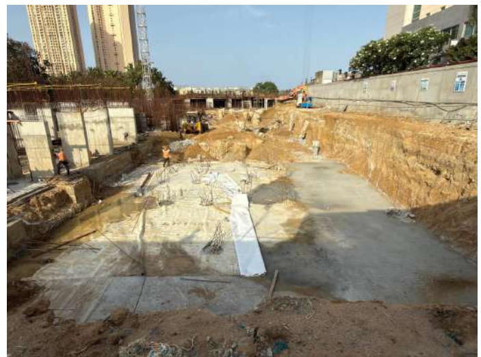
Grade Slab PCC
