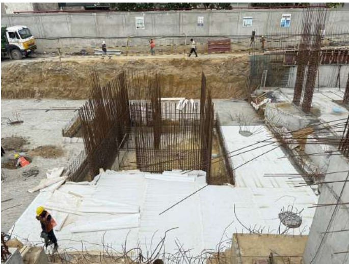
Raft & Pilecap Steel Reinforcement
