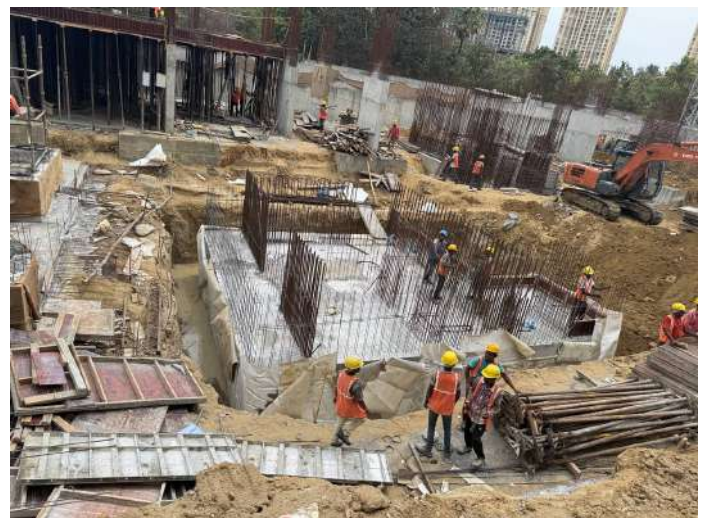
Raft & Pilecap Steel Reinforcement
