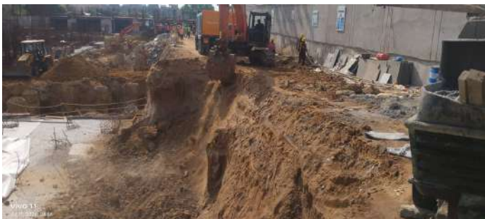
Pile Demolishing Works
