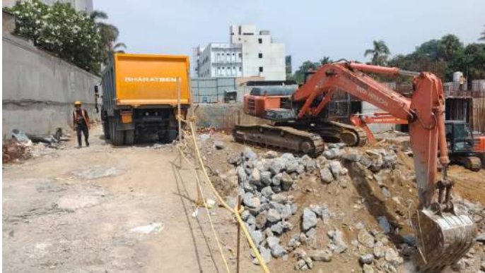
Pile Demolishing Works
