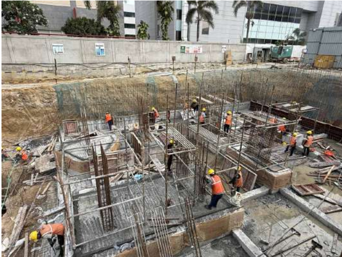
Retaining Wall & Column Starter Fixing
