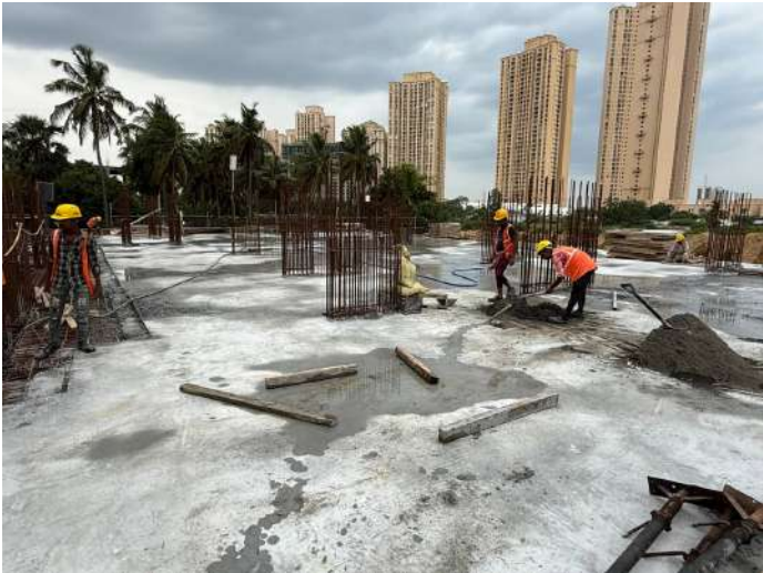
Stilt Floor Slab Shuttering
