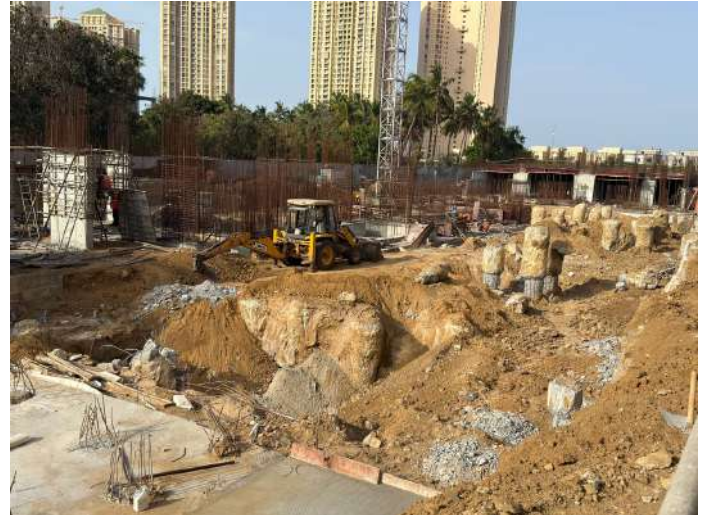
Pile Demolishing Works
