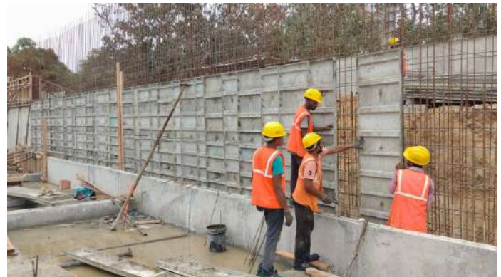
Retaining Wall & Column Starter Fixing
