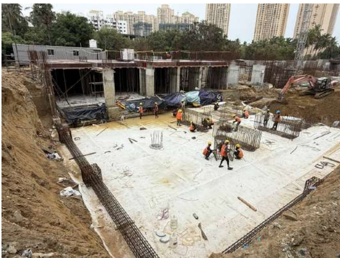
Raft & Pilecap Steel Reinforcement
