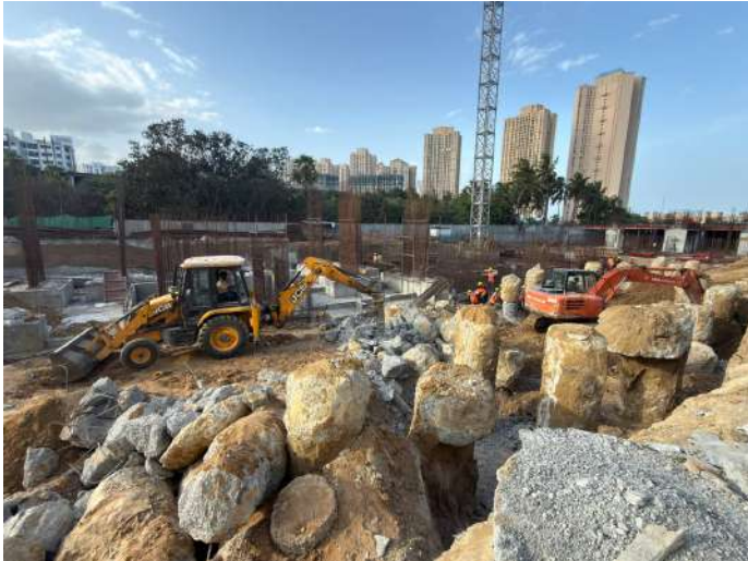
Pile Demolishing Works
