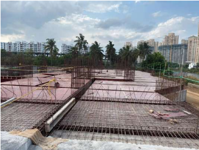
Stilt Floor Slab Shuttering
