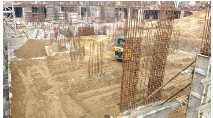
Backfilling & Compaction
