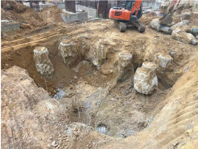
Pile Demolishing Works
