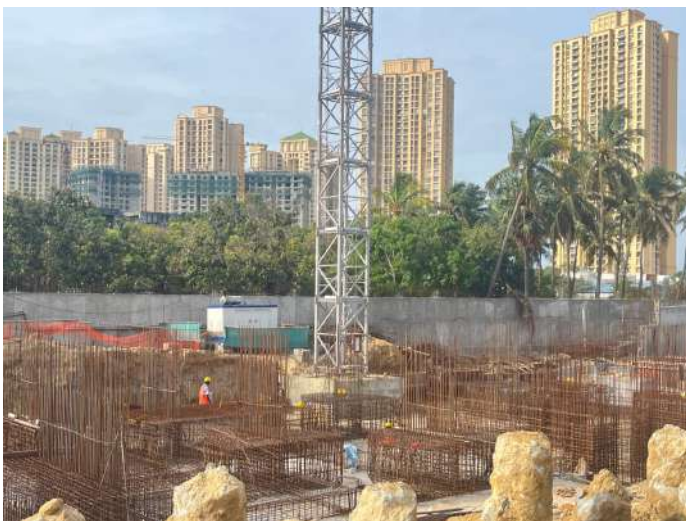
Raft & Pilecap Steel Reinforcement
