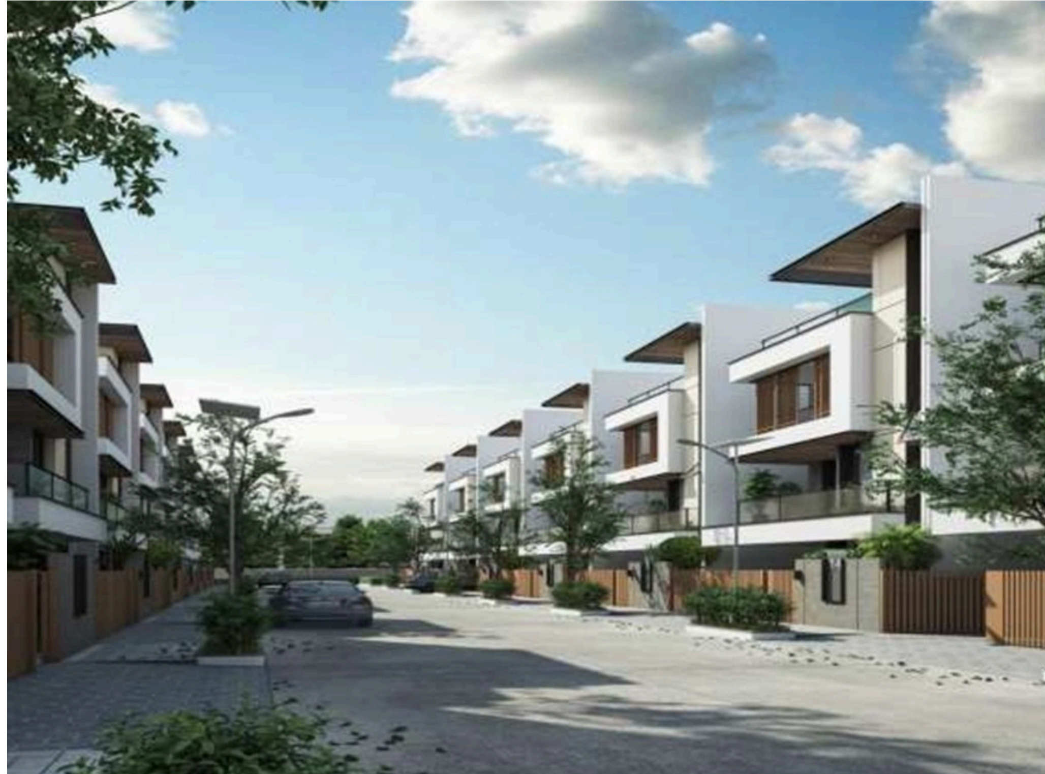
DRA INARA Monthly Progress Photos –April 2026 – Phase 2
