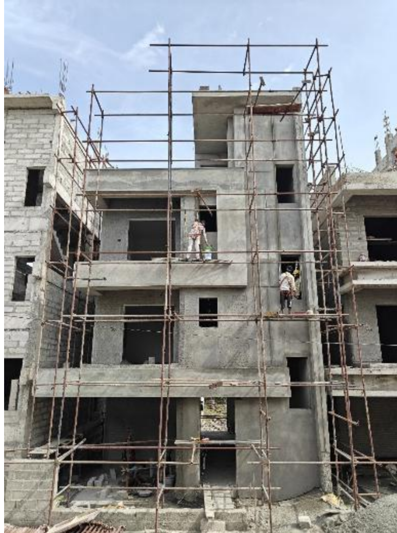
Villa No 9 – External plastering work in progress
