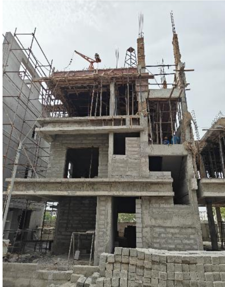
Villa No 13– Head room Column concreting work completed
