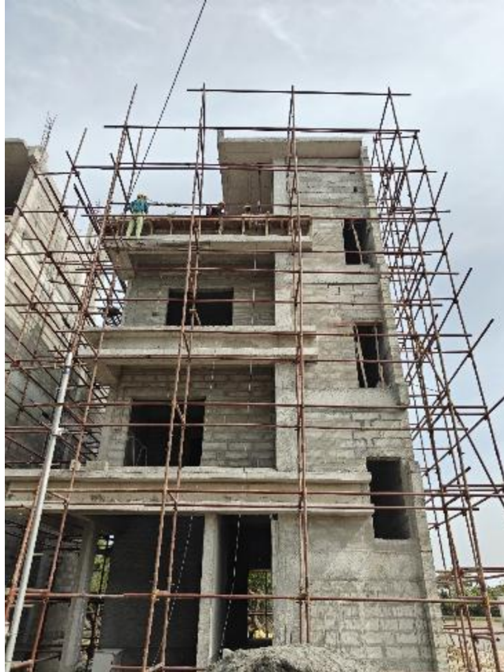
Villa No 11- External plastering work in progress
