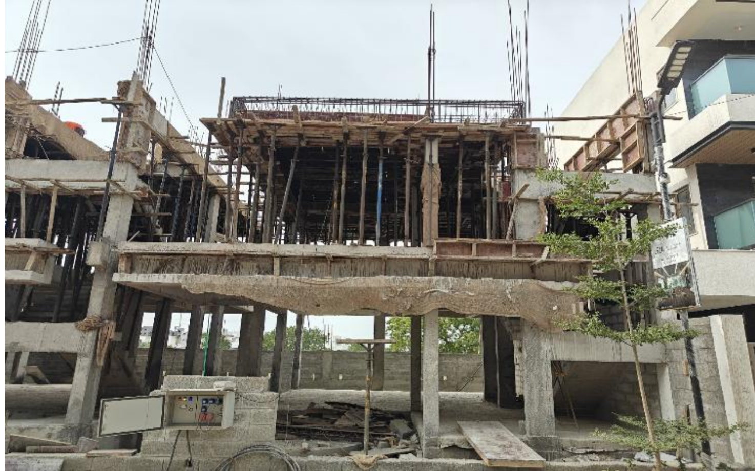
Villa No 15 – FF Roof slab Reinforcement work in progress
