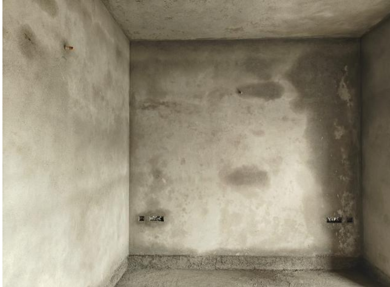
Villa No 3- SF Bedroom Internal plastering work in progress
