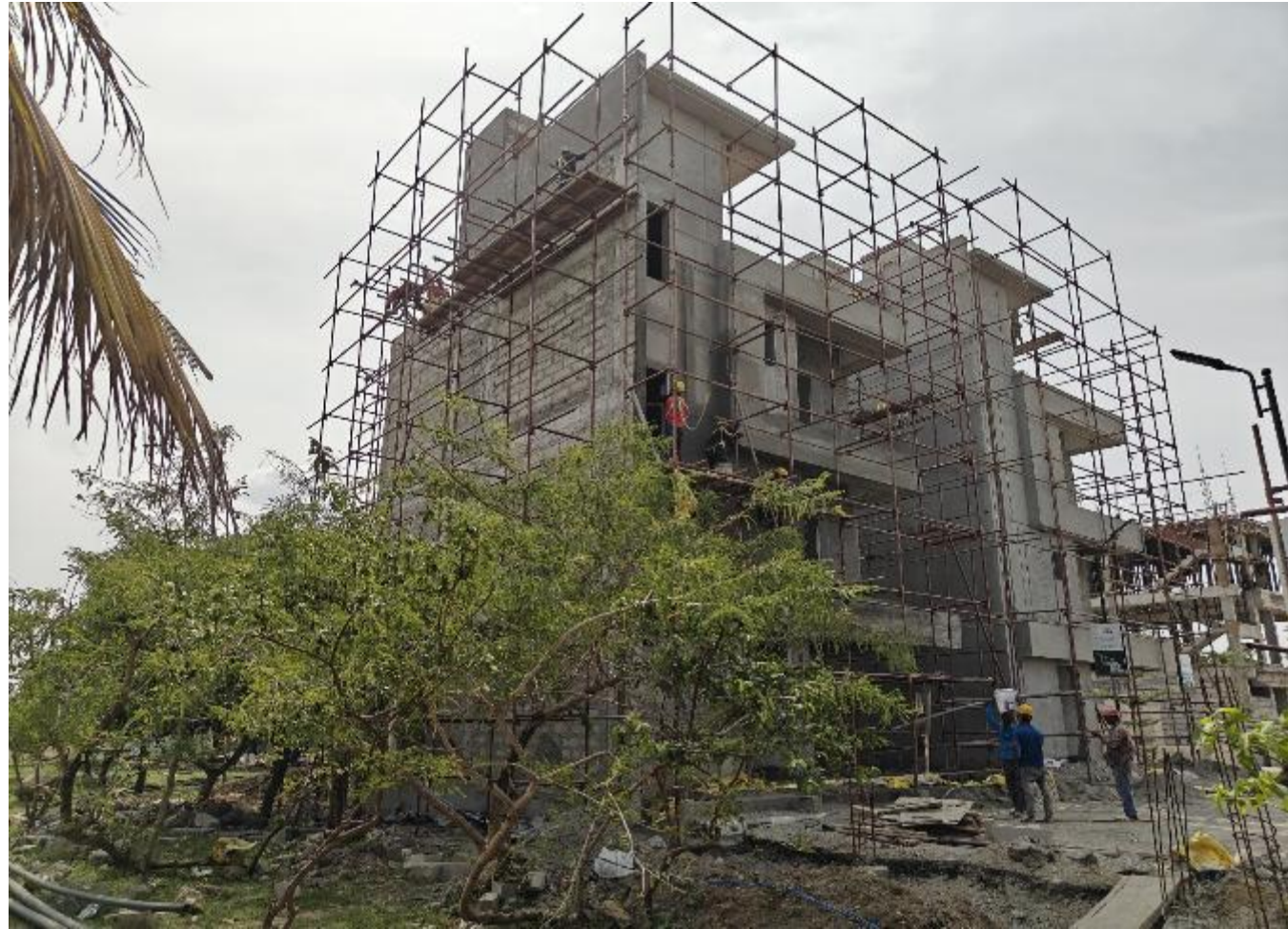
Villa No 4 & 5 External Plastering Work in Progress
