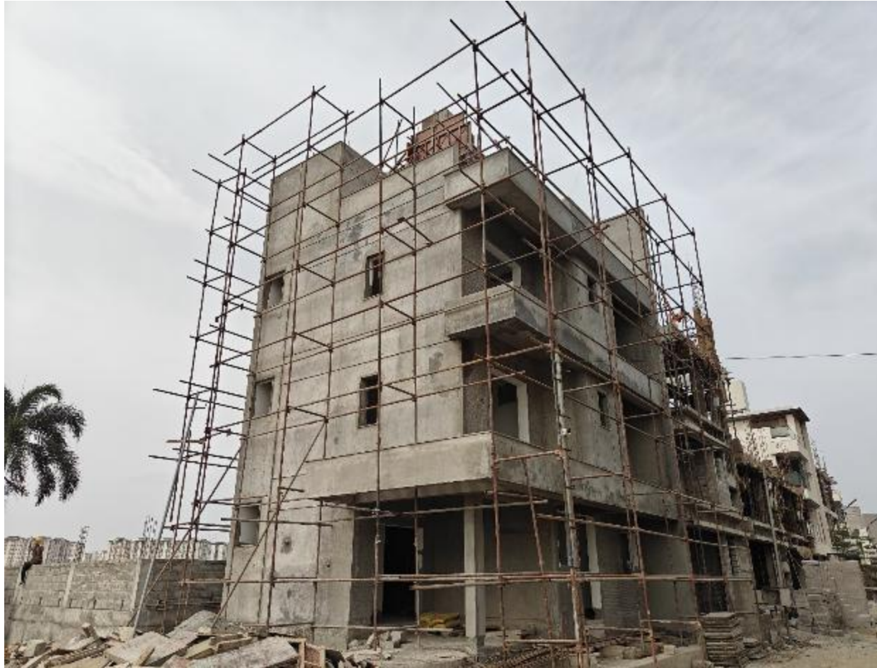
Villa No 12 – External plastering work in progress
