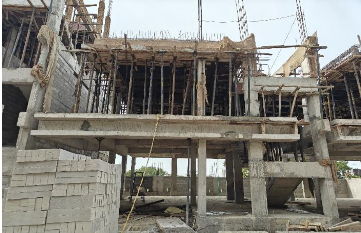
Villa No 14 – FF Roof slab concreting work completed
