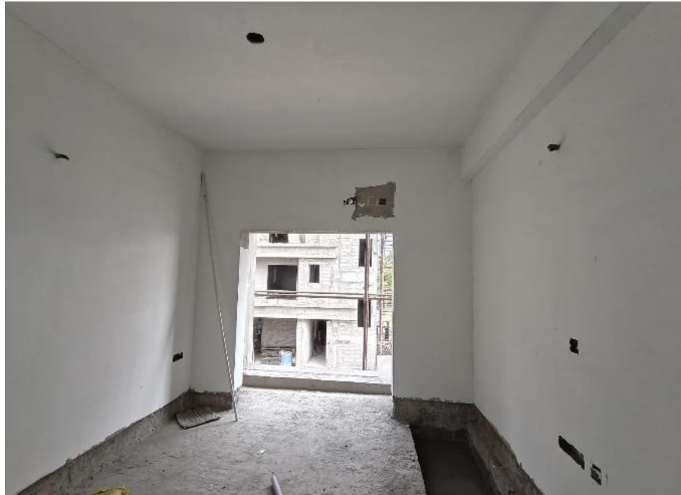
Villa No 12 – FF Bedroom Wall putty 1 st work in progress
