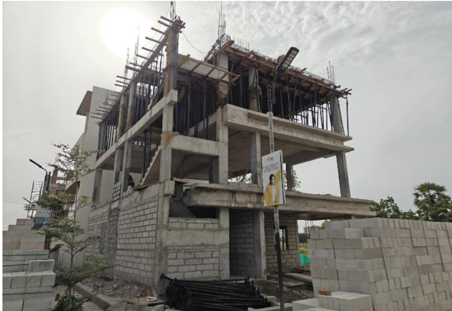
Villa No 17 – SF Roof slab reinforcement work in progress
