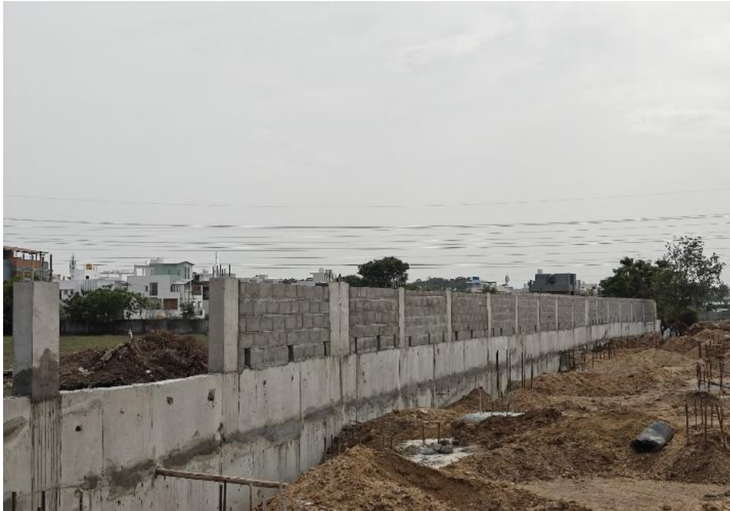
South Side Compound wall blockwork in progress
