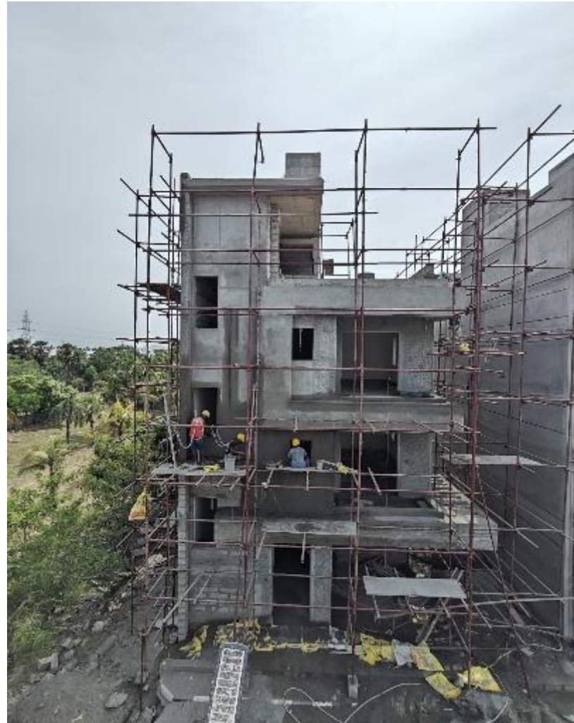
Villa No 4 - External plastering work in progress
