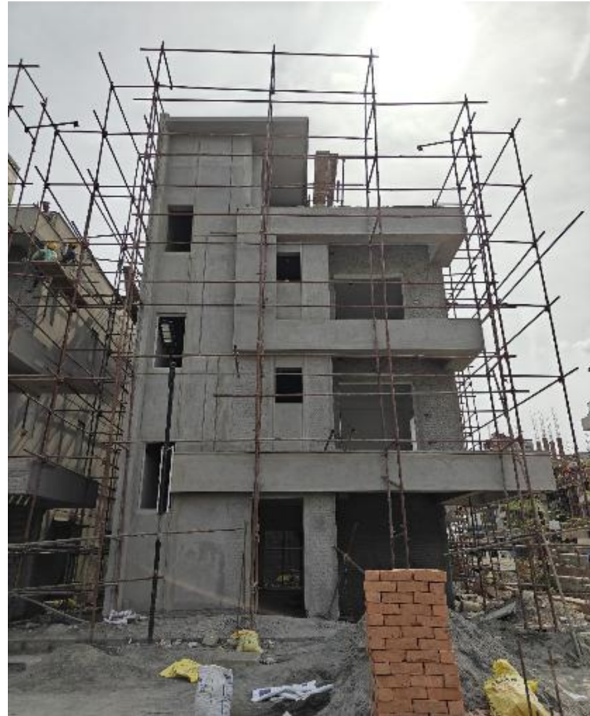
Villa No 5 – External plastering work in progress
