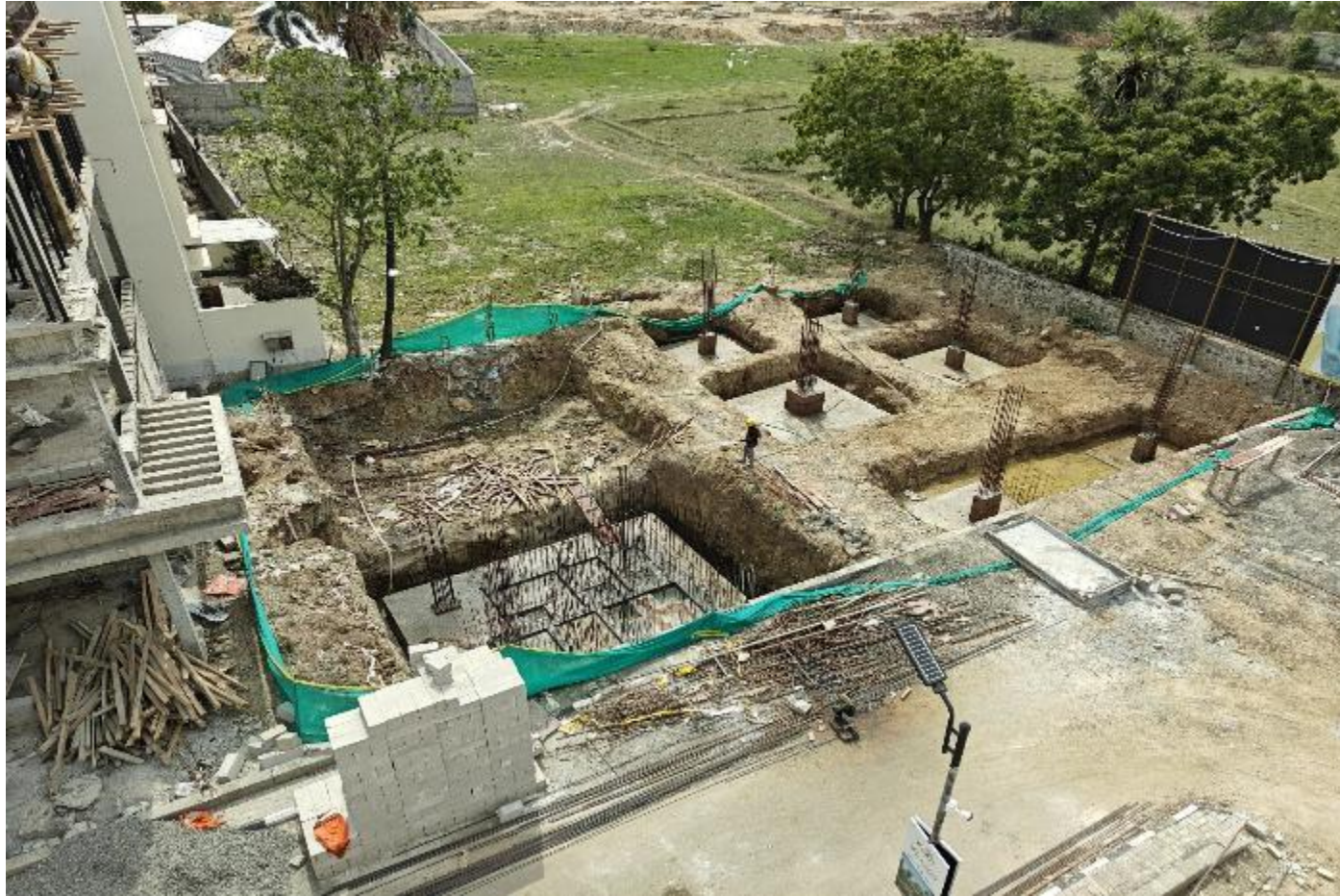
Clubhouse sub-structure column concreting work completed
