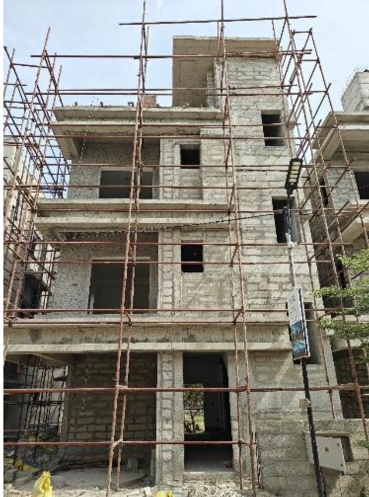
Villa No 6 – External plastering work in progress
