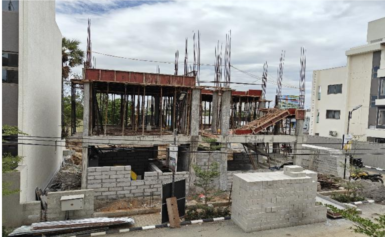
Villa No 17 – FF Roof slab shuttering work in progress
