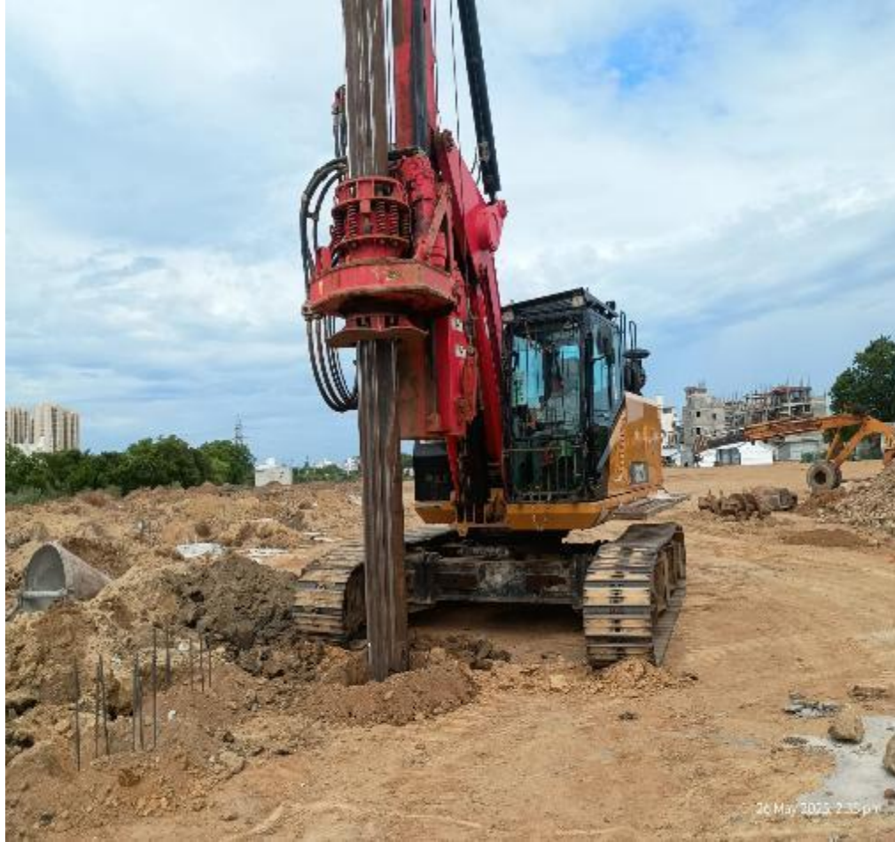
Phase-2 Pile Boring and concrete casting Work in progress
