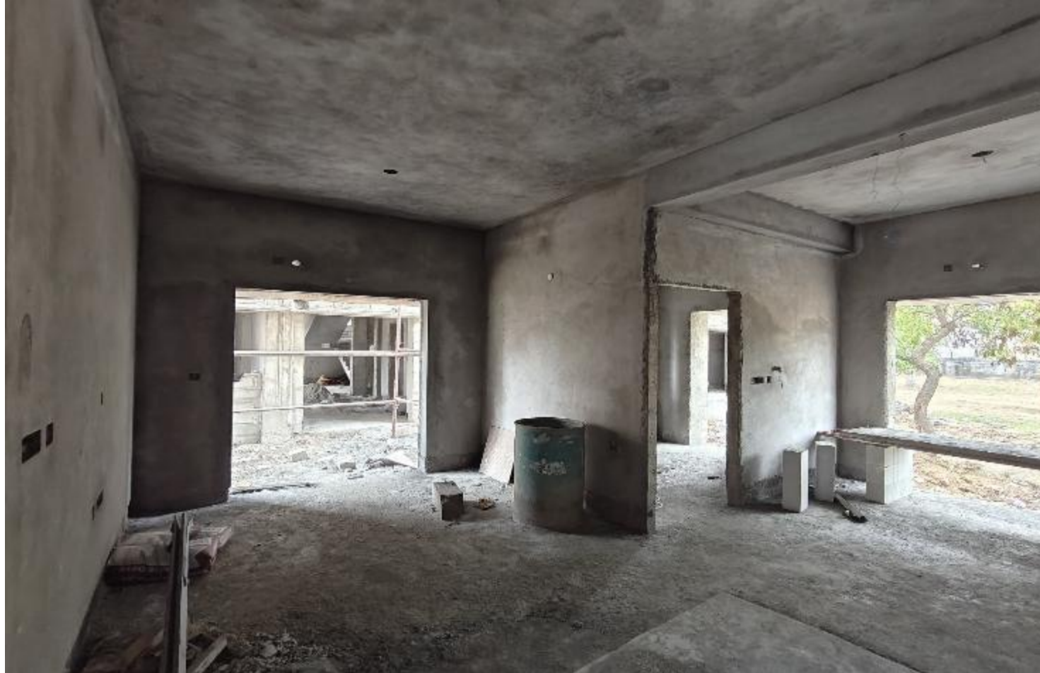
Villa No 6 – GF Living hall plastering work in progress
