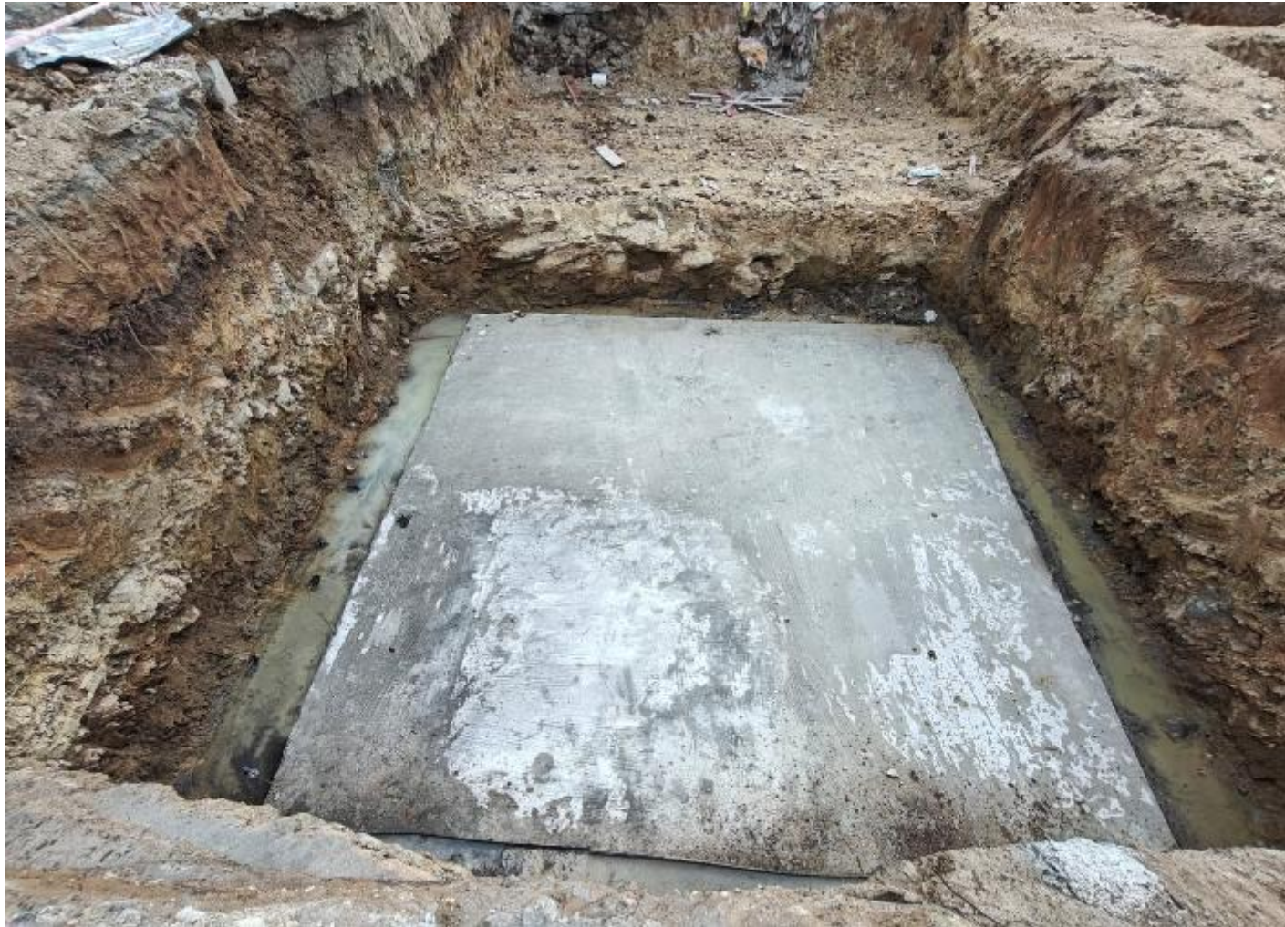
Villa No 18,19 – STP Levelling course PCC Laying work completed
