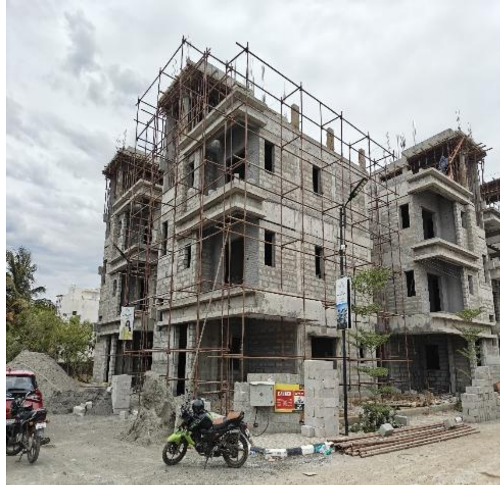
Villa No 5 - External Scaffolding Fixing work in progress
