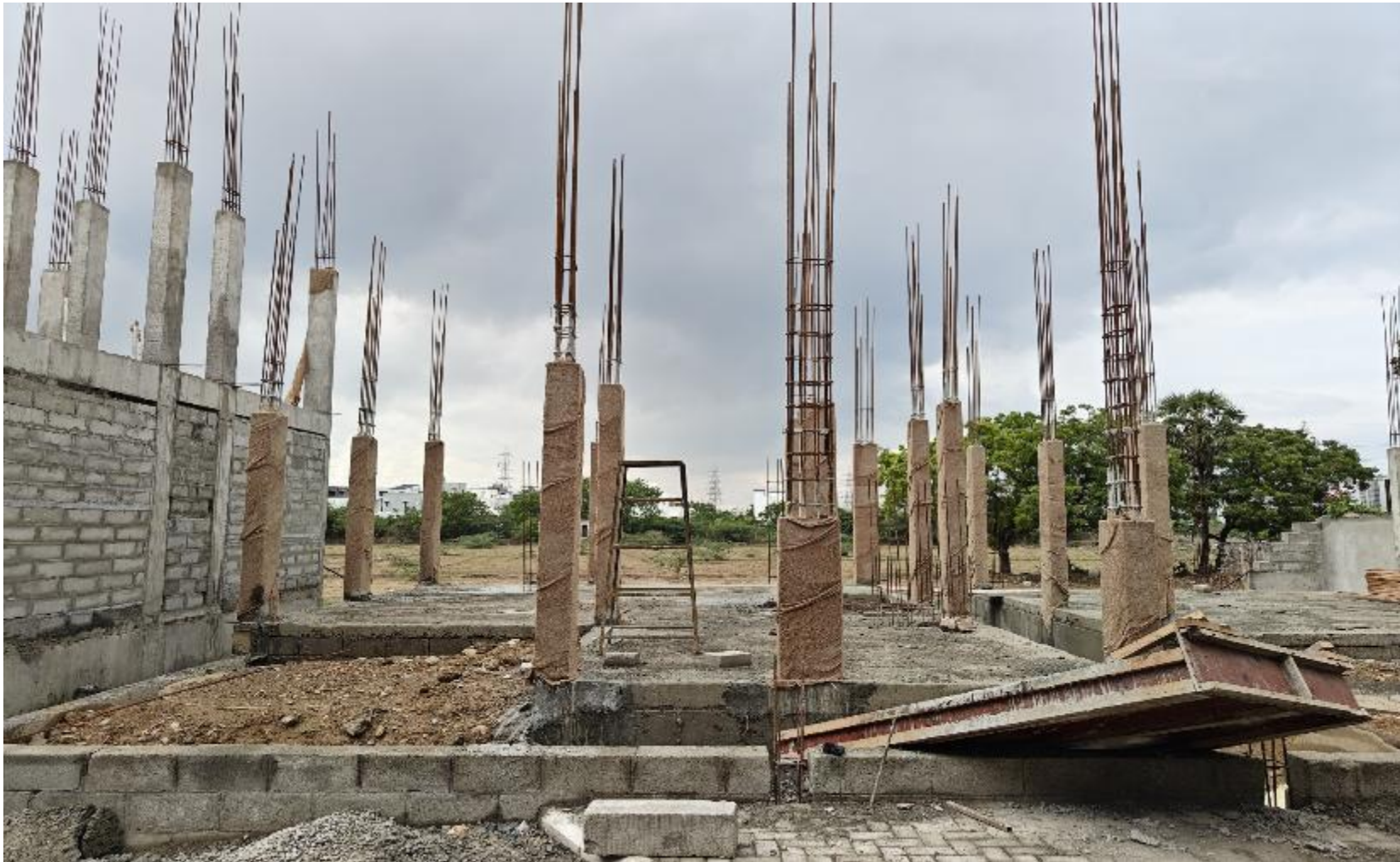
Villa No 14–GF Column concreting work completed
