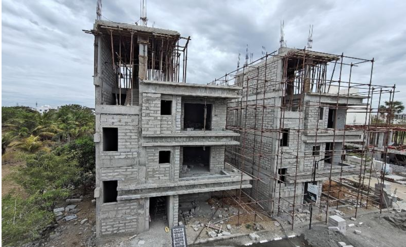
Villa No 4 & 5 Front Elevation View
