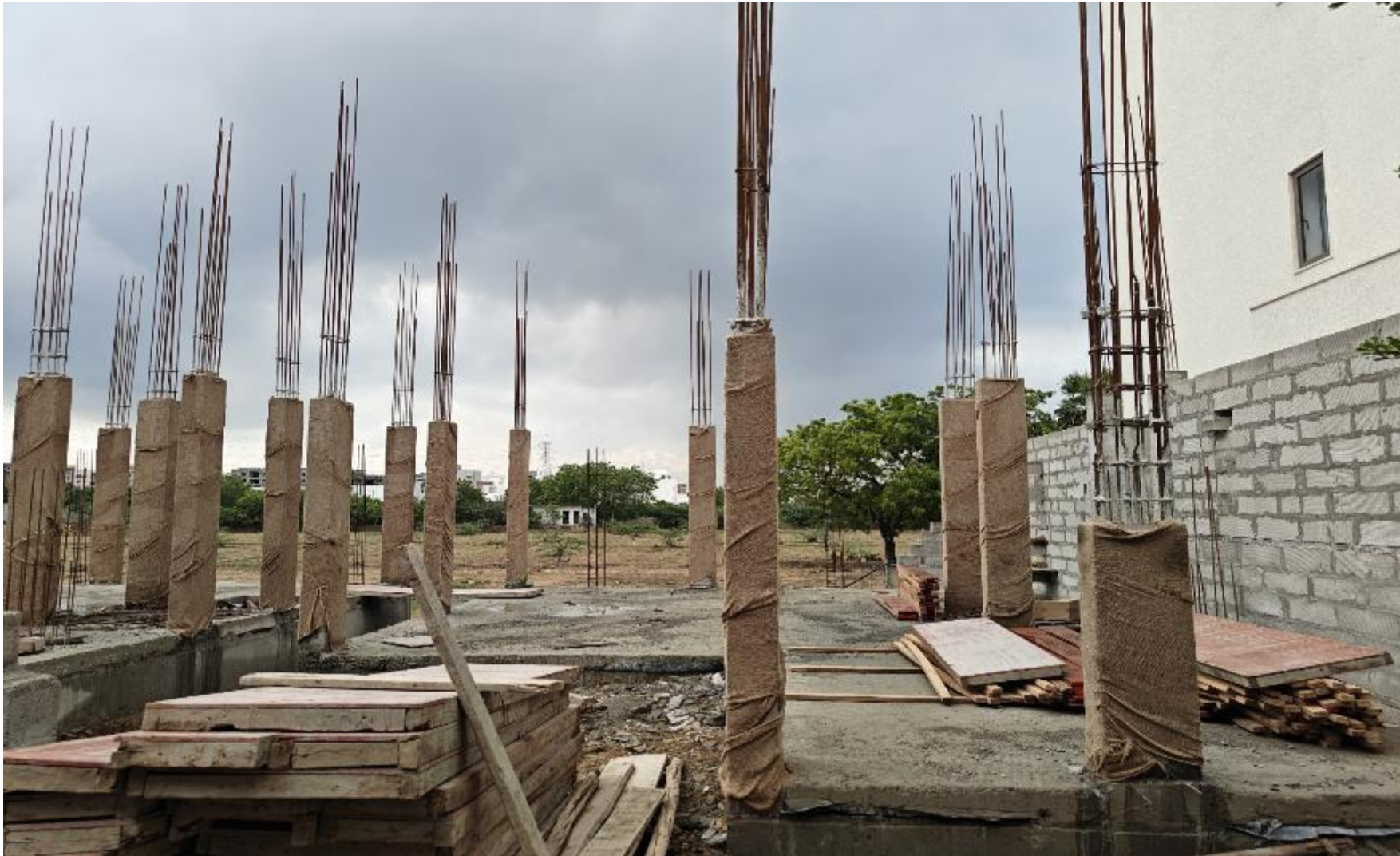
Villa No 15– GF Column Concreting work completed
