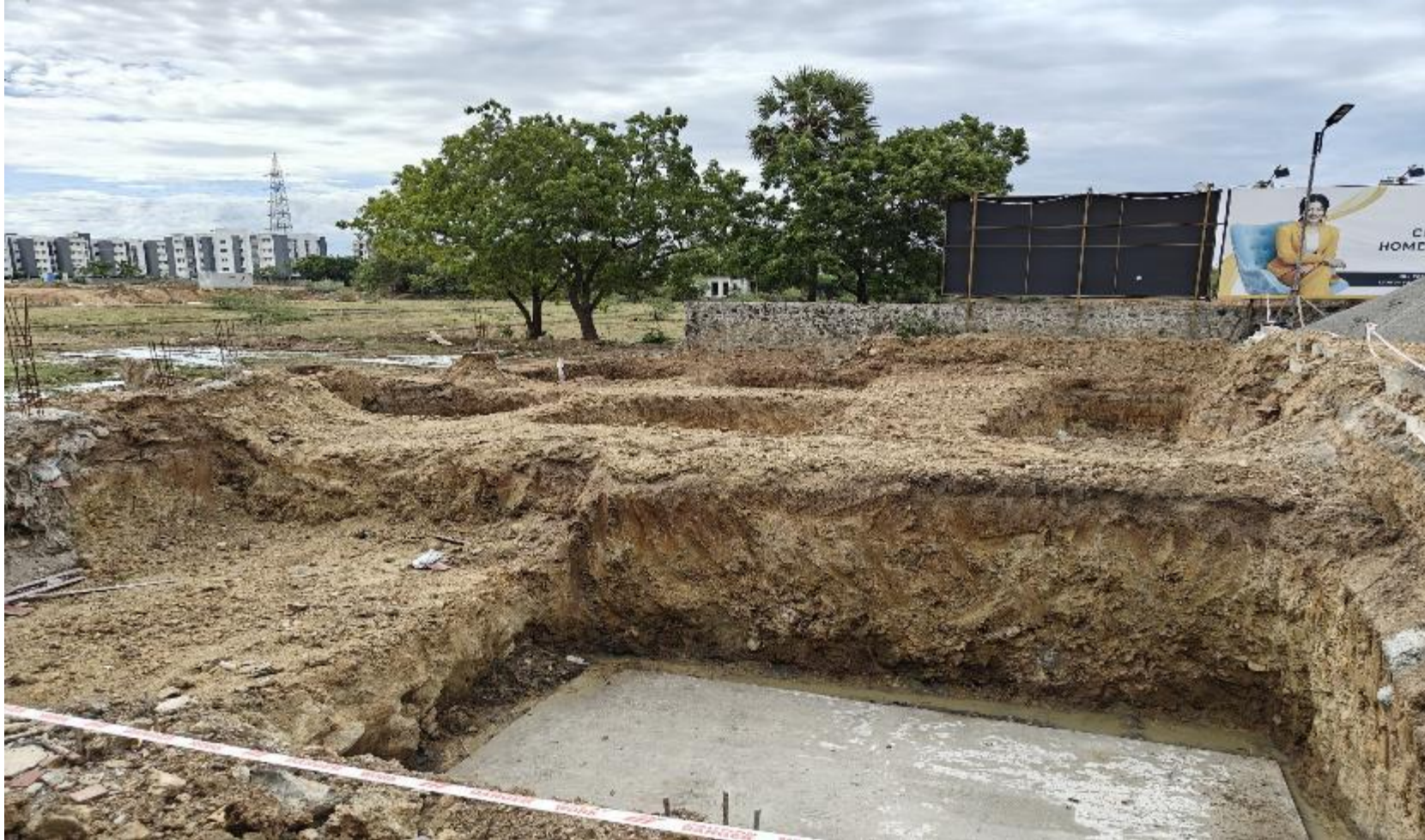
Villa No 18,19 – CLUBHOUSE & STP Soil Earthwork Excavation in progress
