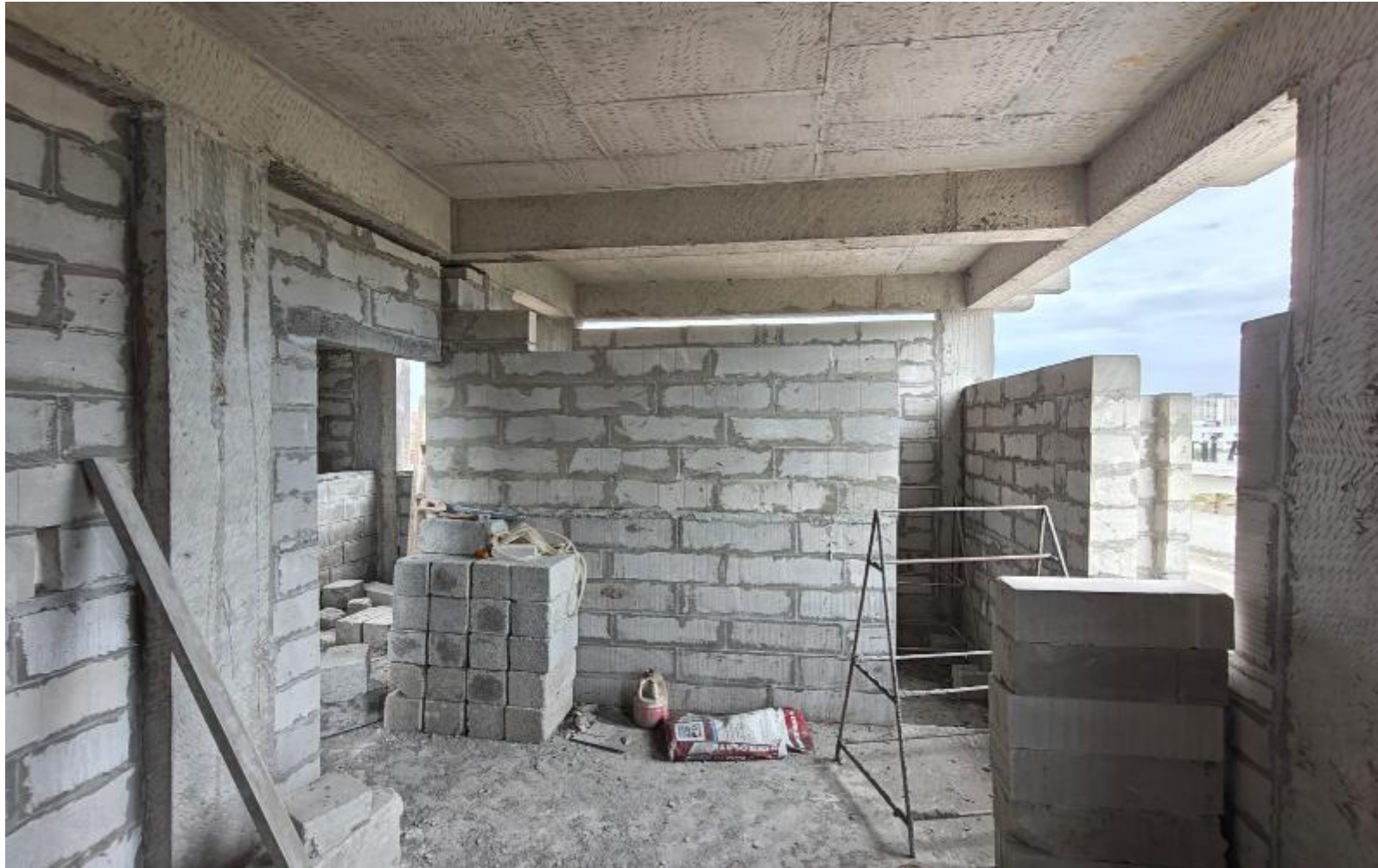
Villa No 3- SF Bedroom Blockwork in progress
