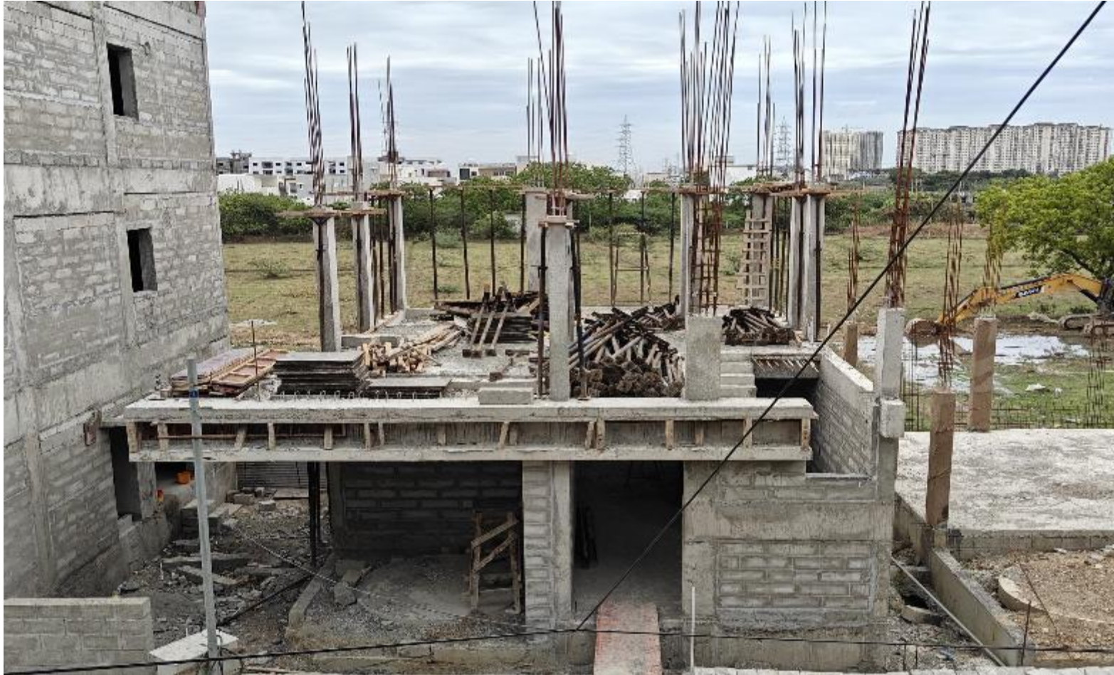
Villa No 13 – FF Roof slab beam bottom shuttering work in progress
