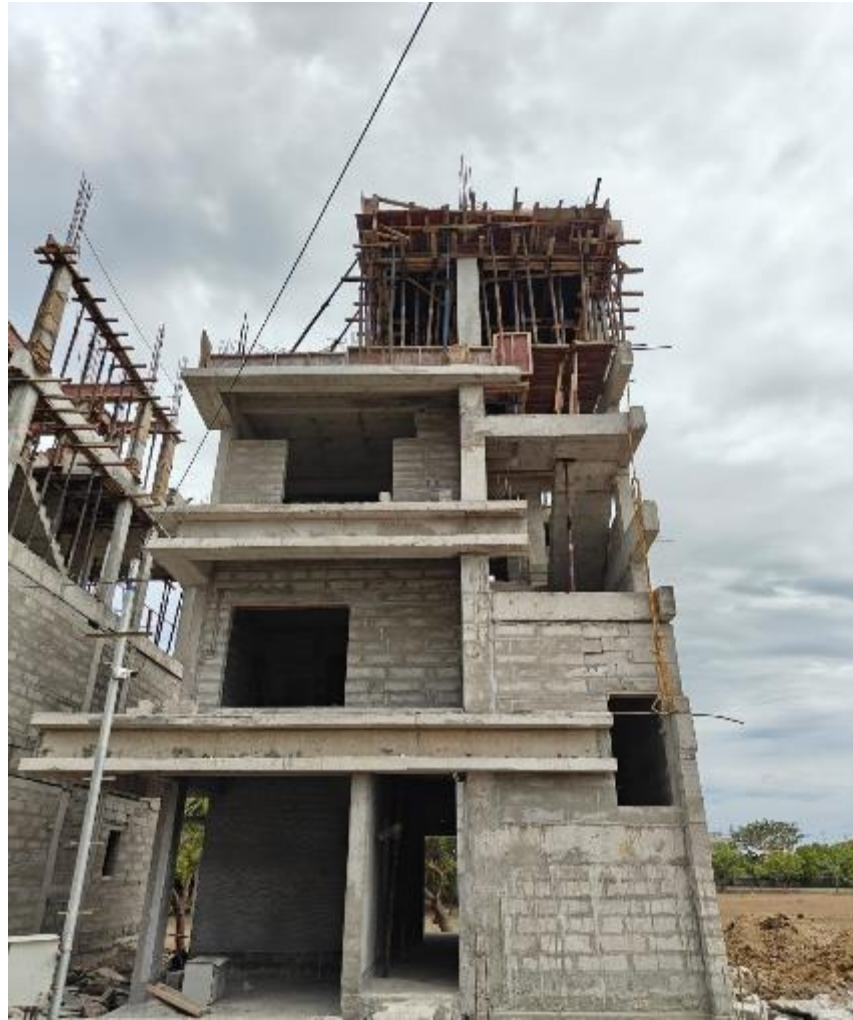
Villa No 11- Front Elevation view
