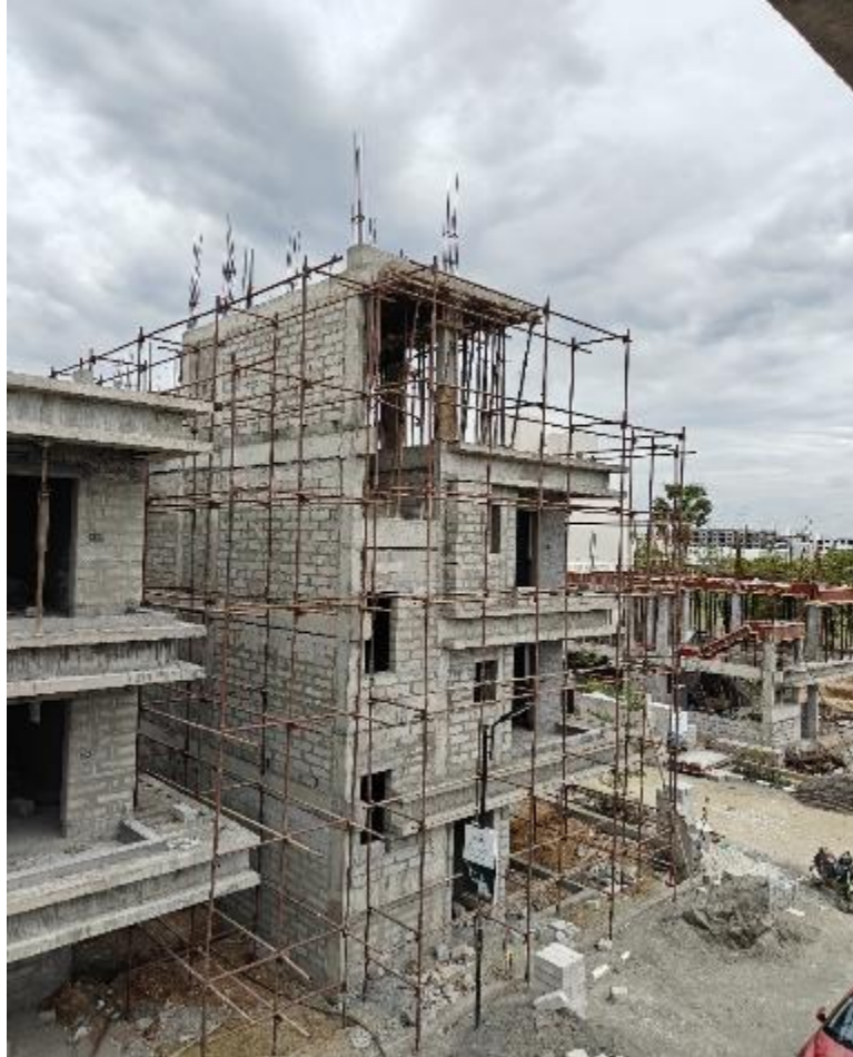
Villa No 5 - External Scaffolding Fixing work in progress
