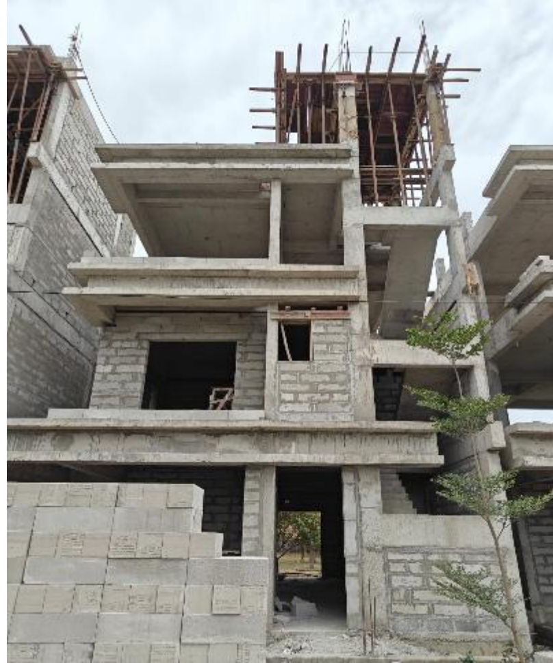
Villa No 7- Front Elevation view
