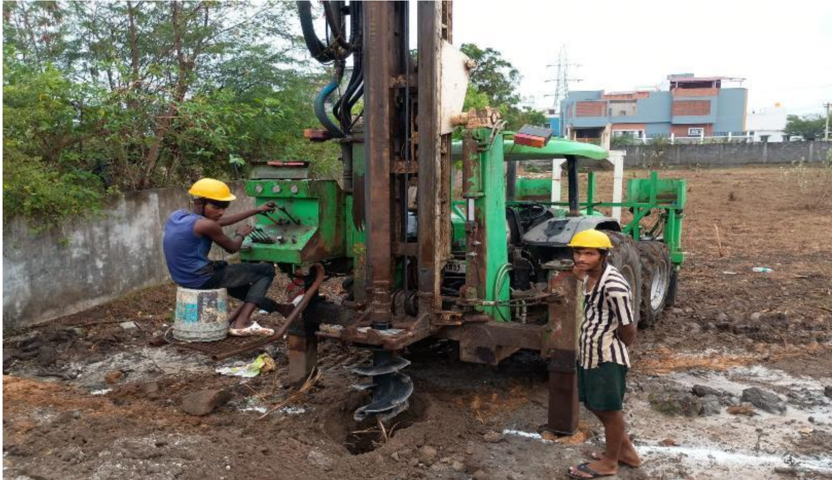
Phase-2 Boundary compound wall Pile boring Work in progress
