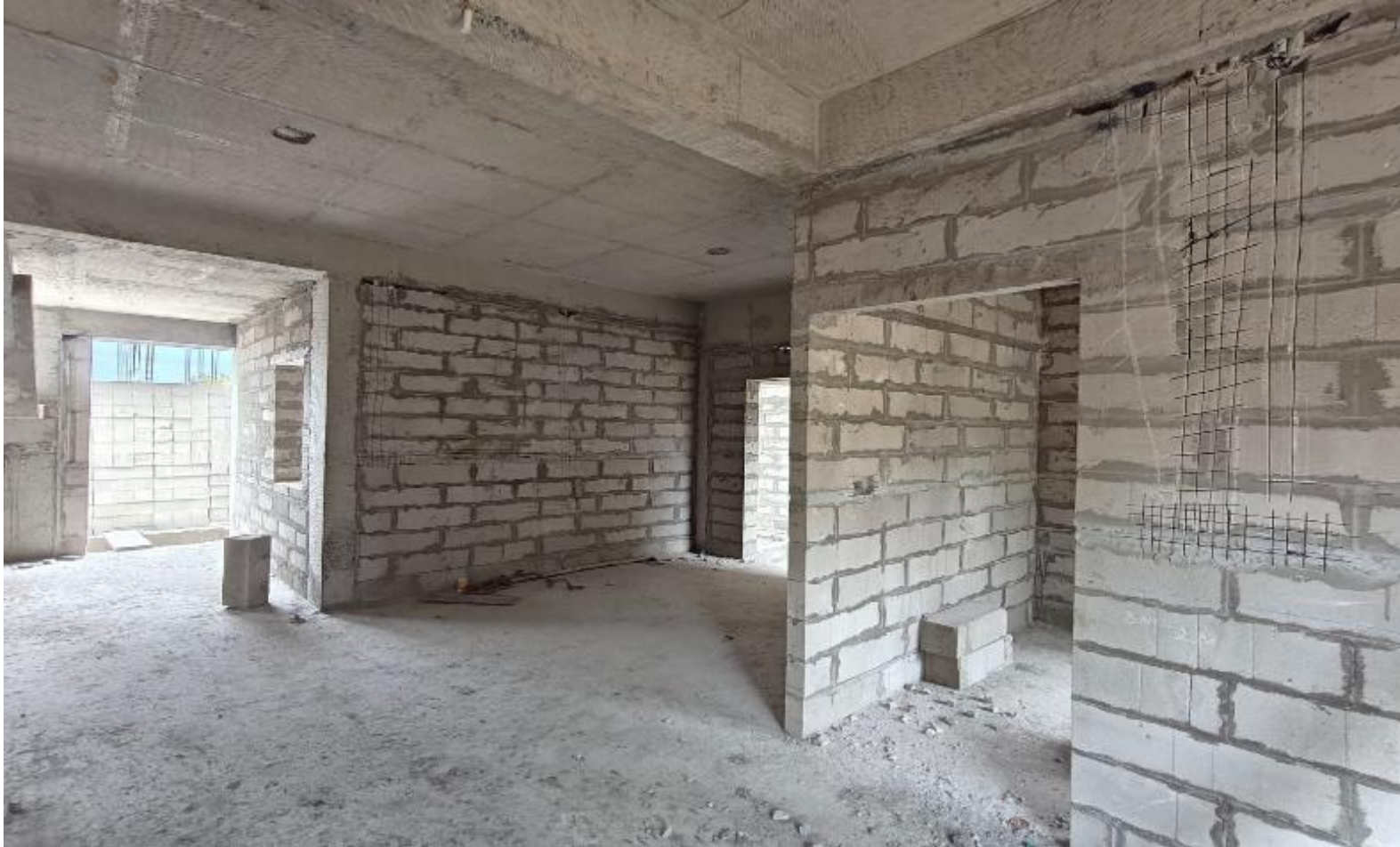
Villa No 8- GF Living hall Electrical Wall Chasing work in progress
