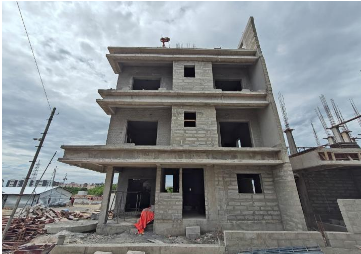
Villa No 12 – Front Elevation view
