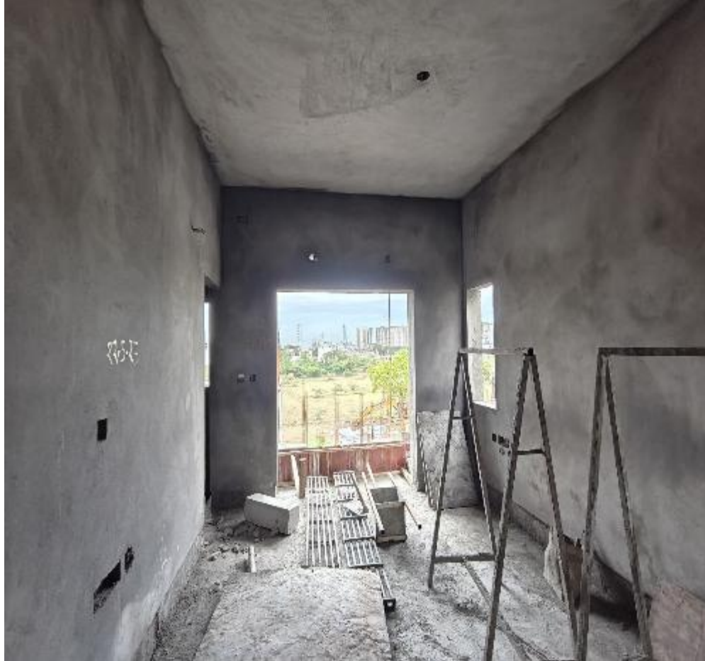
Villa No 9 – SF Bedroom 1&2 Internal wall plastering work in progress
