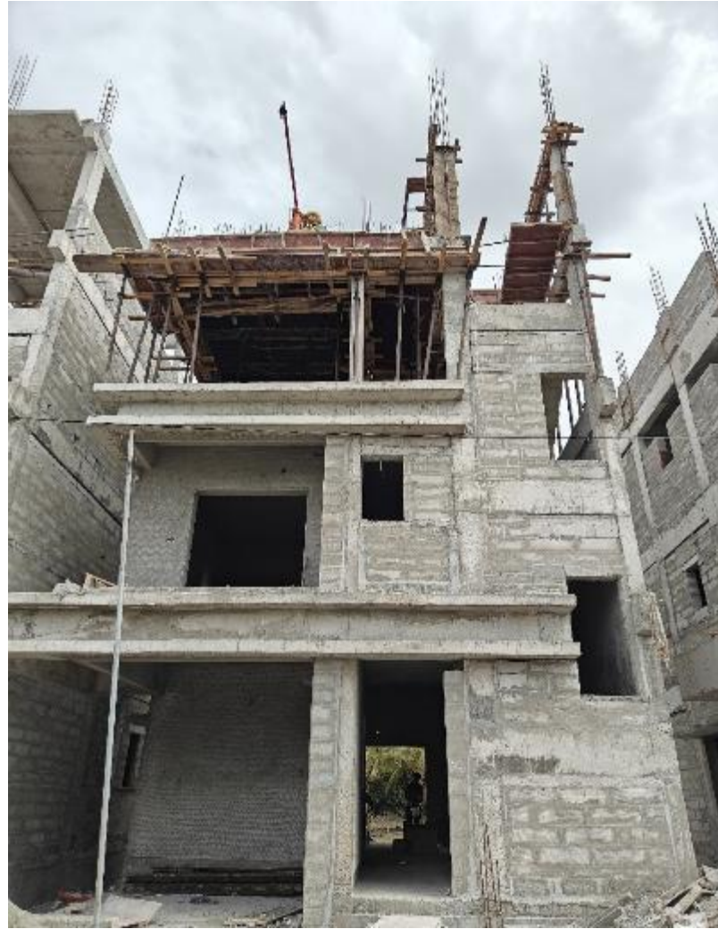
Villa No 10- Front Elevation view
