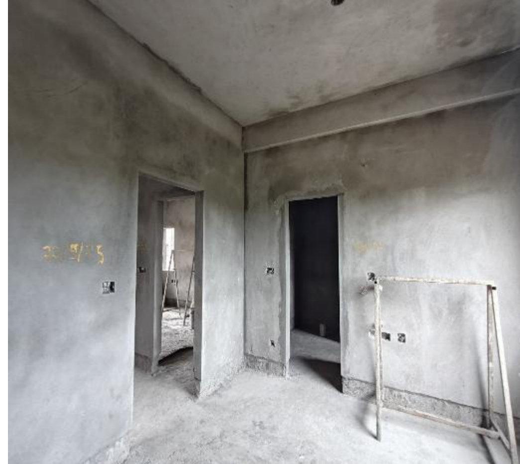
Villa No 9 – SF Bedroom 1&2 Internal wall plastering work in progress
