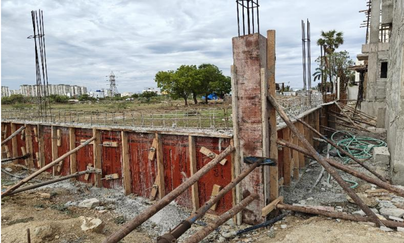
Phase-1 Compound RCC wall concreting work in Progress
