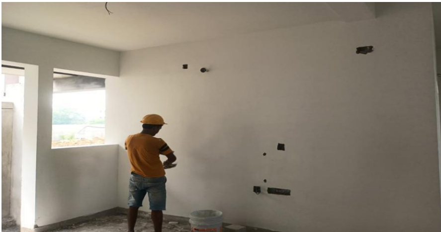
Villa 12 2 nd Coat Putty Applying Progress
