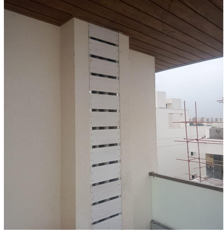
Villa 4 to 10 Plumbing Shaft Cera Board Fixing Work Completed
