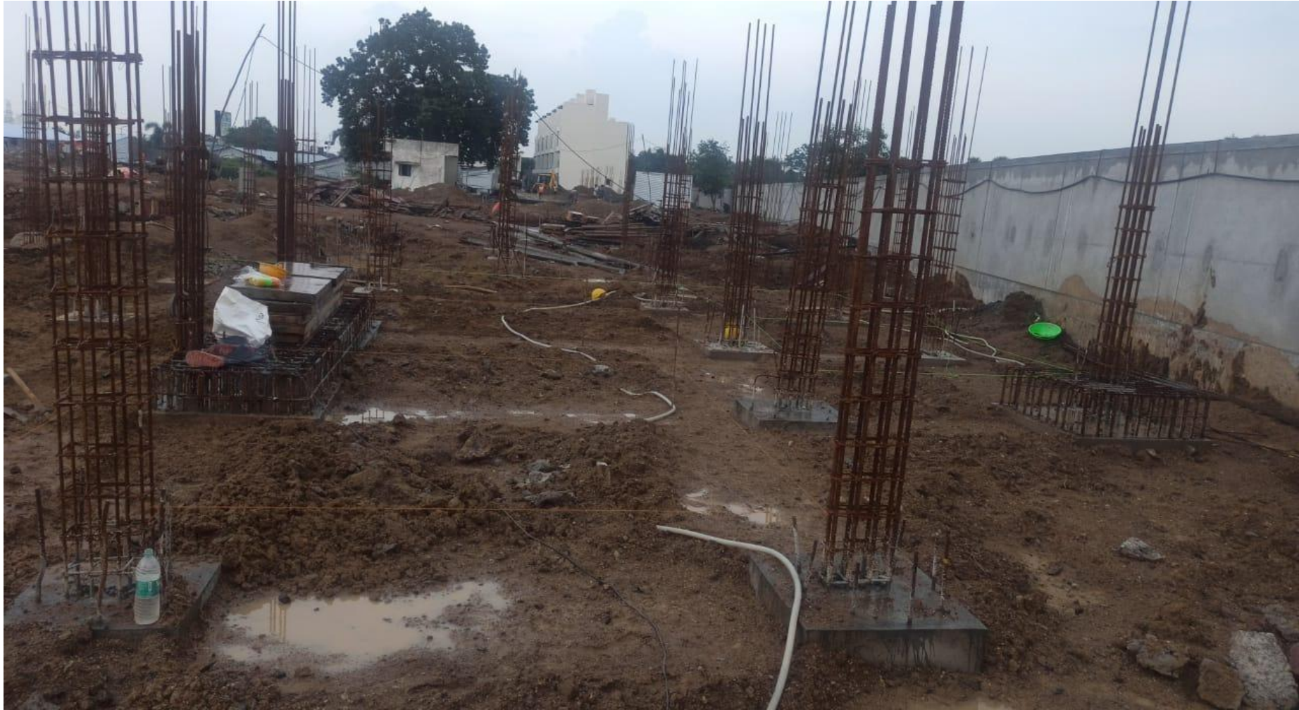
Phase 2 – villa no 45 Plinth Beam PCC Preparation Work On Progress
