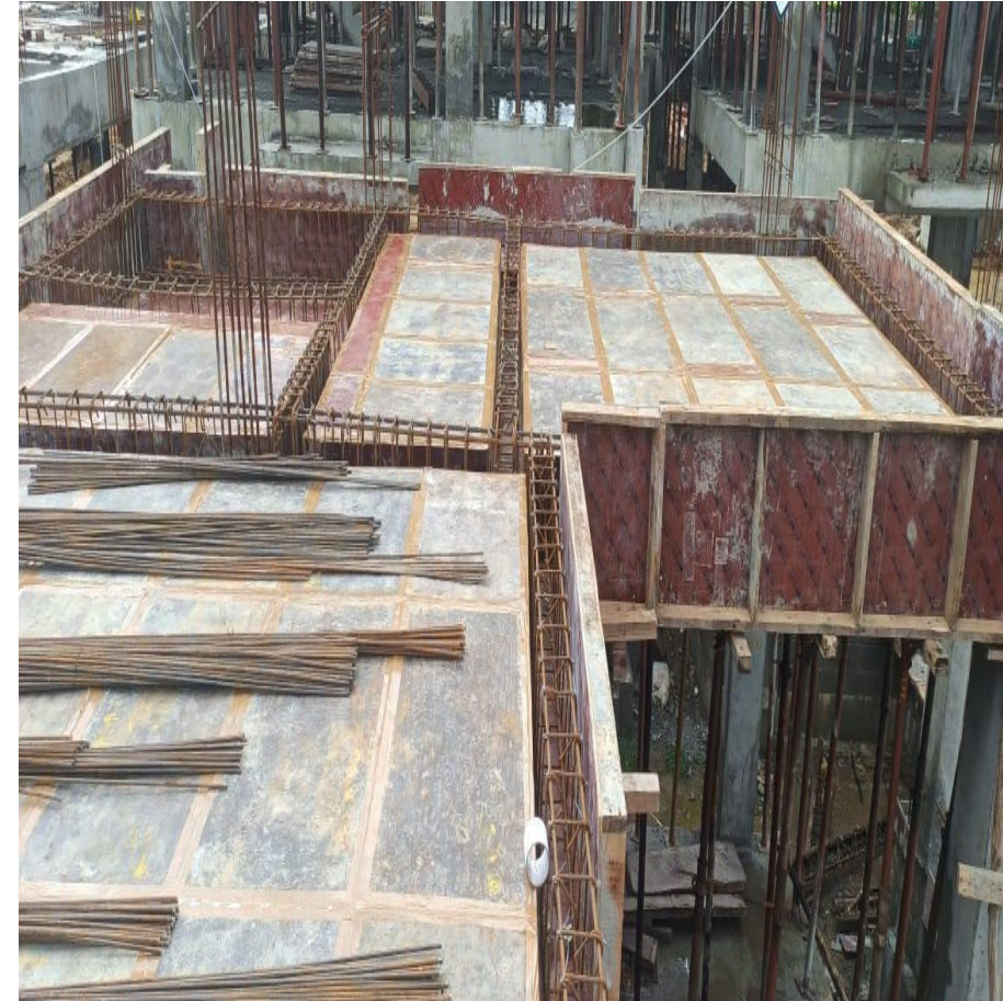
Villa 57 GF Roof Slab Reinforcement Work On Progress
