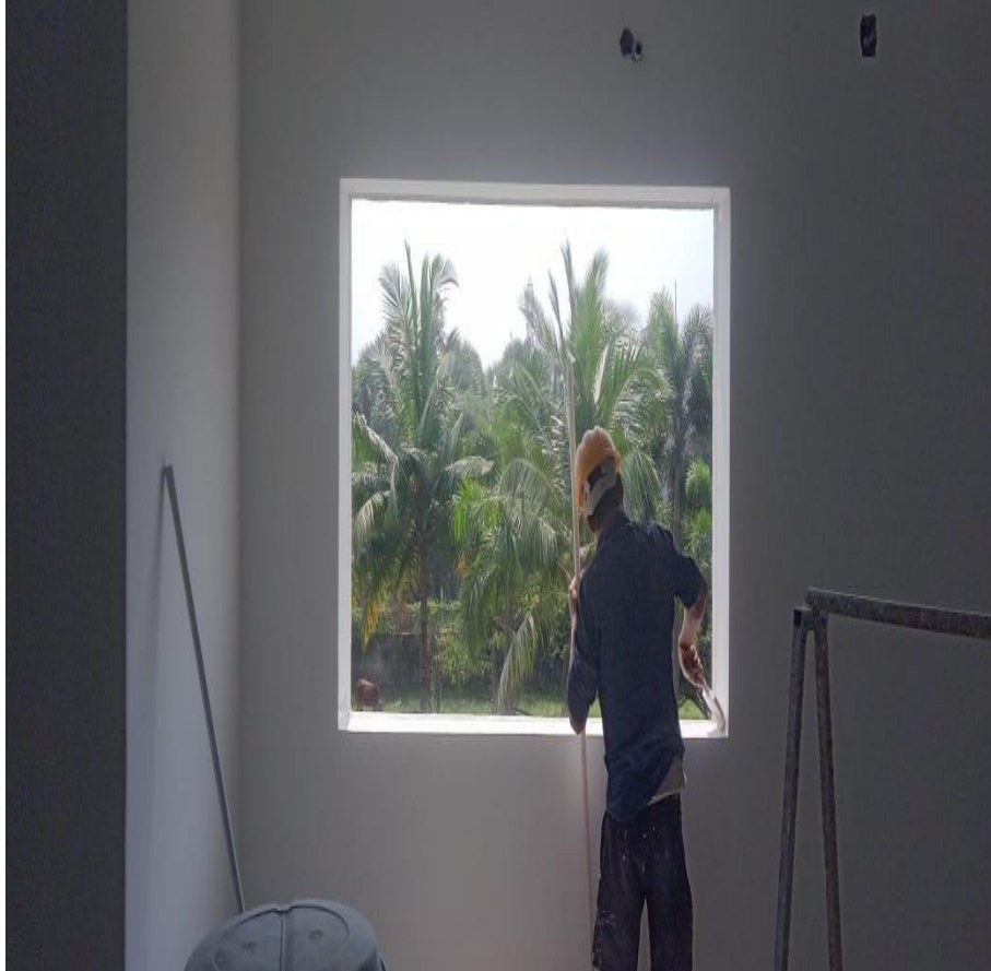
Villa 9 SF Primer Applying Work On Progress
