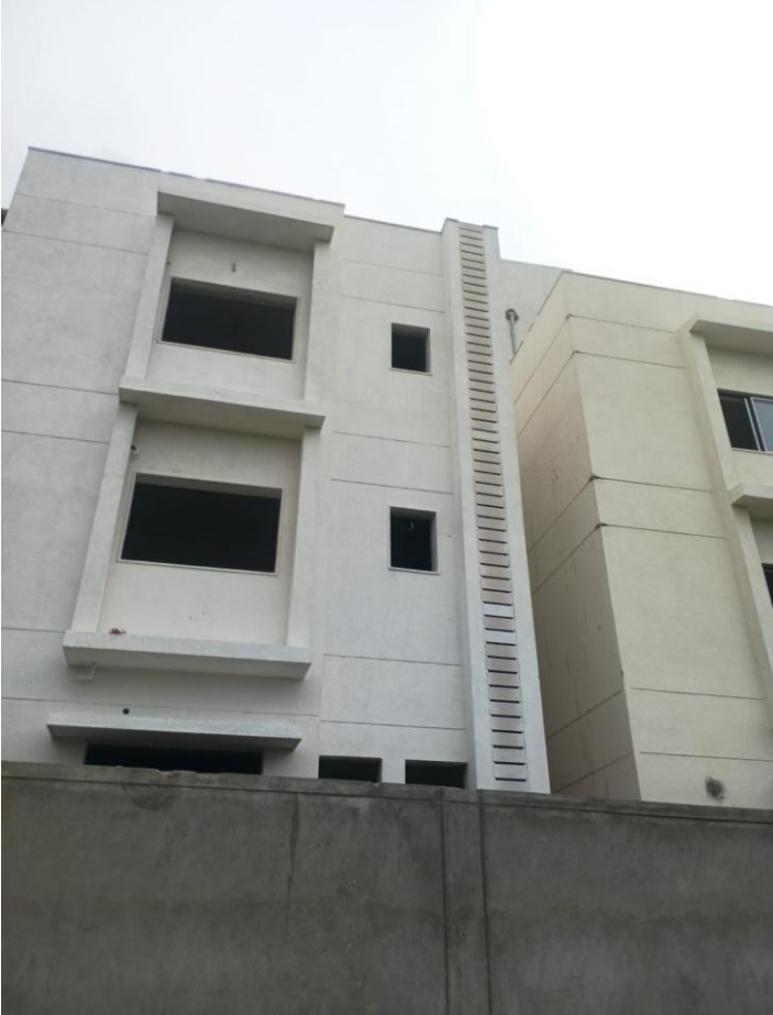
Villa 14 Plumbing Shaft Cera Board Fixing Work Completed
