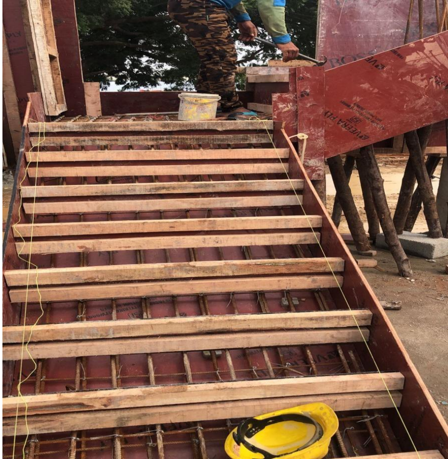
Villa 29 Staircase Shuttering Work On Progress
