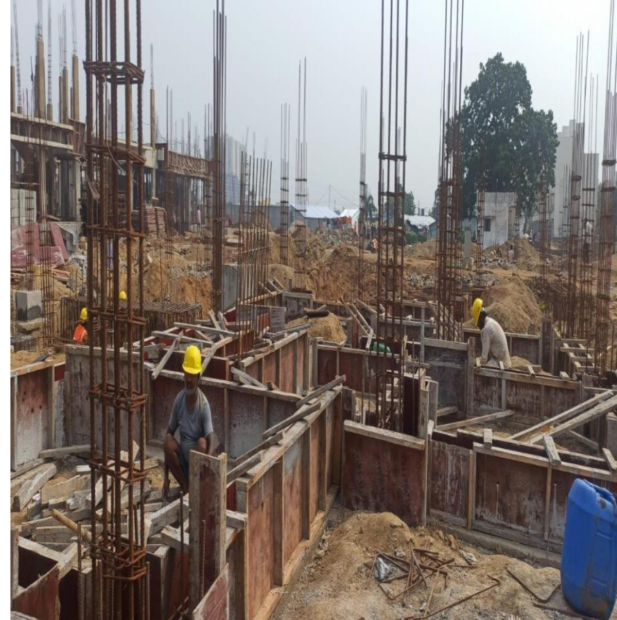
Villa 44 Plinth Beam Shuttering Work Progress
