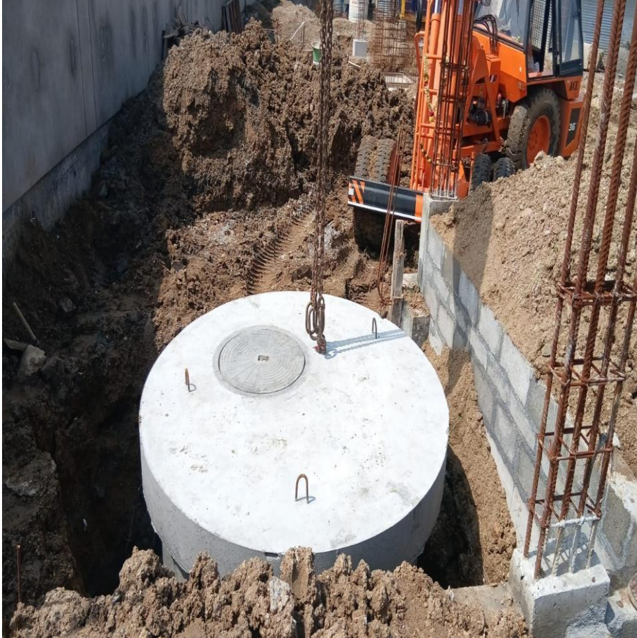
Villa 45 UG Sump Fixing Completed
