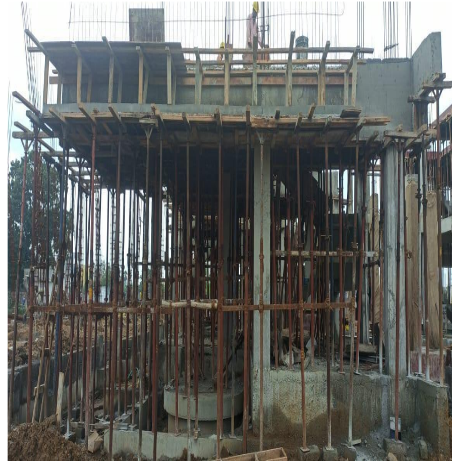
Villa 56 GF Roof Slab Concrete Work Completed
