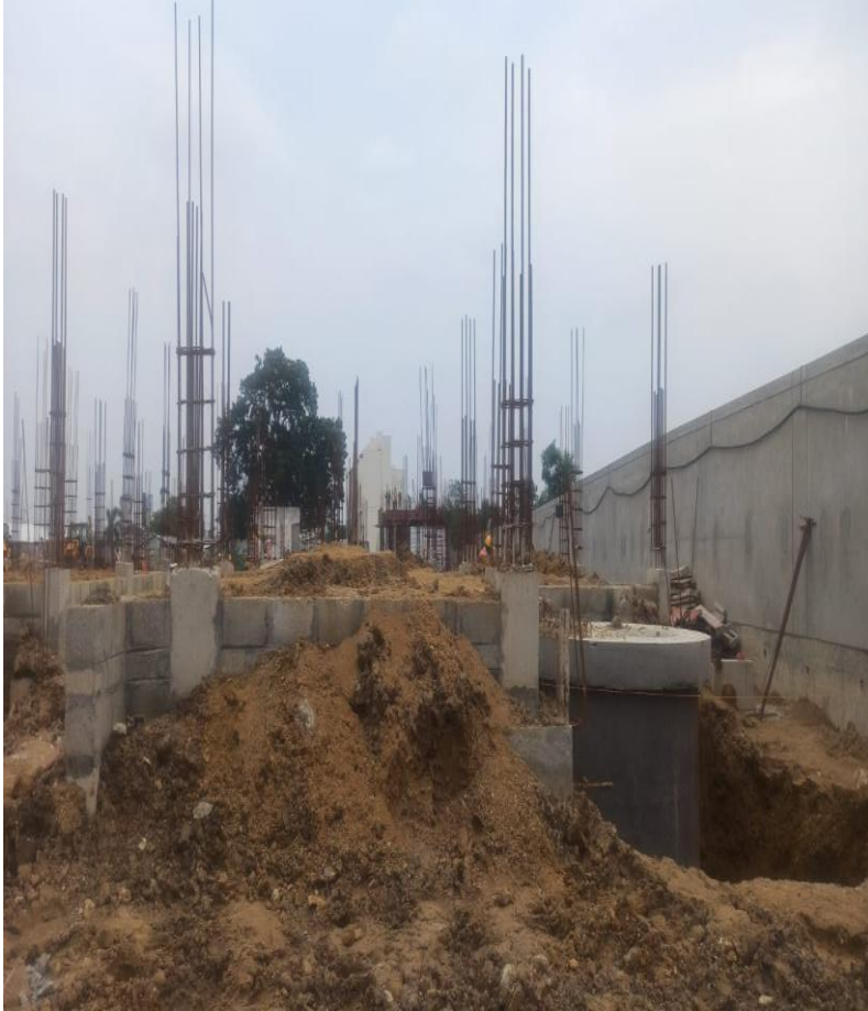
Villa 45 Basement Back Filling Work On Progress
