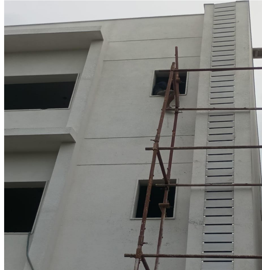
Villa 15 Plumbing Shaft Cera Board Fixing Work Completed
