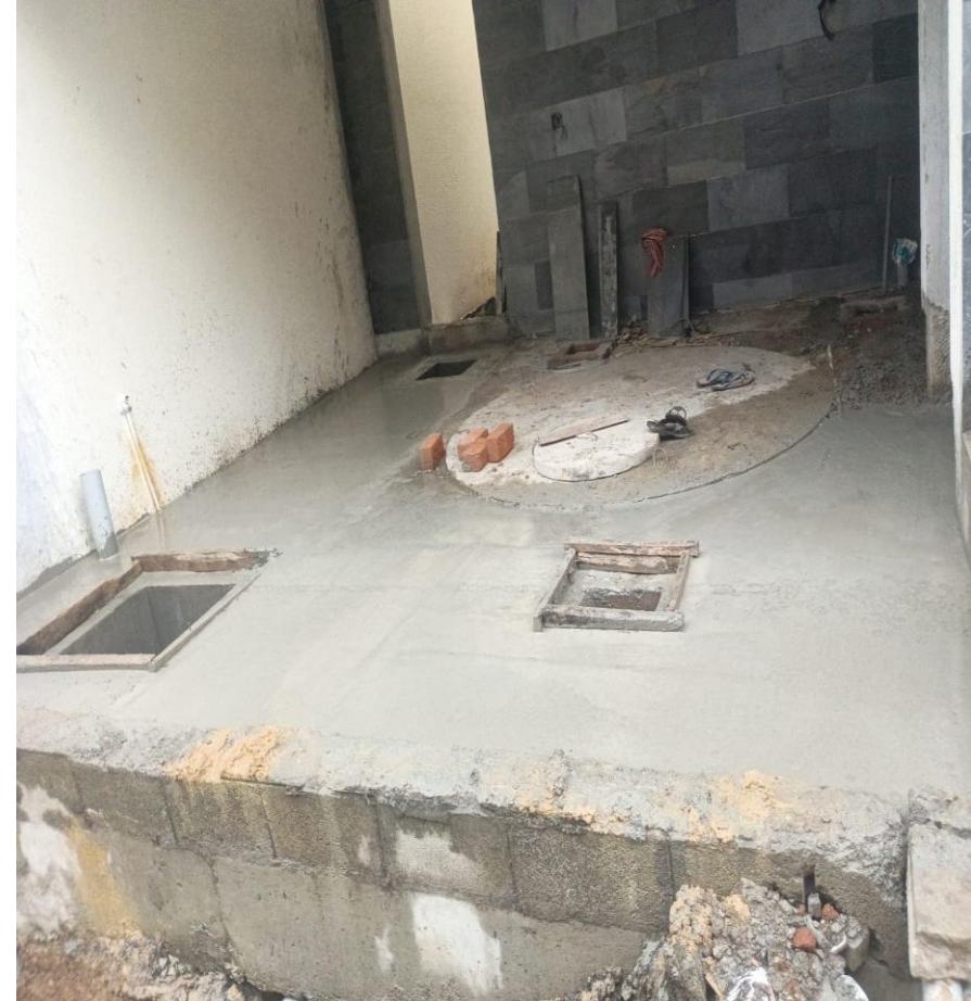
Villa 5&6&7 Carparking PCC Concrete Work Completed
