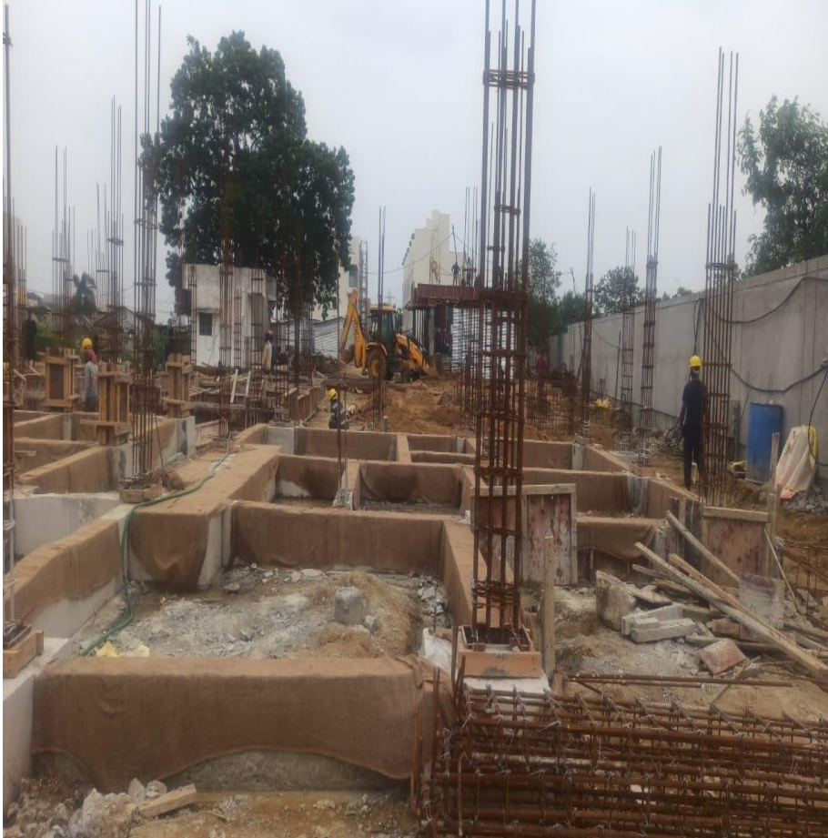
Villa 38 Plinth Beam Concrete Completed
