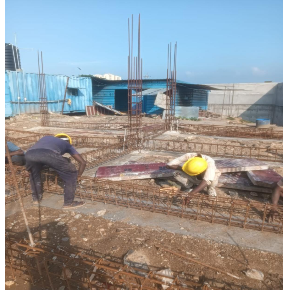
Villa 103 Plinth Beam Reinforcement Work On Progress
