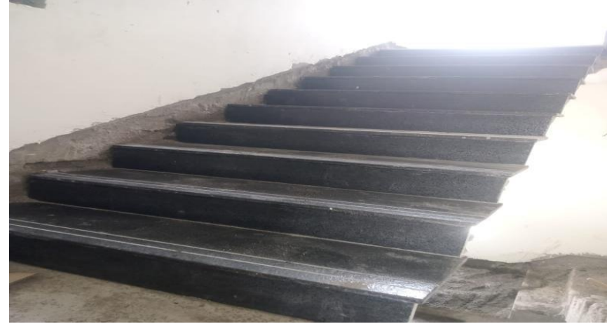
Villa 11 Staircase Granite Laying Progress
