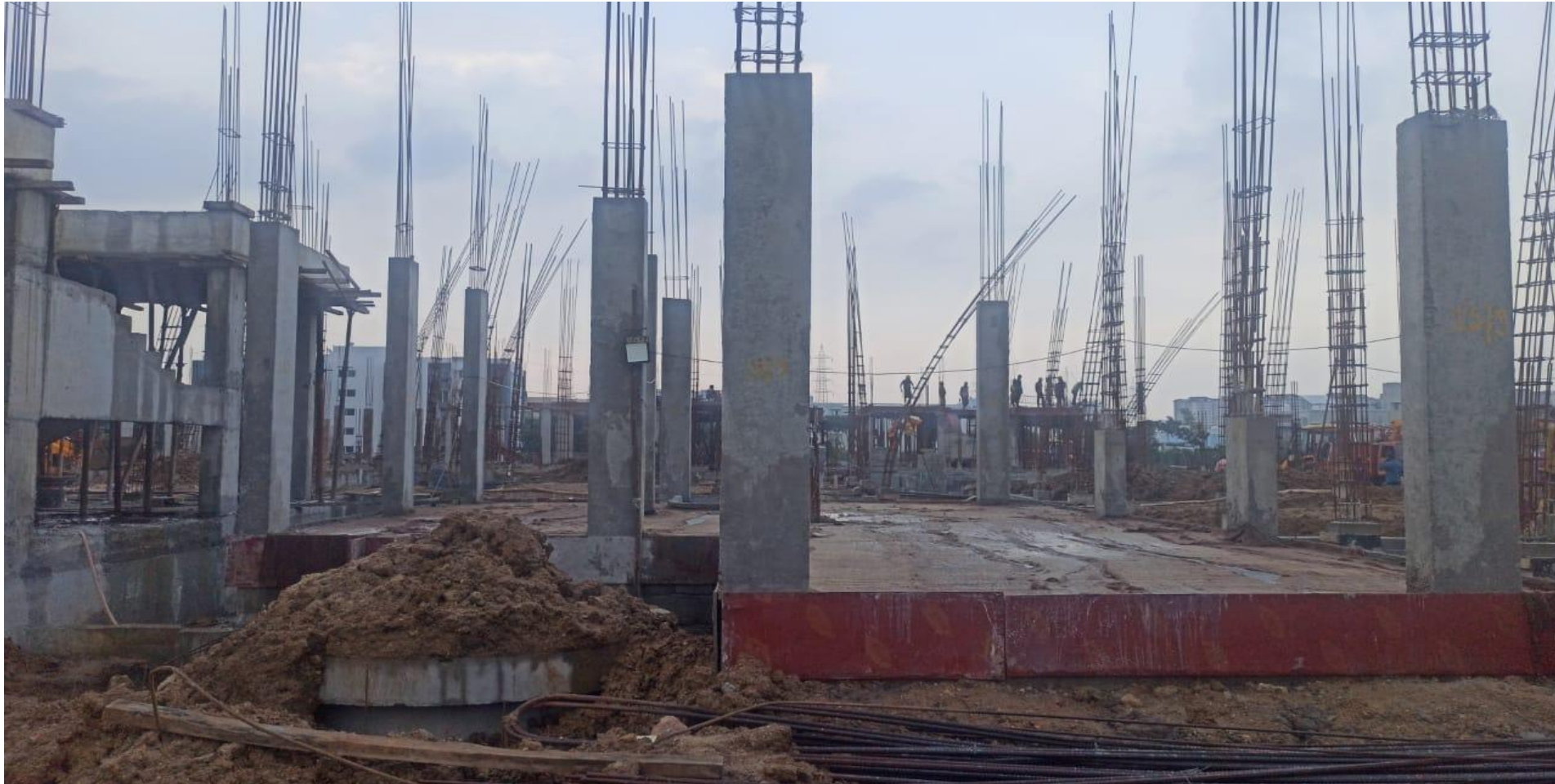
Phase 2 – villa no 52 GF Column Concrete Pouring Completed
