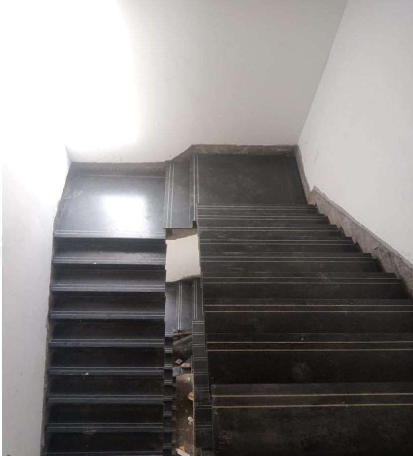
Villa 17 Staircase Granite Laying On Progress
