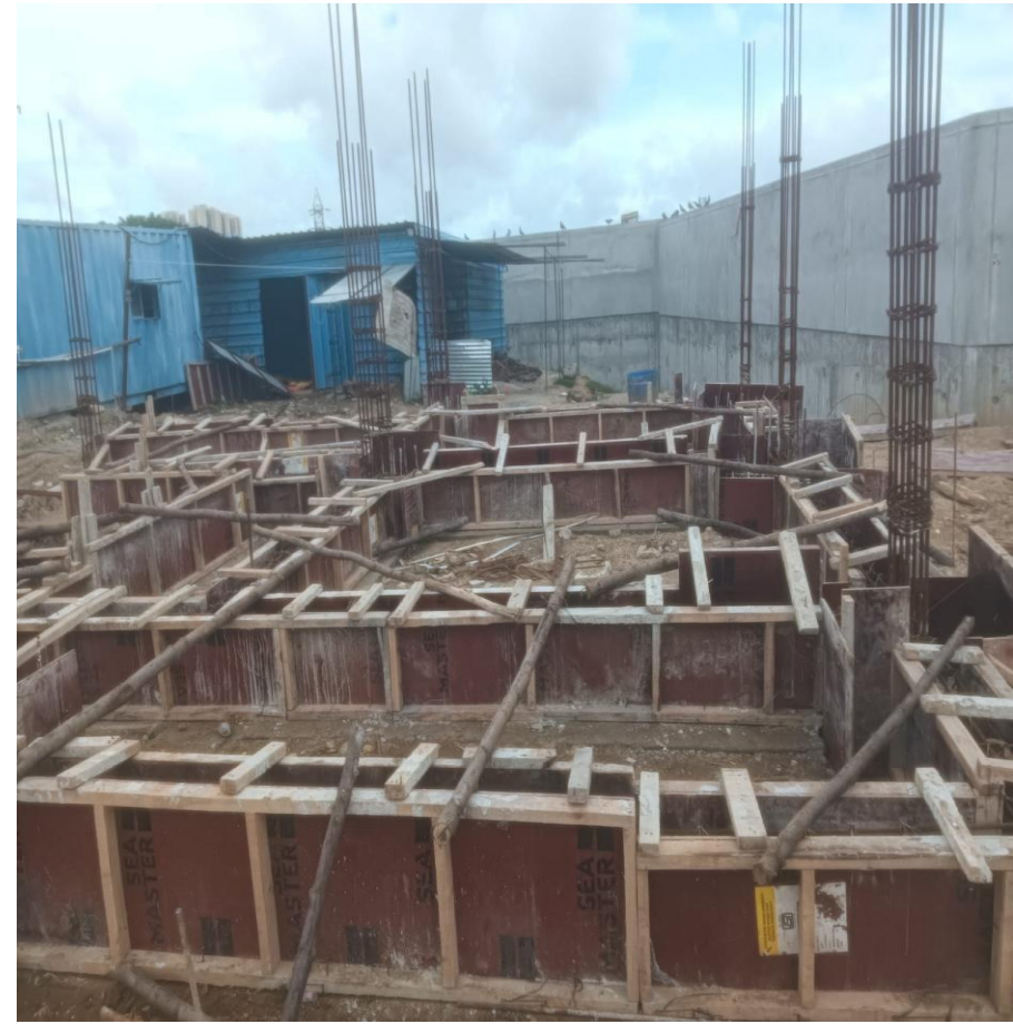
Villa 108 Plinth Beam Shuttering Work On Progress
