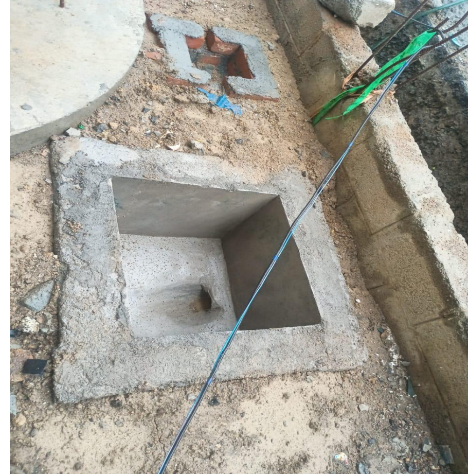
Villa 4&5&6 Manhole Chamber Plastering Work On Progress
