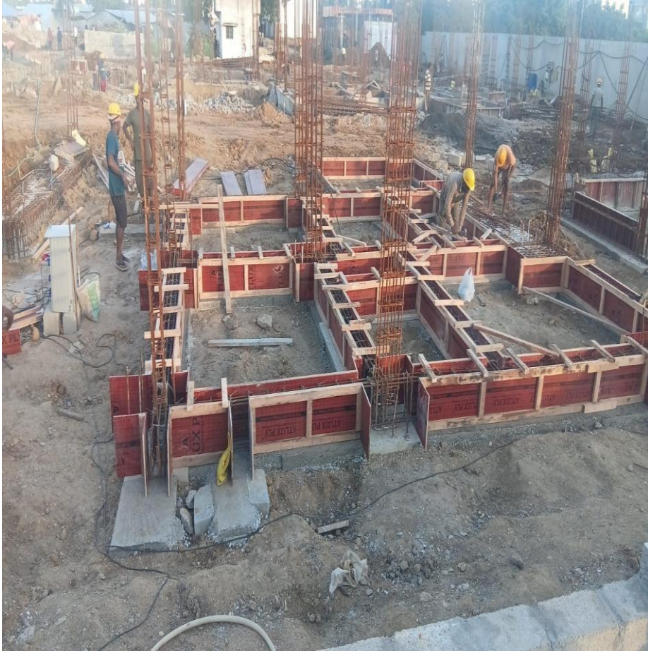
Villa 40 Plinth Beam Shuttering Work On Progress
