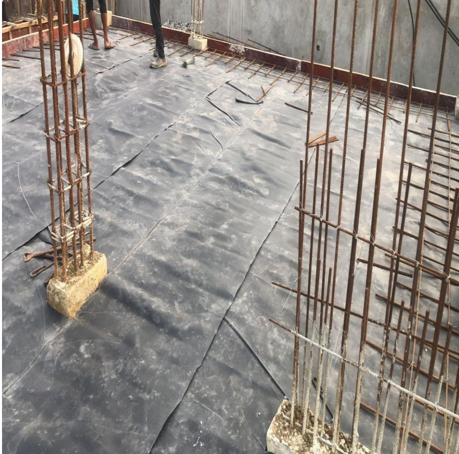
Villa 29 Basement PCC HDPE Sheet Laying Work Completed
