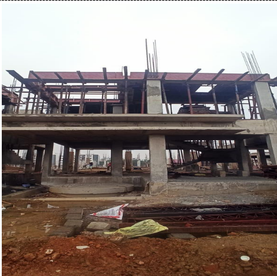
Villa 50 FF Roof Slab Shuttering Work On Progress
