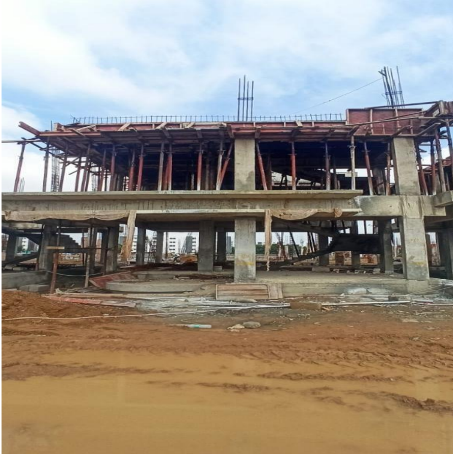
Villa 49 FF Roof Slab Concrete Completed
