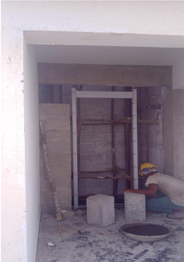
Villa 9 Lift Frame Fixing Completed
