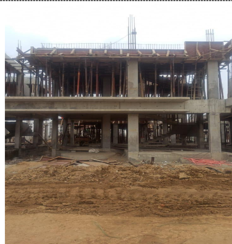
Villa 50 FF Roof Slab Concrete Work Completed
