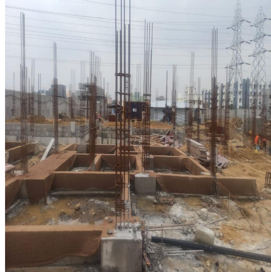
Villa 40 Plinth Beam Concrete Completed
