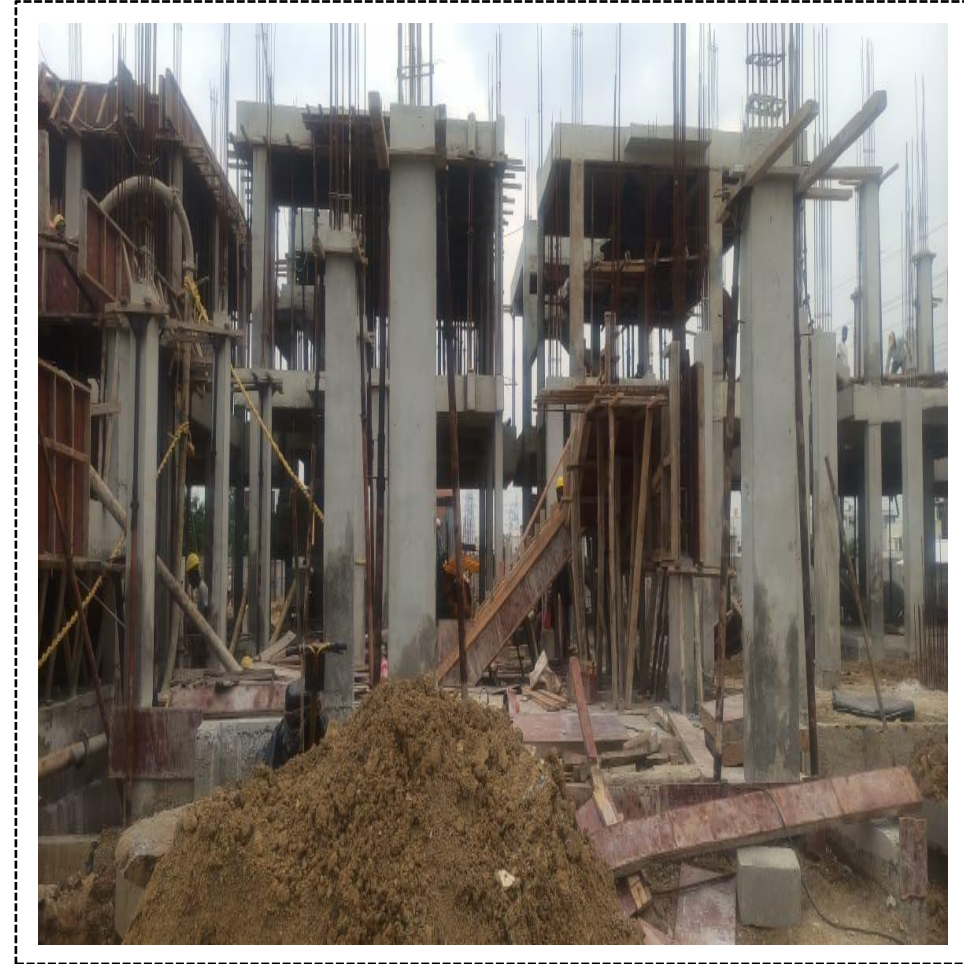
Villa 50 GF Roof Slab Shuttering Work On Progress
