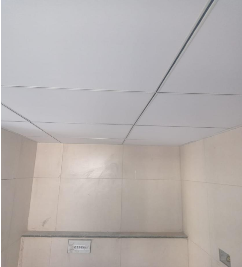
Villa 9 Toilet Grid False Ceiling Laying Completed
