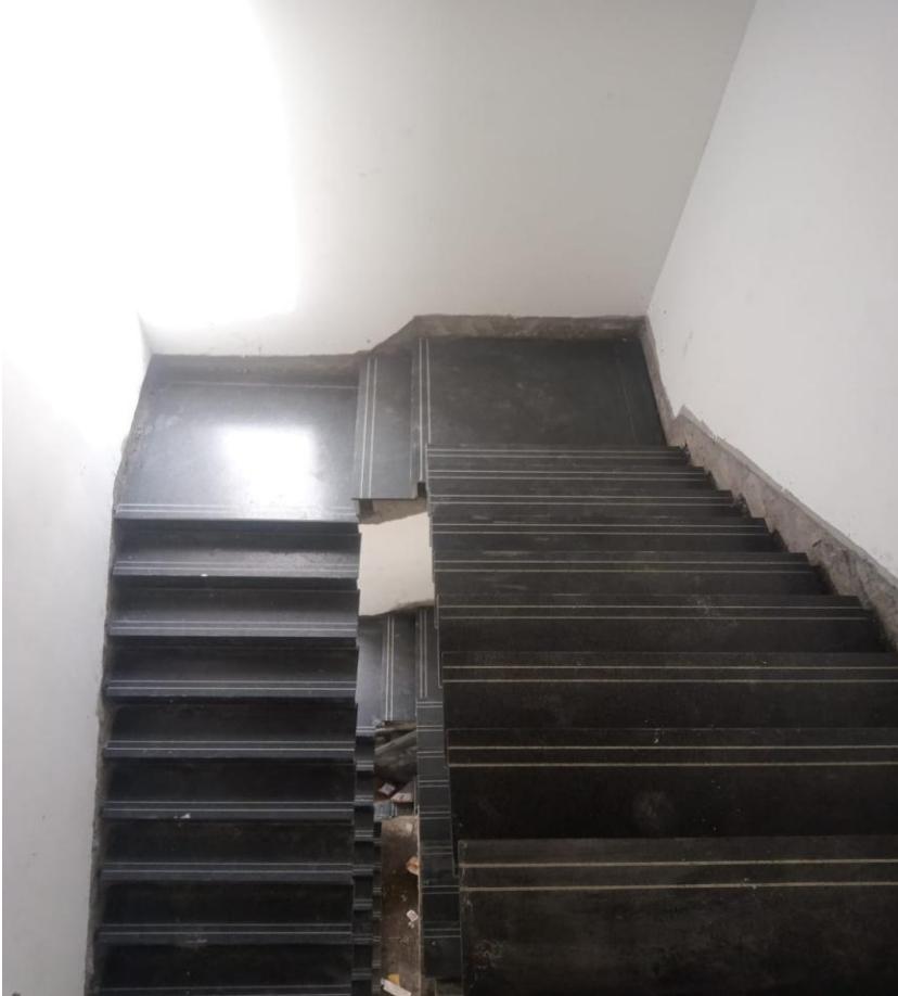
Villa 11 Staircase Granite Laying On Progress
