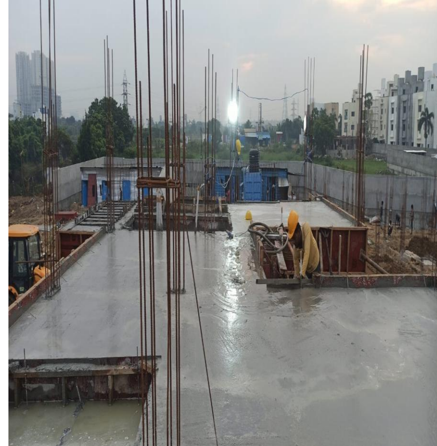
Villa 73 GF Roof Slab Concrete Completed
