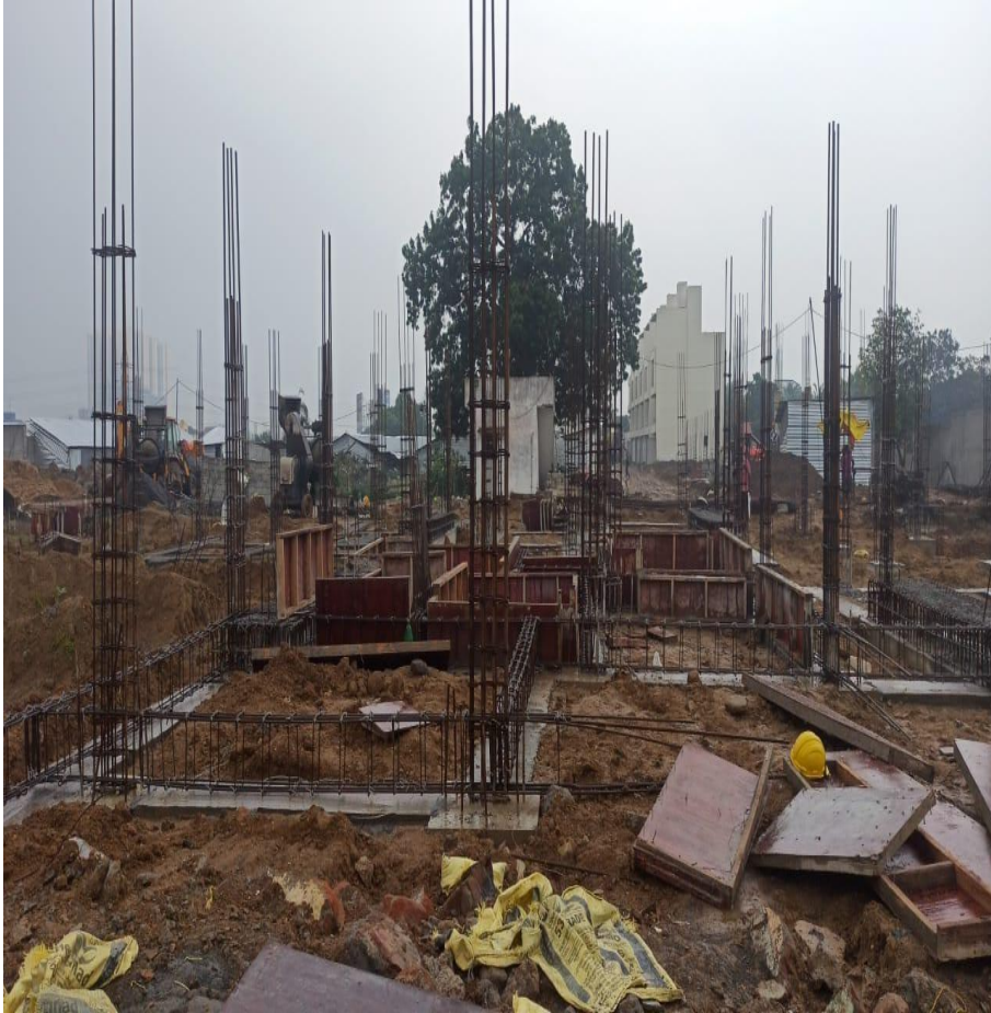
Villa 37 Plinth Beam Reinforcement Work On Progress
