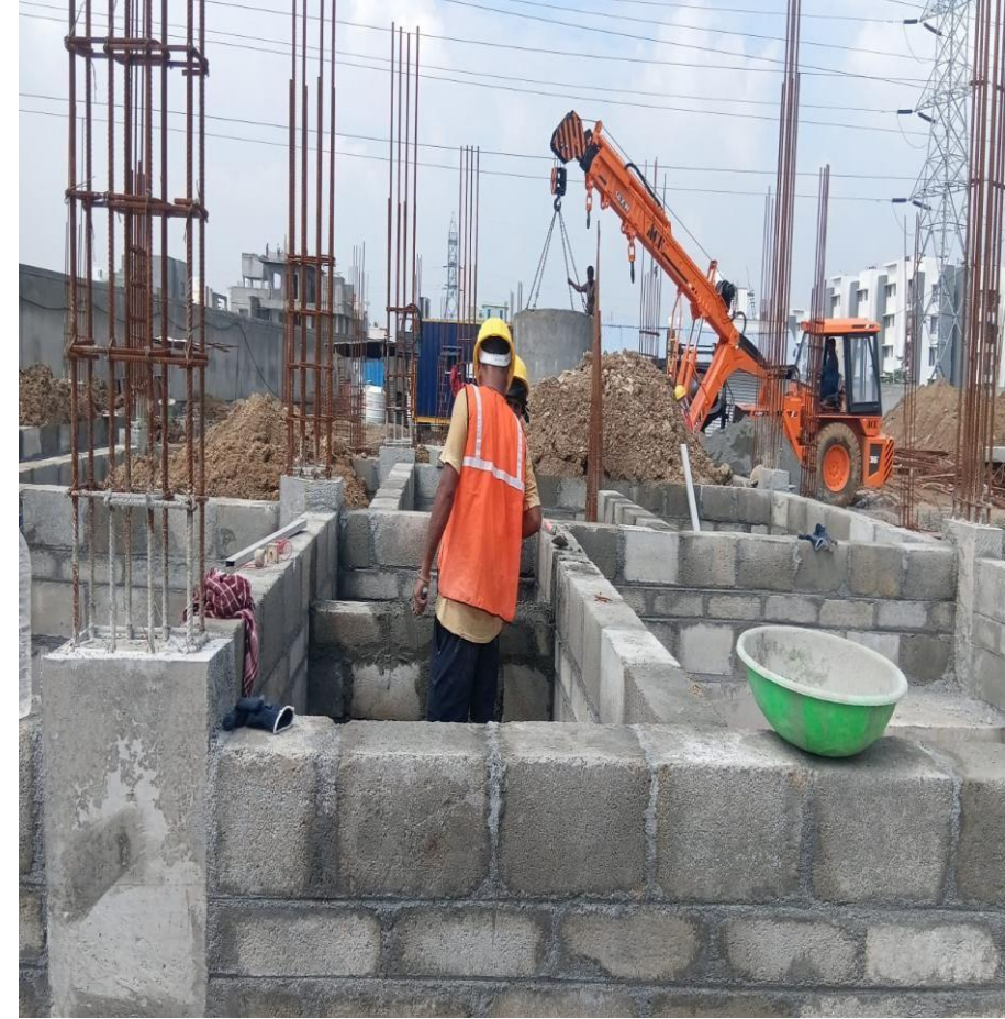
Villa 44 Basement Block Work On Progress
