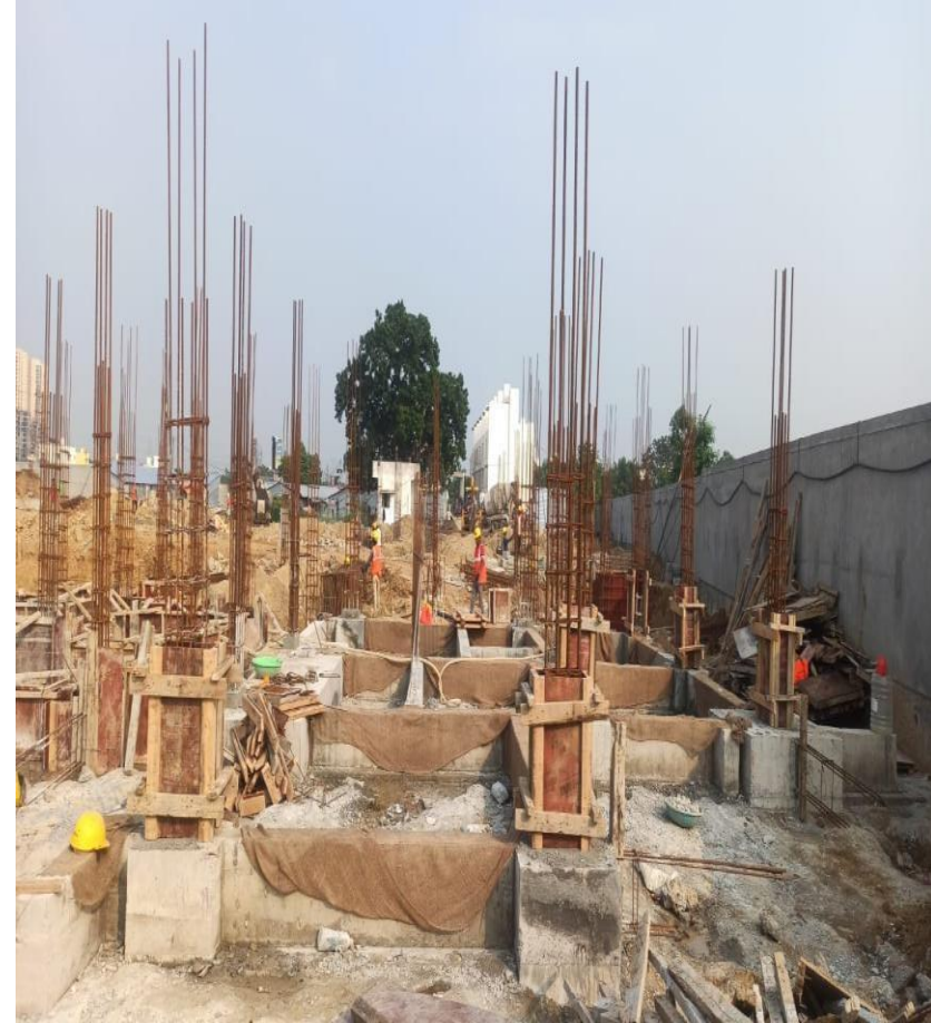
Villa 45 Pedestal Column Shuttering Work Progress
