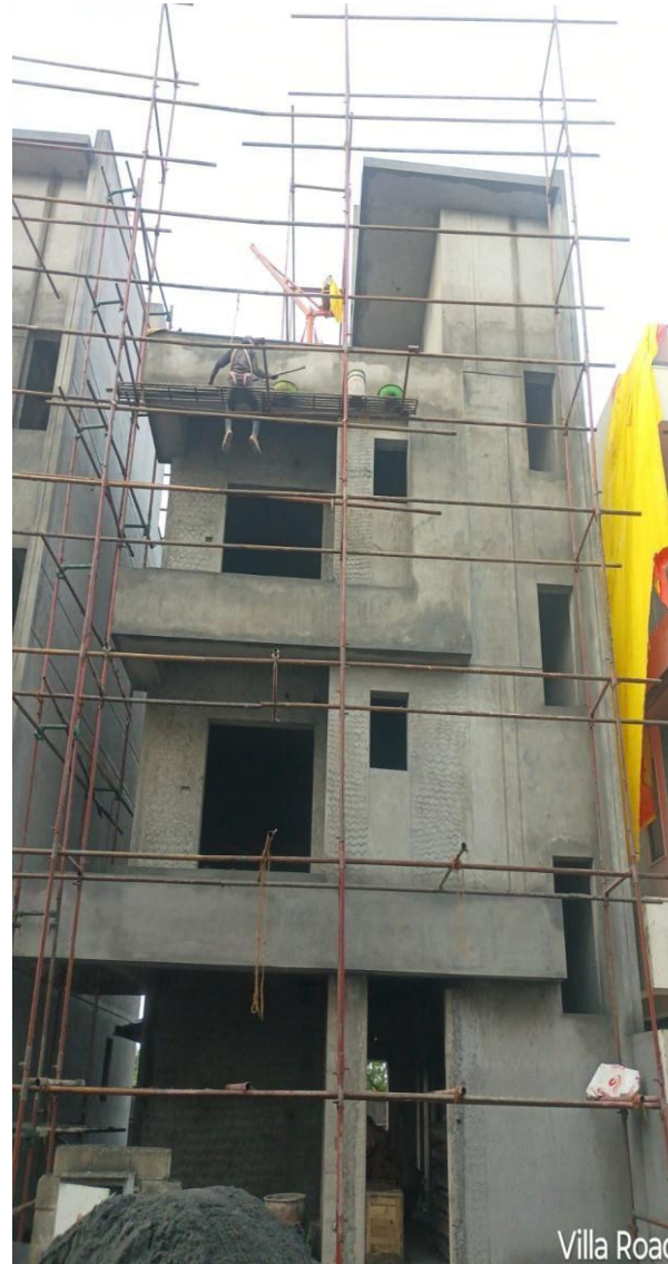
Villa No 15 – South Side Plastering Work Completed
