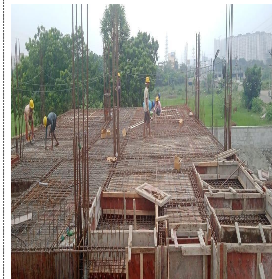
Clubhouse GF Roof Slab Reinforcement Work On Progress
