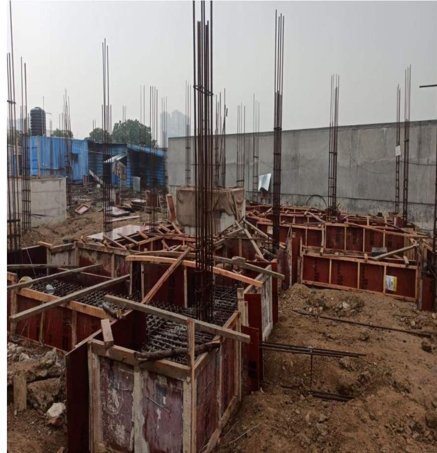
Villa 108 Pile Cap Shuttering Work On Progress
