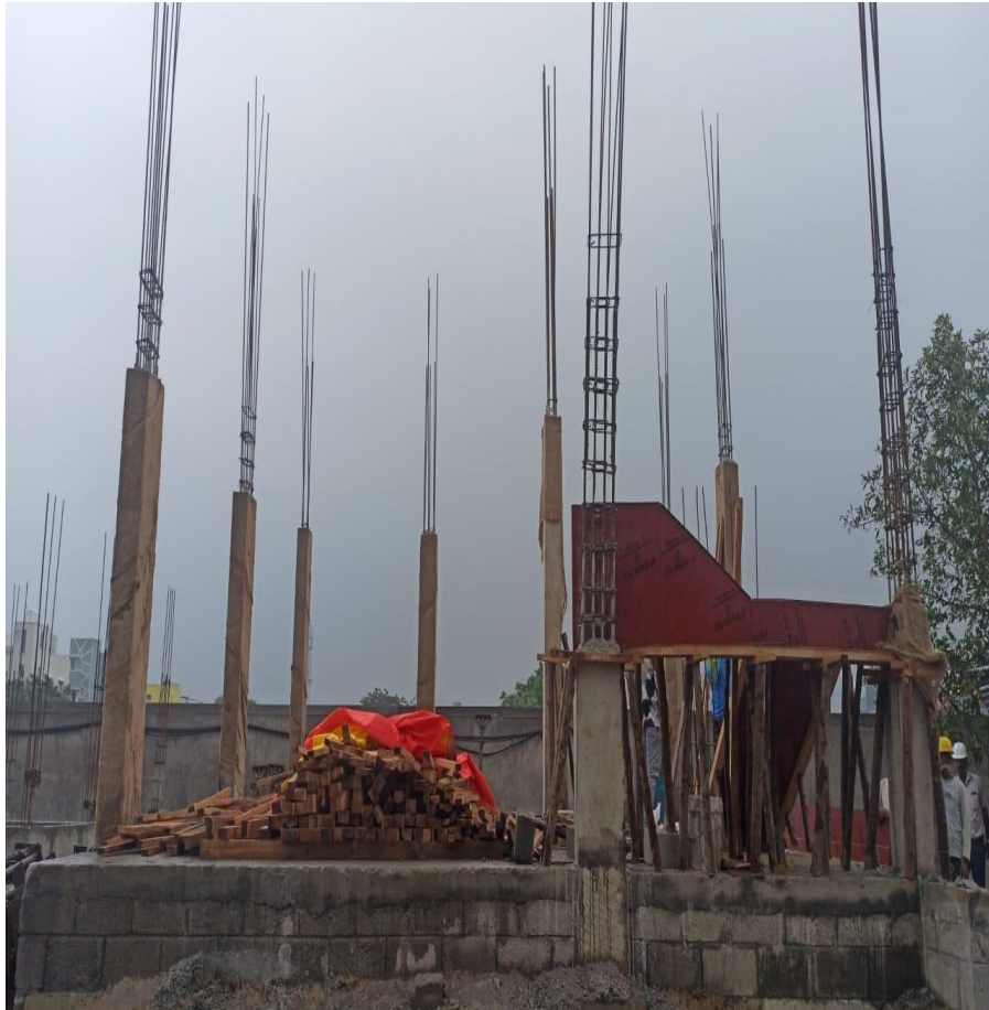
Villa 29 GF Staircase Shuttering Work On Progress
