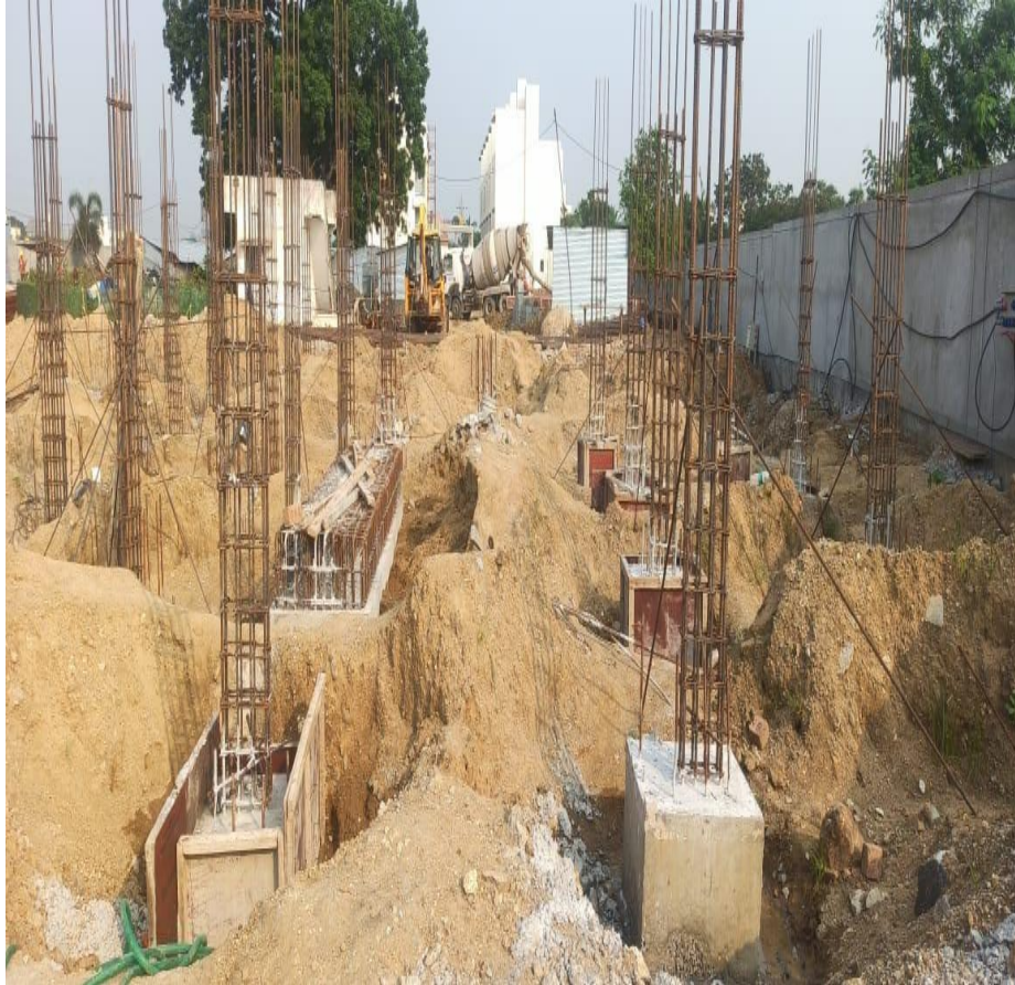
Villa 38 Pile Cap Concrete Completed
