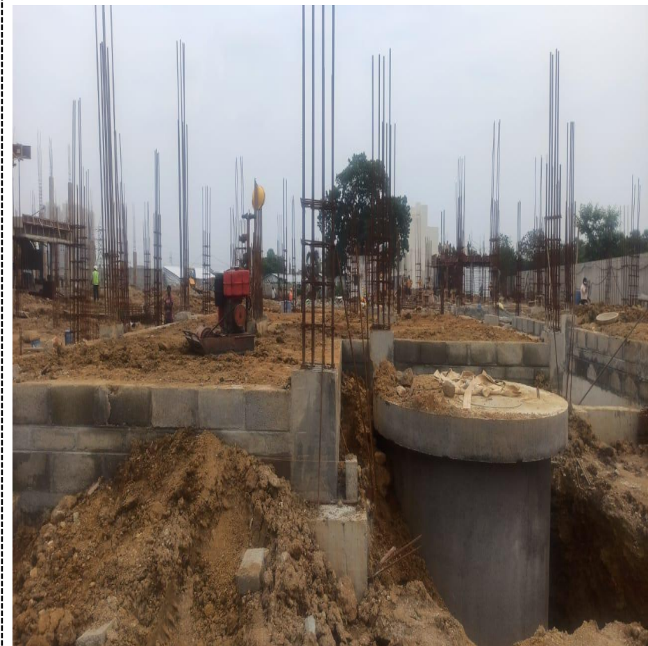
Villa 44 Basement Soil Compacting Work On Progress
