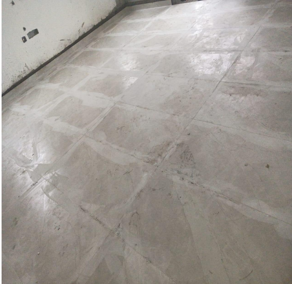
Villa 17 Flooring Tiles Laying On Progress
