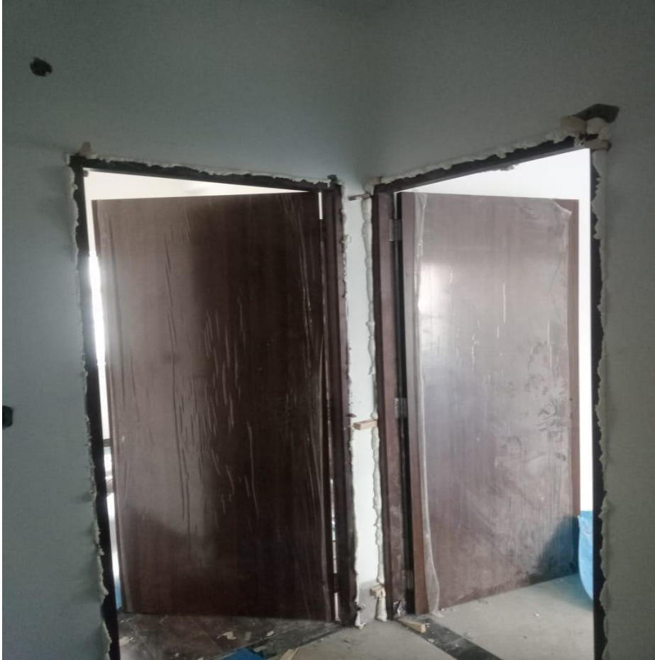
Villa 4 Door Fixing Work On Progress
