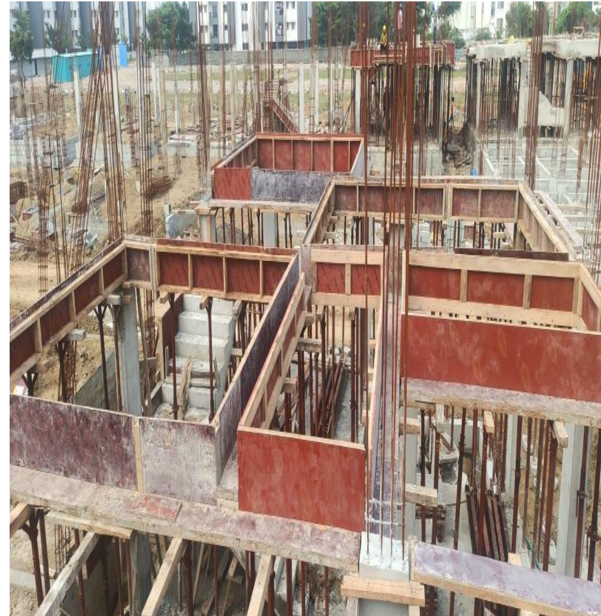
Villa 56 GF Roof Slab Shuttering Work Progress
