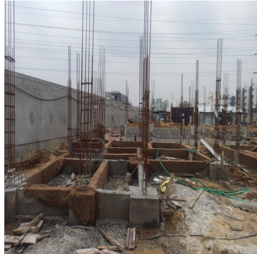
Villa 39 Plinth Beam Concrete Completed
