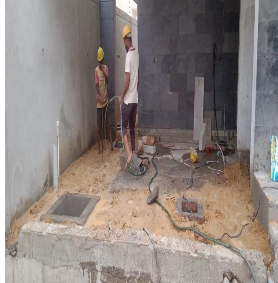
Villa 6&7 Carparking Soil & Consolidation Work On Progress
