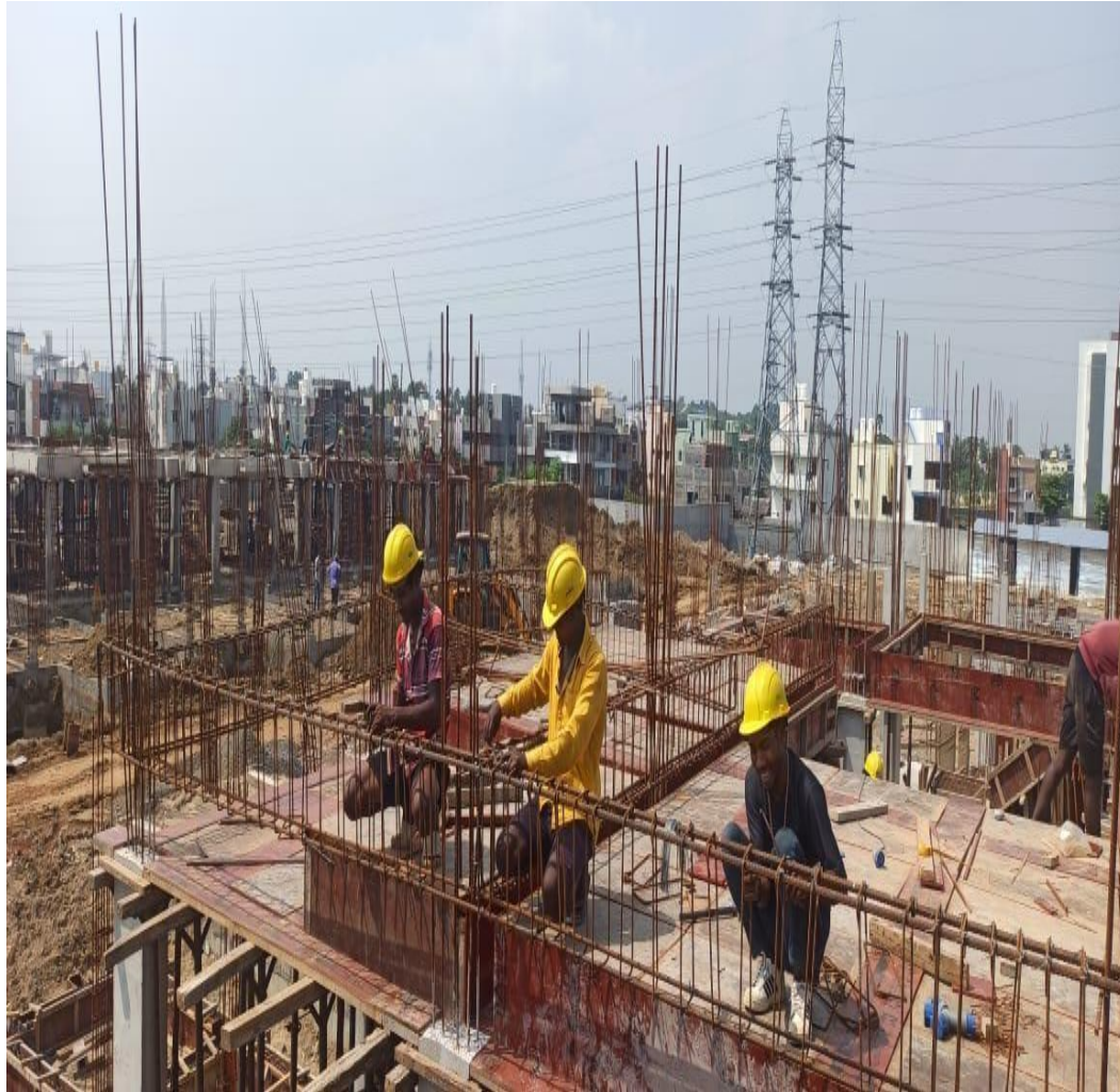
Phase 2 – villa no 73&74 GF Roof Slab Reinforcement Work On Progress
