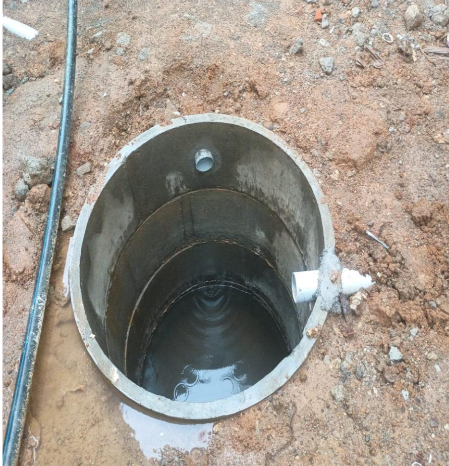
Villa 4&5&6 Rain Water Soak Pit Fixing Completed
