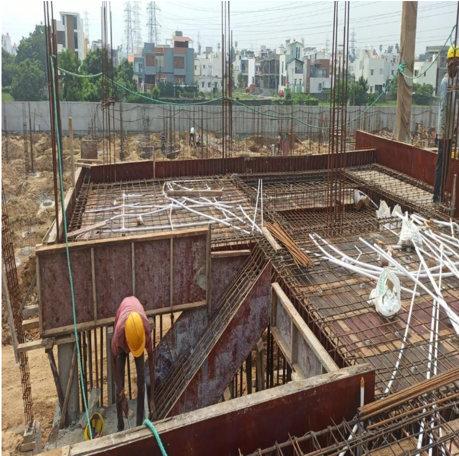
Villa 52GF Roof Slab Electrical Conduit Laying Work Progress
