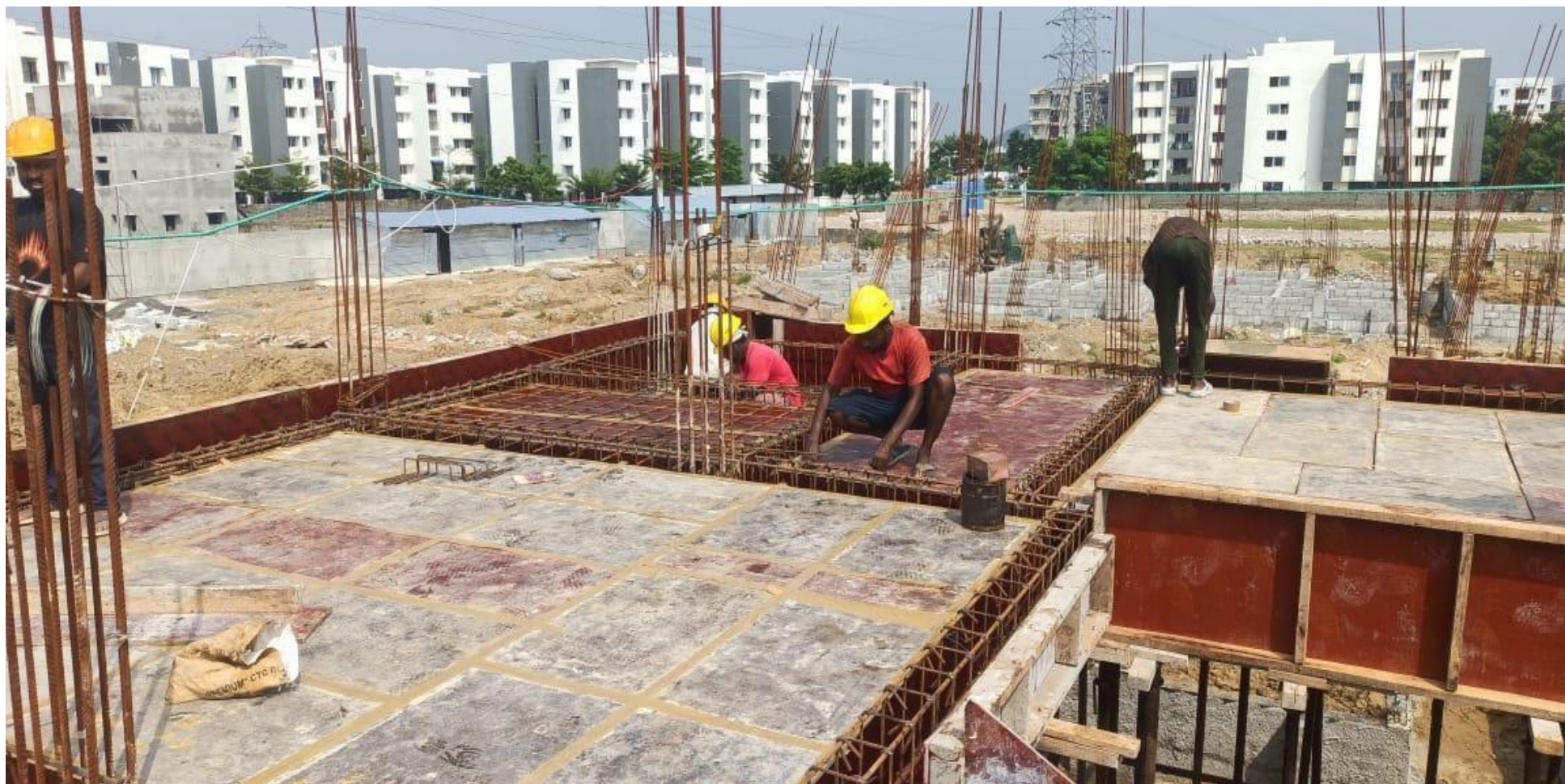
Phase 2 – villa no 47 GF Roof Slab Reinforcement Work On Progress
