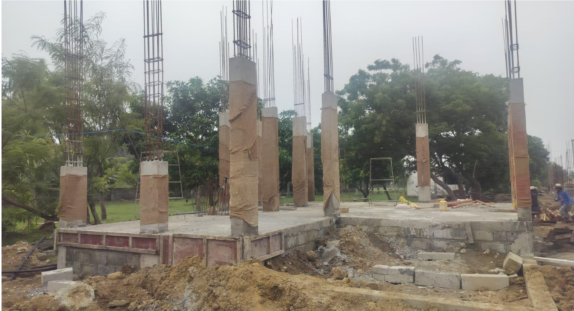
Villa No 4 GF Column Concrete Concrete Completed
