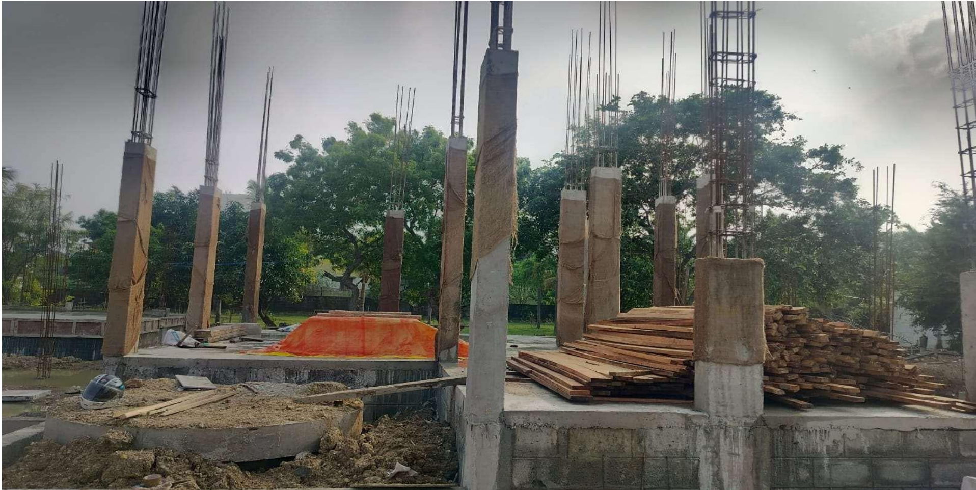
Villa No 6 GF Column Concrete Completed
