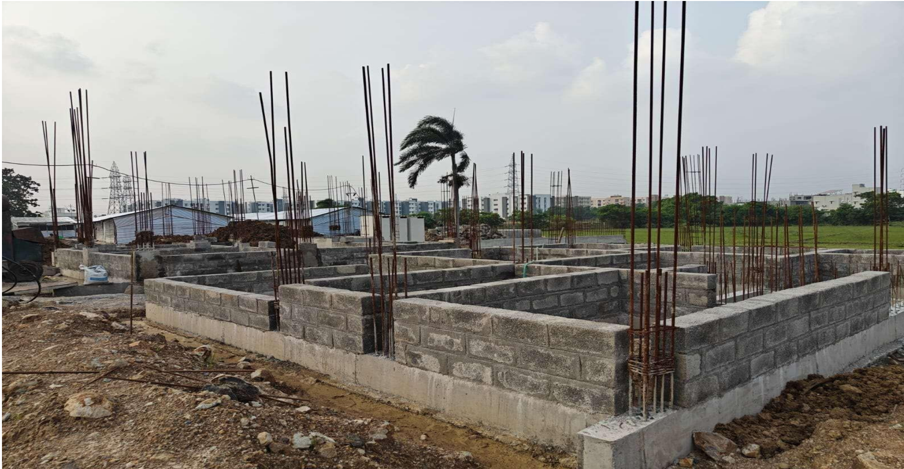
Villa no 12 and 13 Plinth beam above block work completed
