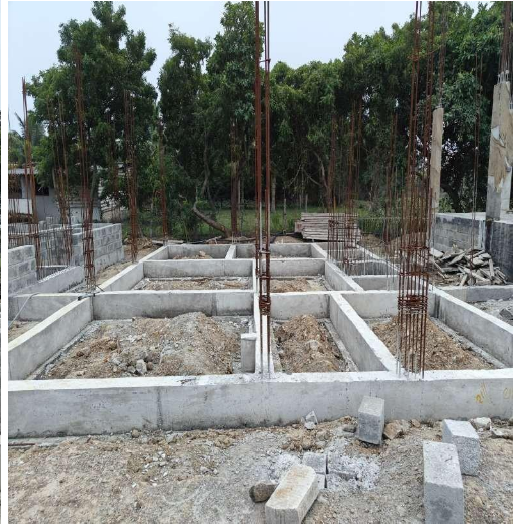
Villa No 9 & 10 Plinth Beam Concrete Completed
