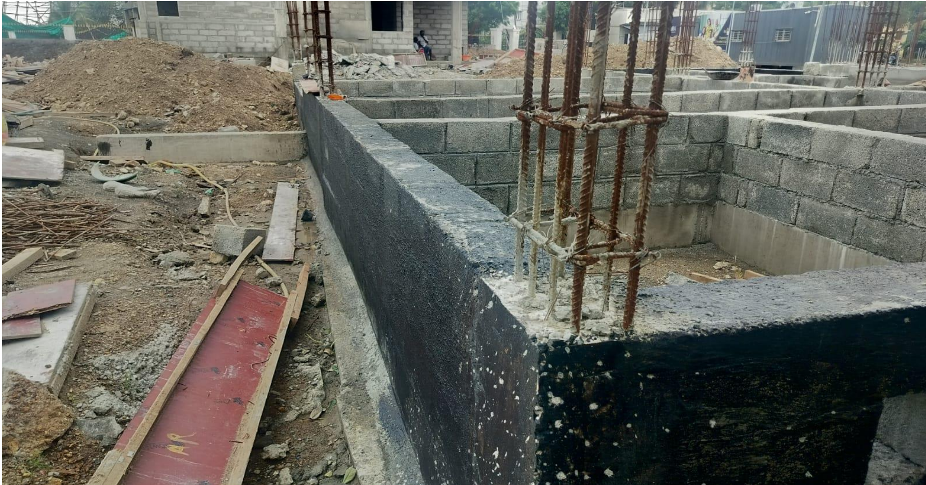
Villa no 17- DPC Waterproofing work in Progress
