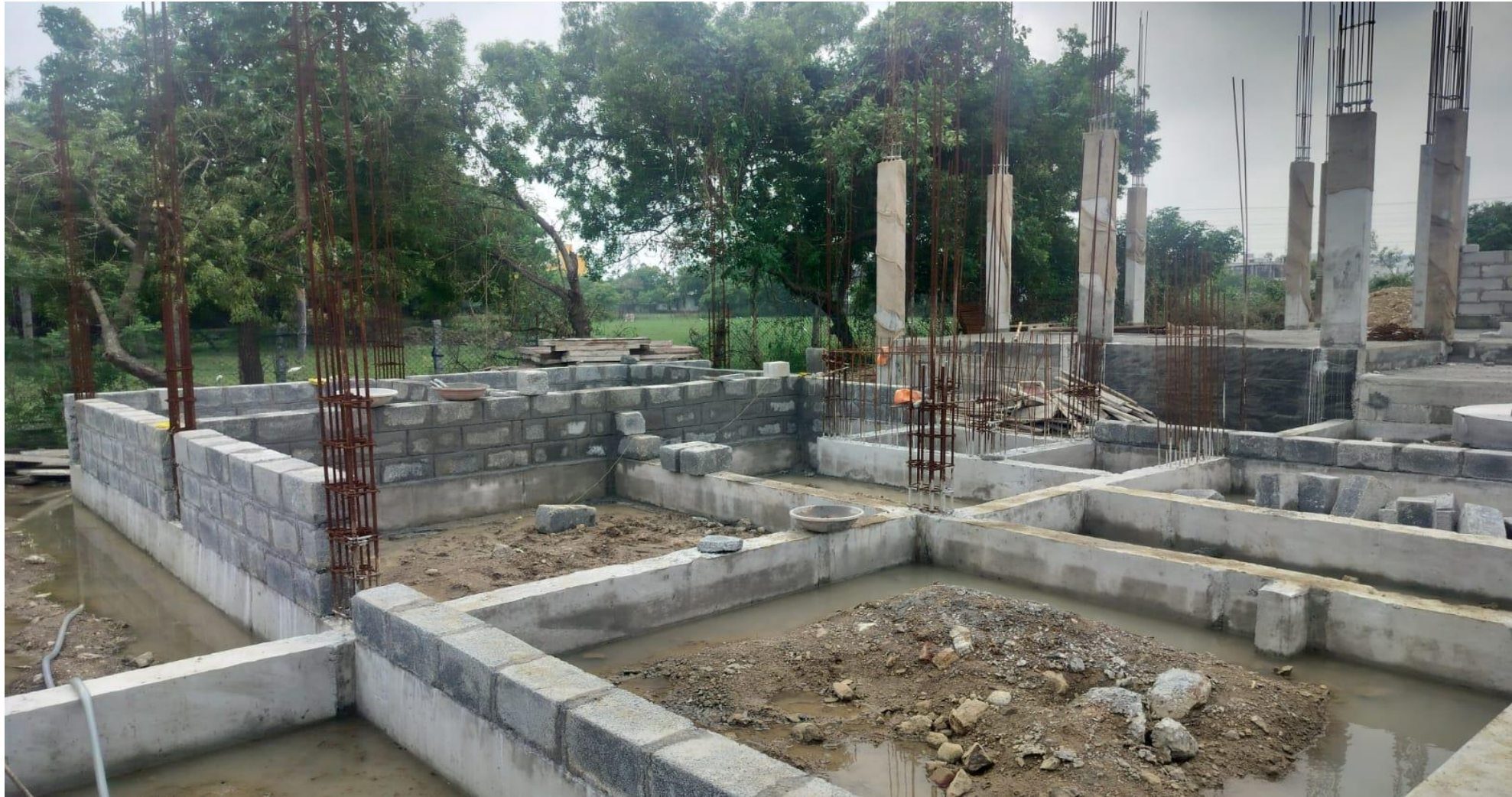
Villa No 10 Above Plinth beam block work in Progress
