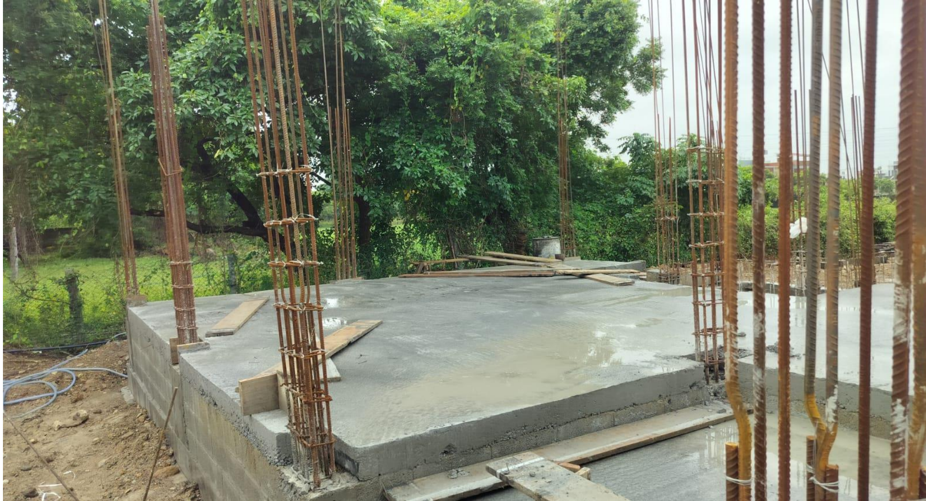
Villa No 11 GF PCC Concrete Completed
