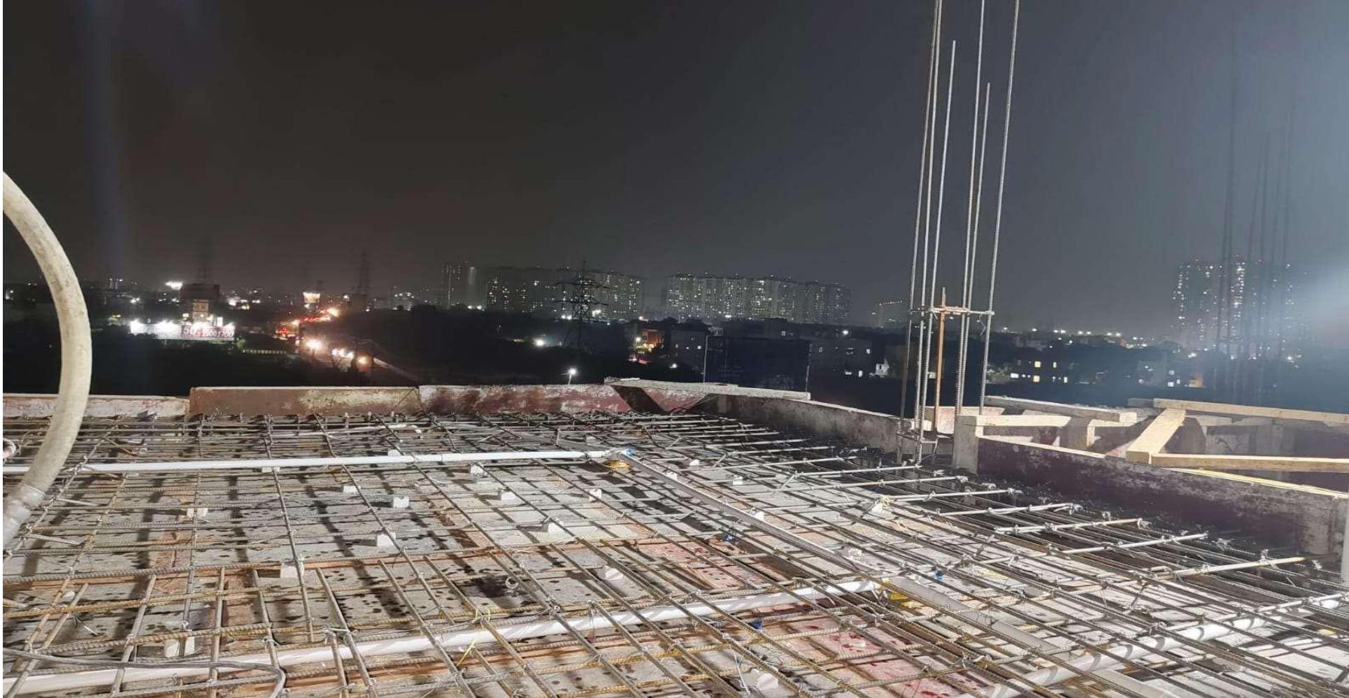
Villa No 20 Head Room Slab Ready For Concrete
