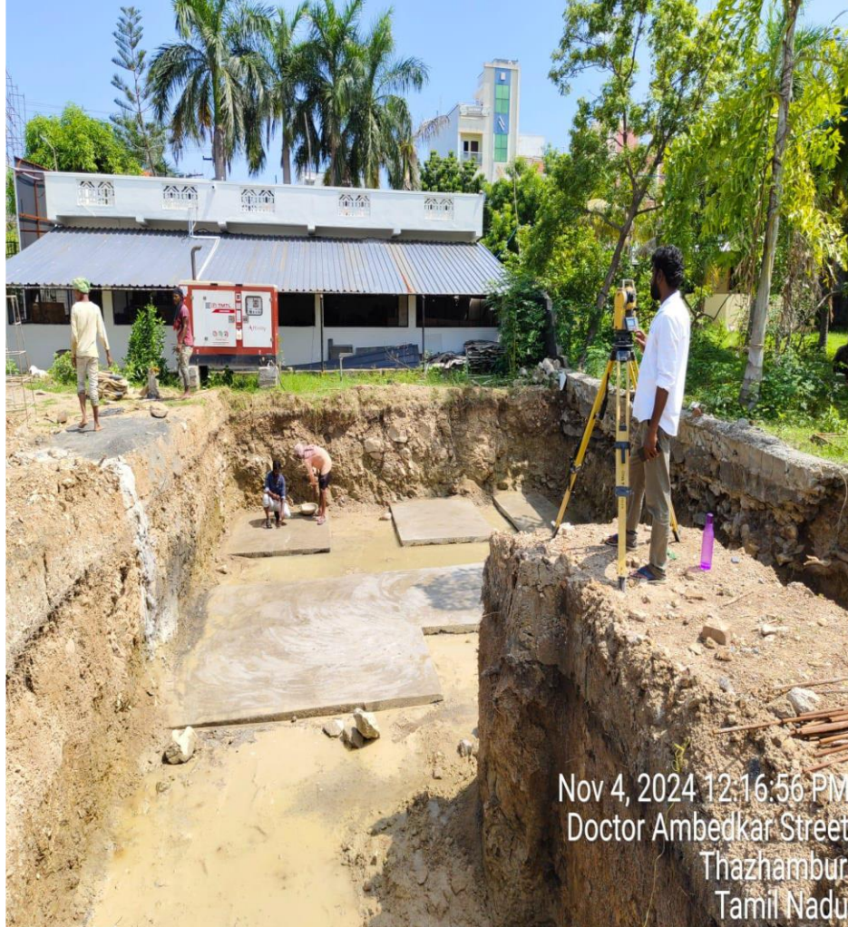
Villa no 3 Footing PCC and RCC Completed
