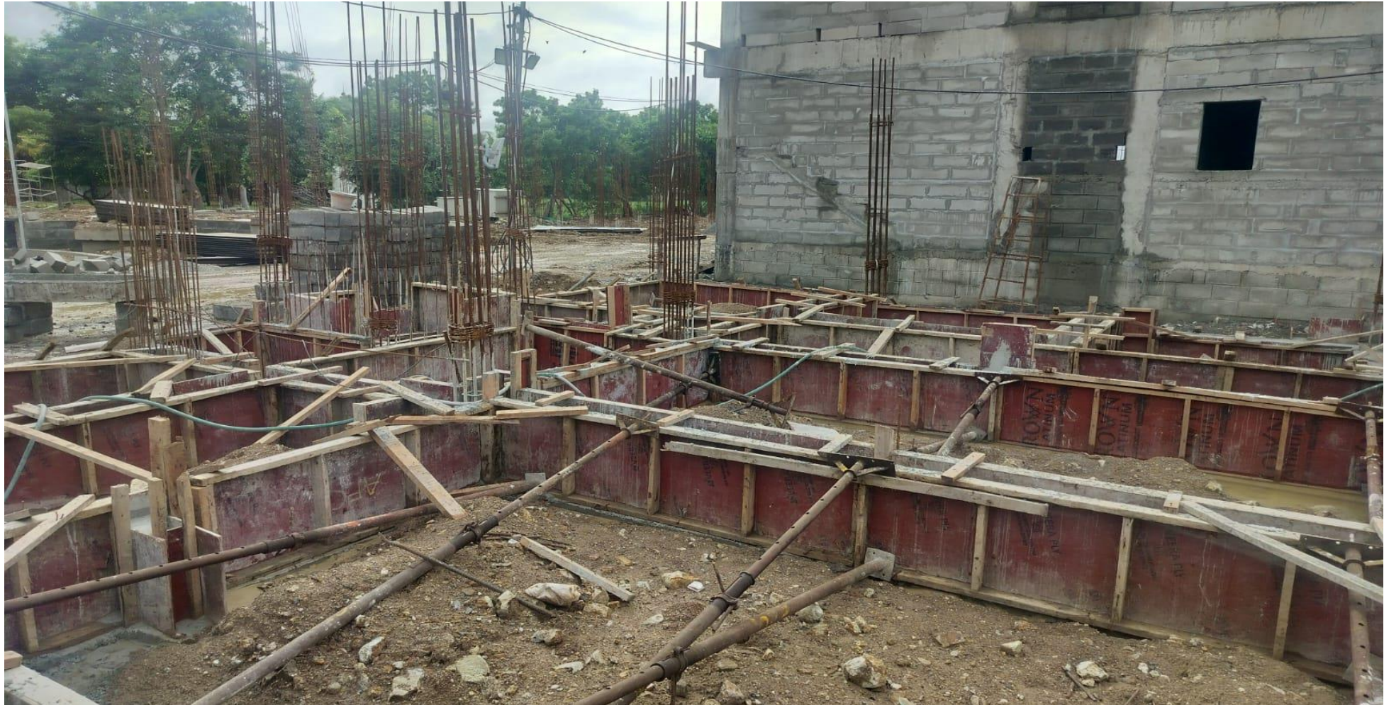
Villa No 17 Plinth Beam Concrete Completed
