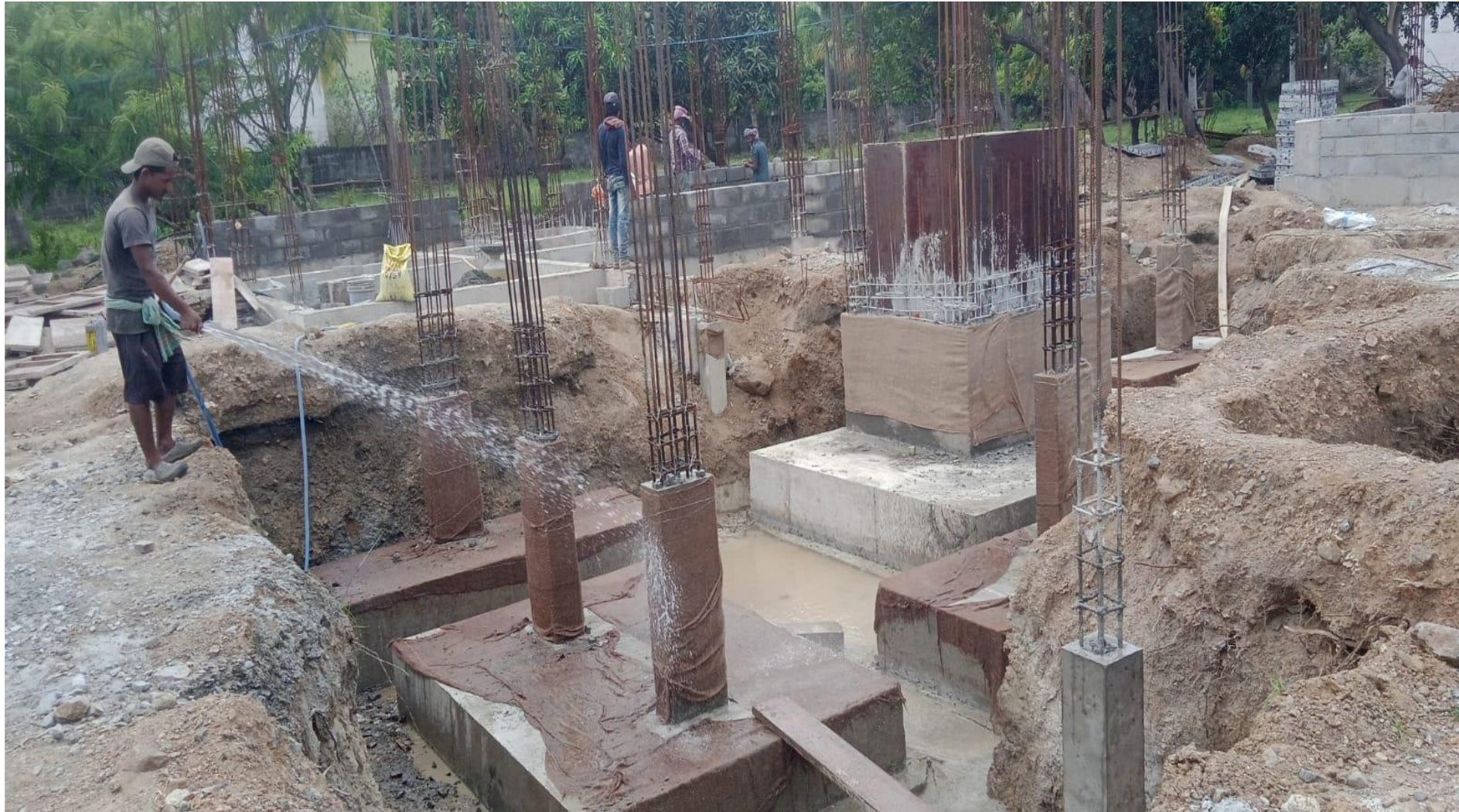
Villa No 5 Pedestal Column Concrete Completed
