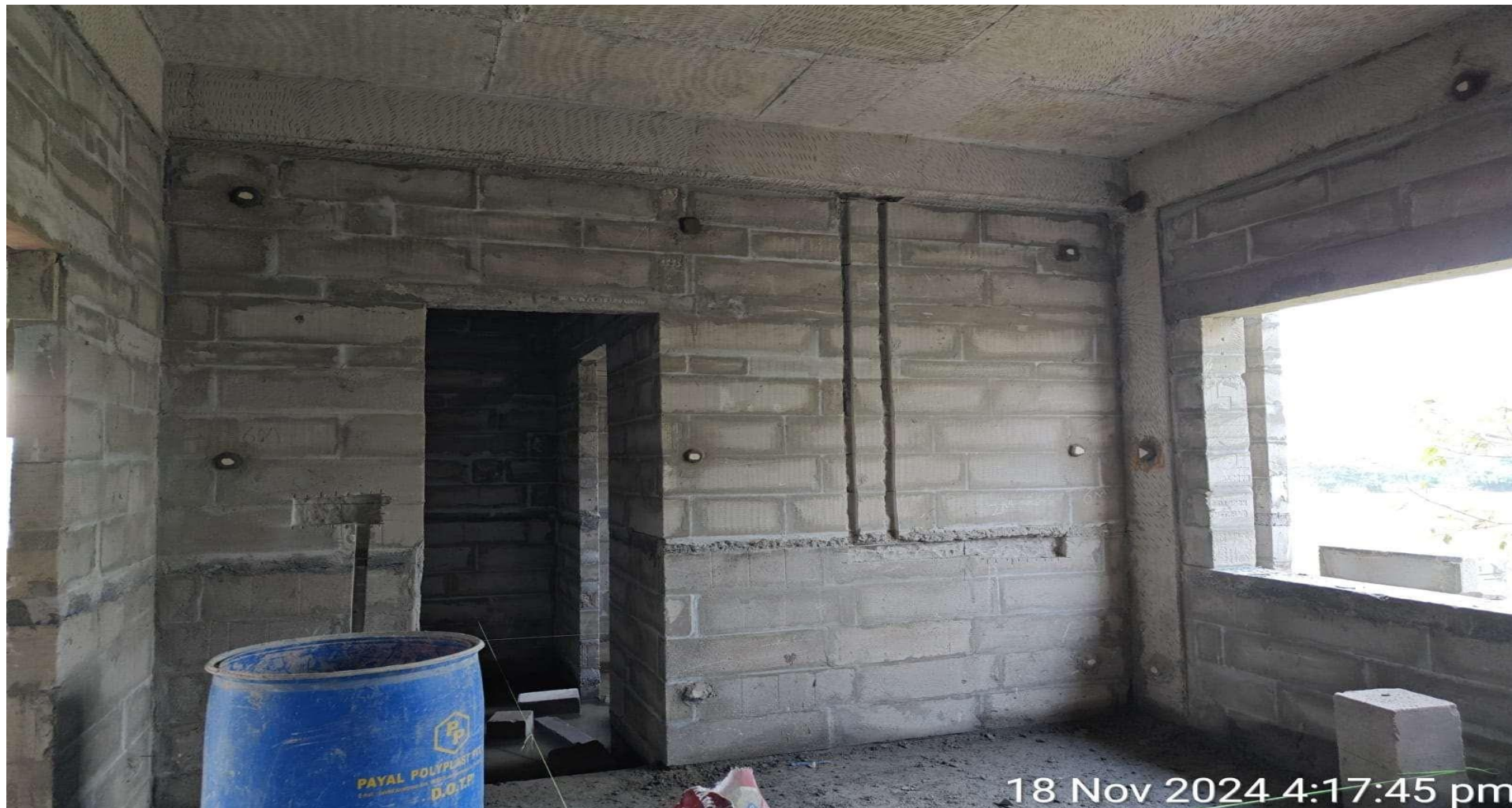
Villa No 16 FF Block work Completed
