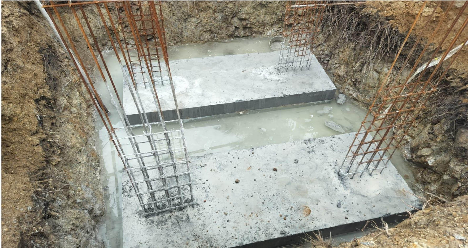
Entrance Arch Footing Concrete Completed
