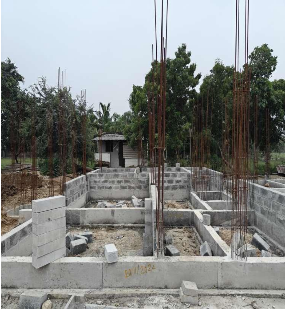
Villa No 9 & 10 Plinth Beam Concrete Completed
