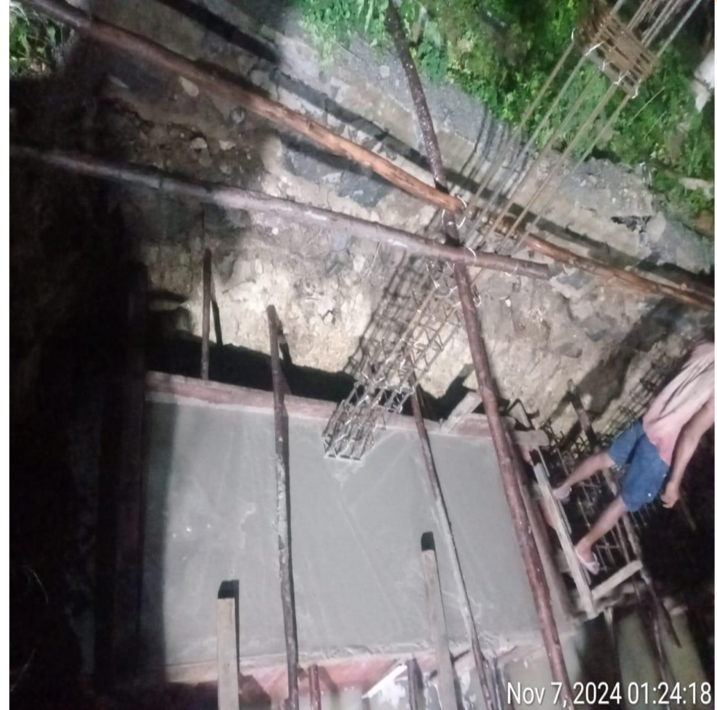
Villa no 3 Footing PCC and RCC Completed
