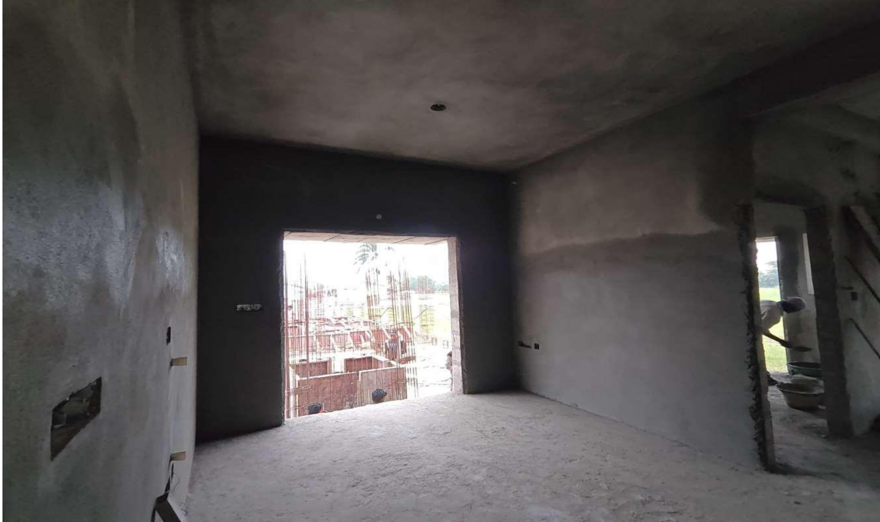
Villa No 16 GF Plastering Work in Progress
