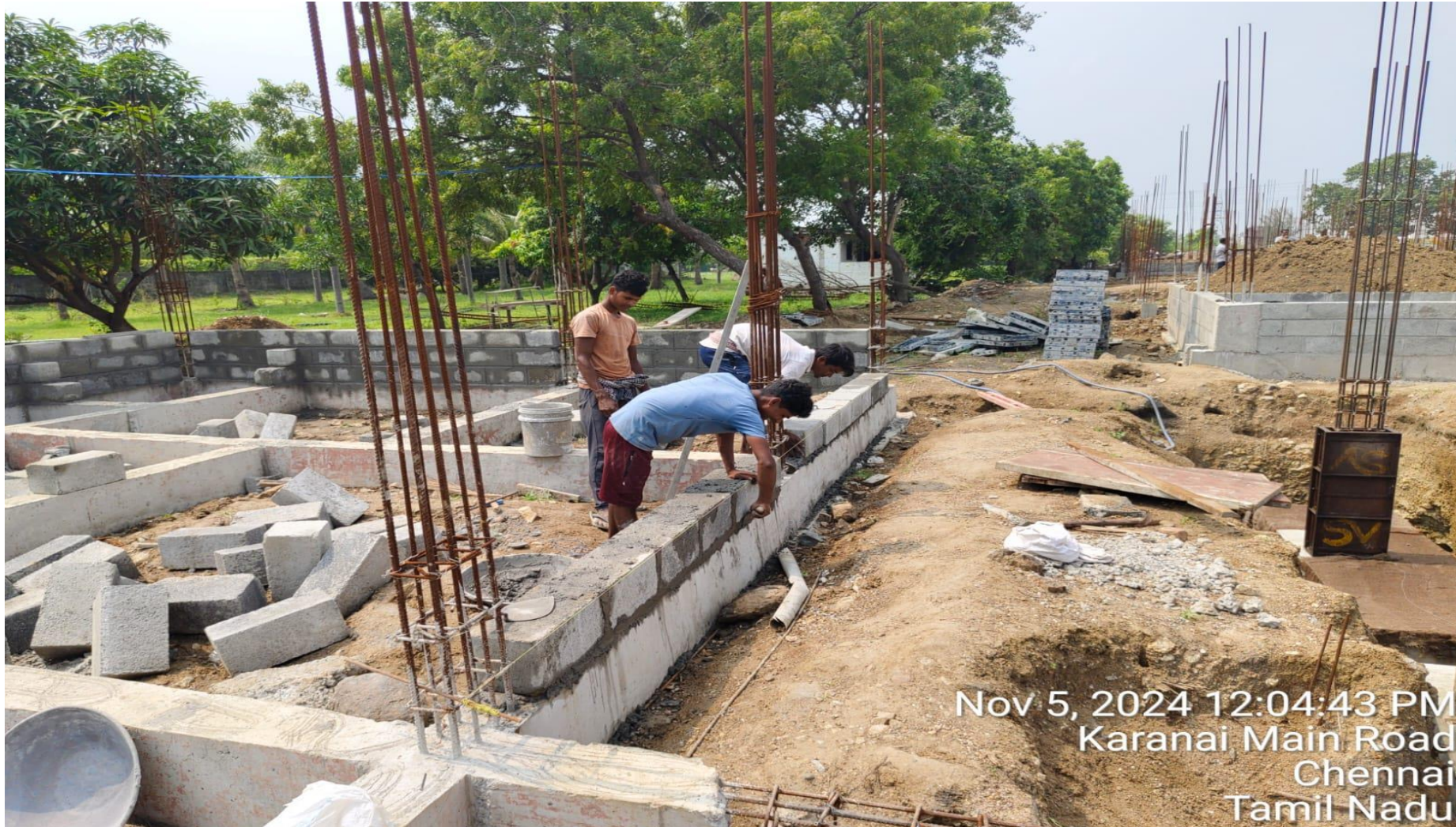
Villa No 4 Above plinth beam level Block Work in Progress
