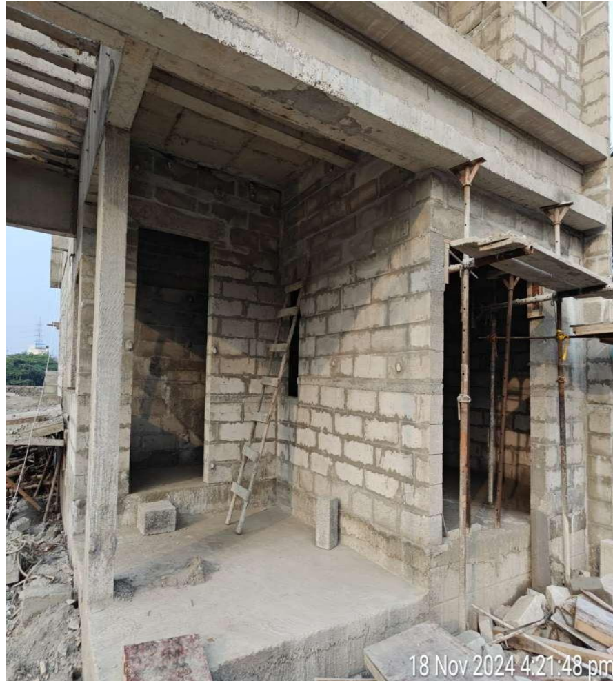
Villa No 20 GF Block Work Completed
