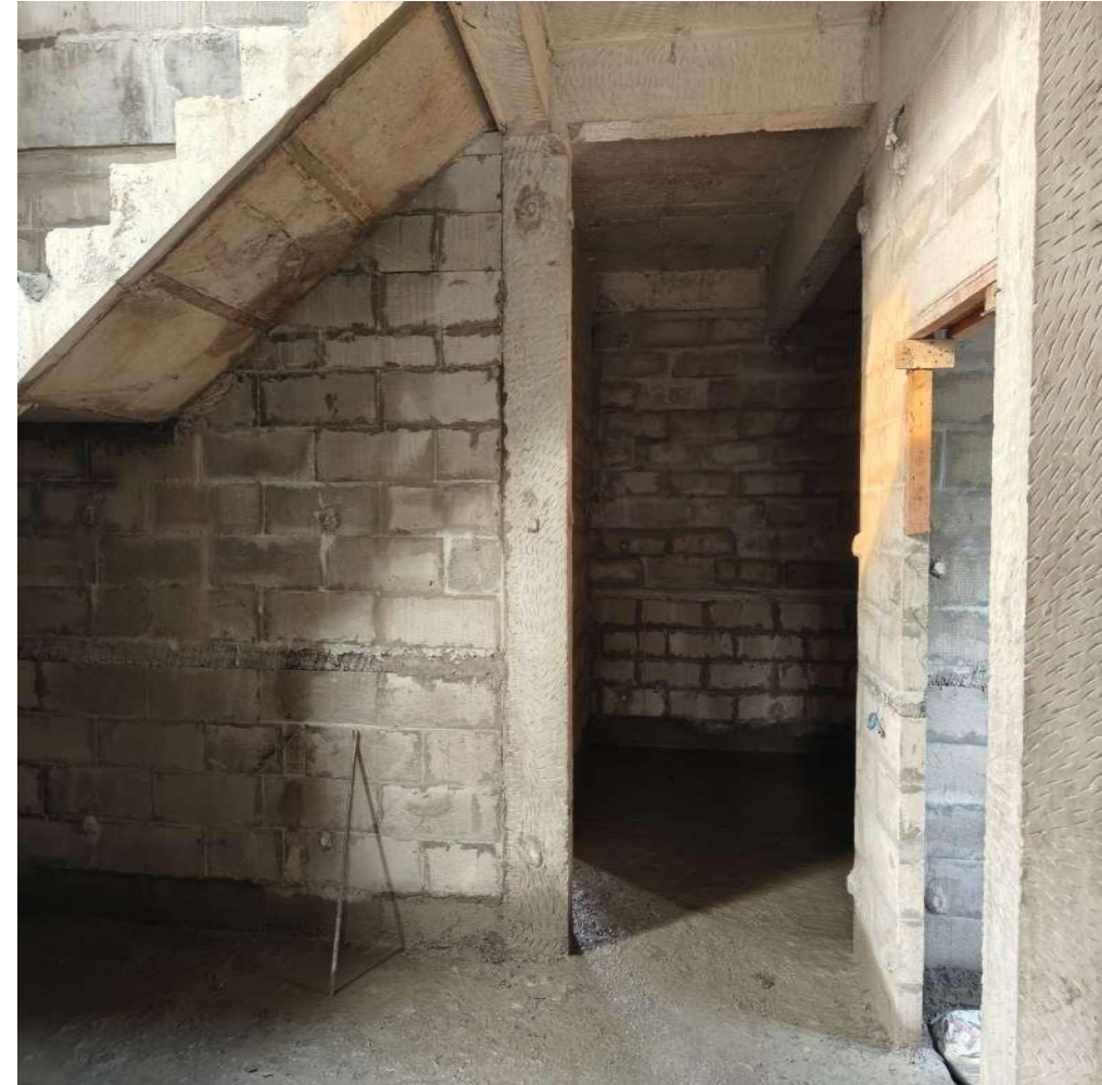
Villa No 20 GF Block Work Completed
