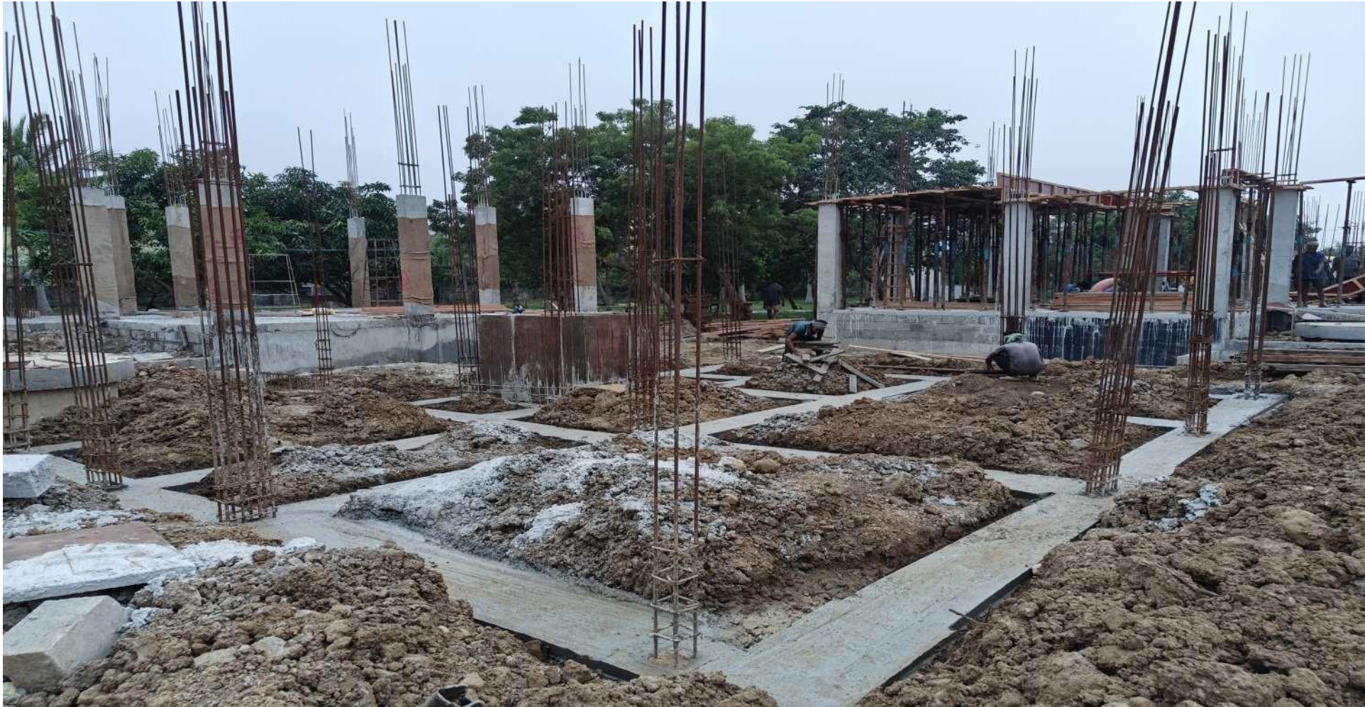
Villa No 5 Plinth PCC Concrete Completed
