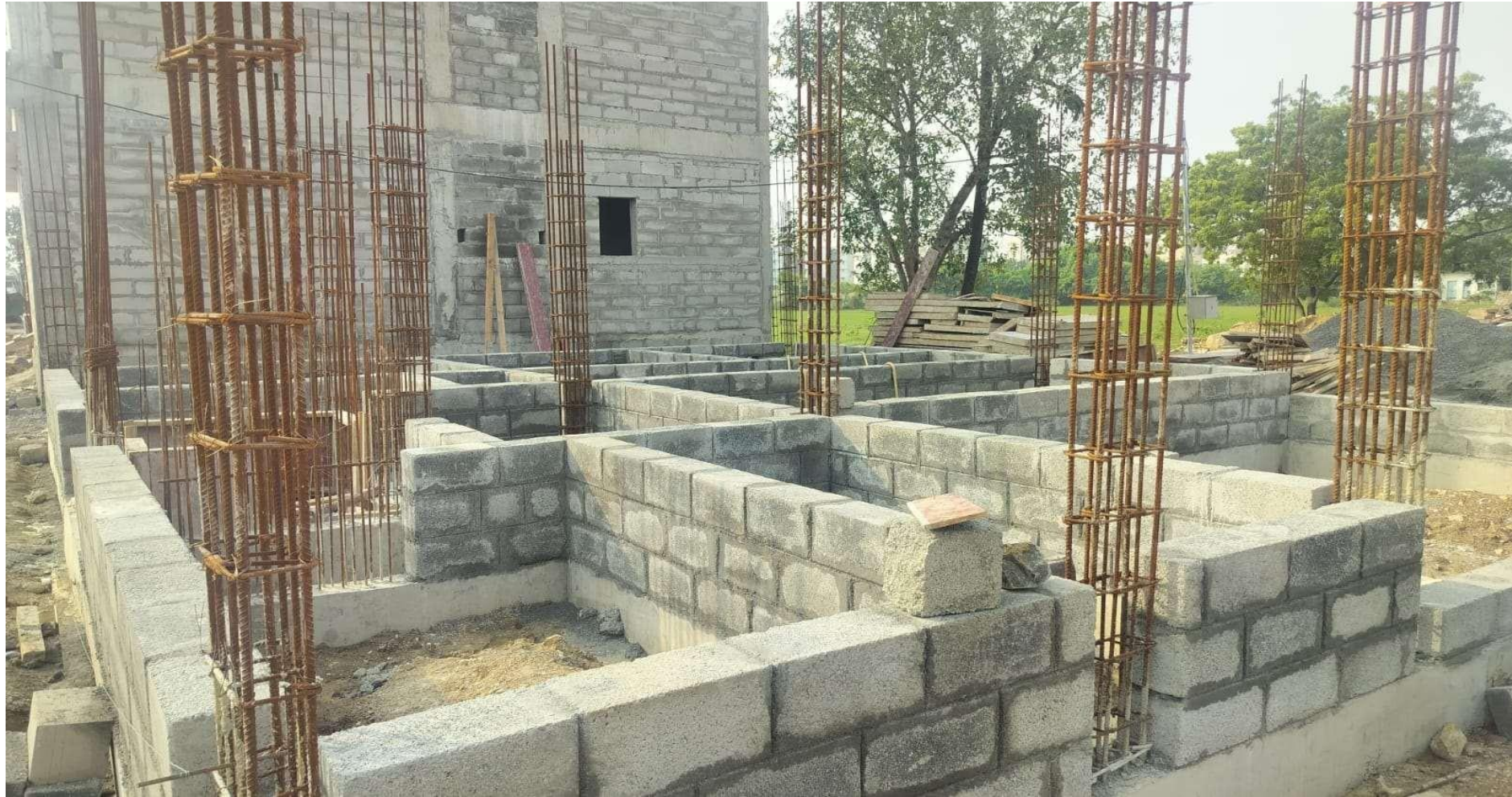
Villa No 17 Above Plinth Beam Block Work in Progress
