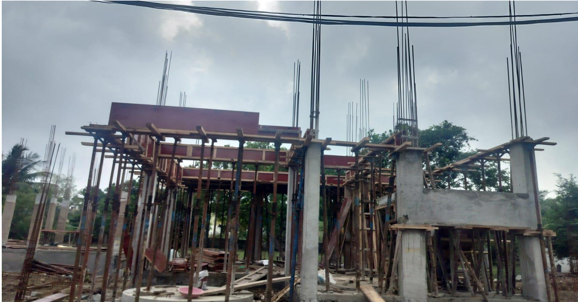
Villa No 6 GF Roof Shuttering work in Progress
