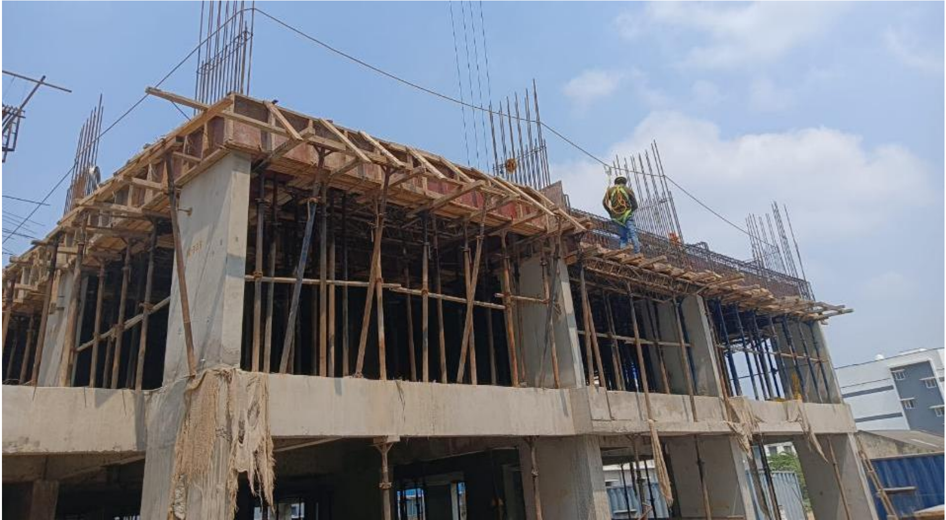
Pour 2 – 1 st Floor roof outer shuttering work in progress.
