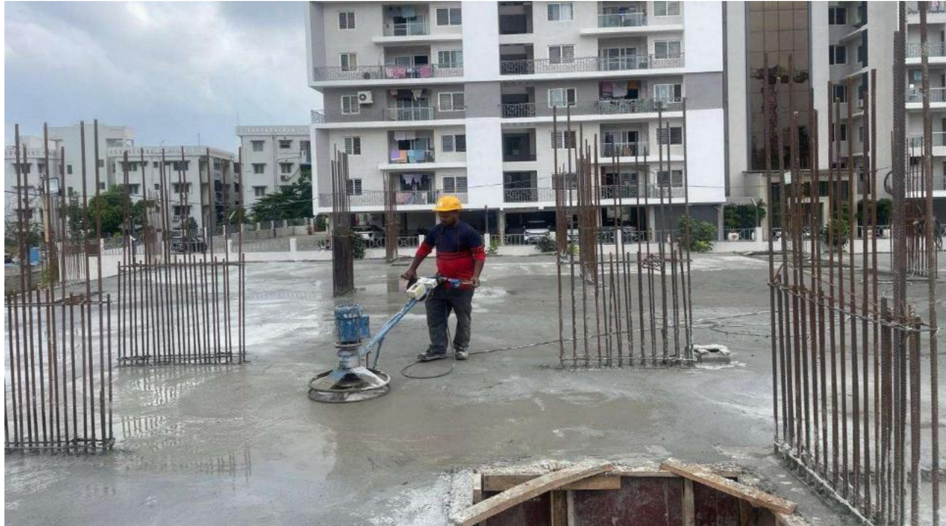
Pour 2 – Stilt floor roof slab finishing work work completed..
