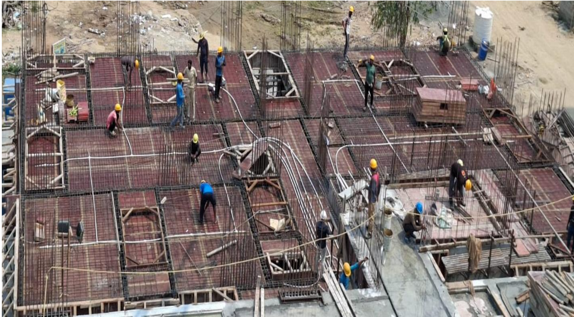
Pour 2 – 1st Floor roof electrical conduit laying work completed.
