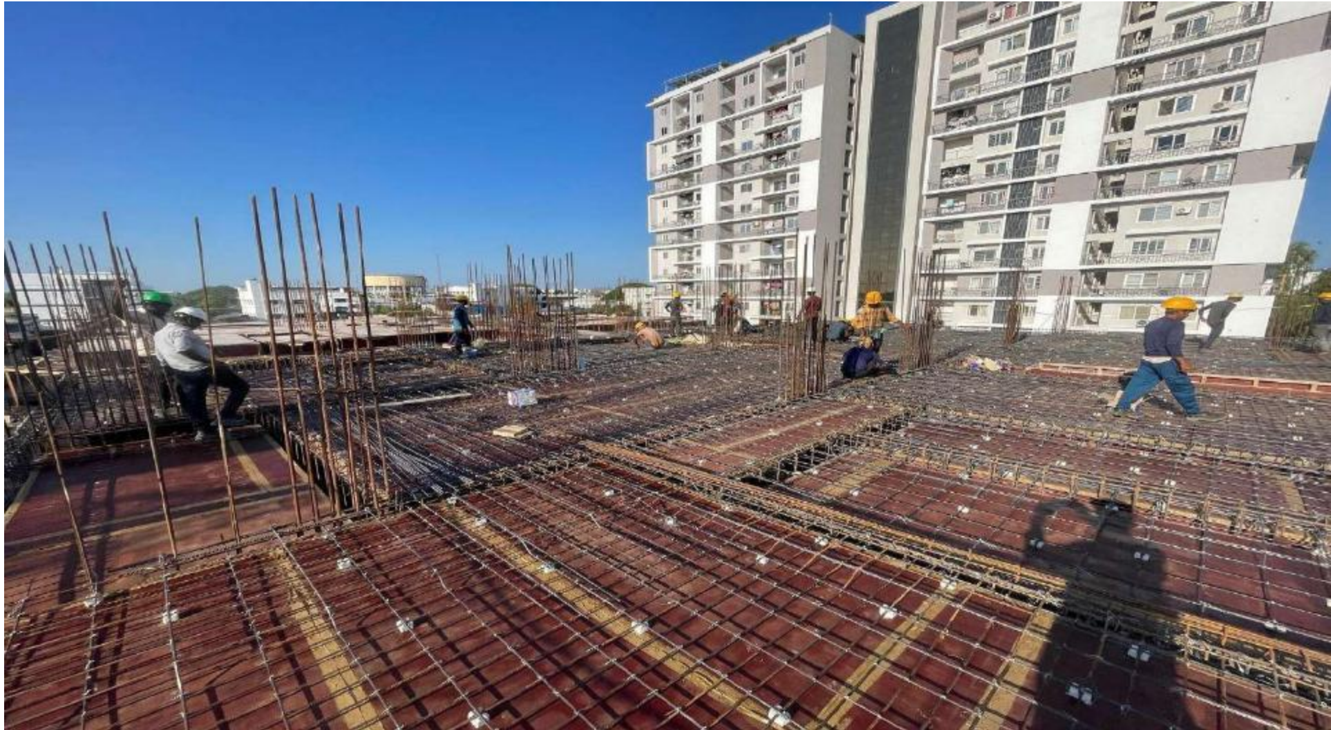
Pour 1 – 2 nd Floor roof slab reinforcement work completed.
