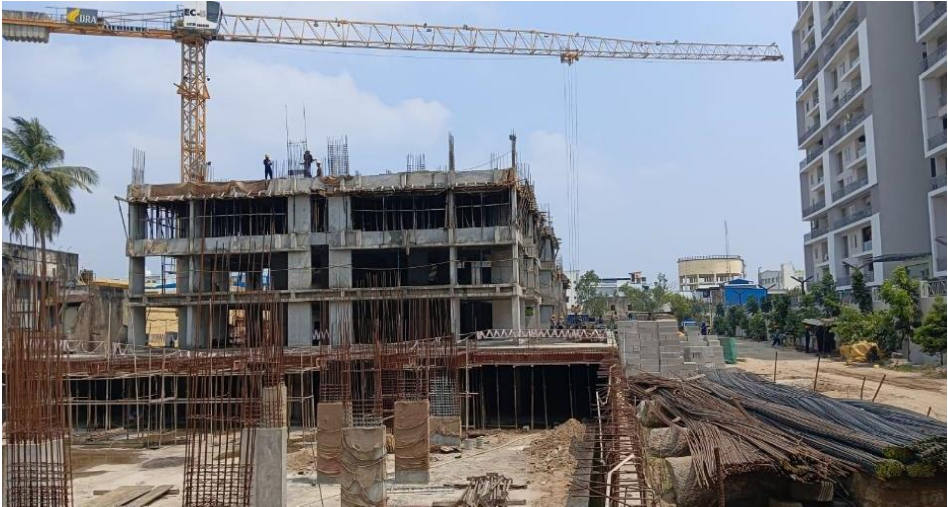
South east corner view.
