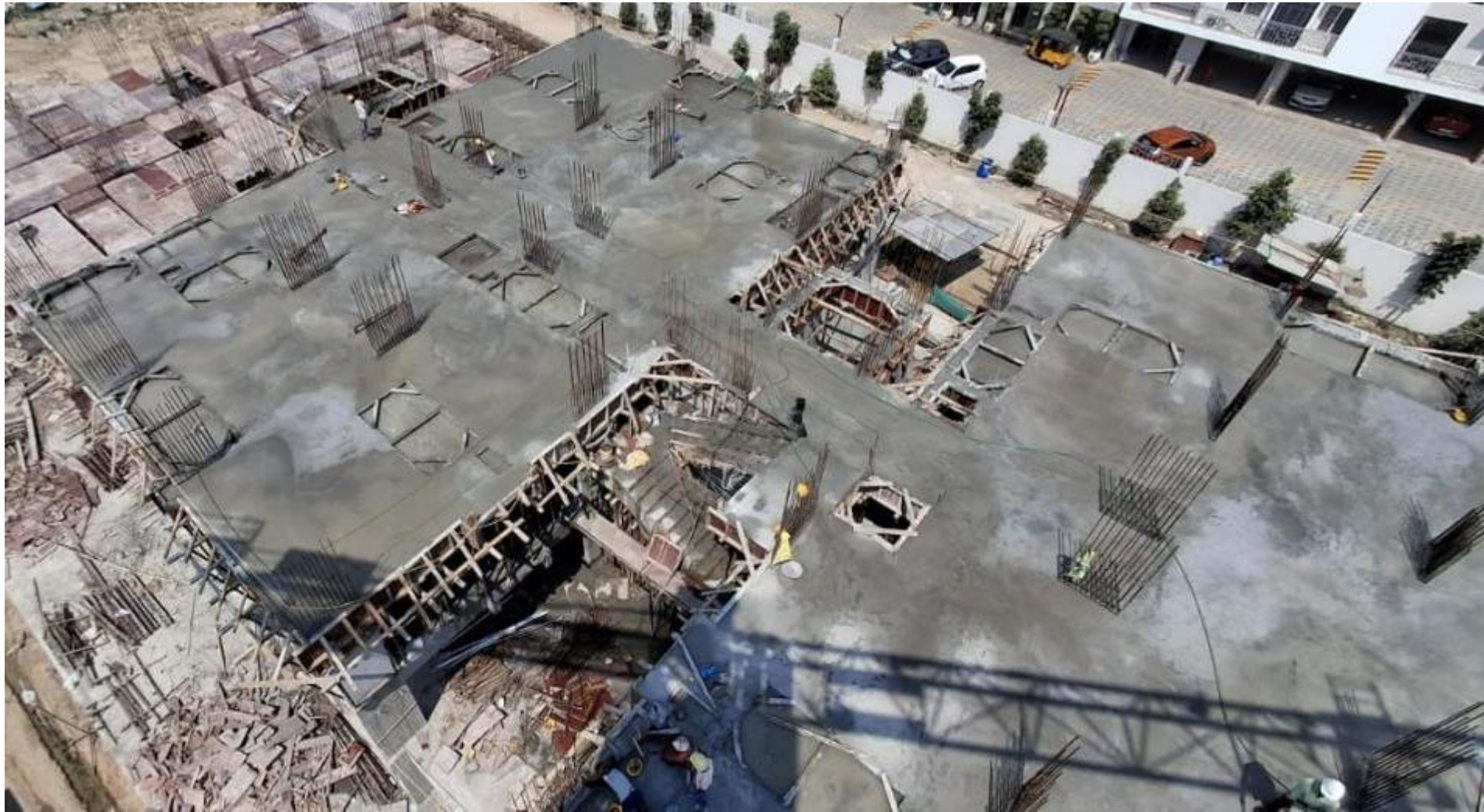
Pour 1 – 2 nd Floor roof concrete work completed.
