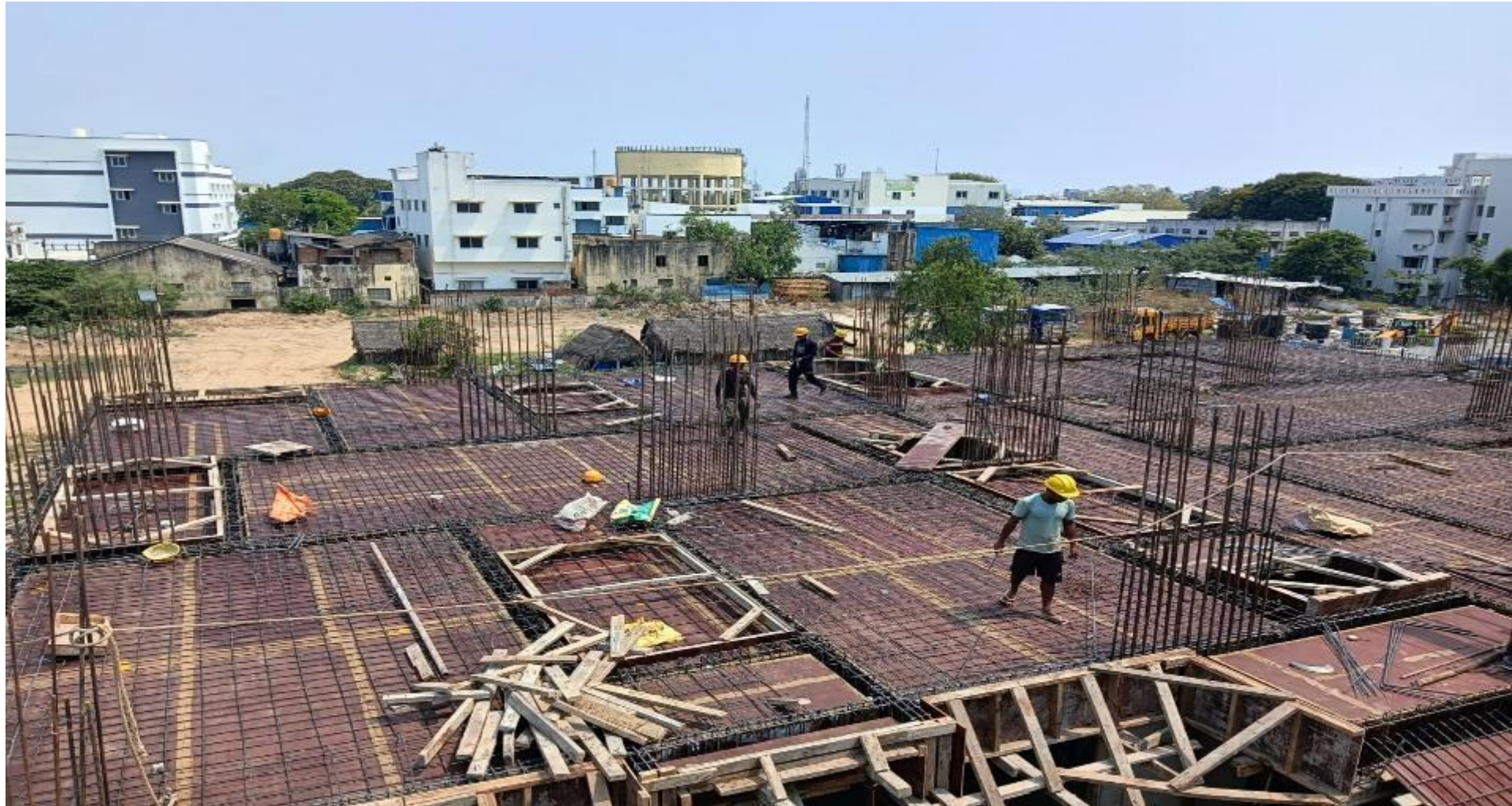
Pour 2 – 1 st Floor roof sunken slab shuttering work completed.
