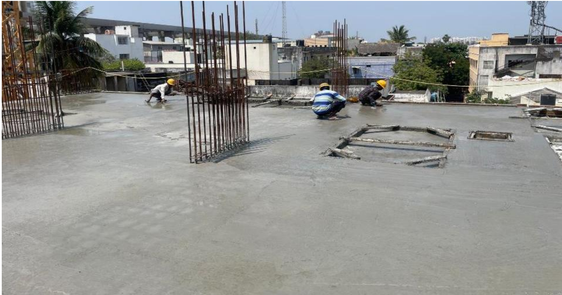
Pour 1 – 2 nd Floor roof slab float finishing work completed.
