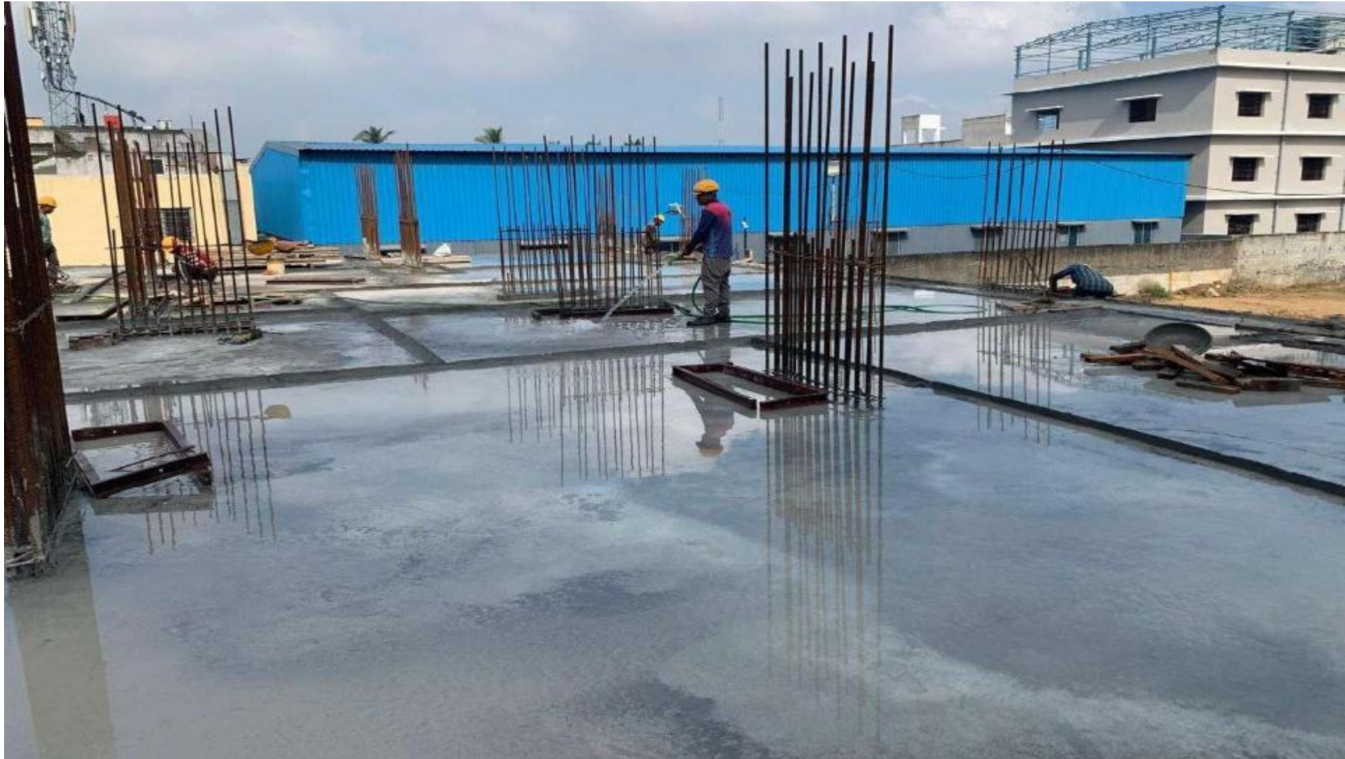
Pour 2 – stilt floor roof curing work in progress.
