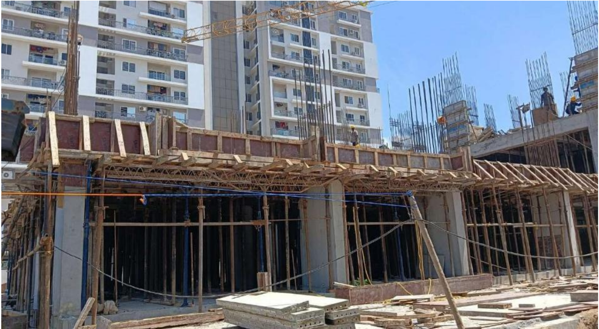
Pour-2 stilt floor roof outer shuttering work completed.
