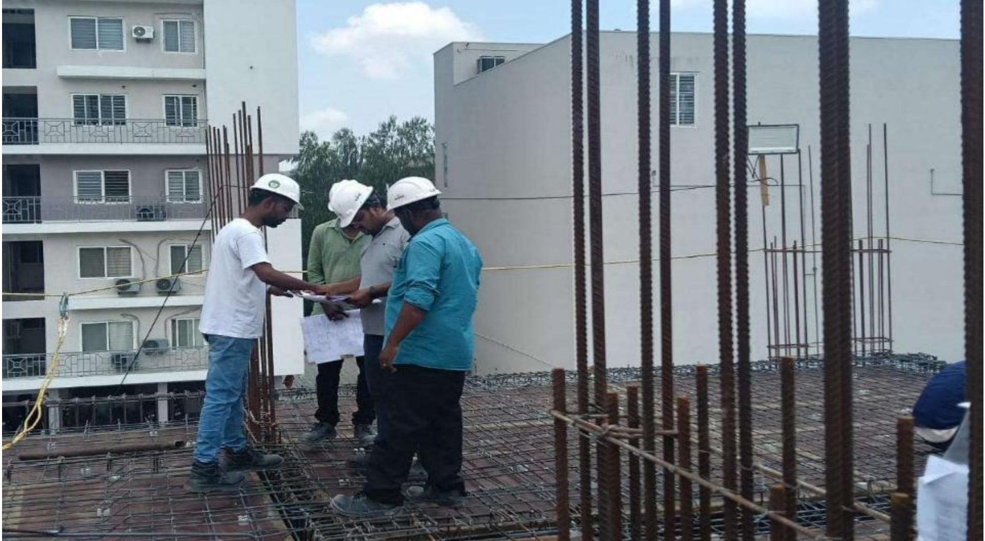
Pour 1 – 2 nd Floor roof reinforcement structural consultants inspection completed.
