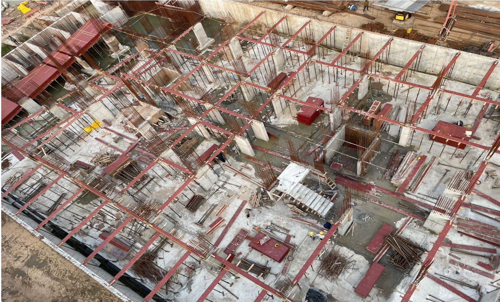
Tower-01 beam bottom shuttering work in progress.
