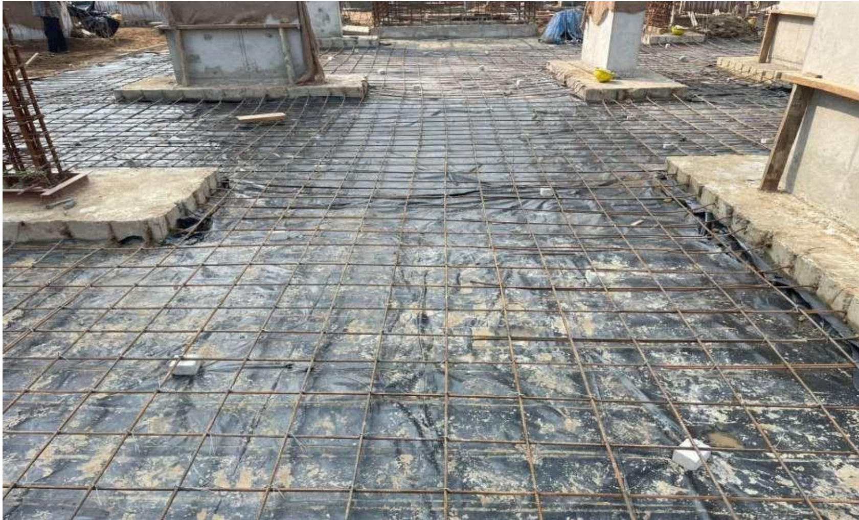
Pour-2 grade slab balance area reinforcement work completed .
