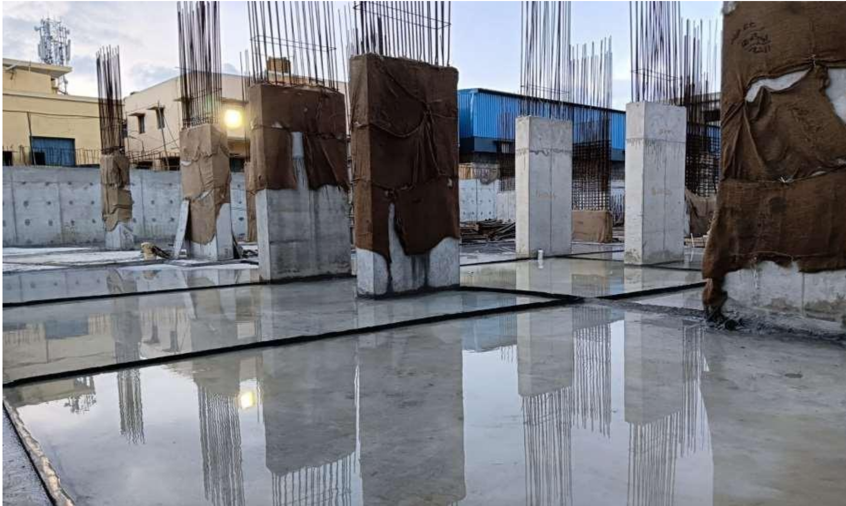
Grade slab curing work in progress.
