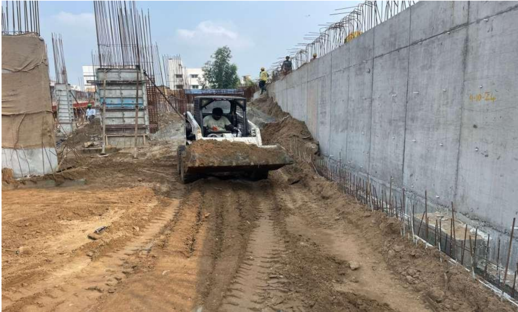
Basement Pour-2 remaining area soil backfilling work completed.
