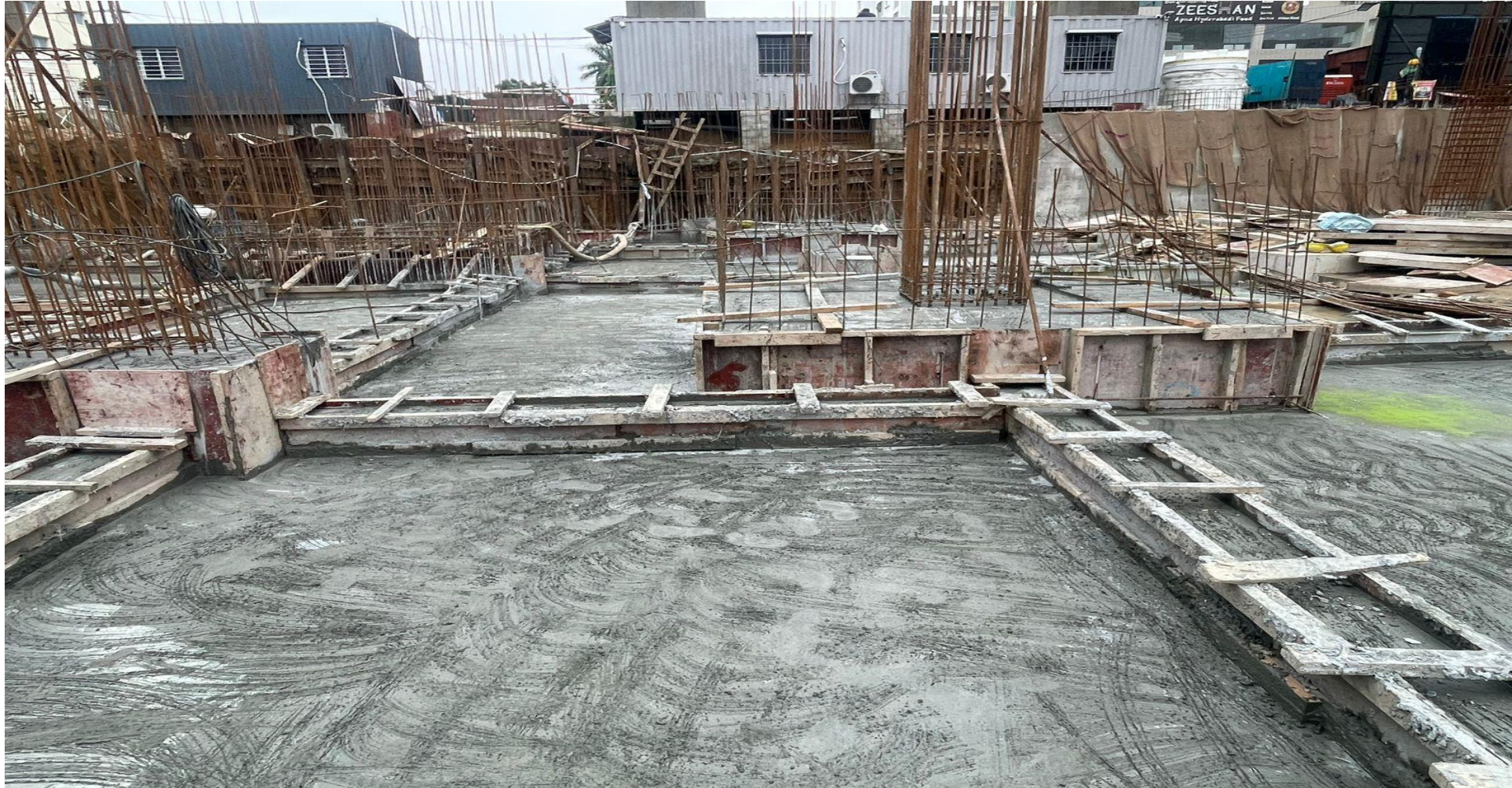
Tower -02 pour-03 pile cap raft concrete work completed.
