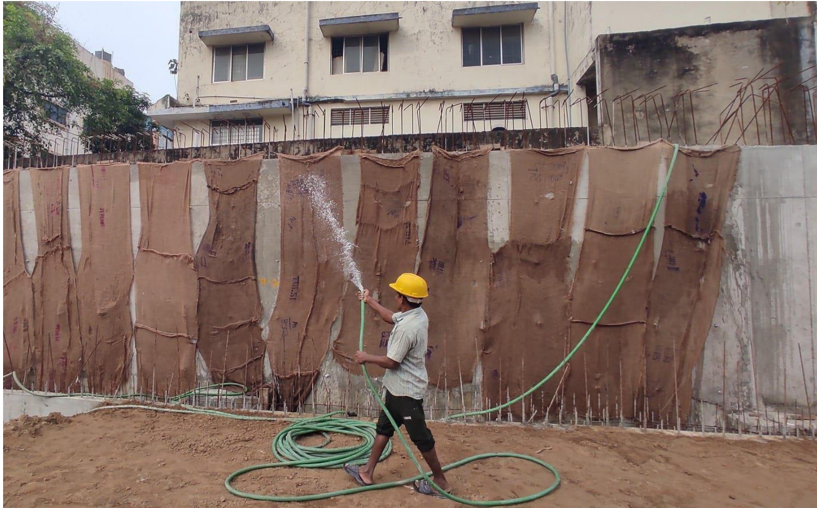
West side retaining wall curing work in progress.
