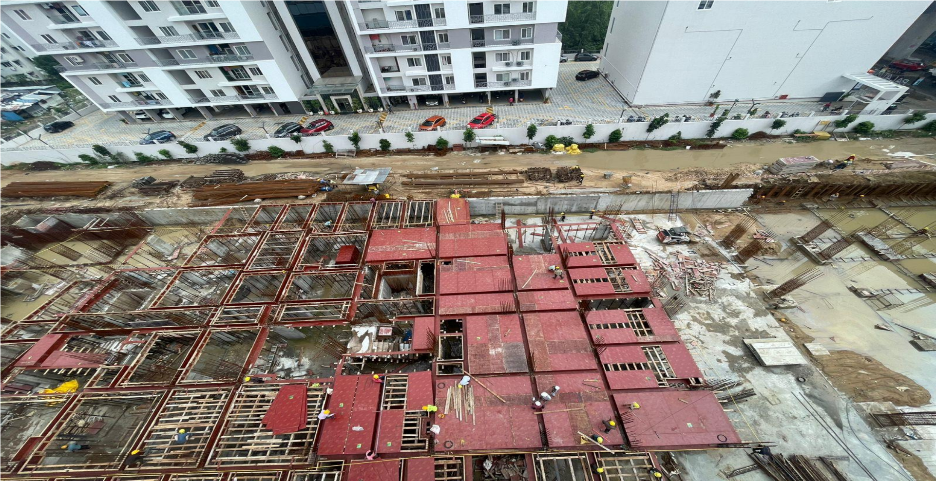
Tower -01 Roof slab Shuttering work in progress.
