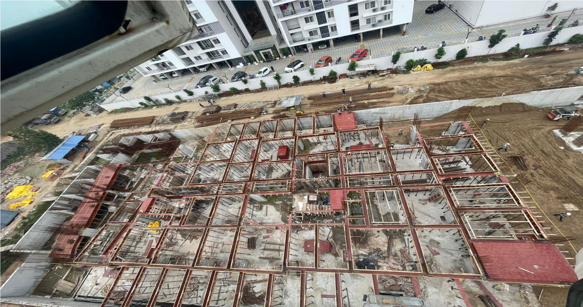
Tower -01 Roof Beam Shuttering work in Progress.
