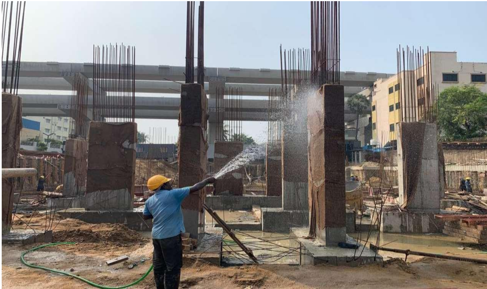
Second lift column curing work in progress.
