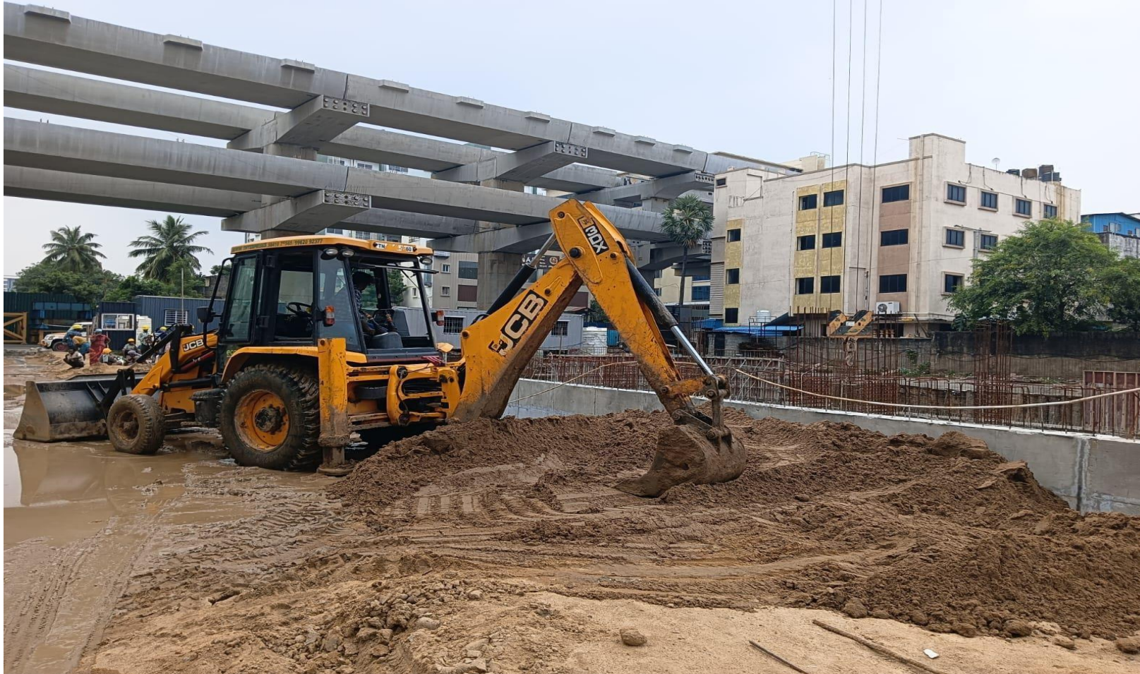
East side retaining wall backfilling work in progress.
