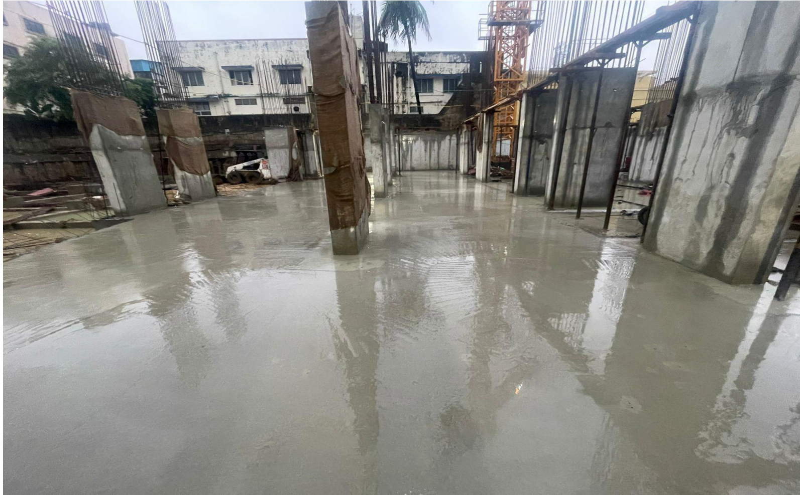
Basement pour-2&3 grade slab concrete work completed .
