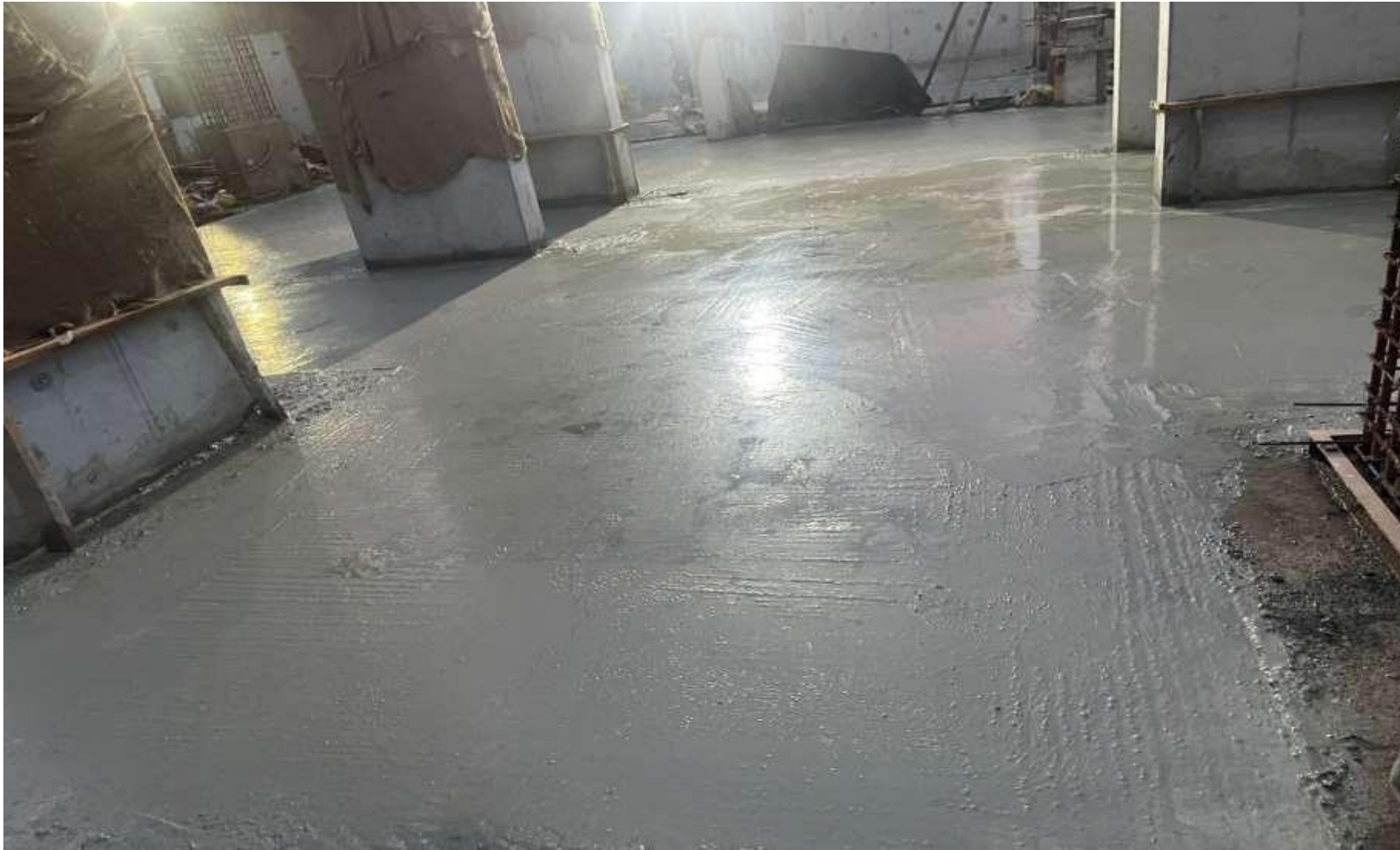
Pour-2 grade slab balance area concrete work completed.
