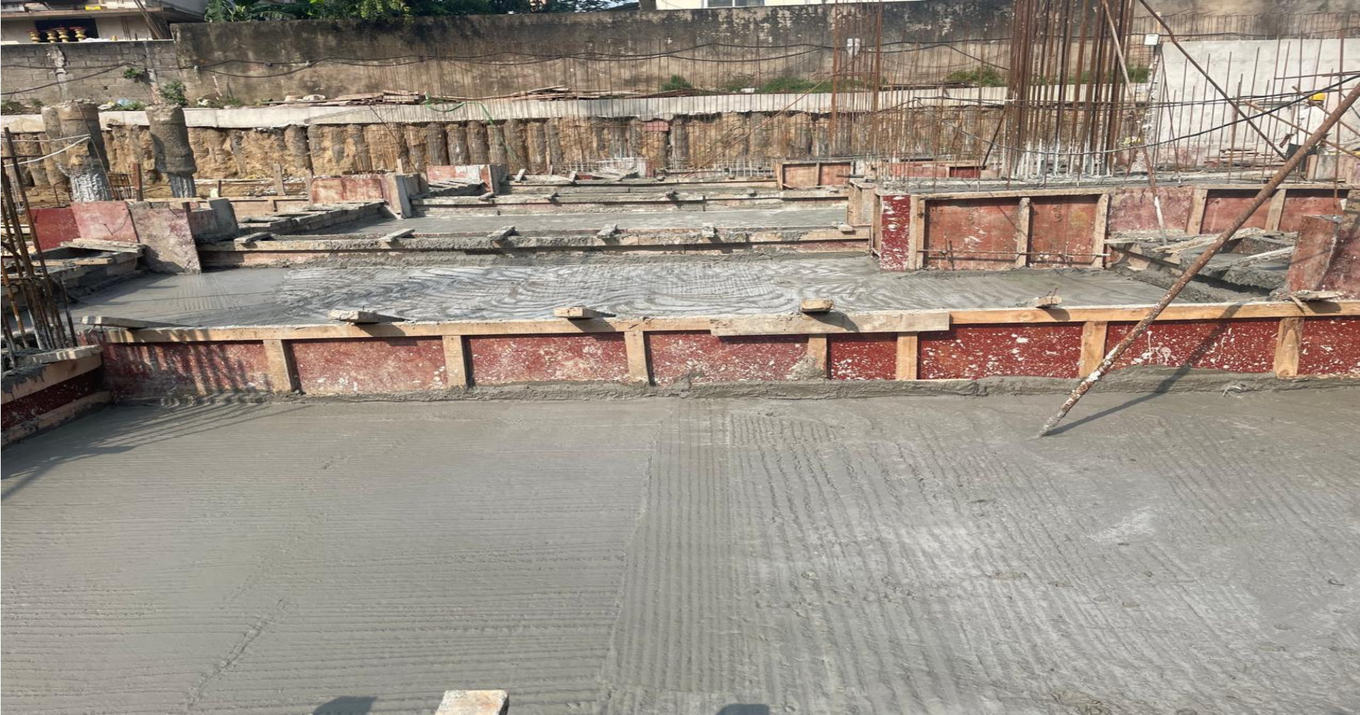
Basement pour-3 raft slab concrete work completed.
