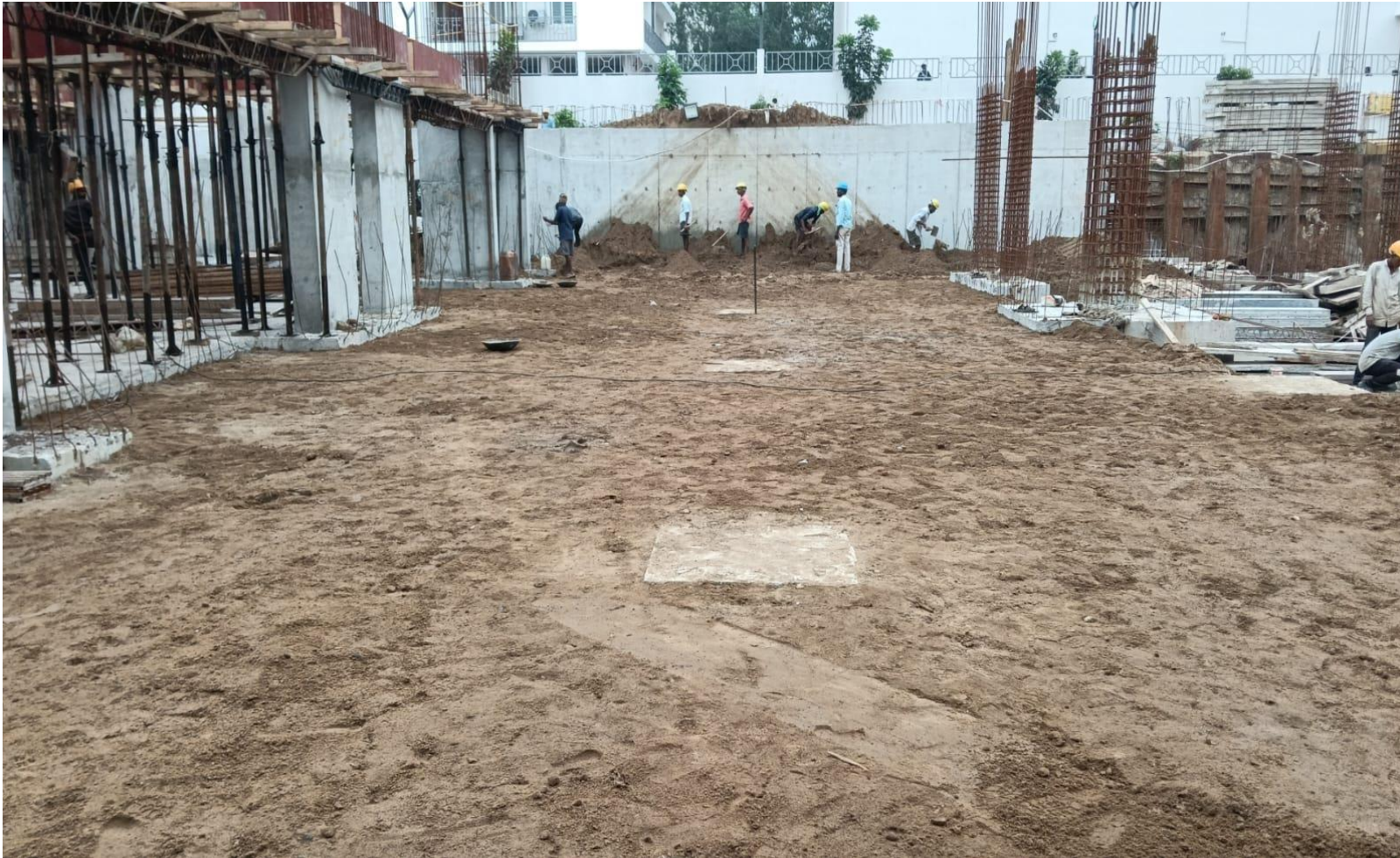
Basement Pour-3 soil levelling work in progress for grade slab .
