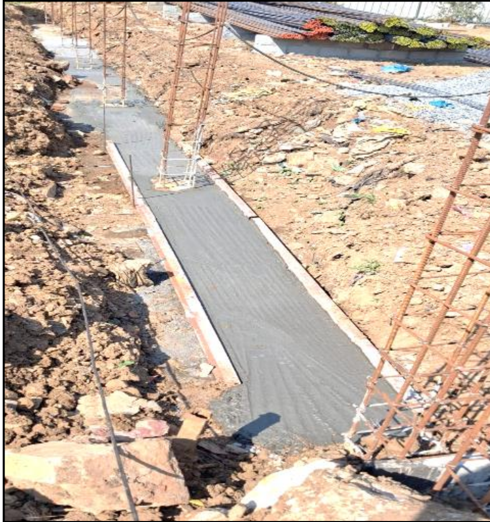
Compound wall – Plinth beam PCC work 39m completed (94/113m)
