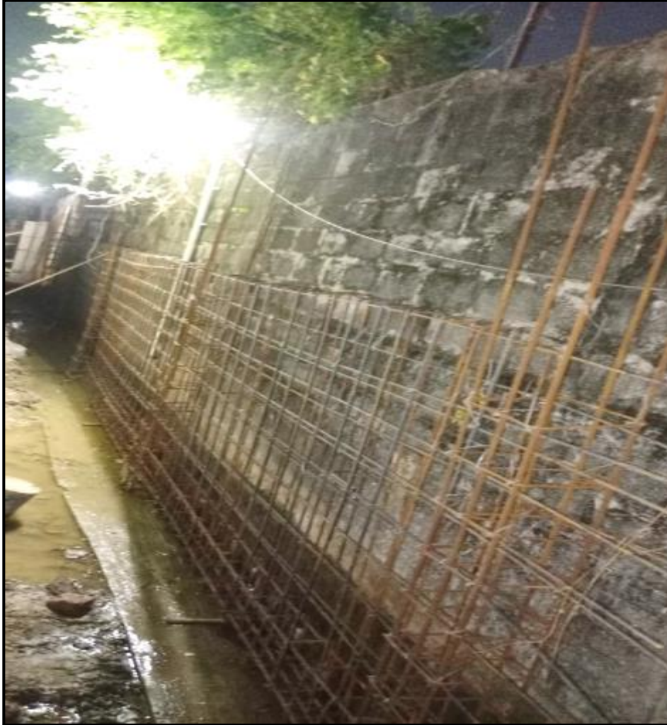
Compound wall plinth beam & RC wall reinforcement work 29m completed (70/113 m)
