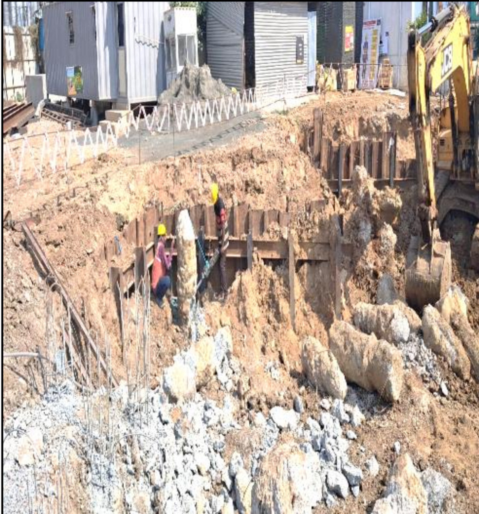
UG sump & Main building – Pile chipping 25 no's completed (110/182 Nos)
