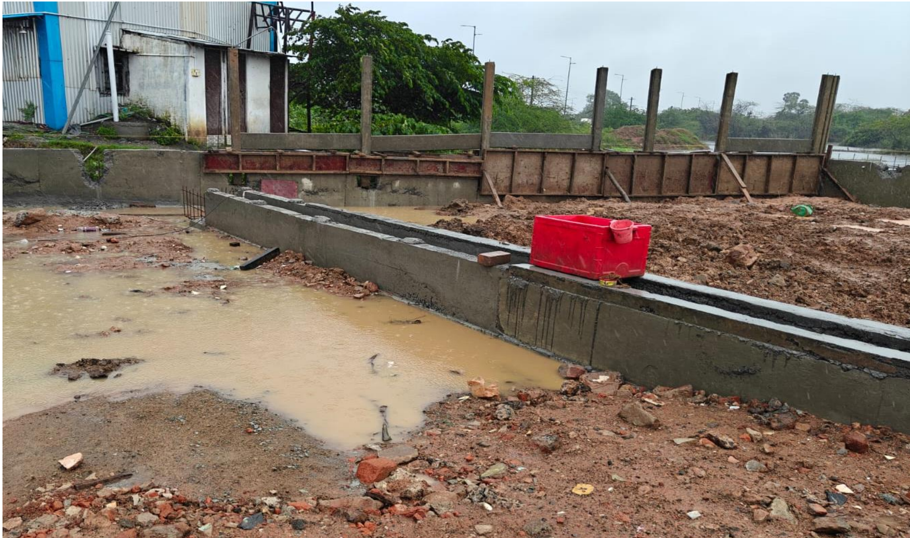
Trench Wall Concrete Work In Progress
