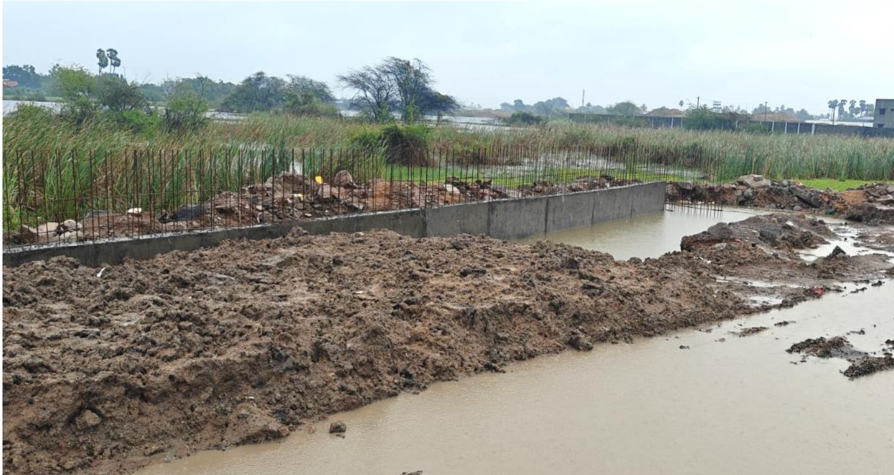
East Side Retaining Wall 1 st Lift Concrete Work In Progress
