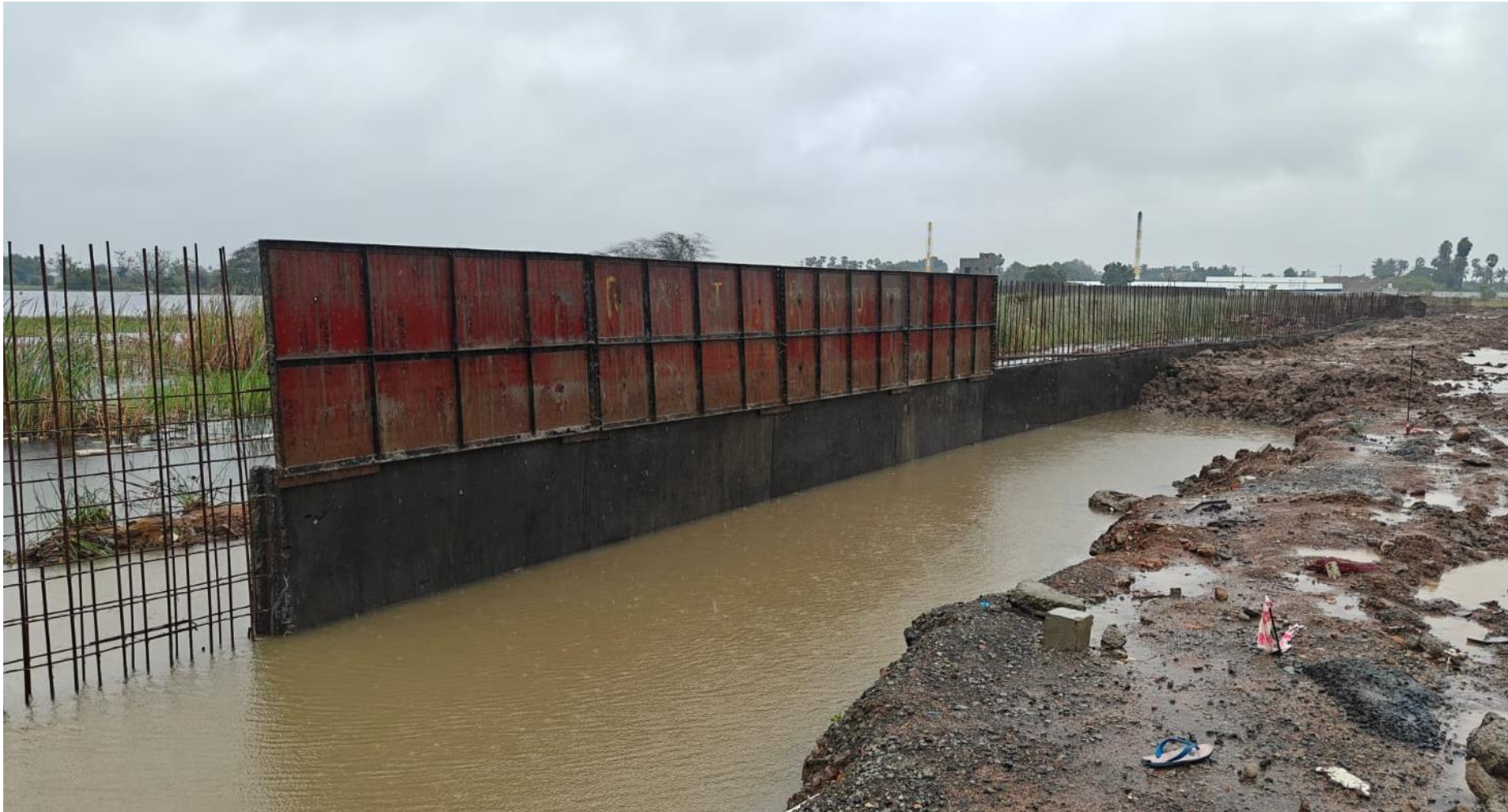
East Side 2 nd Lift Shuttering Work In Progress
