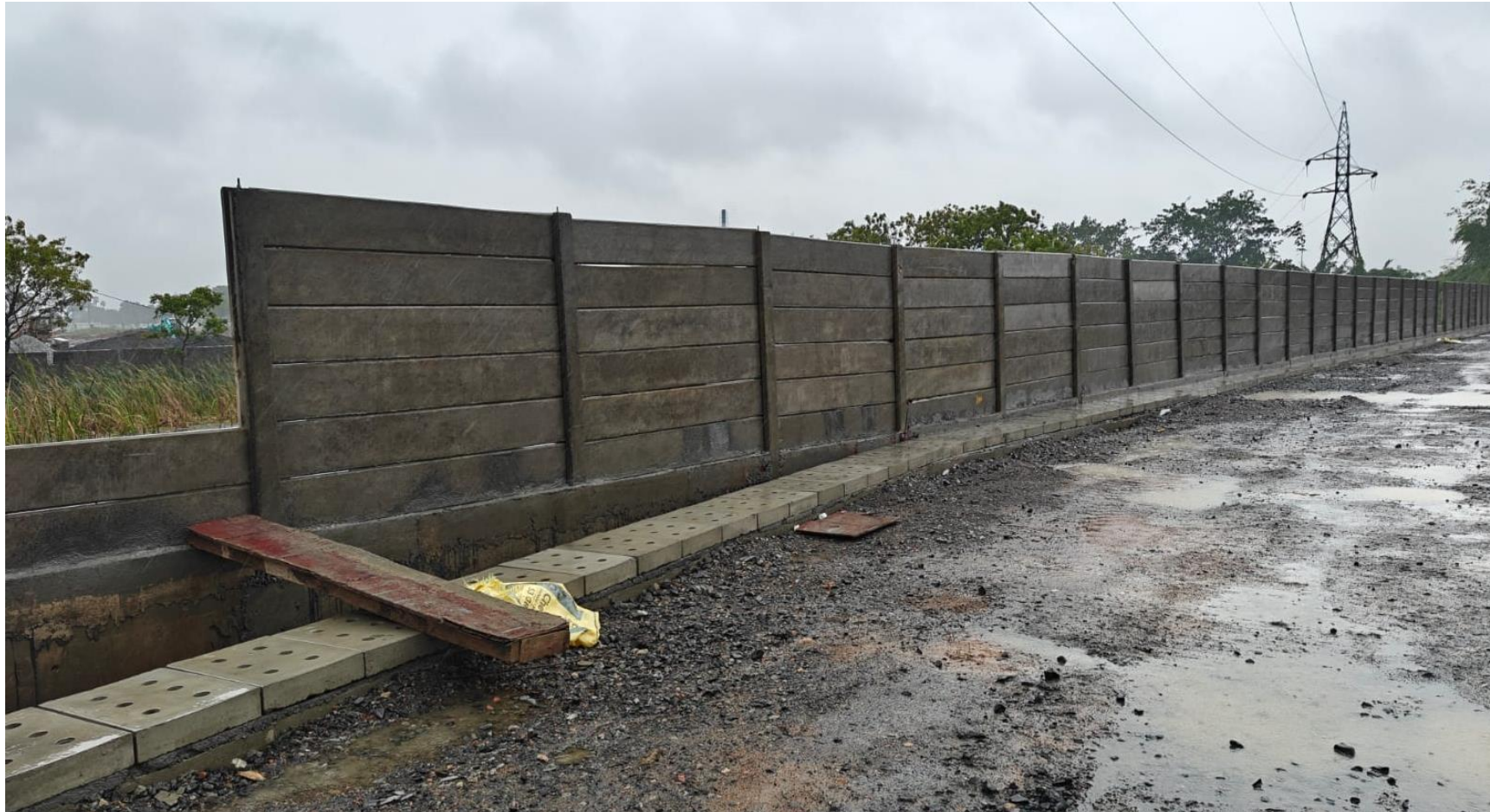
Pre-cast Compound Wall Slab Erection In Progress
