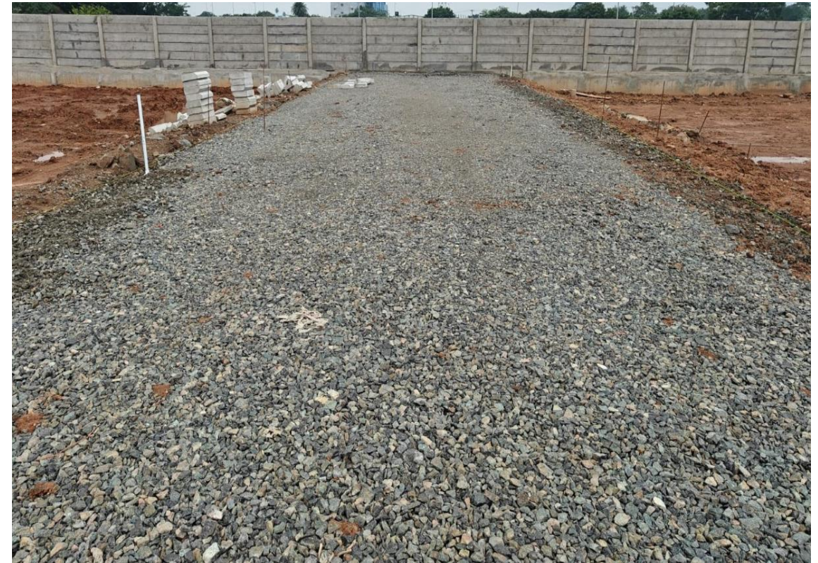
Road WMM Compaction Works In Progress
