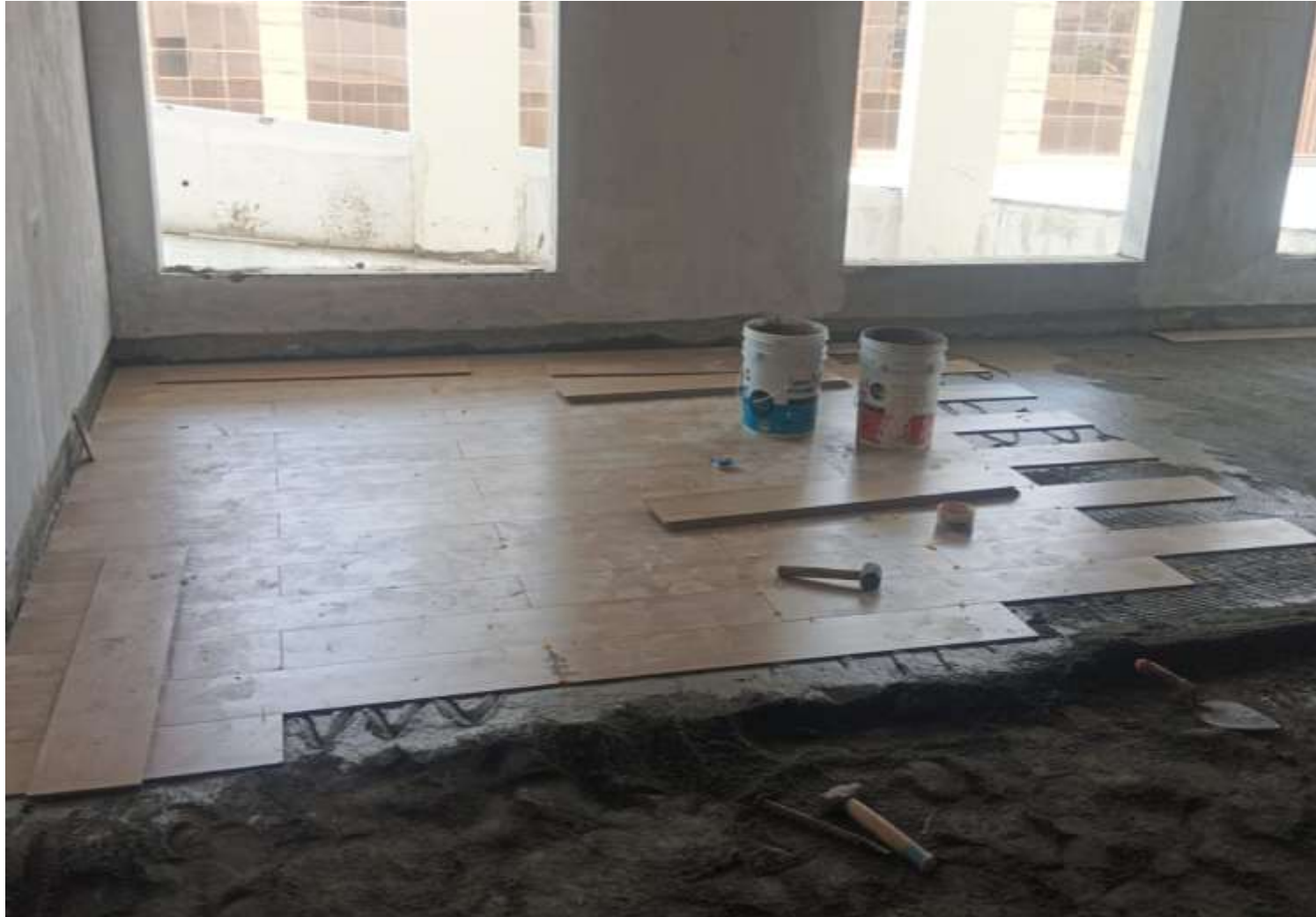
MULTIPURPOSE HALL TILE LAYING WORK IN PROGRESS
