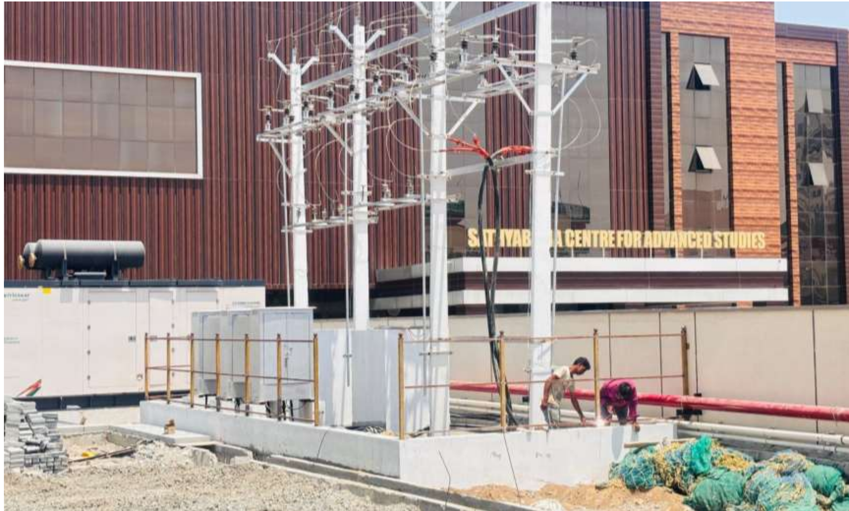
TRANSFORMER YARD FENCING WORK IN PROGRESS
