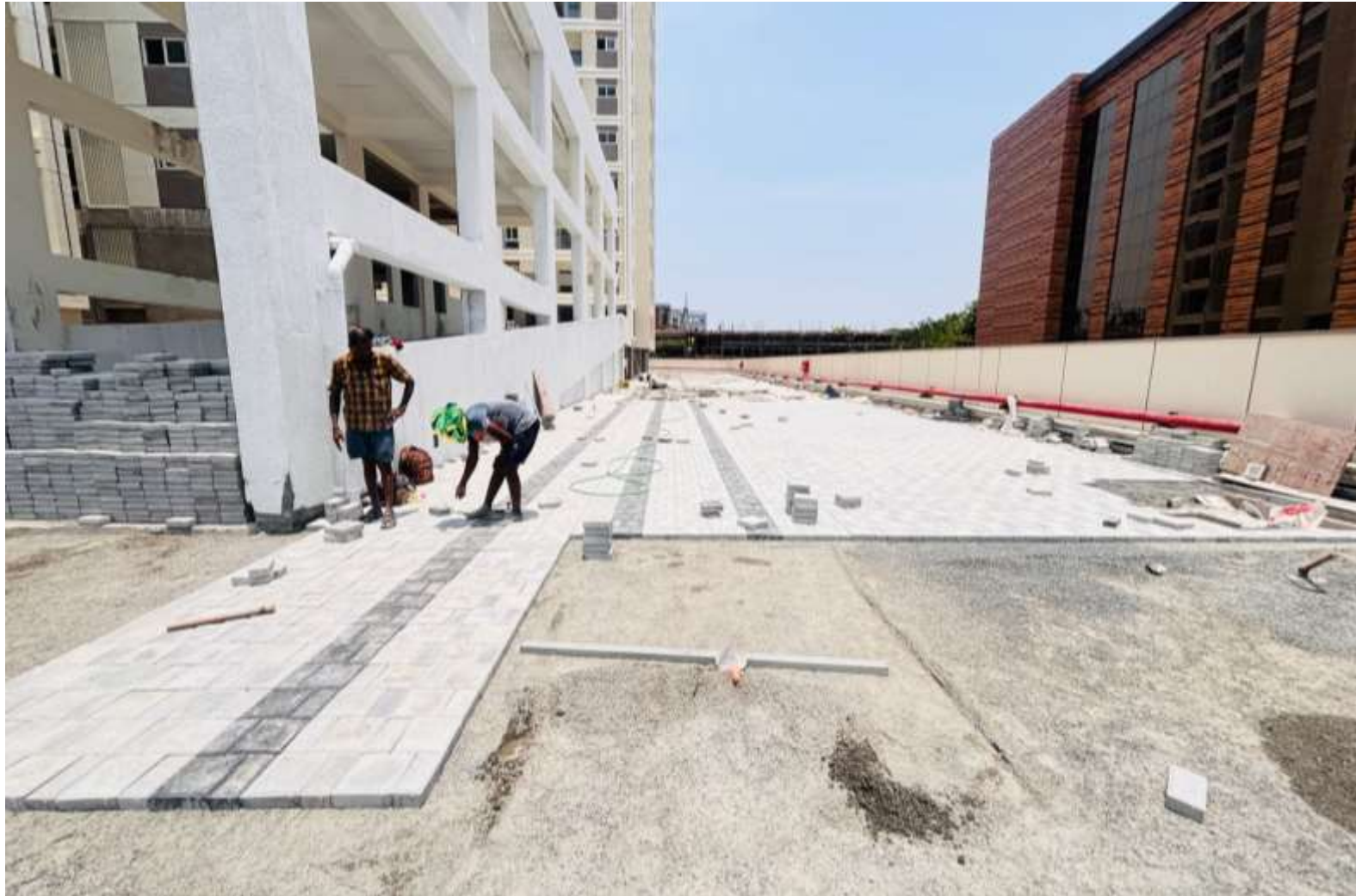
WEST SIDE PAVER BLOCK LAYING WORK IN PROGRESS
