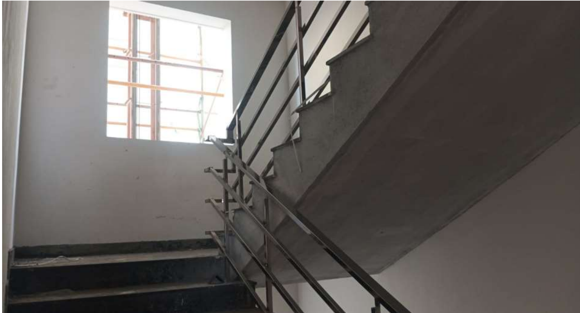
BLOCK 2 POUR 1 – STAIRCASE SS HANDRAIL FINISHING WORK IN PROGRESS
