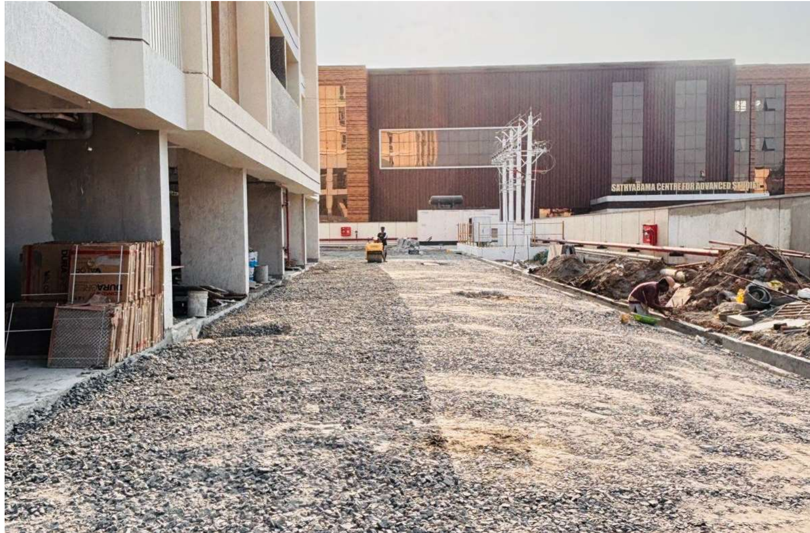
NORTH SIDE GSB COMPACTION WORK IN PROGRESS
