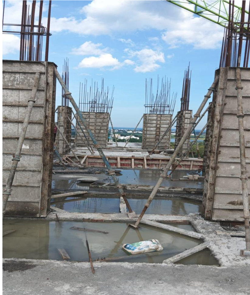
BLOCK 2 POUR 2 – THIRTEENTH FLOOR COLUMN CONCRETE WORKS IN PROGRESS
