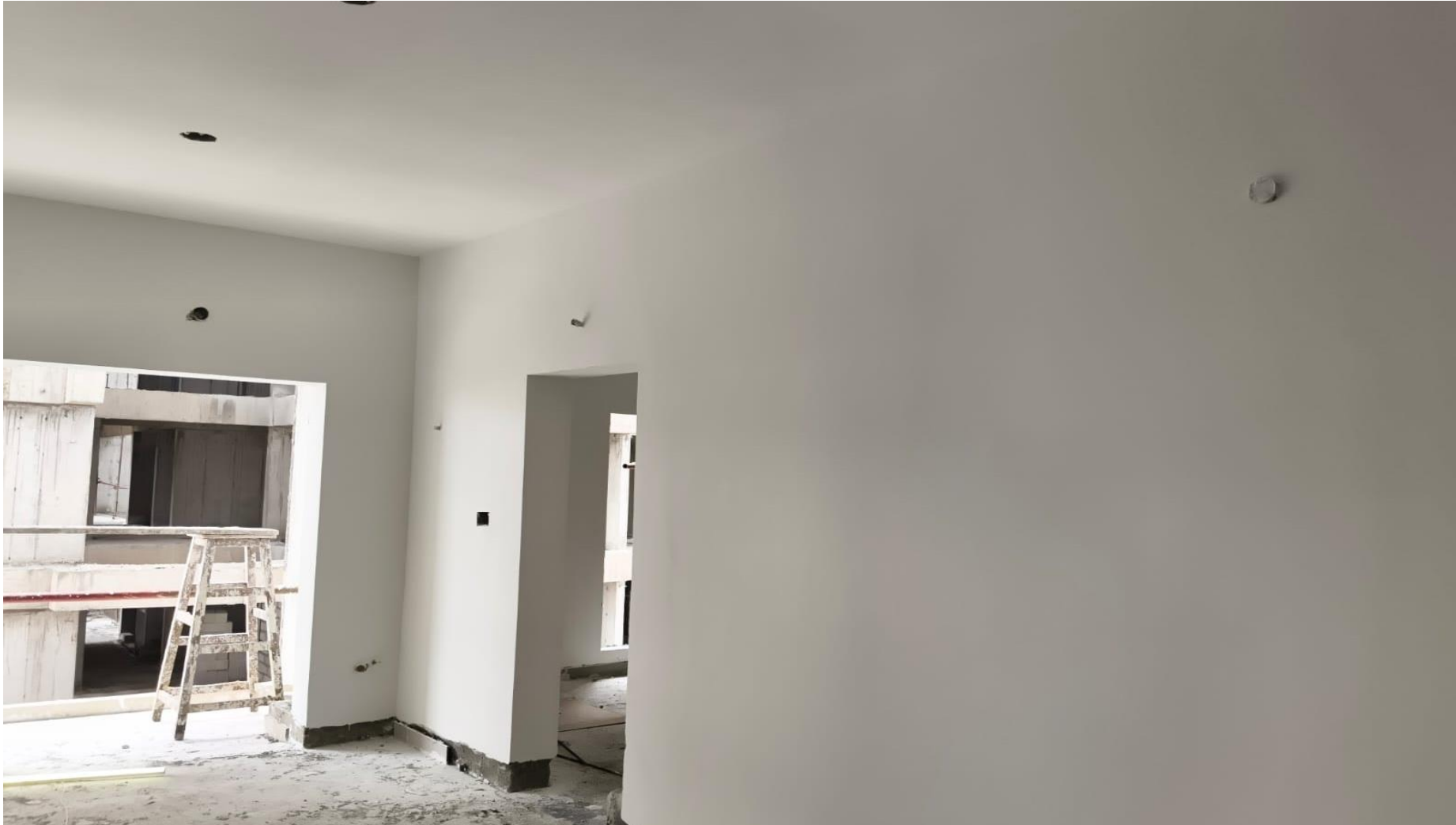
BLOCK 1 – NINTH FLOOR SECOND COAT PUTTY WORK IN PROGRESS
