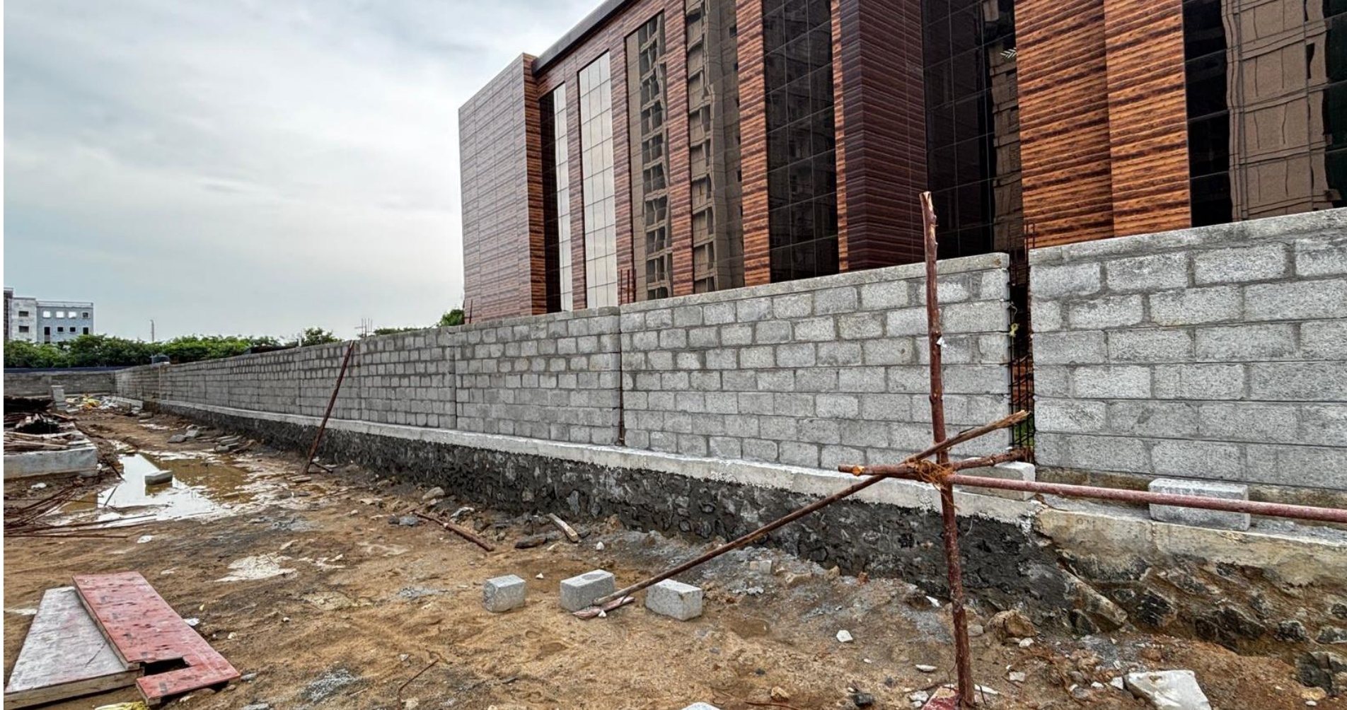
WEST SIDE COMPOUND WALL BLOCKWORK COMPLETED
