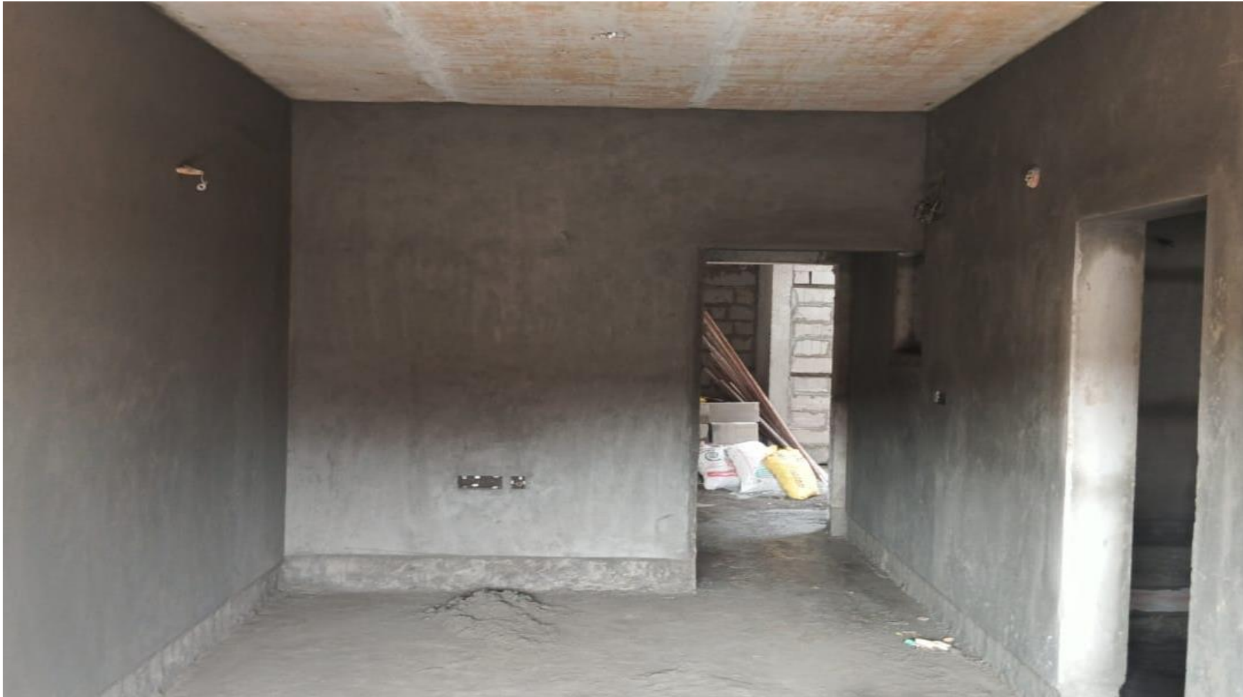
BLOCK 2 POUR 2 – SECOND, THIRD & FOURTH FLOOR INTERNAL PLASTERING COMPLETED
