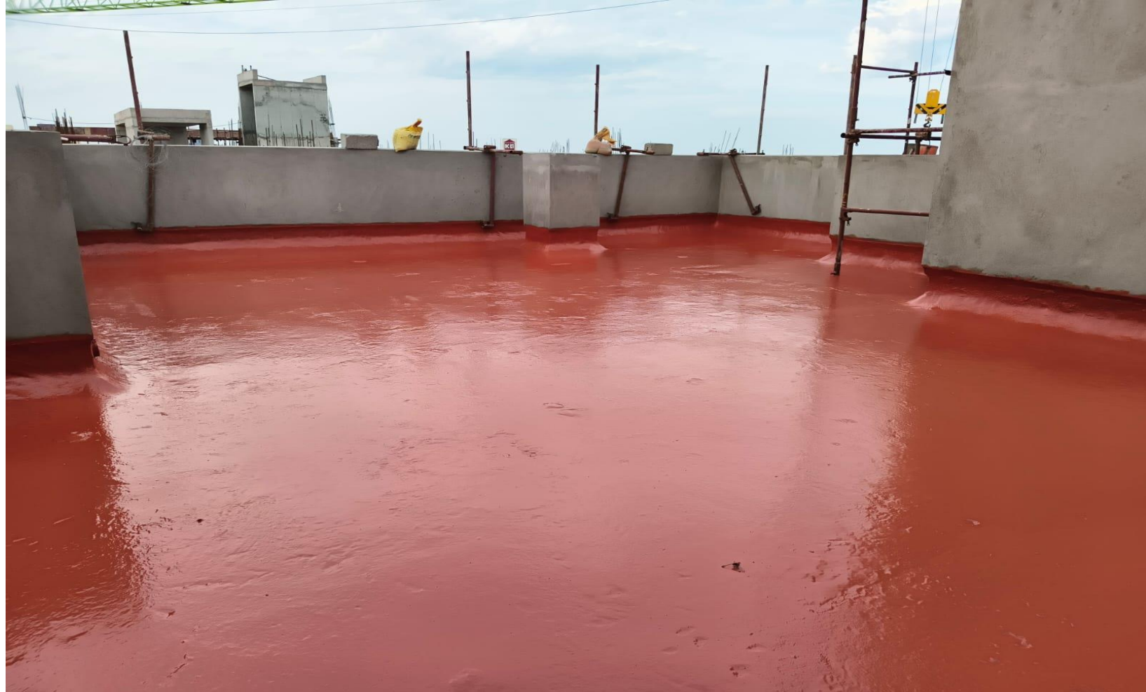
BLOCK 1 – TERRACE BAY 2 PU COATING COMPLETED
