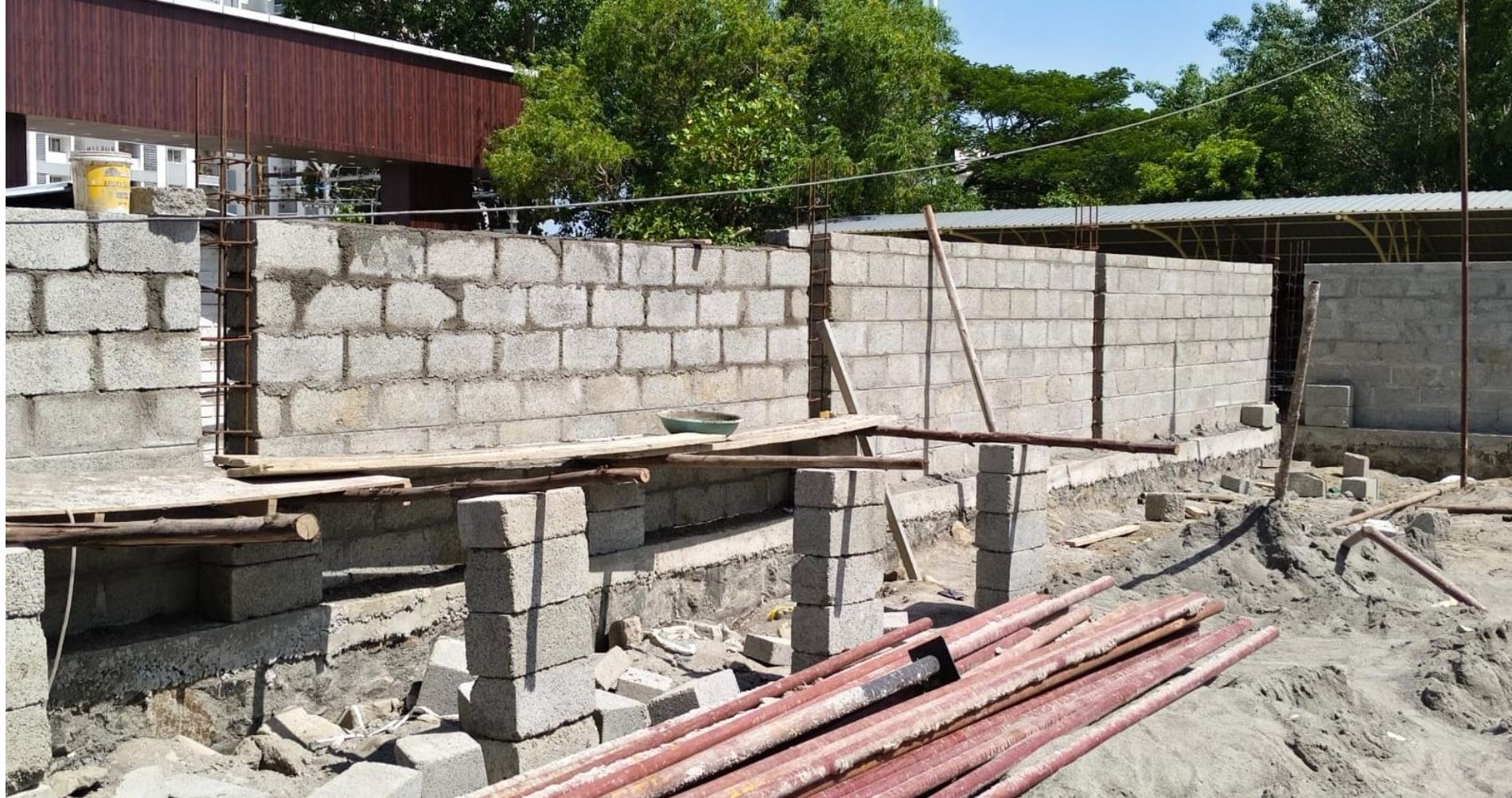
EAST SIDE COMPOUND WALL BLOCKWORK IN PROGRESS
