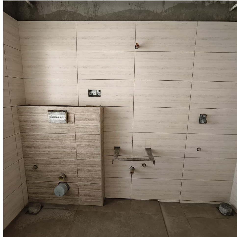
BLOCK 1 – ELEVENTH FLOOR TOILET WALL TILES LAYING WORK IN PROGRESS
