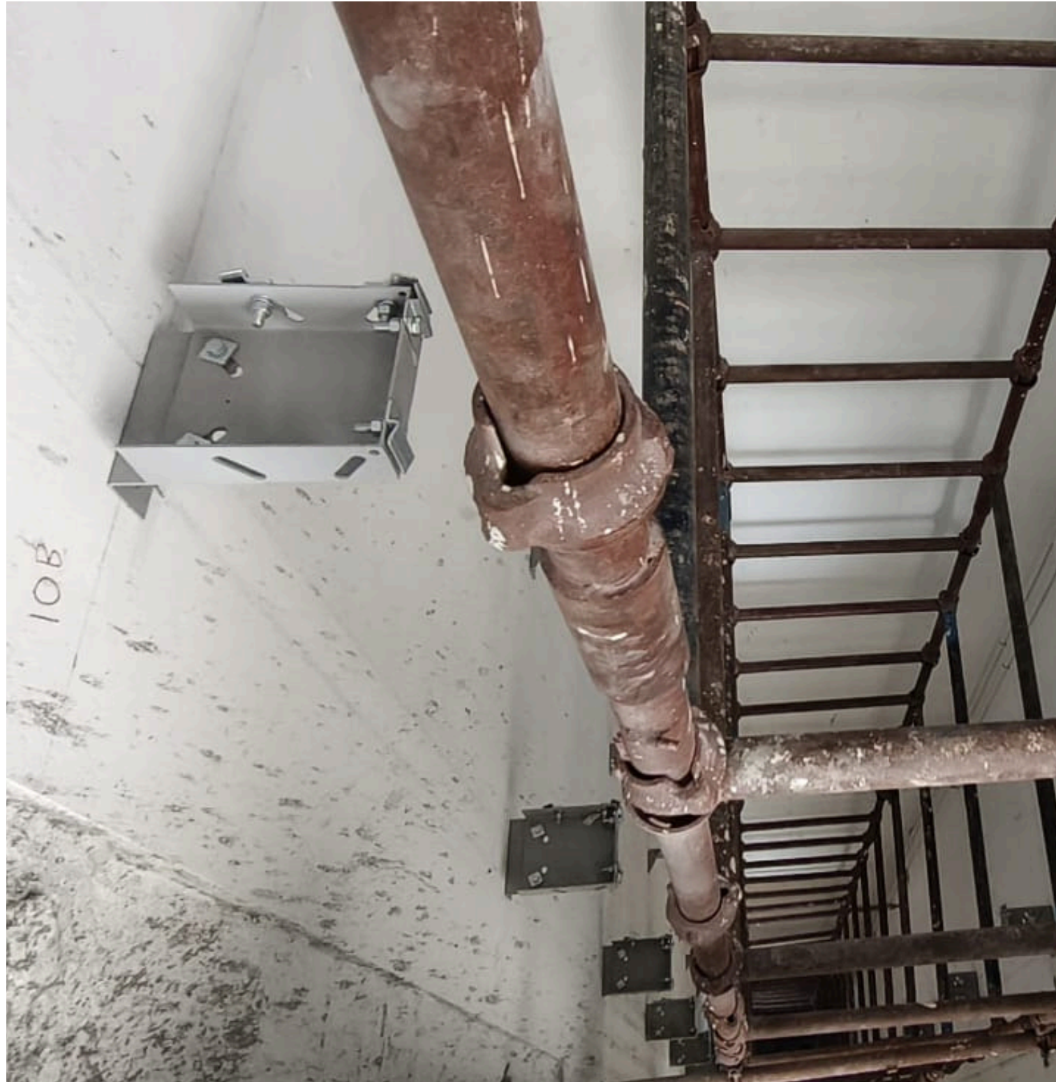
Main Building Pour-1 Lift Fixing Work In Progress.
