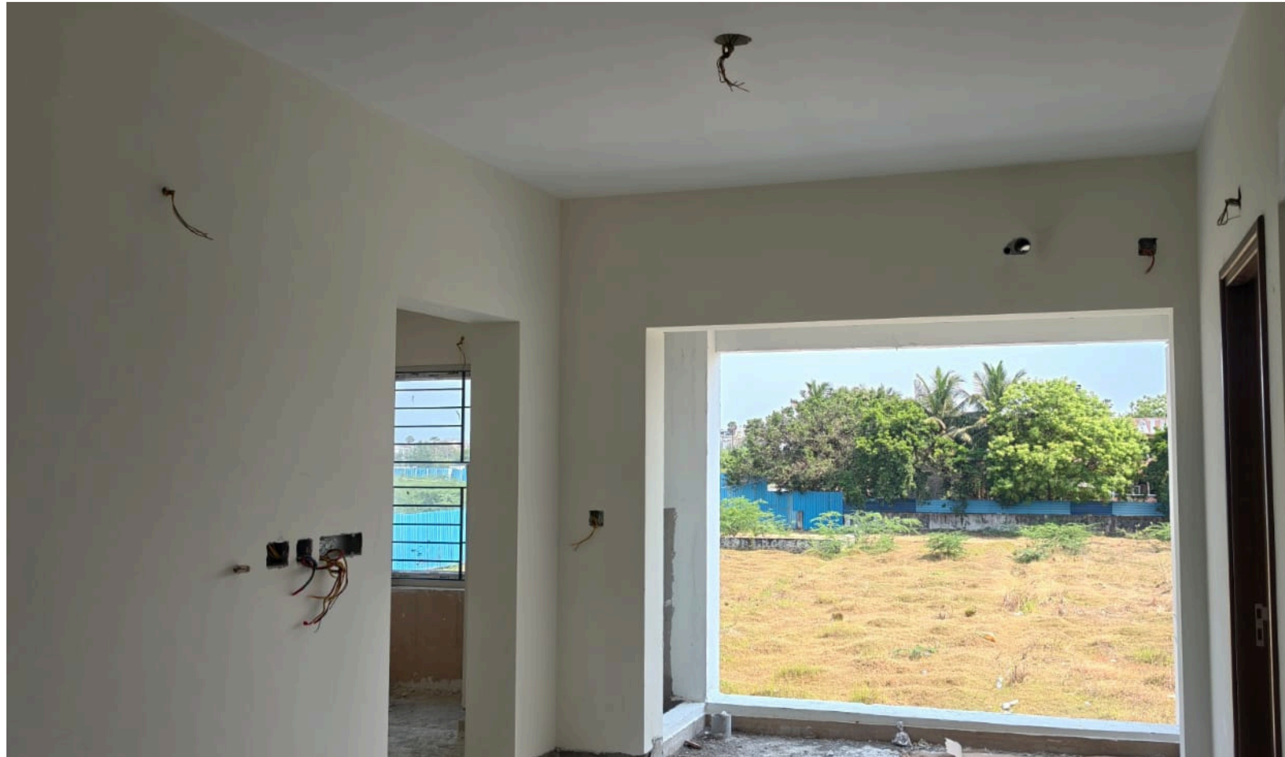
Main Building Pour-1 Electrical 1 st Floor Flat Wiring Work In Progress.
