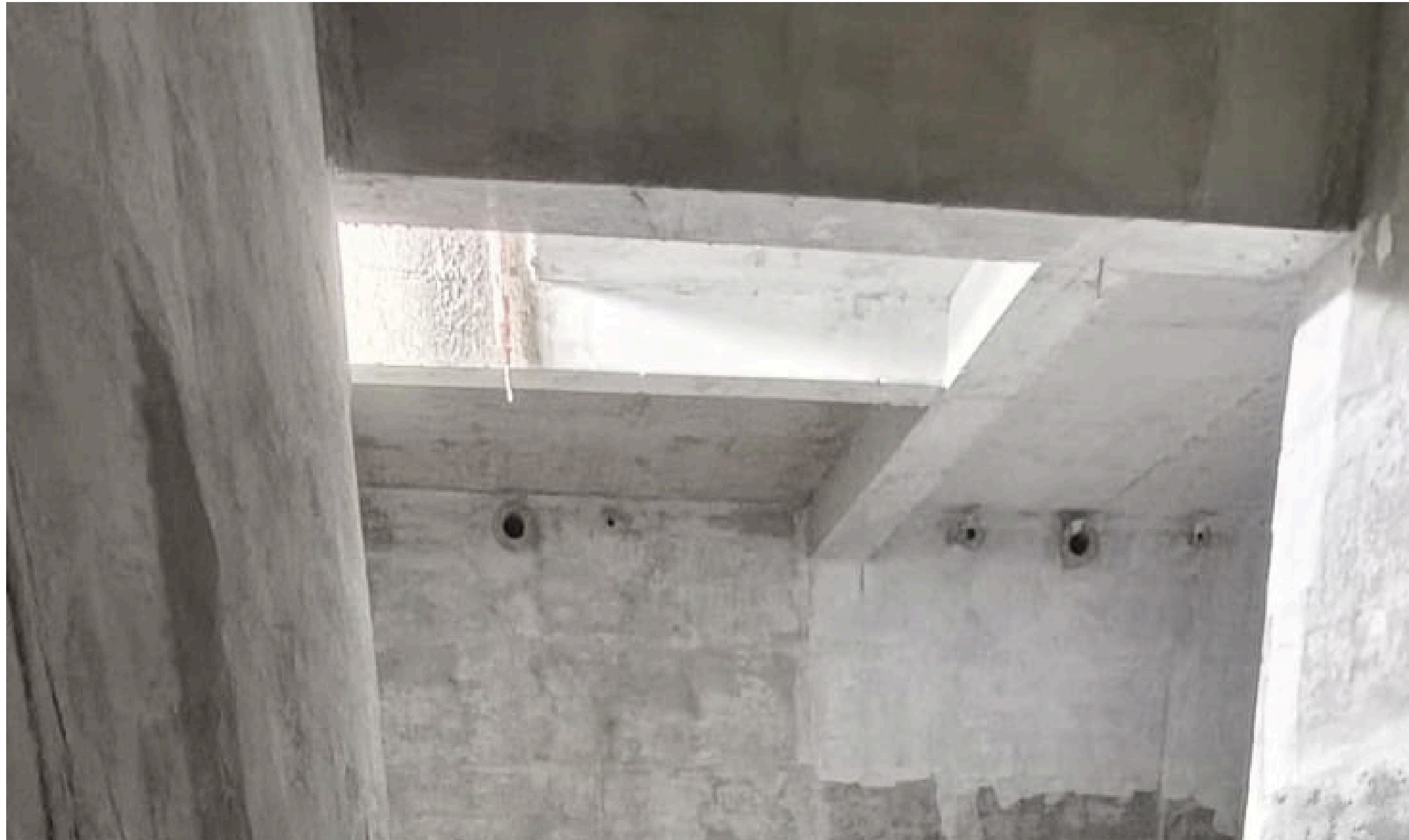
UG Sump Pump and Pedestal Work Completed.
