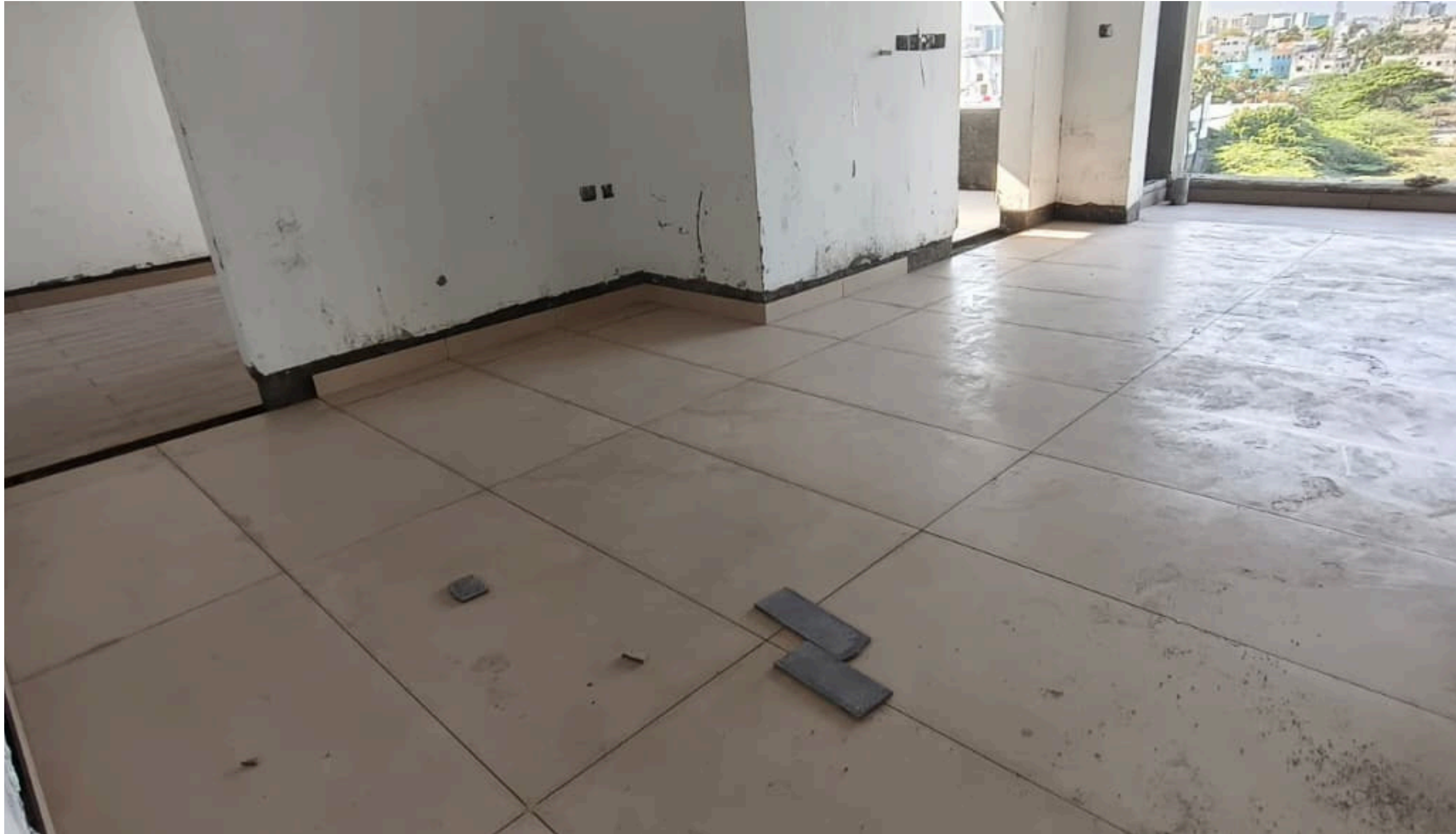
Main Building Pour-2 5 th floor Tiles Work In Progress.
