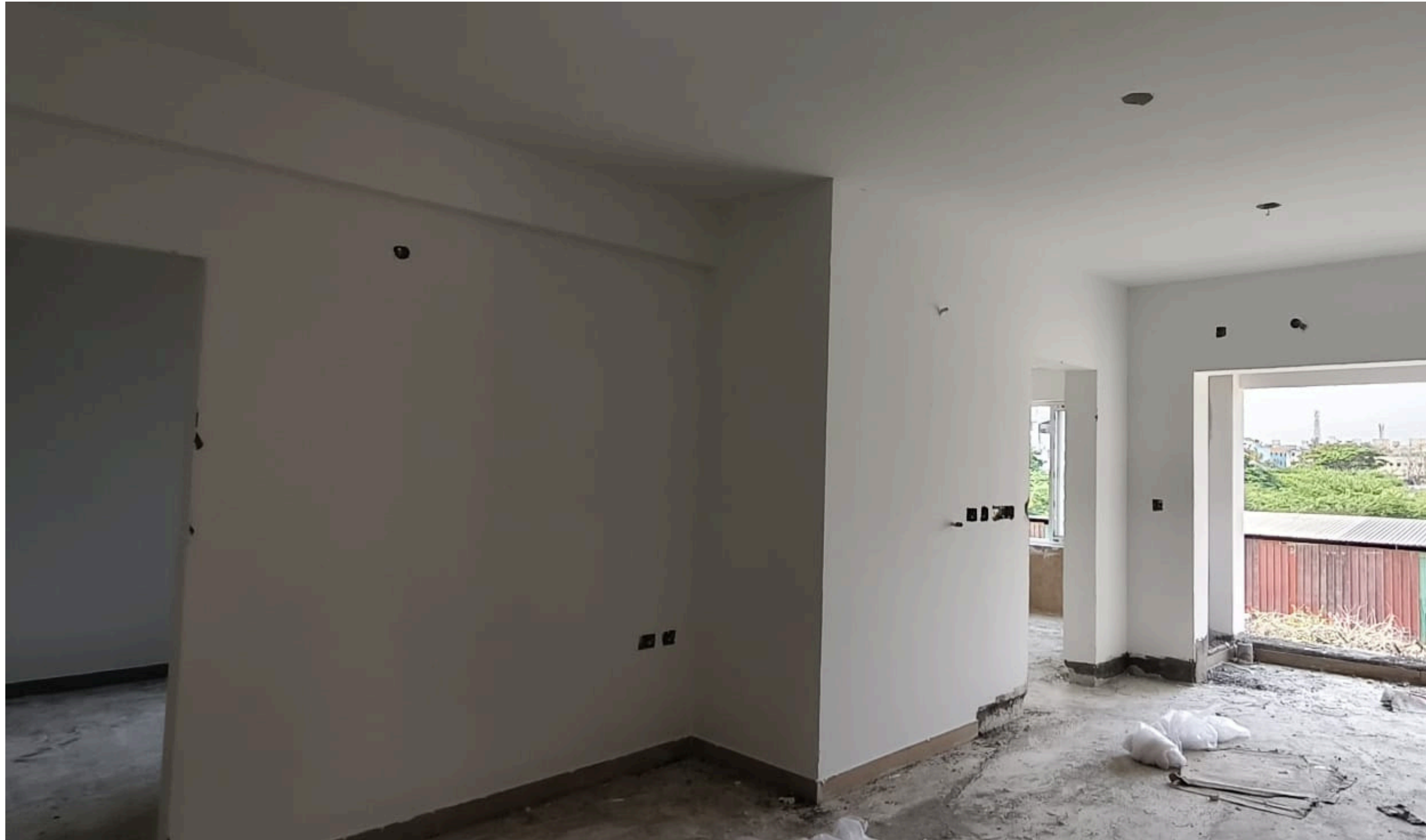
Main Building Pour-2 1 st Floor Putty Work In Progress.
