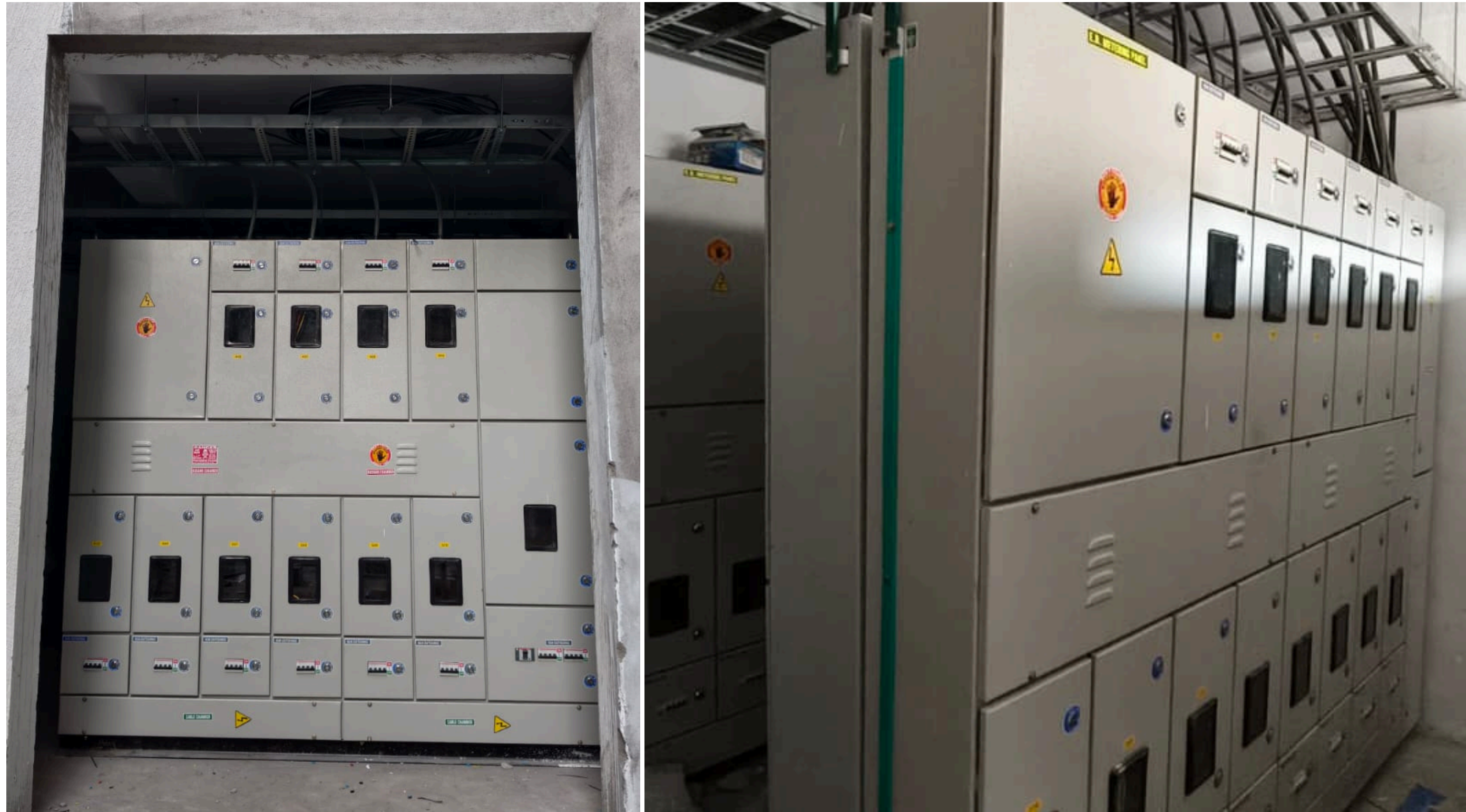
Main Building Electrical Panel Room Cable Connection Work Completed.
