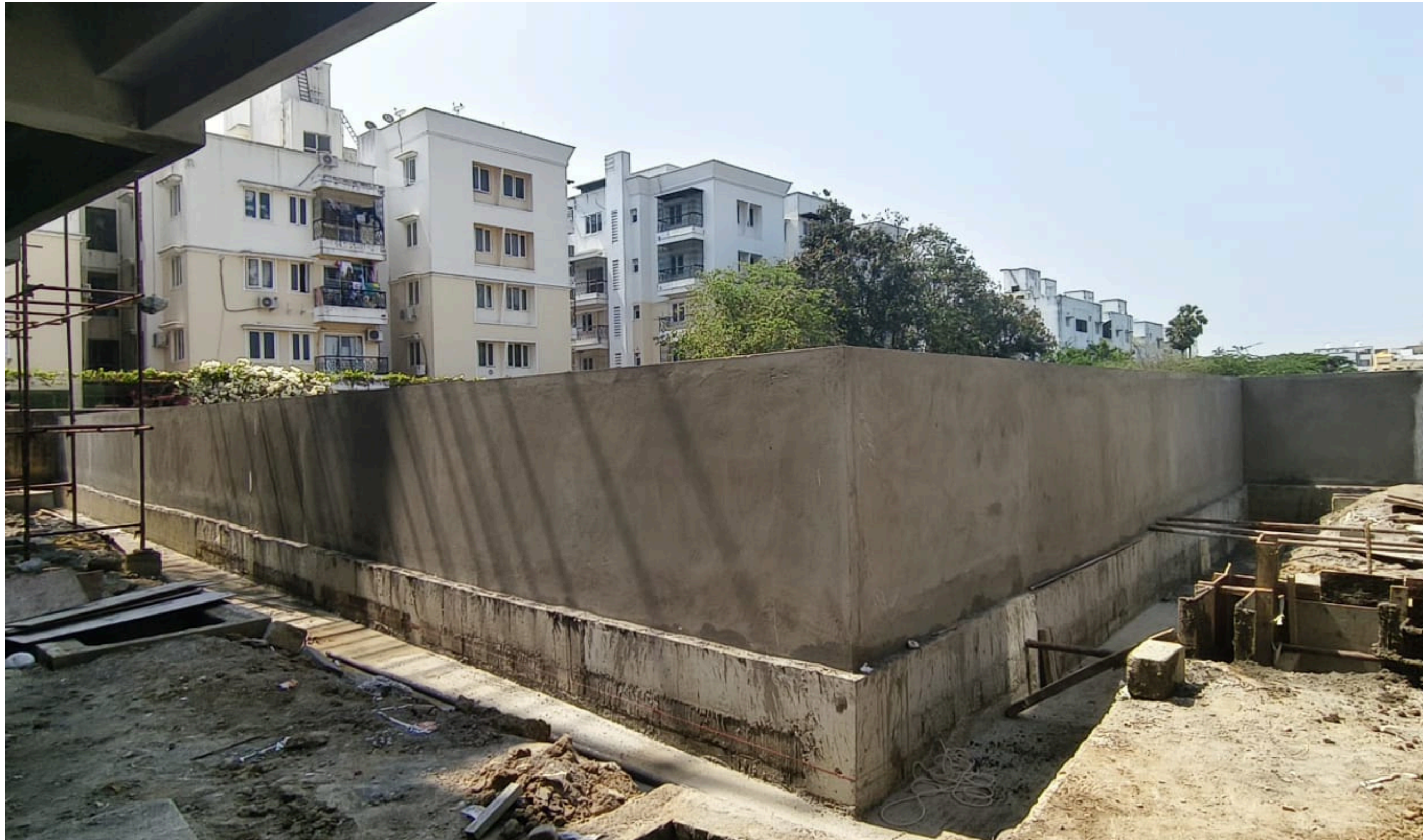
Compound Wall Plastering Work Completed.
