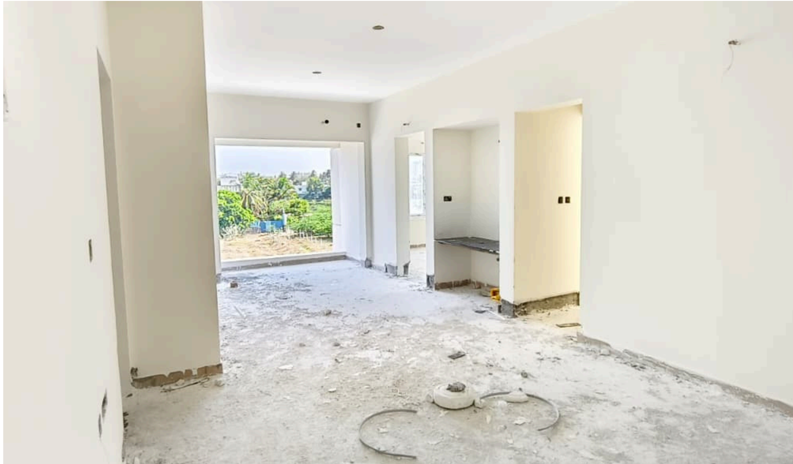
Main Building Pour-1 1 st Floor 1 st Coat Painting Work Completed.
