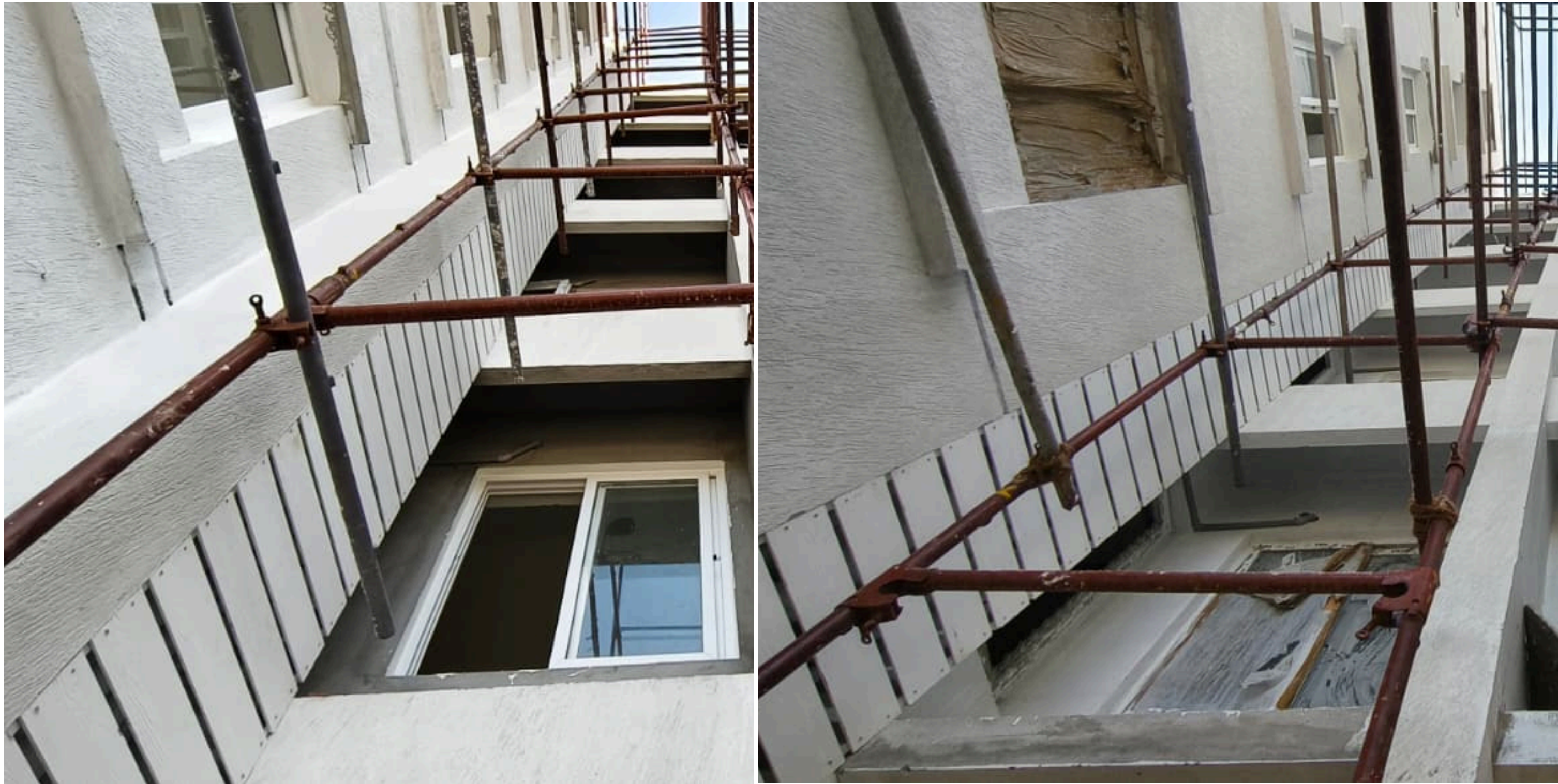
Main Building Plumbing Shaft Shera Plank Covering Work In Progress.
