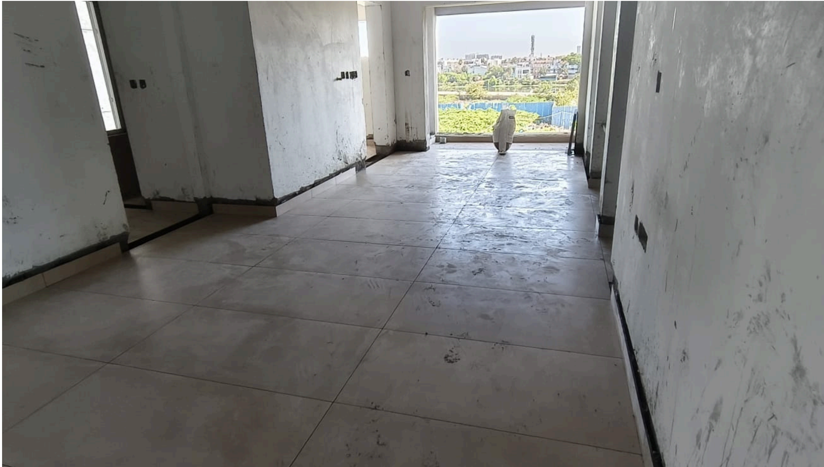
Main Building Pour-2 4 th floor Tiles Work Completed.
