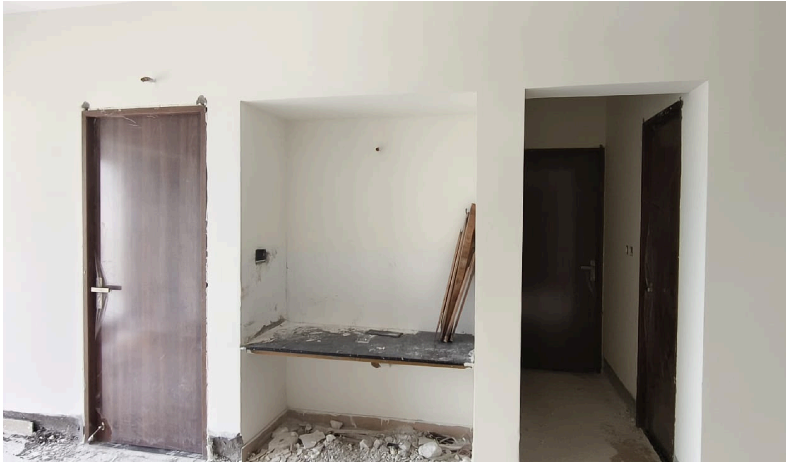
Main Building Pour-1 3 rd Floor Flat Door Fixing Work Completion.
