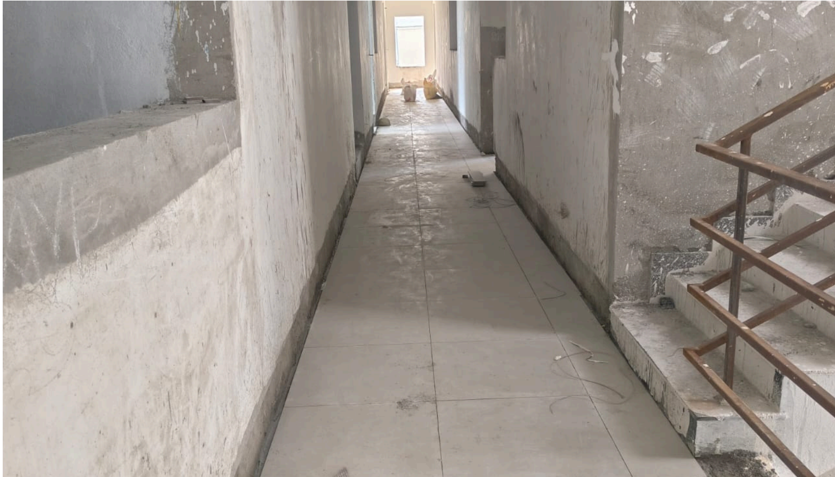
Main Building 3 rd Floor Corridor Tiles Laying Work In Progress.
