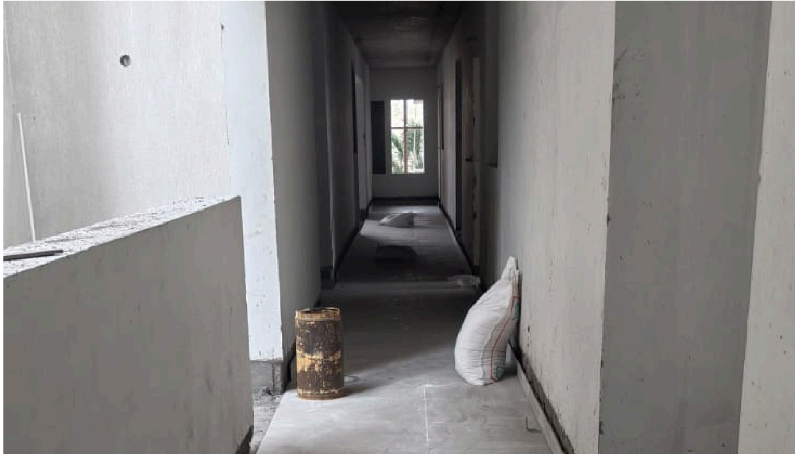
Main Building 1 st Floor Corridor Tiles Laying Work Completed.
