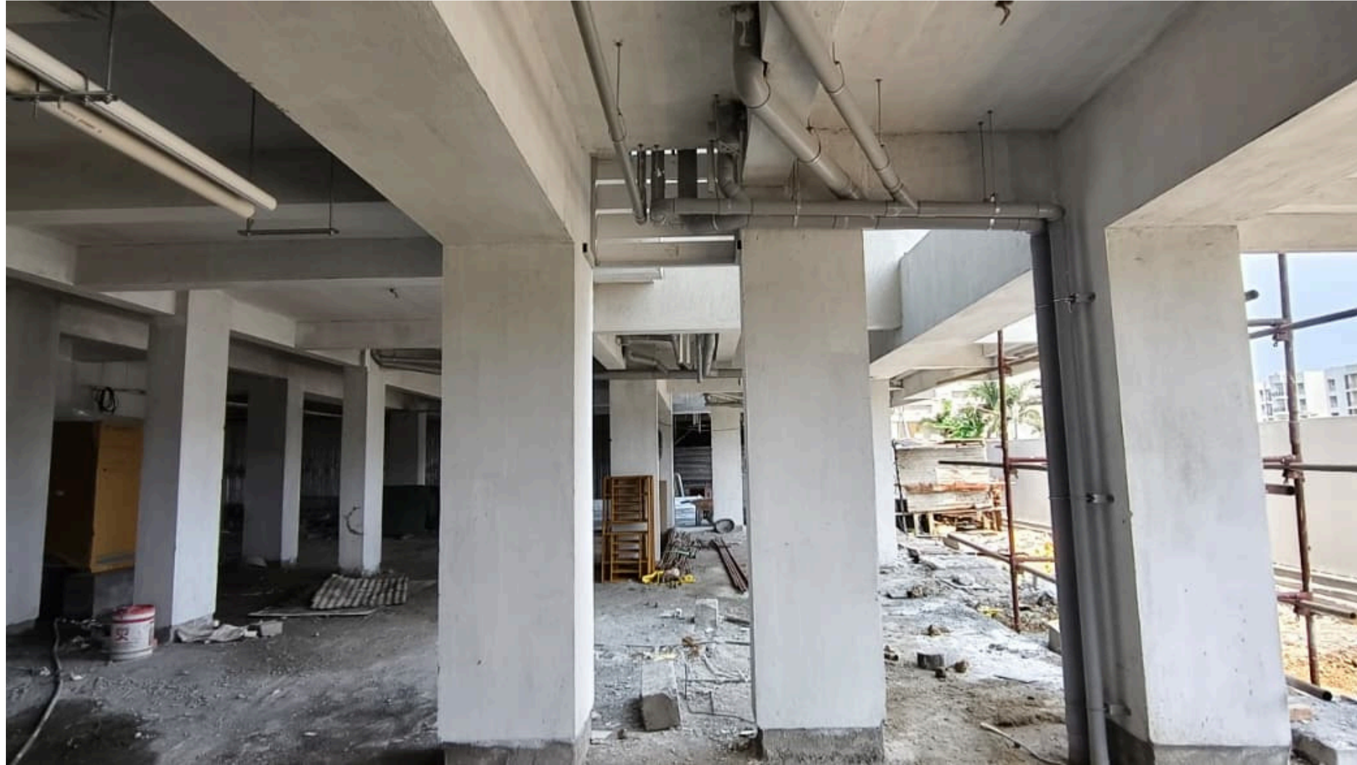
Main Building Pour-2 Stilt Floor Plumbing Work In Progress.
