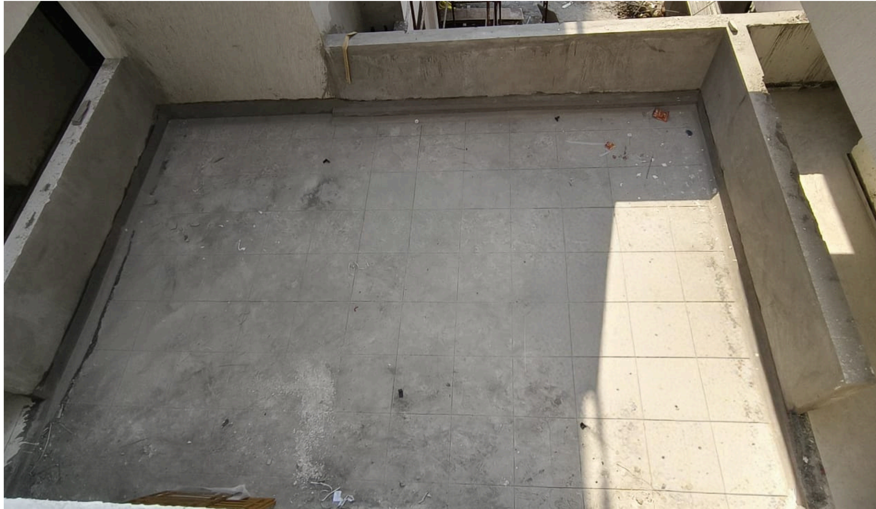
Kids Play Area Waterproofing Work Completed.
