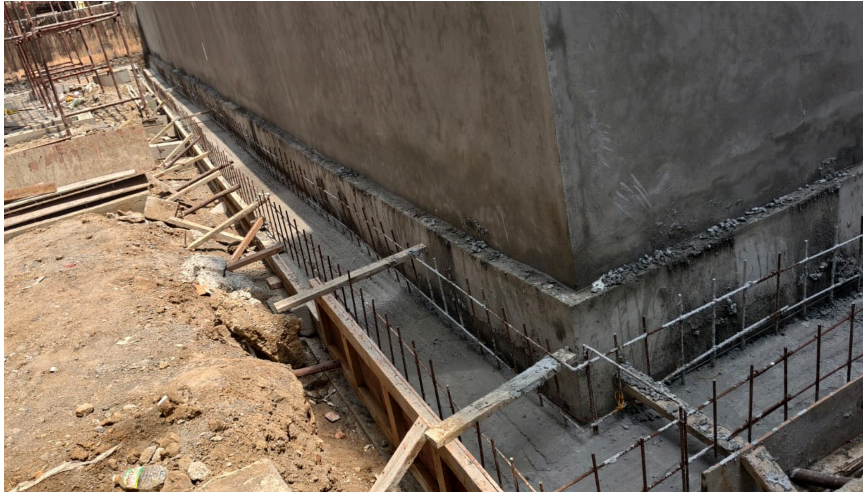
Storm Water Drain Raft Concrete Work Nearing Completion.
