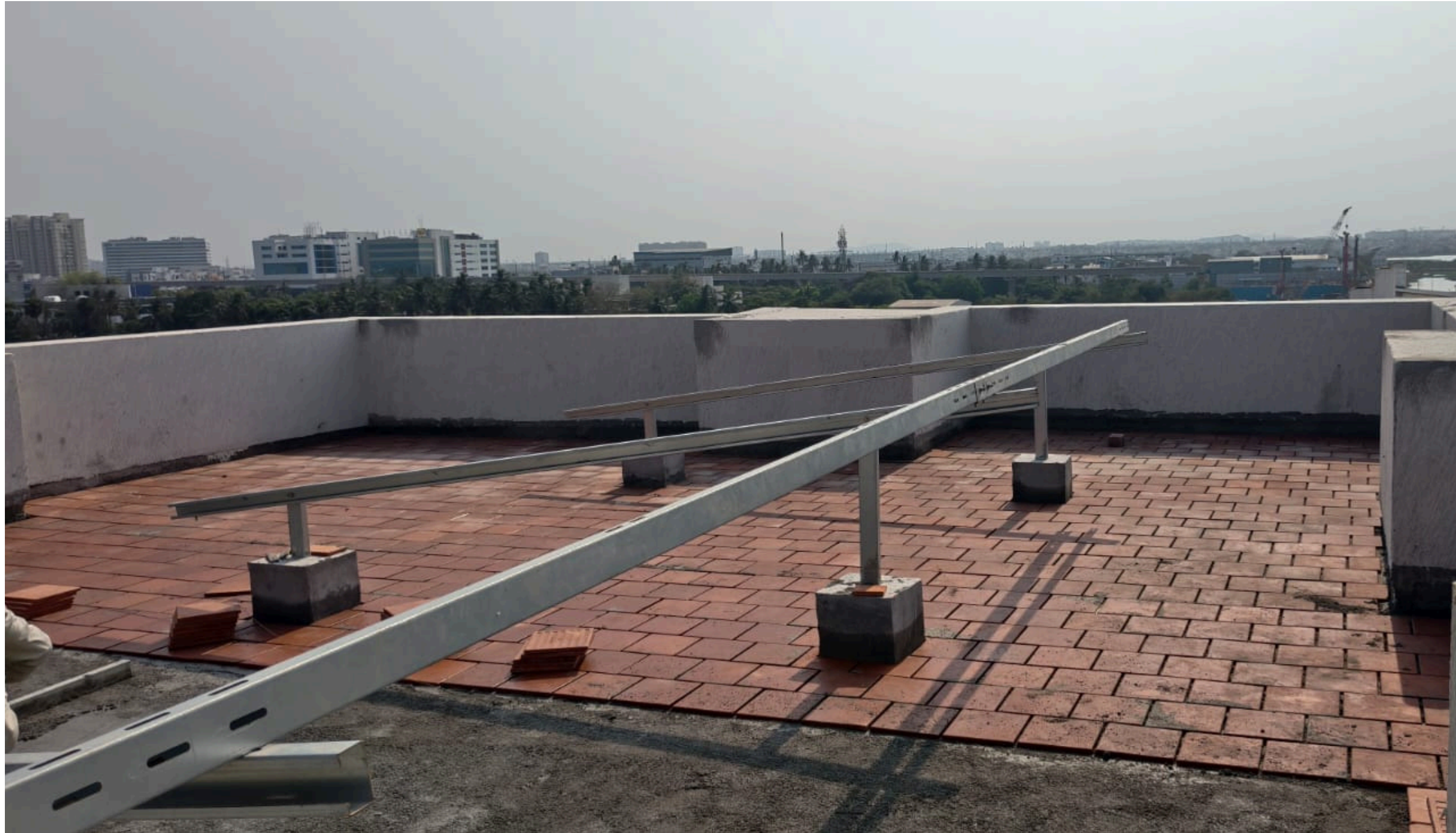
Main Building Terrace Press Tiles Work In Progress.
