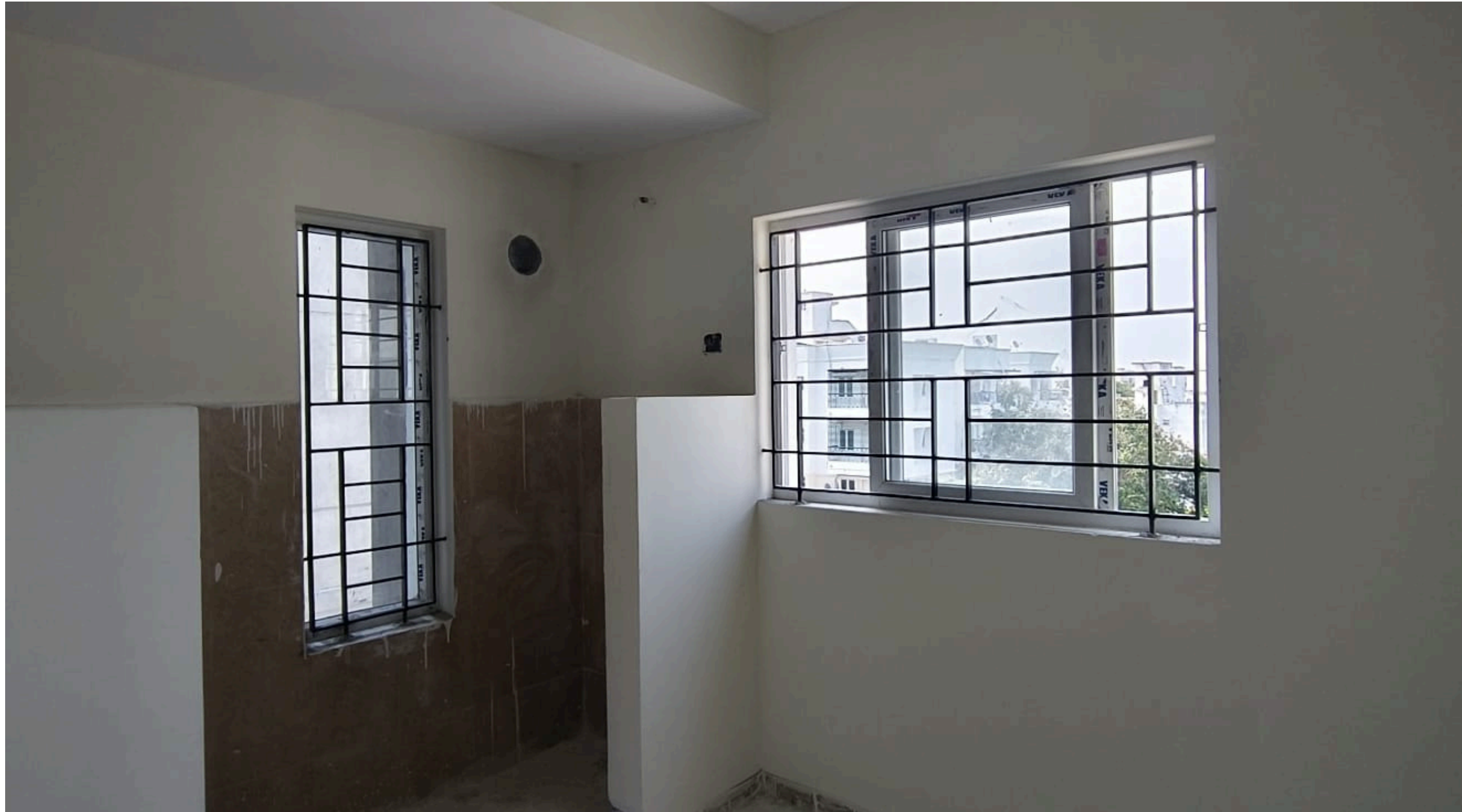
Main Building Pour-1 Window Fixing Work In Progress.
