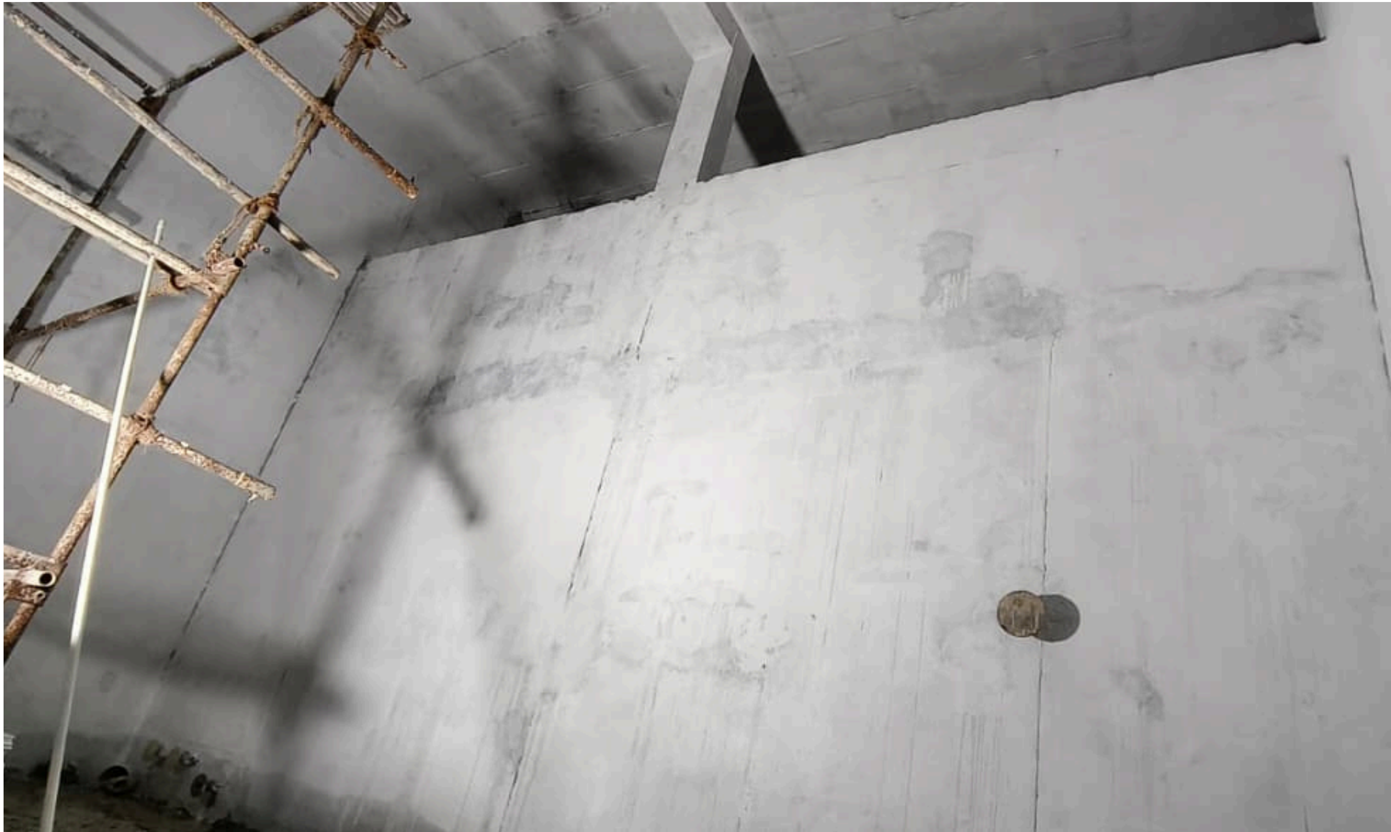
STP Pump Room Primer Work Completed.
