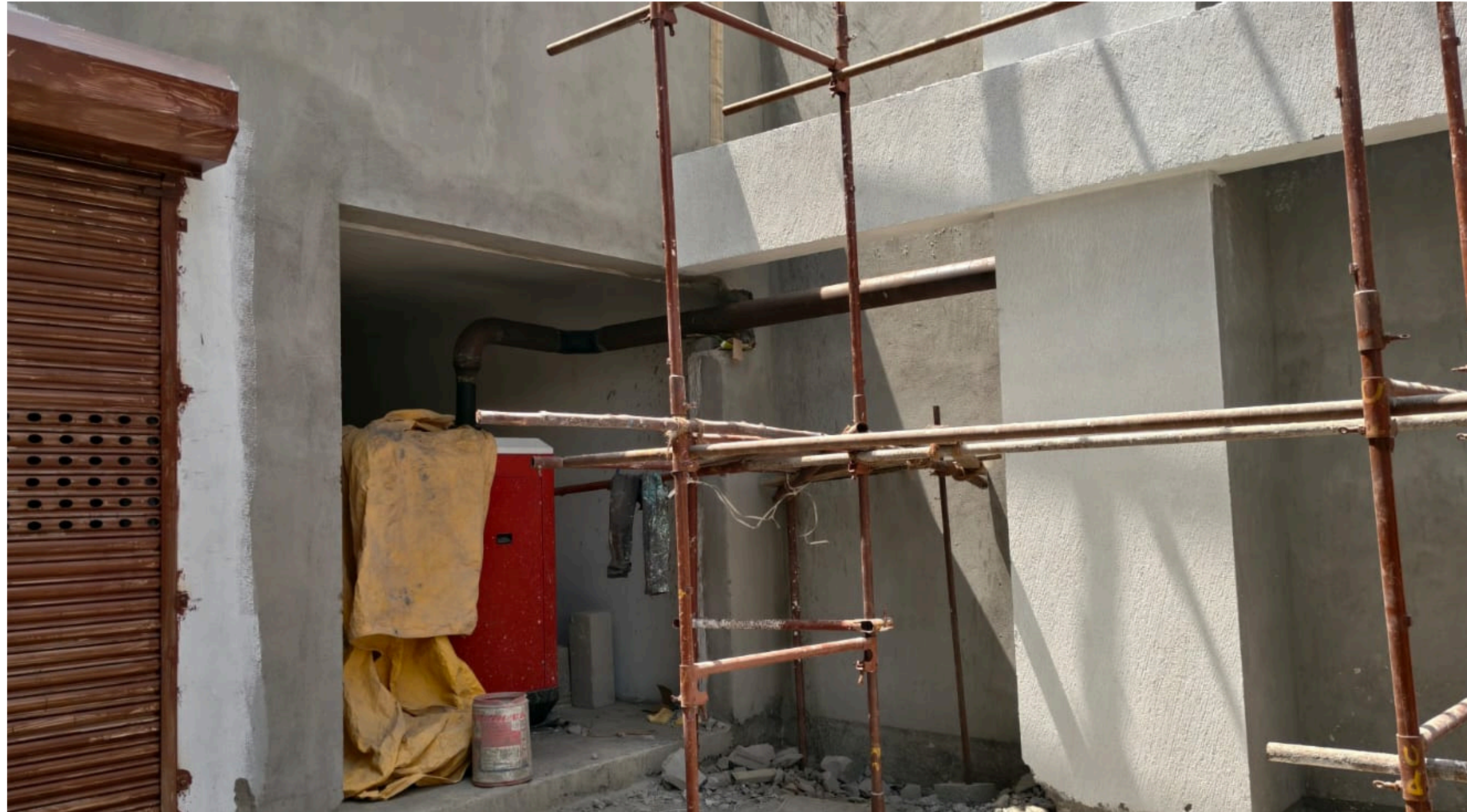
DG Exhaust Pipe Fixing Work In Progress.
