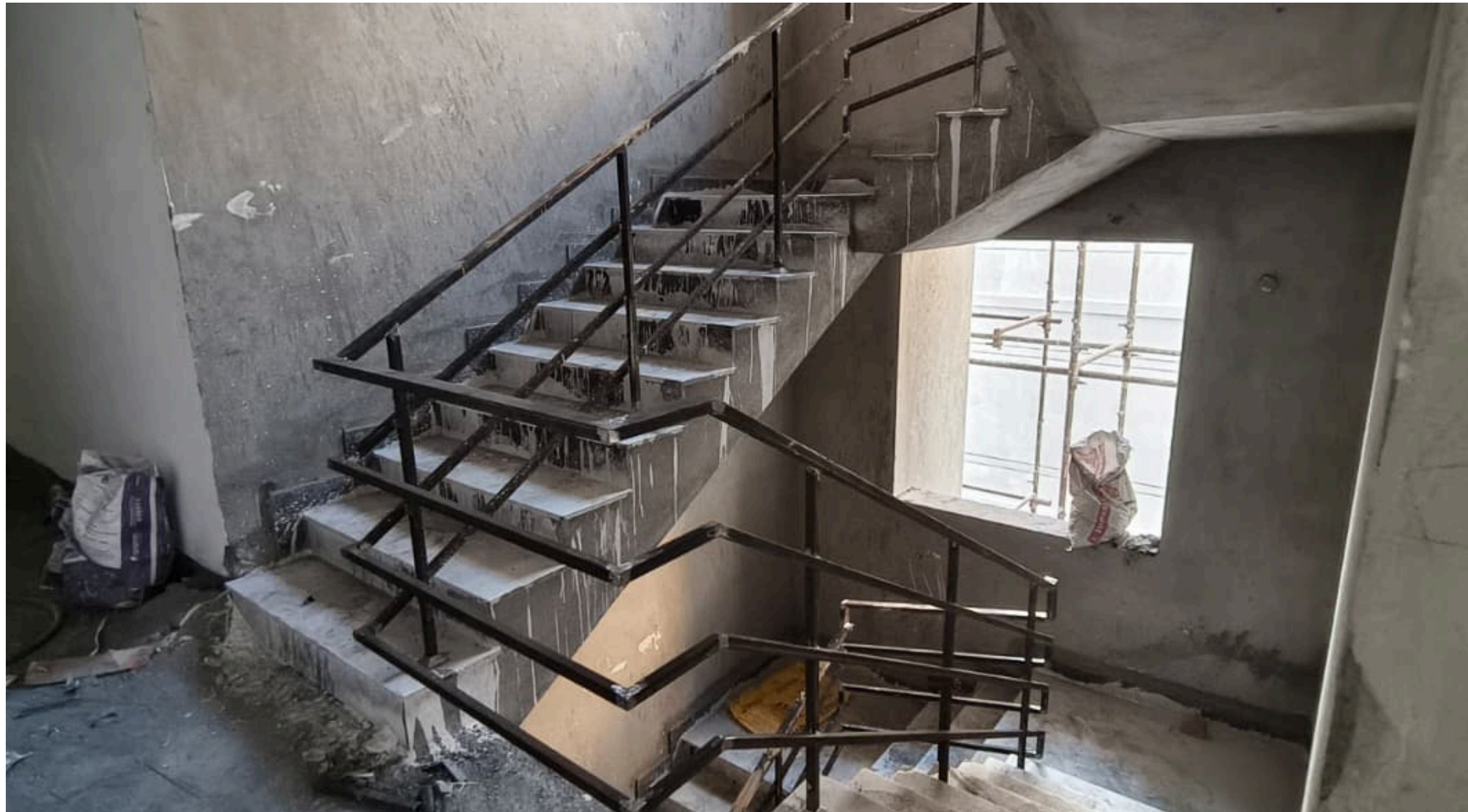
Main Building Pour-1 Staircase Handrail Fixing Work Nearing Completed.
