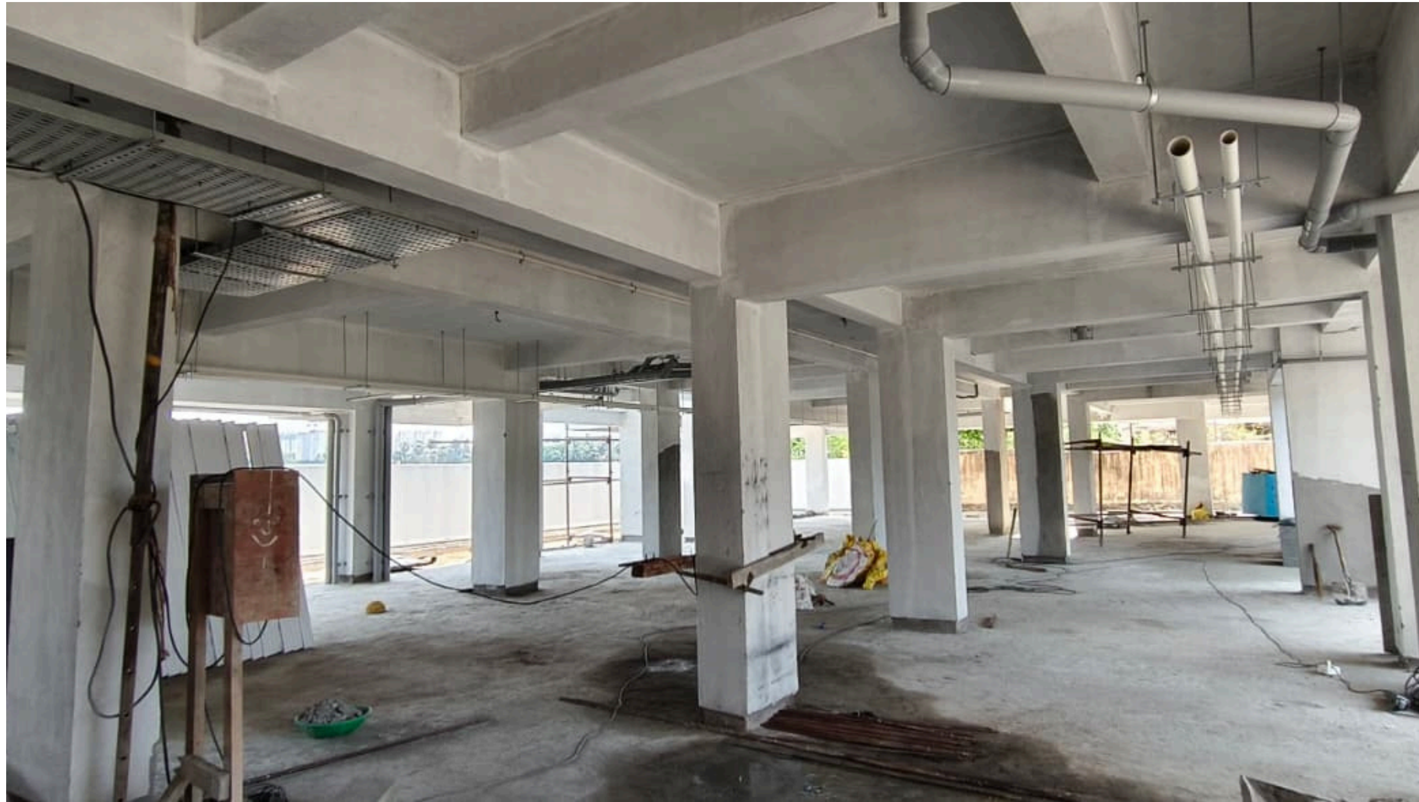
Main Building Pour-1 Stilt Floor Plumbing Work Nearing Completion.
