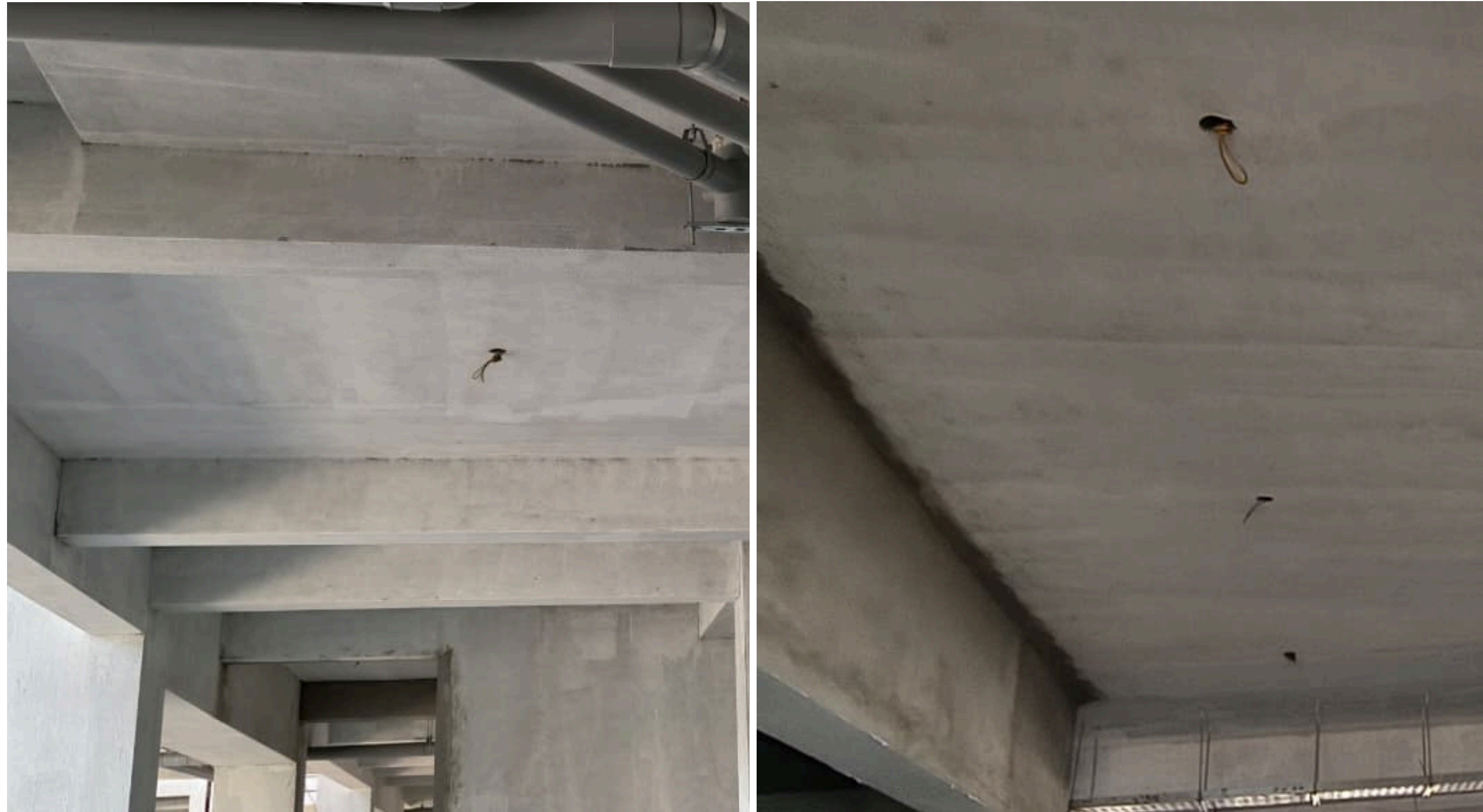
Main Building Stilt Floor Electrical Wiring Work Nearing Completion.
