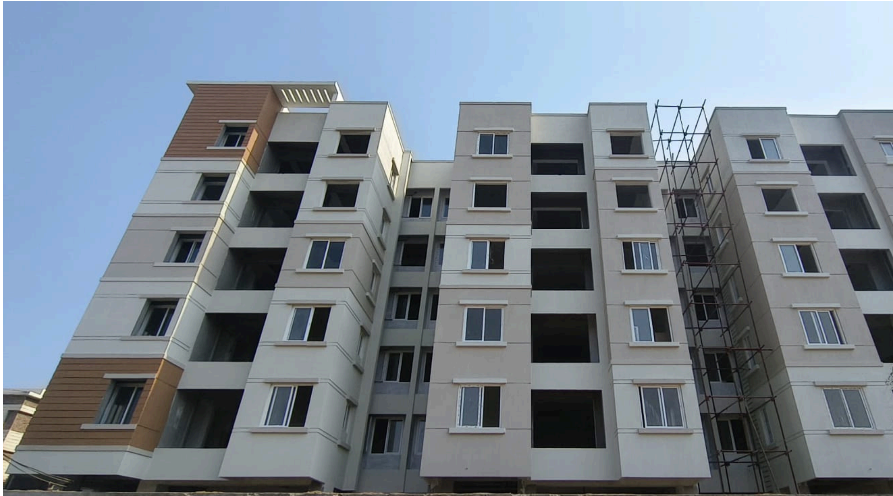
Main Building Pour-2 Window Fixing Work In Progress.
