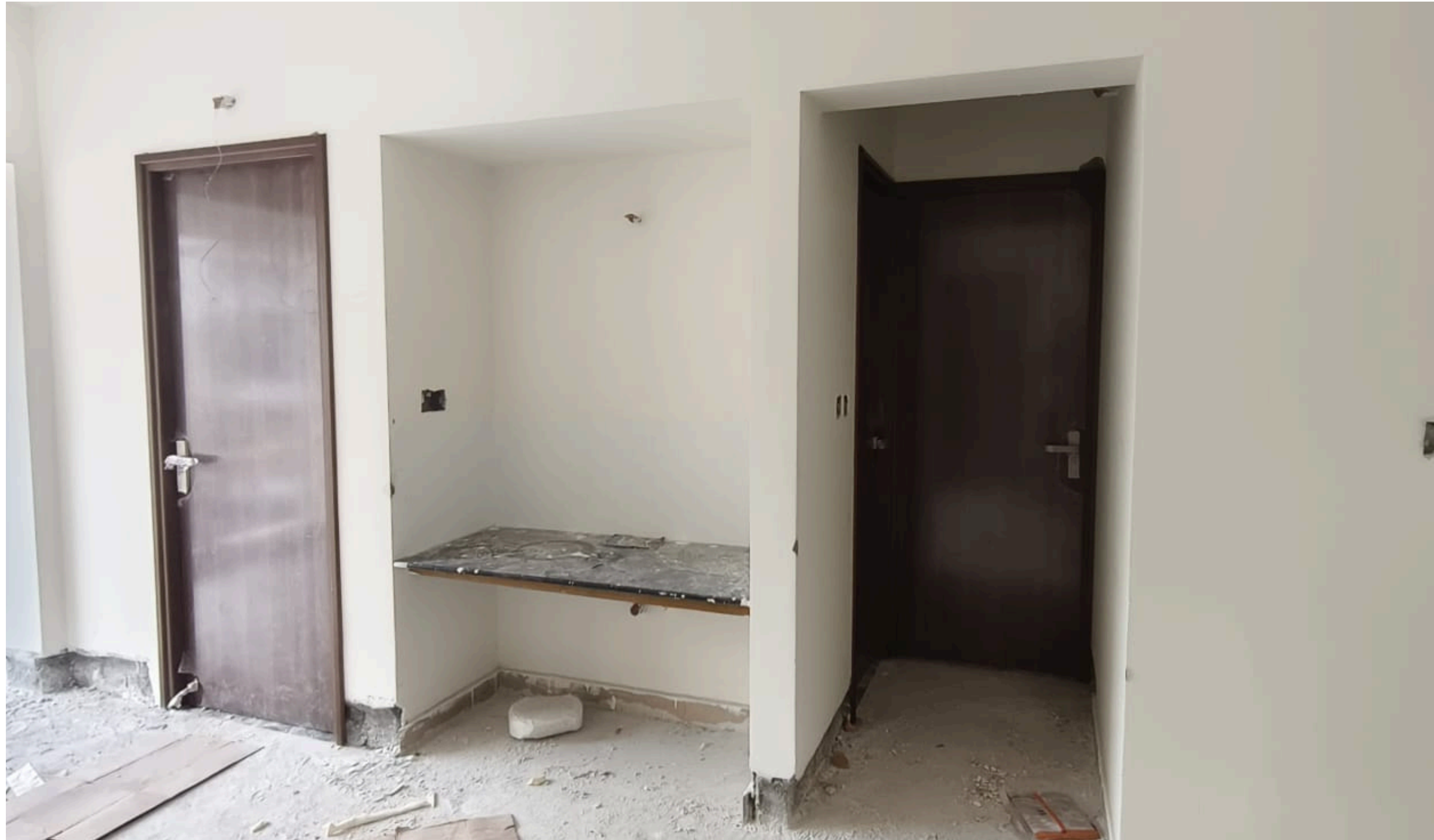
Main Building Pour-1 2 nd Floor Flat Door Fixing Work Completed.
