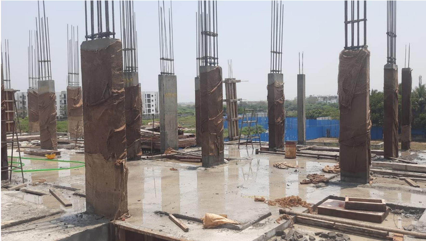
Main Building 2 nd Floor Pour-1 Column Concrete Work Completed.
