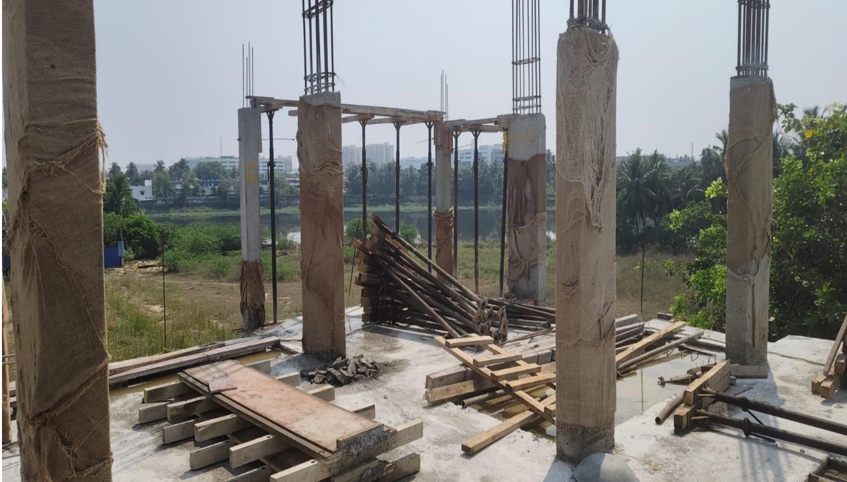
Main Building 2 nd Floor Pour-1 Roof Slab Shuttering Work Commenced.
