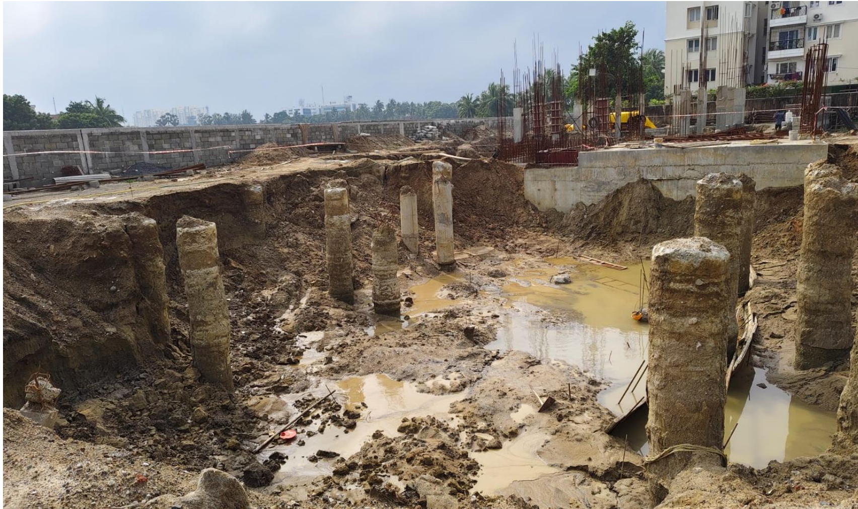
UG Sump Earth Work Excavation Work Nearing Completion.
