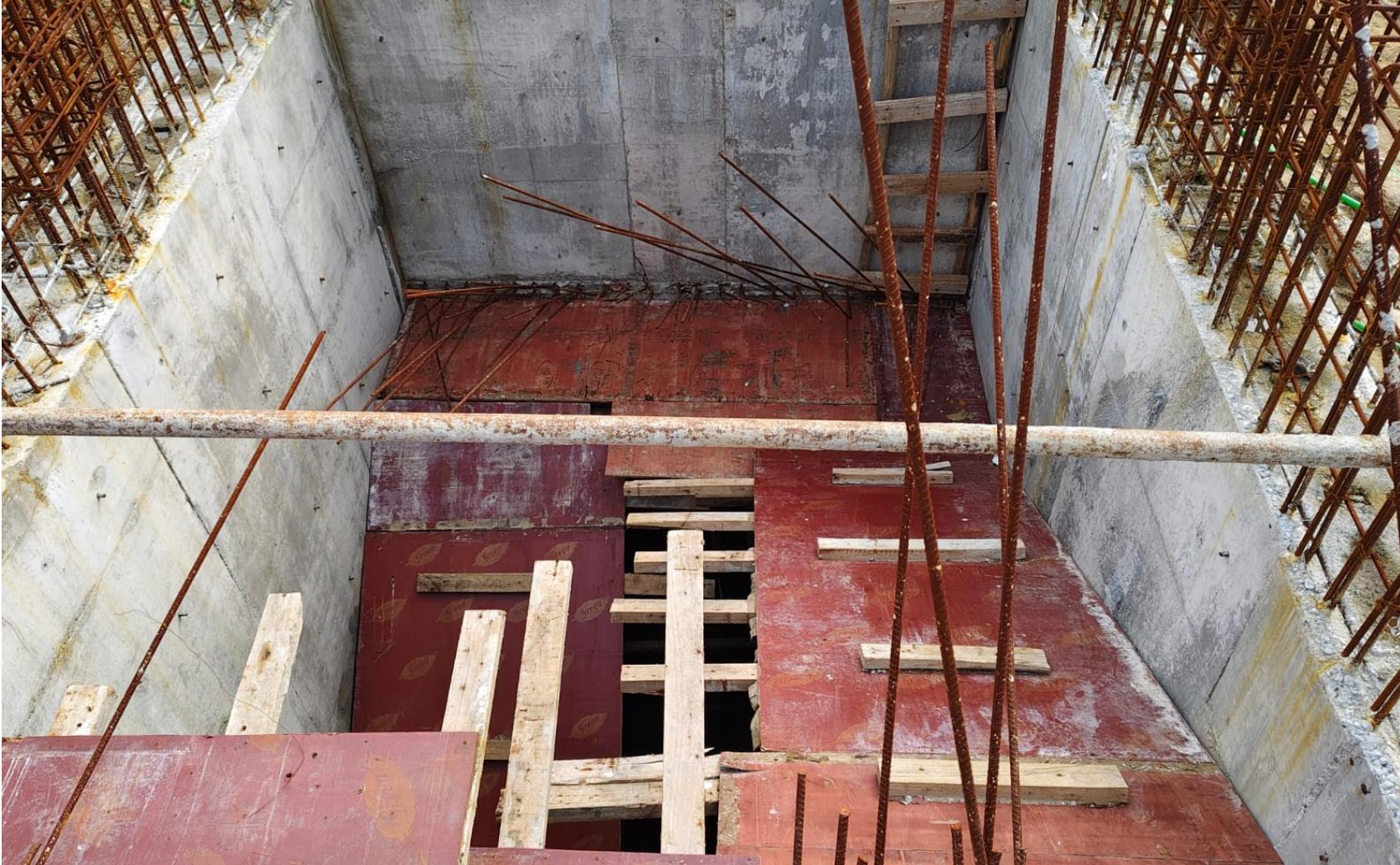
STP Staircase Shuttering work in progress.
