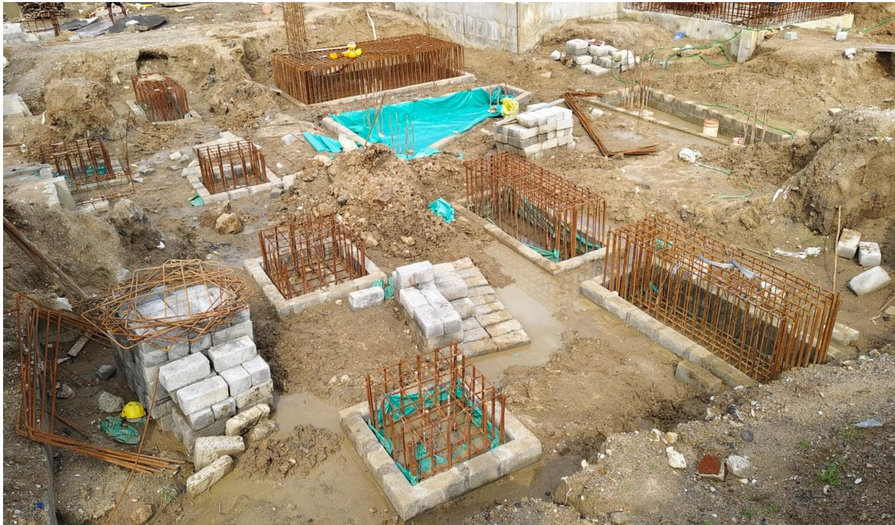
Main Building Pile Cap Reinforcement work in progress.
