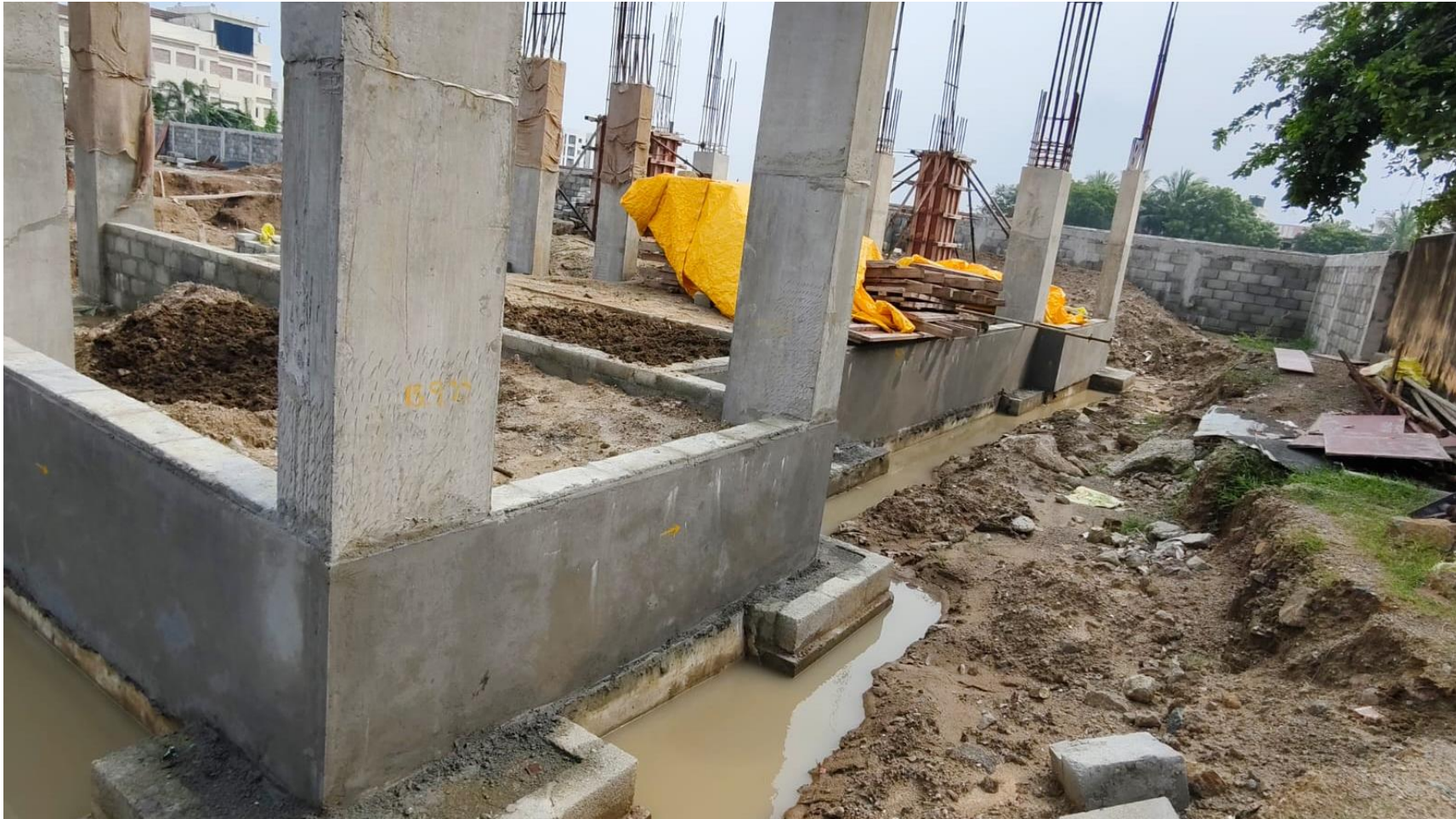
Main Building Below stilt floor blockwork Plastering work in progress.
