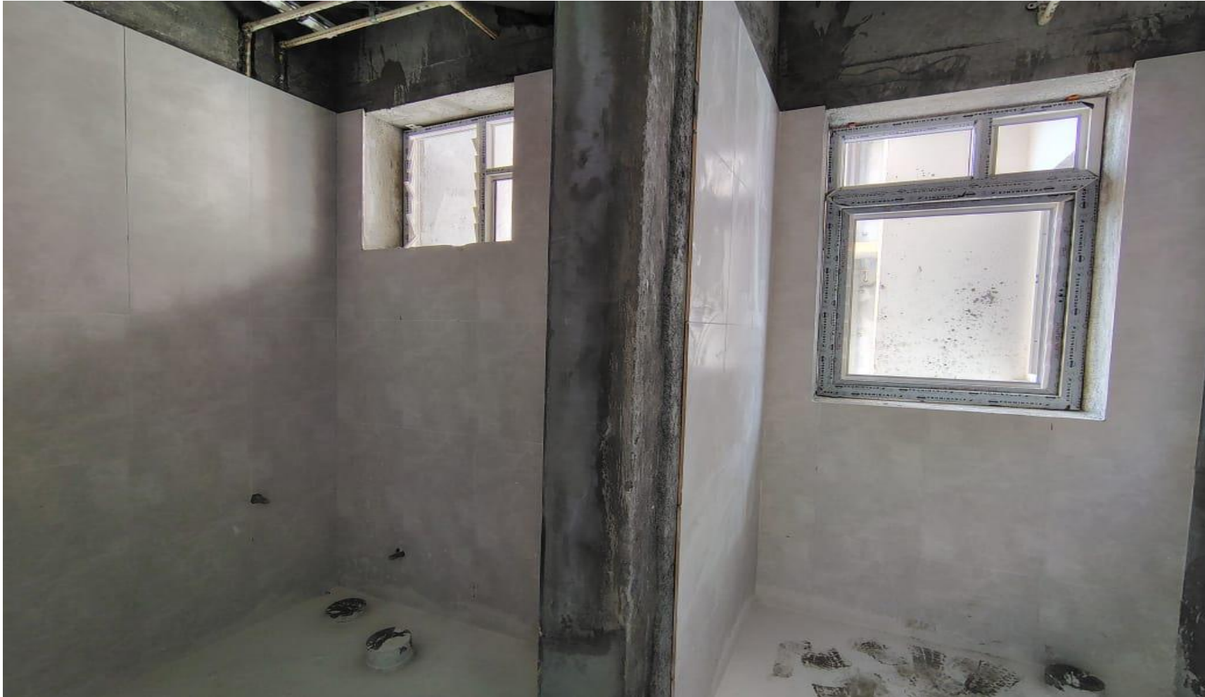
Wing 4A, Common Toilet – Tile Work in Progress
