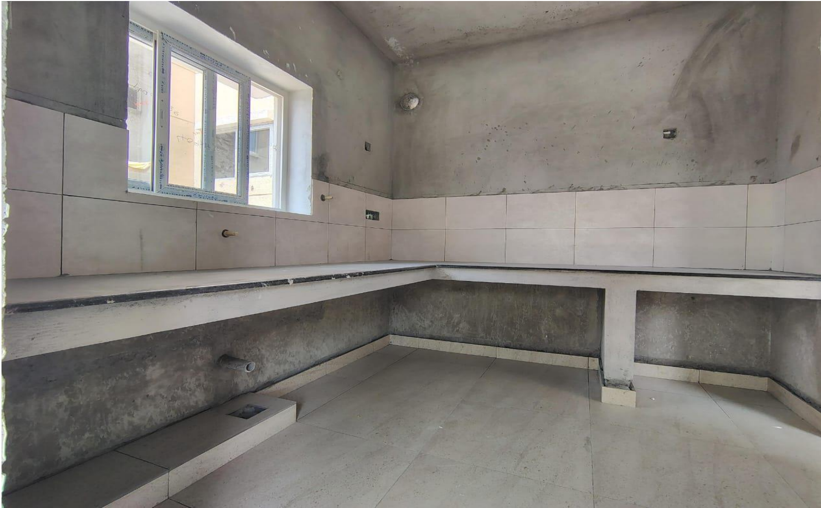
Wing 4B , Kitchen – Tile Dado works in Progress
