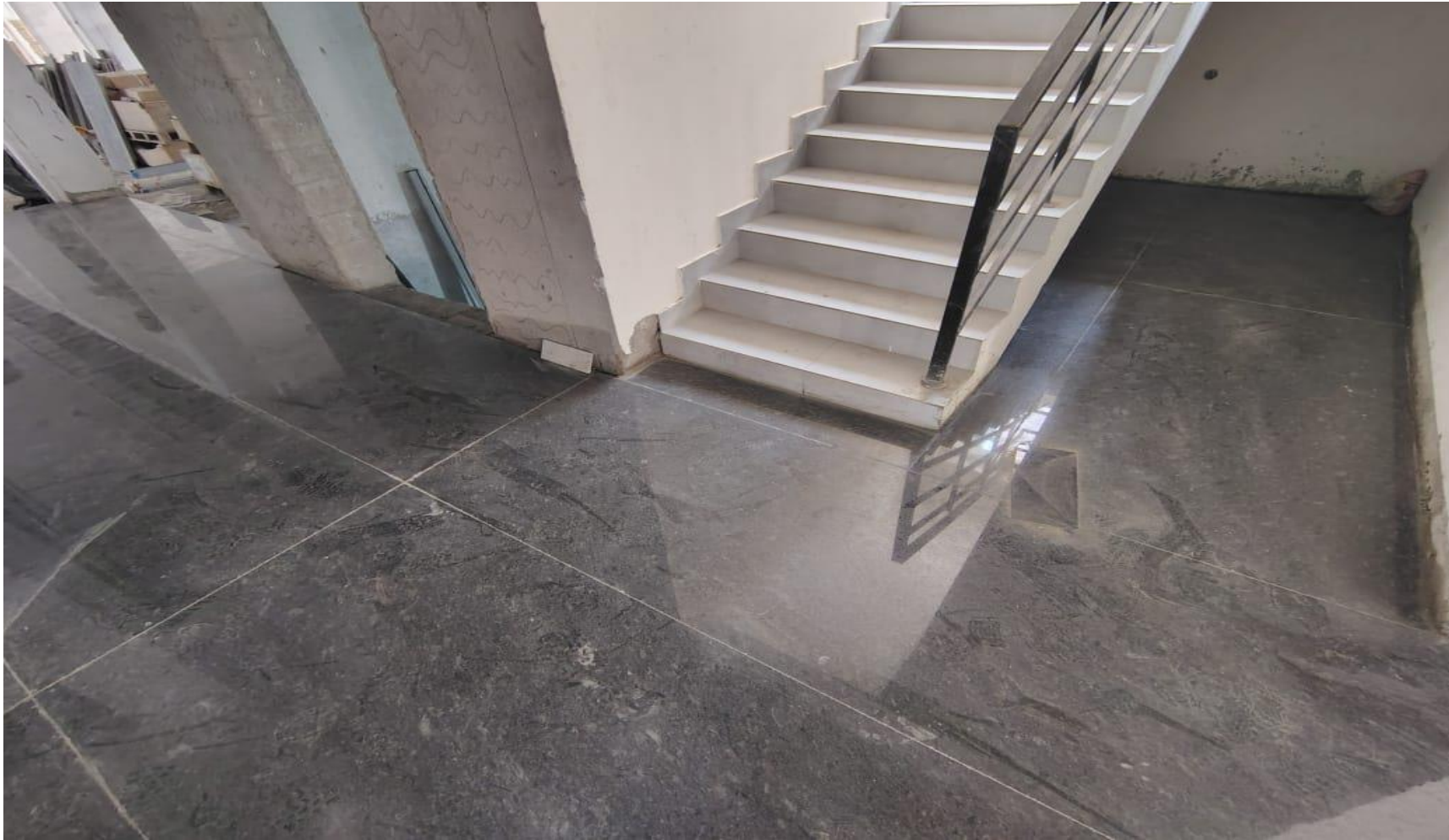
Wing 3A, Stilt Floor – Lobby Granite Works in Progress
