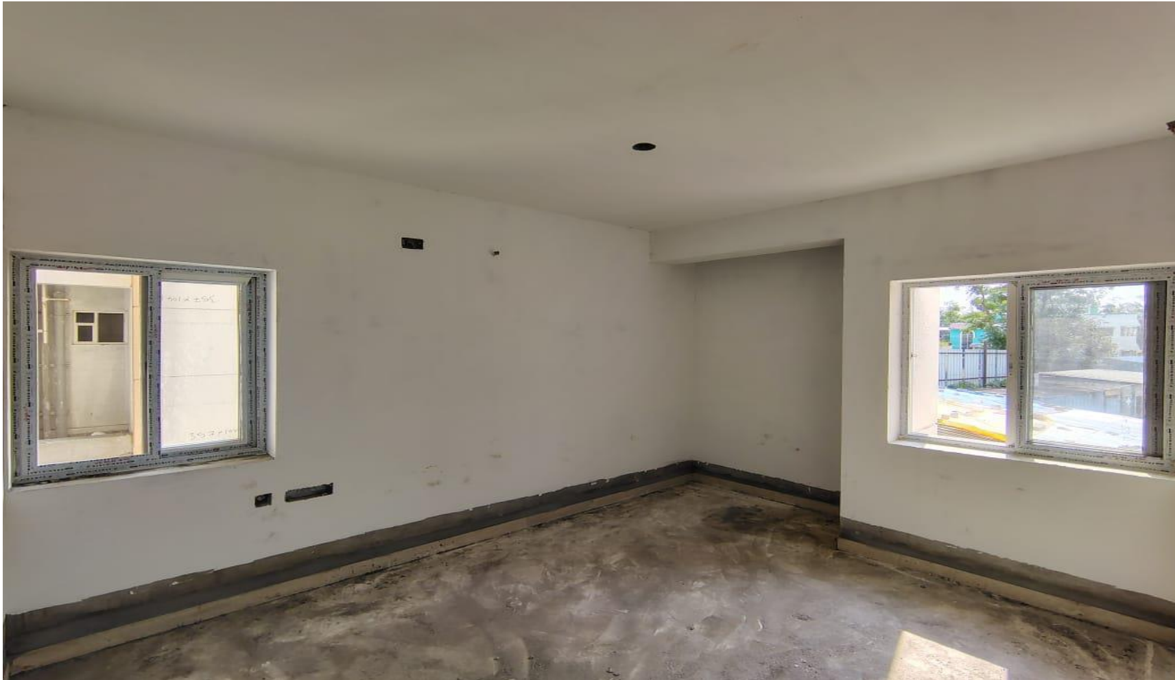
Wing 4A & 4B – Putty Work in Progress
