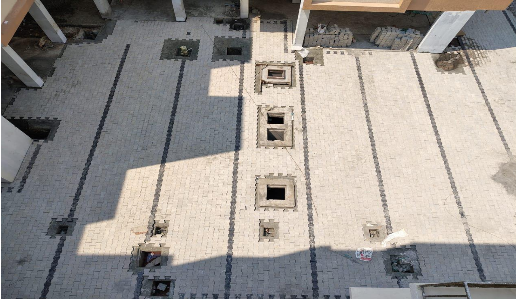
Wing 3B & 3C, External – Paver works in progress
