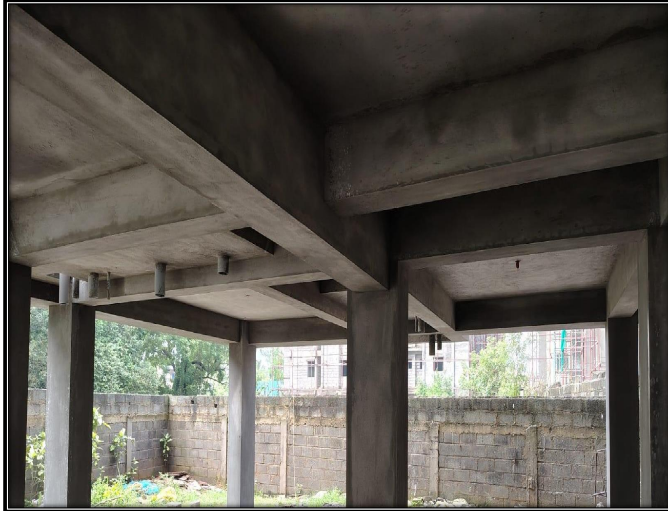
Wing 3D & 3E, Stilt Floor – Ceiling & Column Plastering works in Progress
