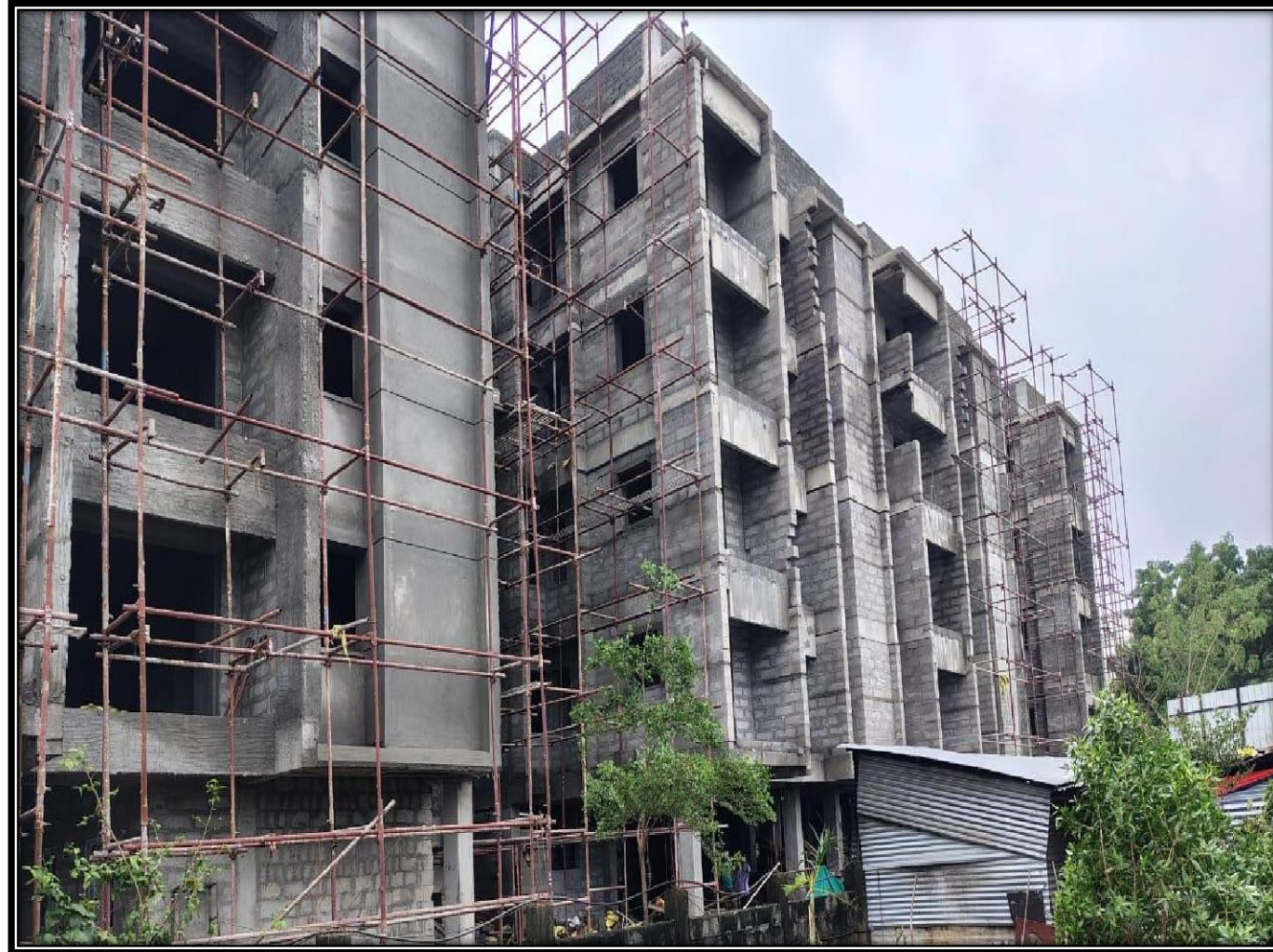
Wing 4A & 4B – West Side Plastering Work in Progress
